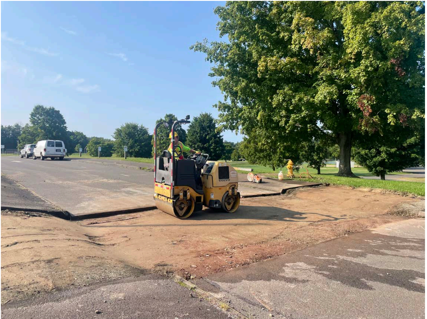
Picture 5: Ludlow compacting the underlying fill on the footprint of a trench overcut located on the access road on the west side of the CRHS. View to the southwest.
