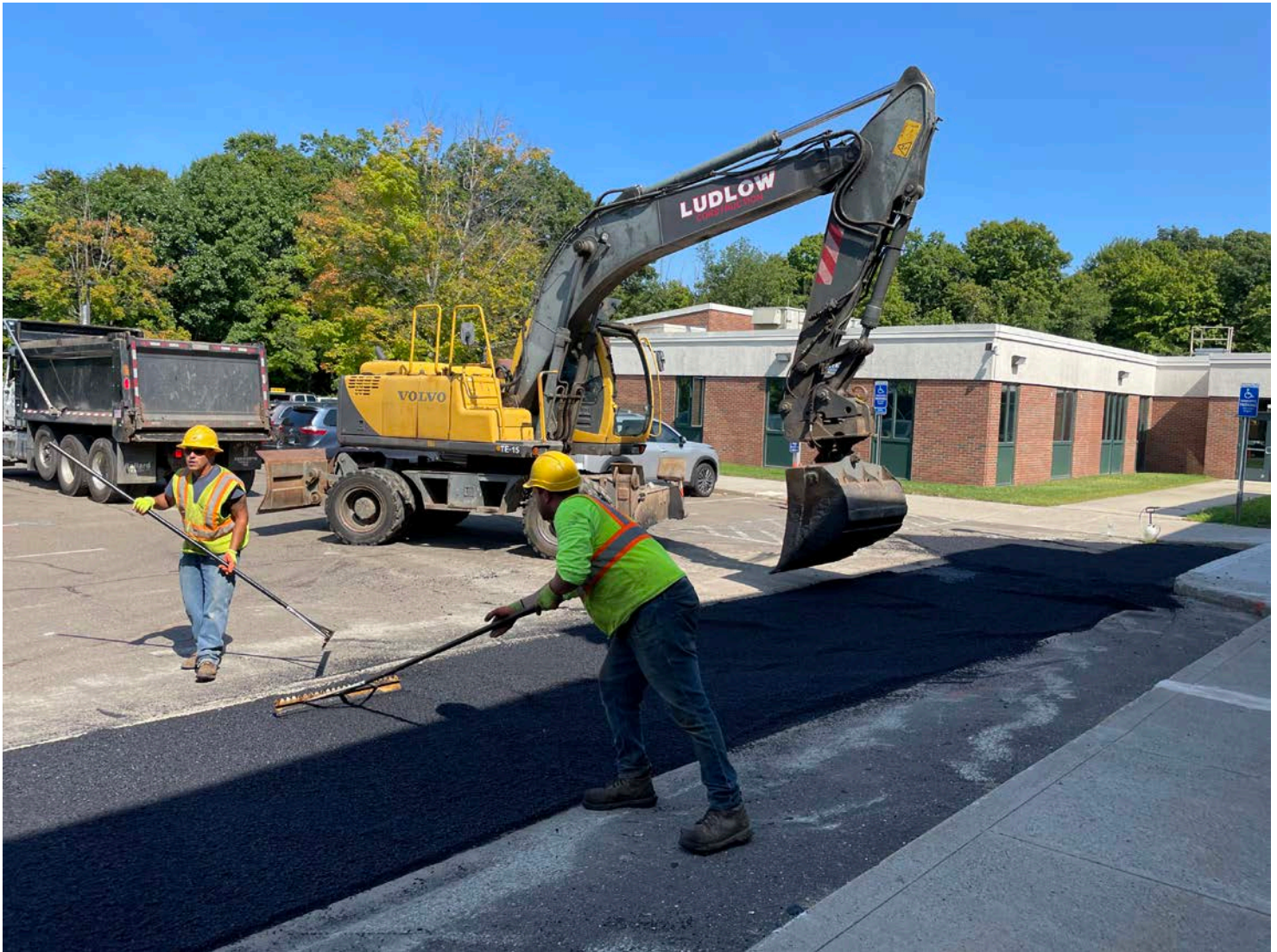
Picture 12: Ludlow grading the second of two lifts of asphalt on the footprint of a trench overcut located on the north side of the CRHS. View to the northeast.
