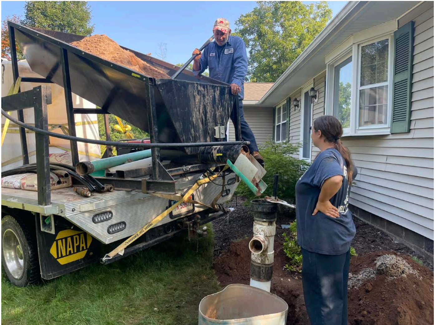
Picture 4: Grela placing sand into the well located on the southwest corner of the 175R Main Street, Durham, residence as part of well decommissioning activities. View to the north.
