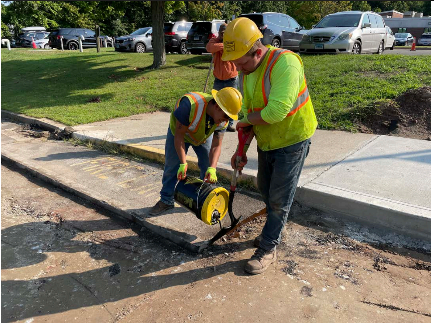
Picture 6: Ludlow placing tack coat on the cut edges of pavement on the footprint of a trench overcut on the west side of the CRHS. View to the southwest. View to the northeast.
