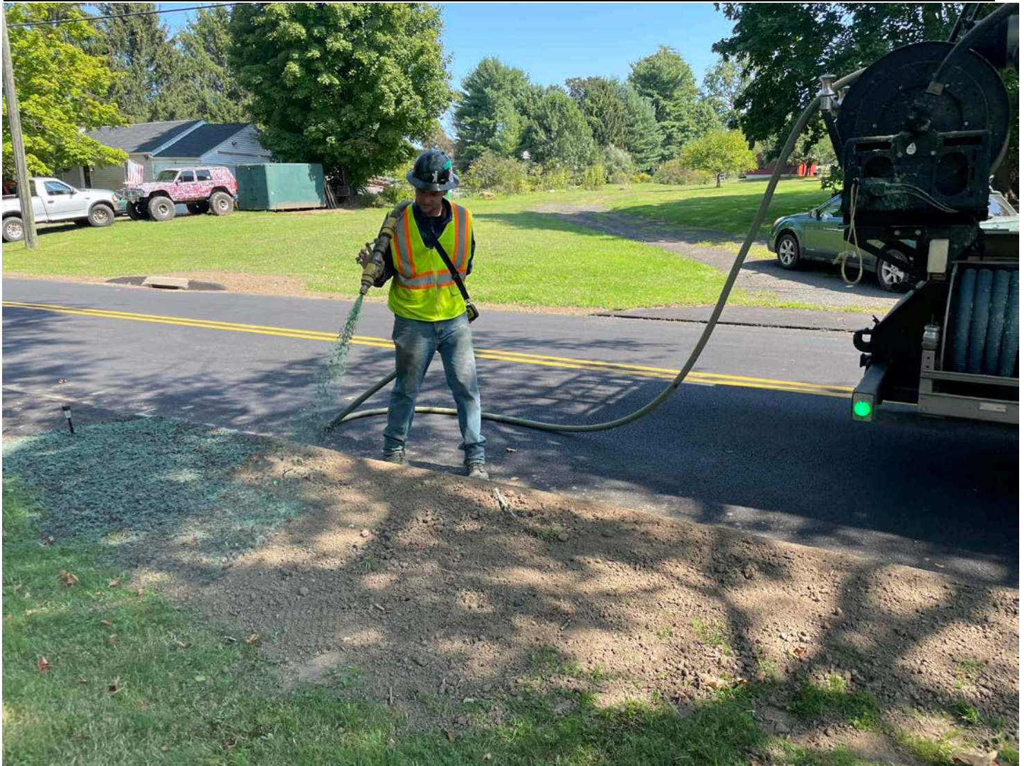
Picture 9: Laydon hydroseeding along the west side of Maple Avenue, Durham, at the 184 Maple Avenue property. View to the northeast.
