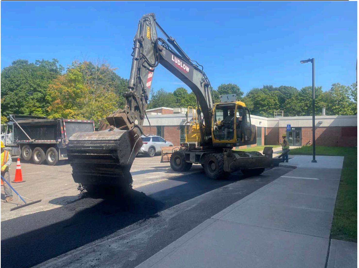
Picture 11: Ludlow placing the second of two lifts of asphalt on the footprint of a trench overcut located on the north side of the CRHS. View to the northeast.
