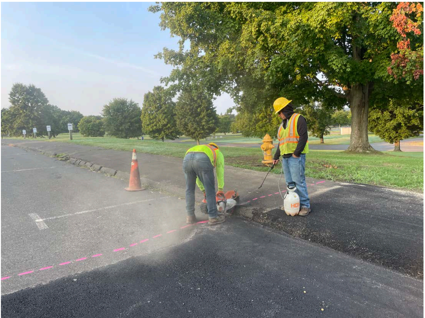
Picture 1: Ludlow saw-cutting the footprint of a trench overcut on the access road located on the west side of the CRHS. View to the southwest.
