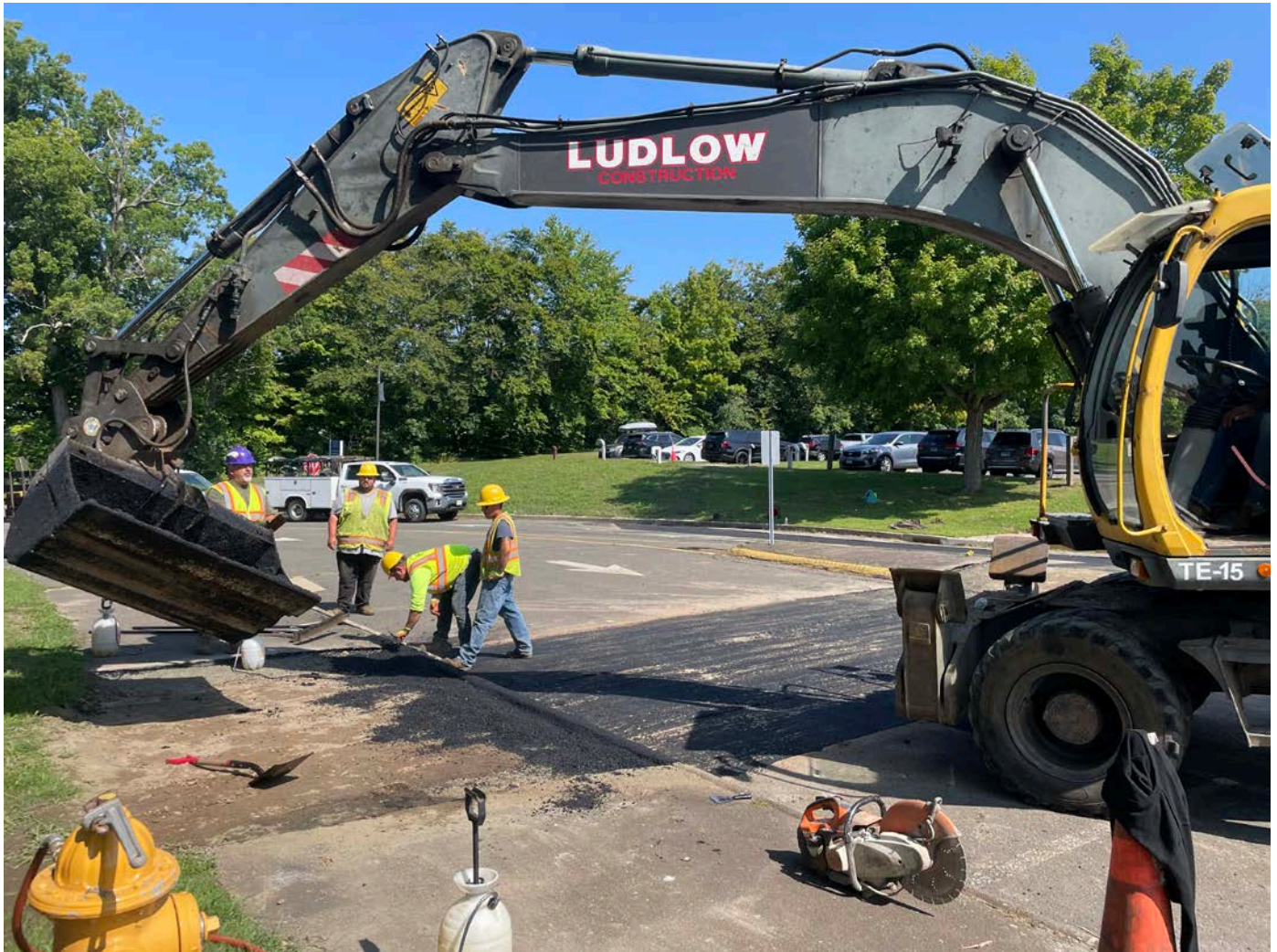
Picture 7: Ludlow placing asphalt on the west side of the access road located on the west side of the CHHS. View to the northeast.
