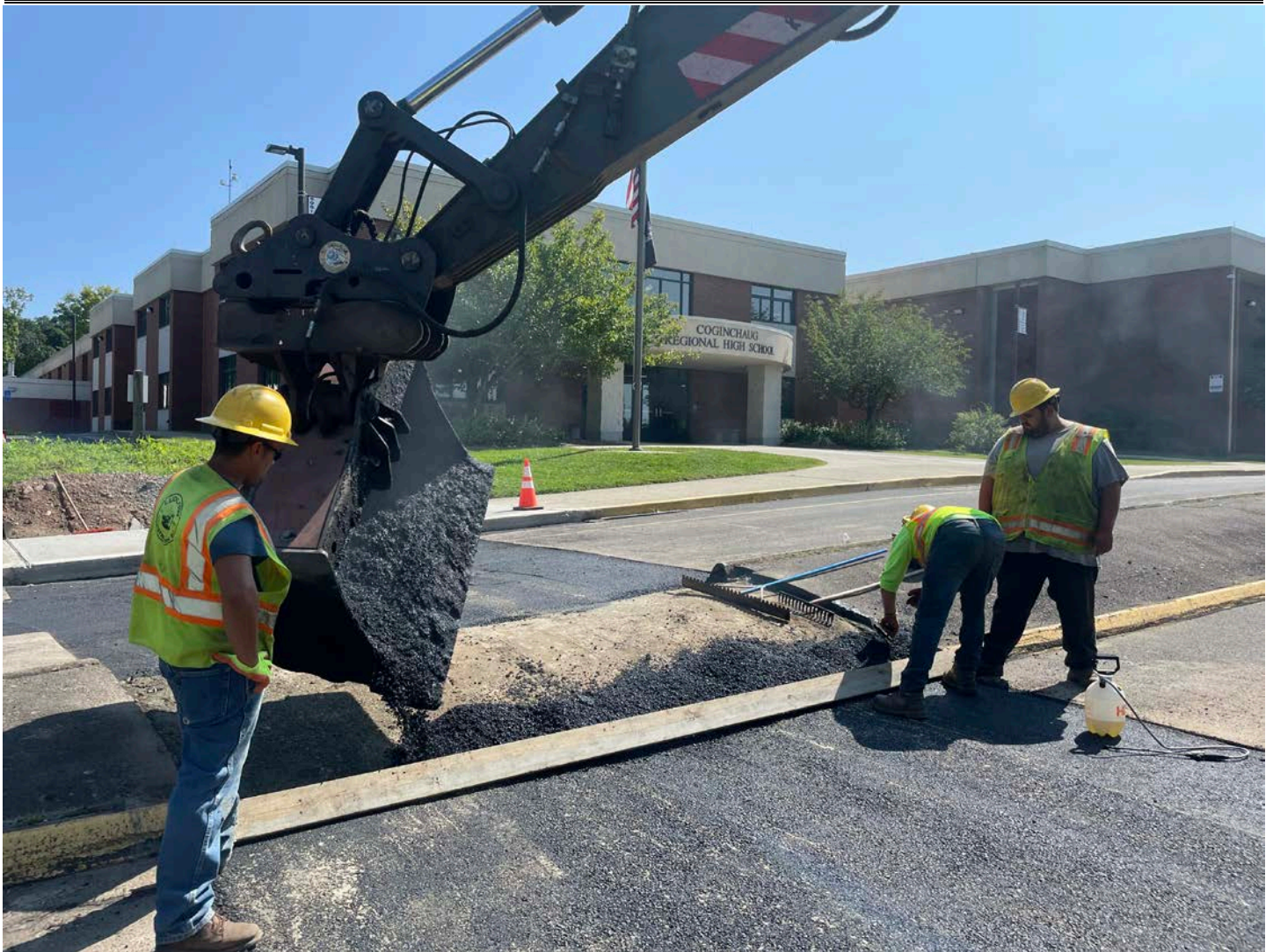
Picture 8: Ludlow placing asphalt on the median strip located between the two lanes of the access road located on the west side of the CRHS. View to the southeast.
