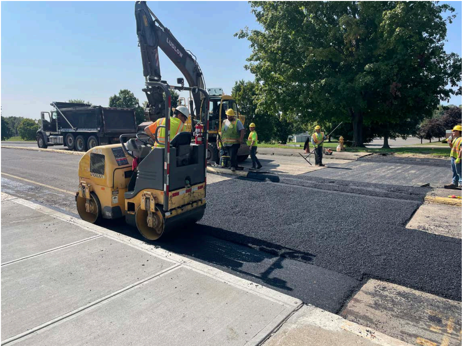
Picture 10: Ludlow placing the second of two lifts of asphalt on the footprint of a trench overcut located on the west side of the CRHS. View to the southwest.
