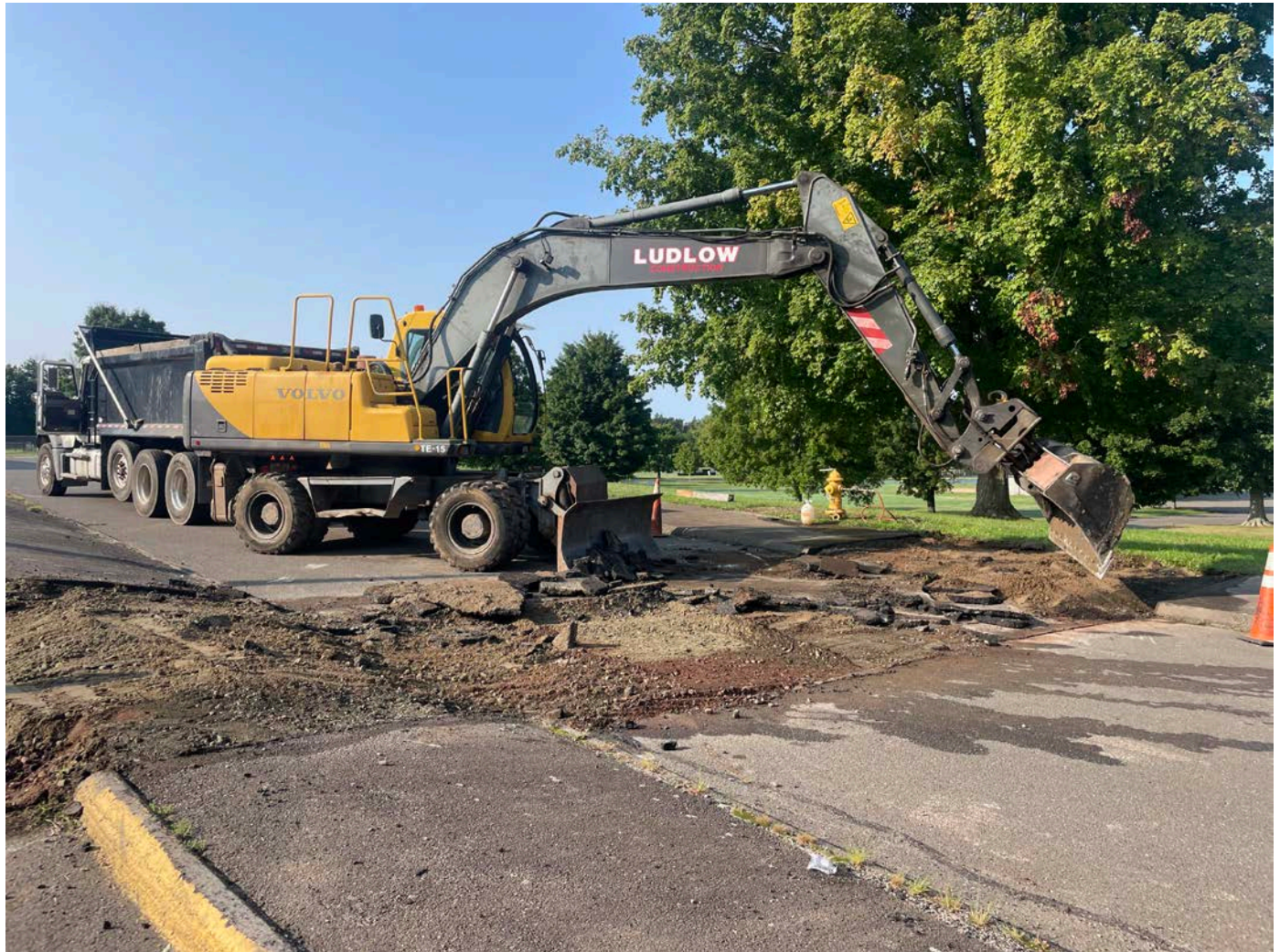
Picture 2: Ludlow removing pavement from the footprint of a trench overcut on the access road located on the west side of the CRHS. View to the southwest.
