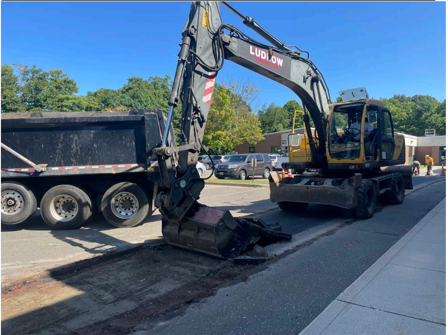
Picture 8: Ludlow stripping pavement from the footprint of a trench overcut located on the north side of the Coginchaug Regional High School as they prepare to place a permanent asphalt patch on the footprint. View to the east.
