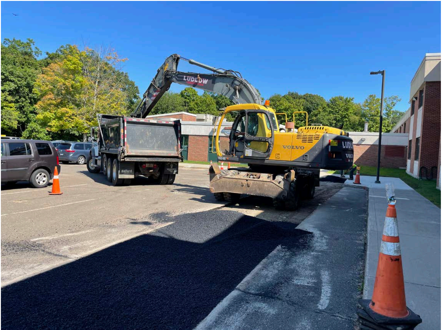
Picture 10: Ludlow placing the first lift of asphalt from the footprint of a trench overcut located on the north side of the Coginchaug Regional High School. View to the east.
