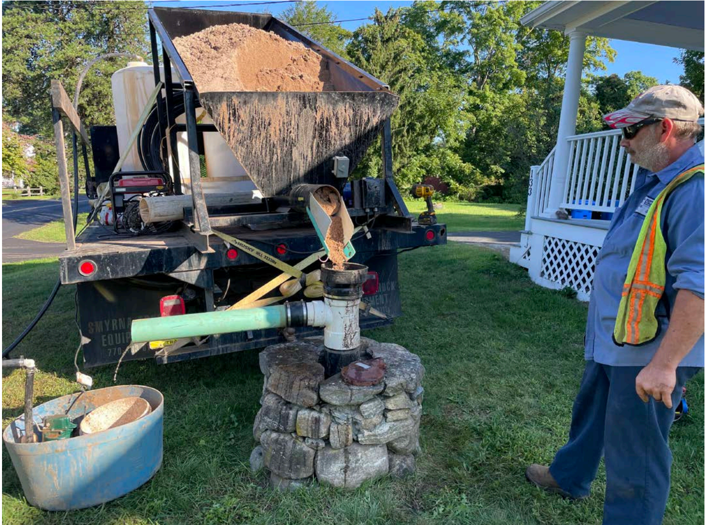
Picture 4: Grela placing sand into the well located on the west side of the 133 Maple Avenue, Durham, residence as part of well decommissioning activities. View to the south.
