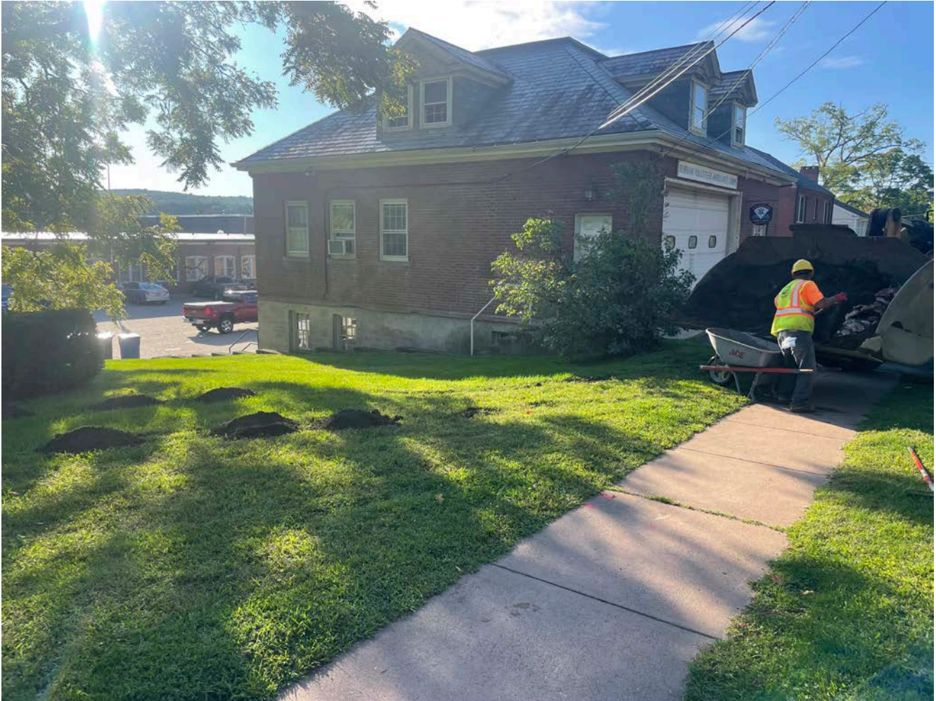
Picture 3: Ludlow placing loam on portions of the 201 Main Street, Durham, property that were disturbed during the previous installation of a meter vault. View to the southeast.
