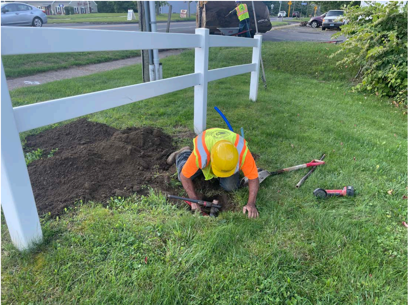
Picture 1: Ludlow cutting a blowoff line below surface grade on the 350 Main Street, Durham, property. View to the southeast.
