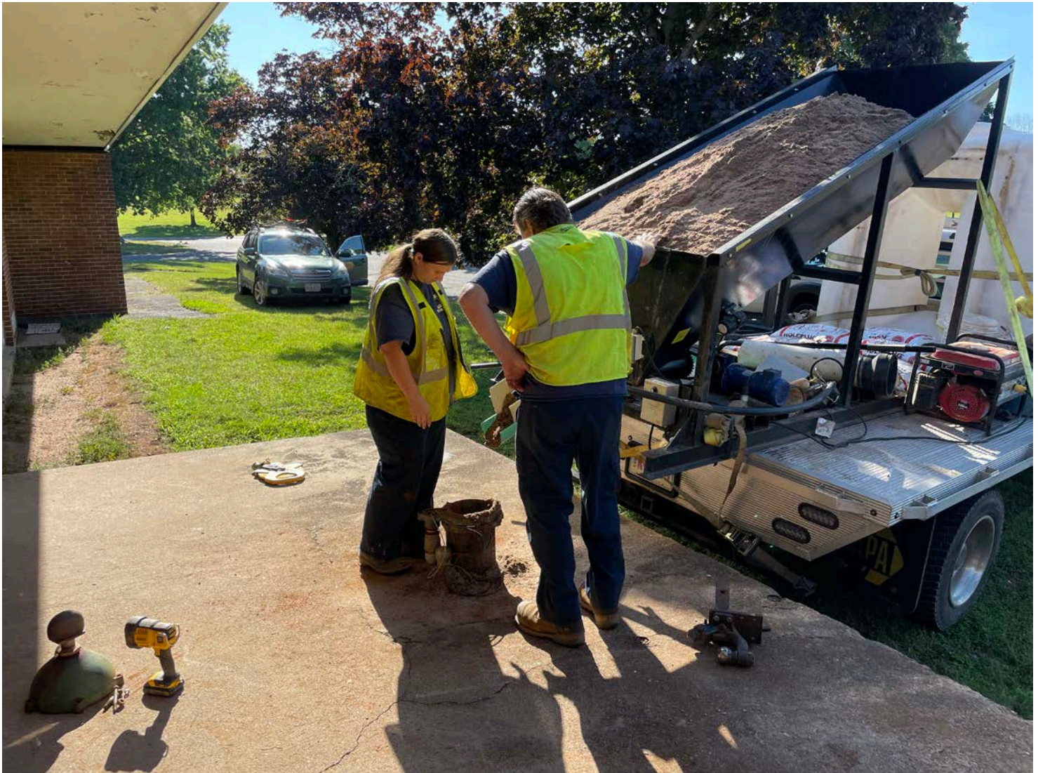
Picture 5: Grela placing sand into the well located on the south side of the Korn School located on Pickett Lane in Durham as part of well decommissioning activities. View to the east.
