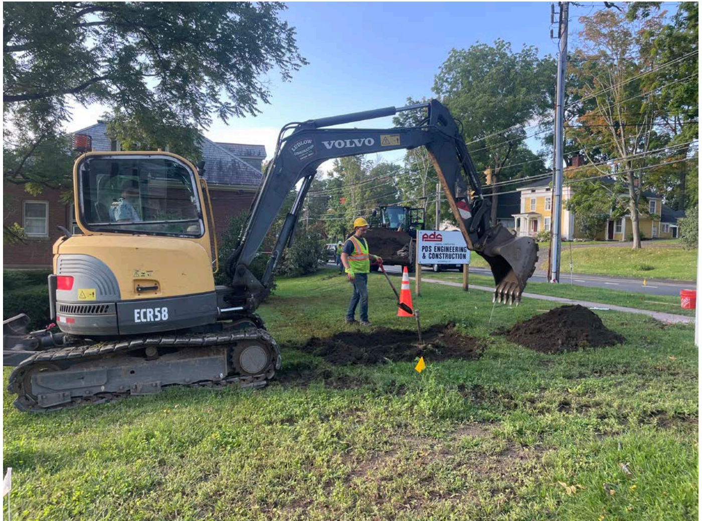
Picture 2: Ludlow excavating around a blowoff valve located on the west side of the 201 Main Street, property as they plan to cut it below surface grade. View to the southwest.
