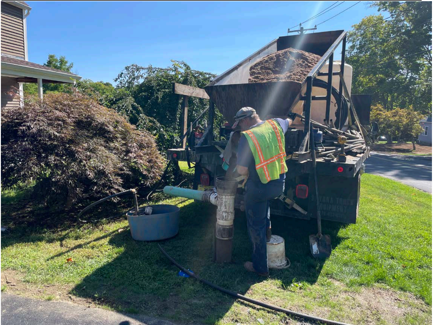
Picture 11: Grela placing sand into the well located on the west side of the 245 Maple Avenue, Durham, residence as part of well decommissioning activities. View to the southeast.
