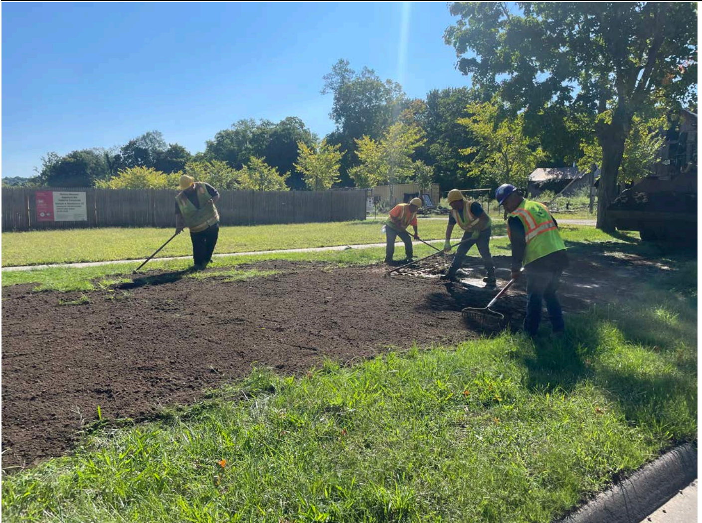
Picture 6: Ludlow grading loam they placed on the west side of the 281 Main Street, Durham, property. View to the southeast.
