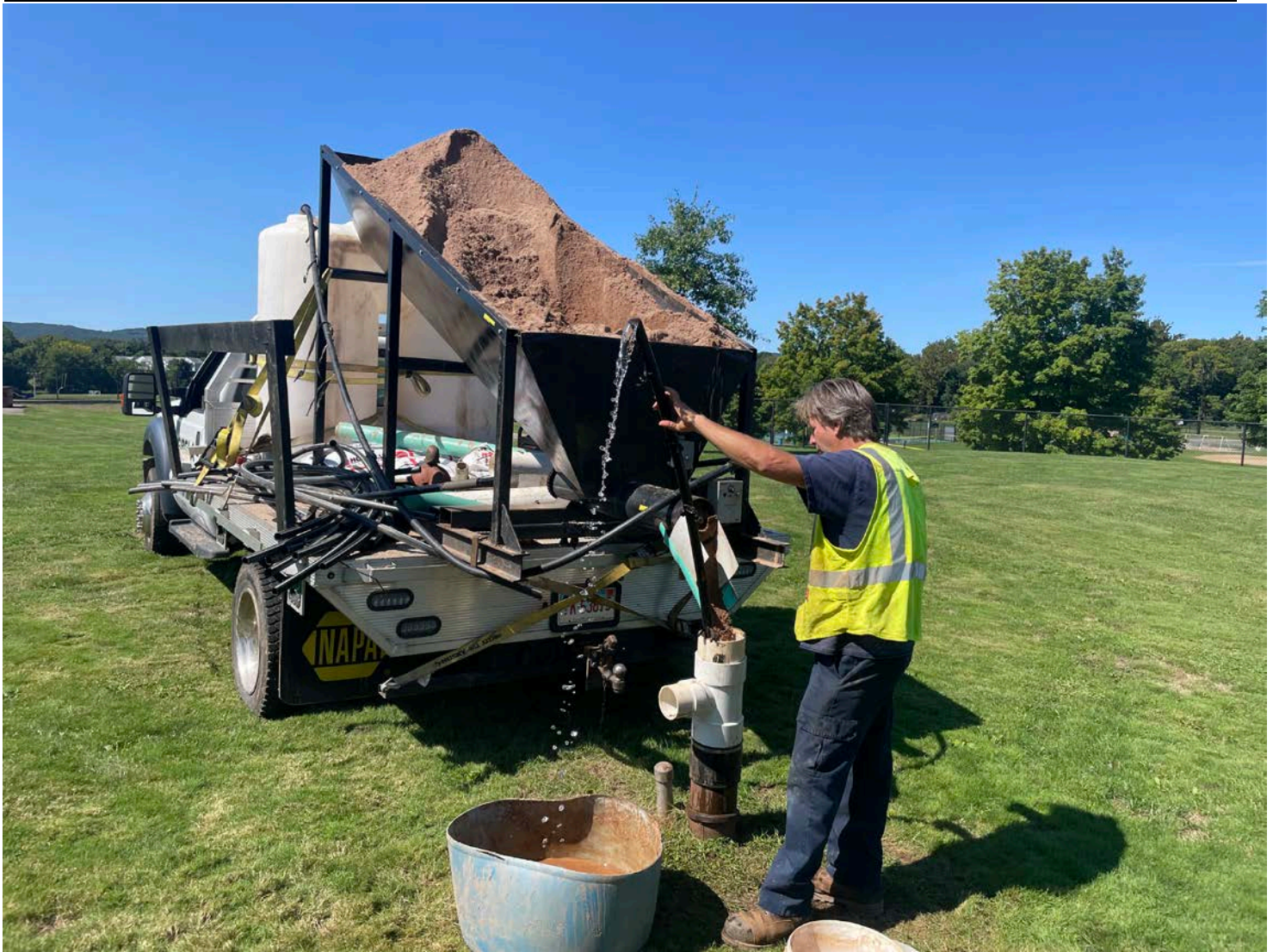
Picture 9: Grela placing sand into the well located on the west side of the Coginchaug Regional High School located south of Pickett Lane in Durham. View to the northwest.
