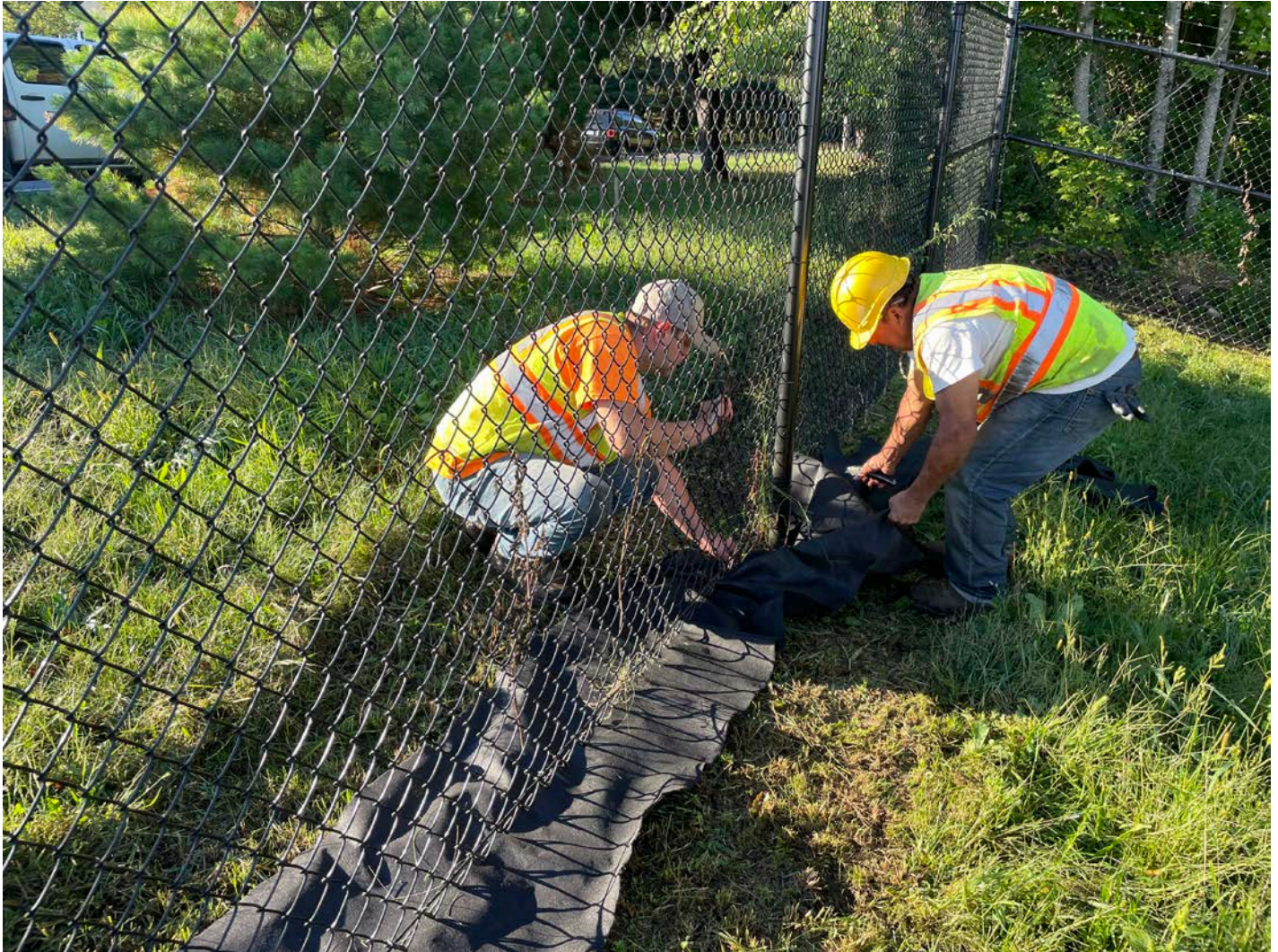
Picture 1: Ludlow placing geofabric at the base of the fence that surrounds the Booster Station located on S. Main Street in Middletown. View to the south.
