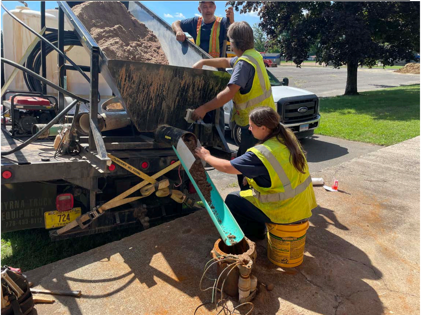
Picture 8: Grela placing sand into the well located on the south side of the Korn School located on Pickett Lane as part of well decommissioning activities. View to the southwest.
