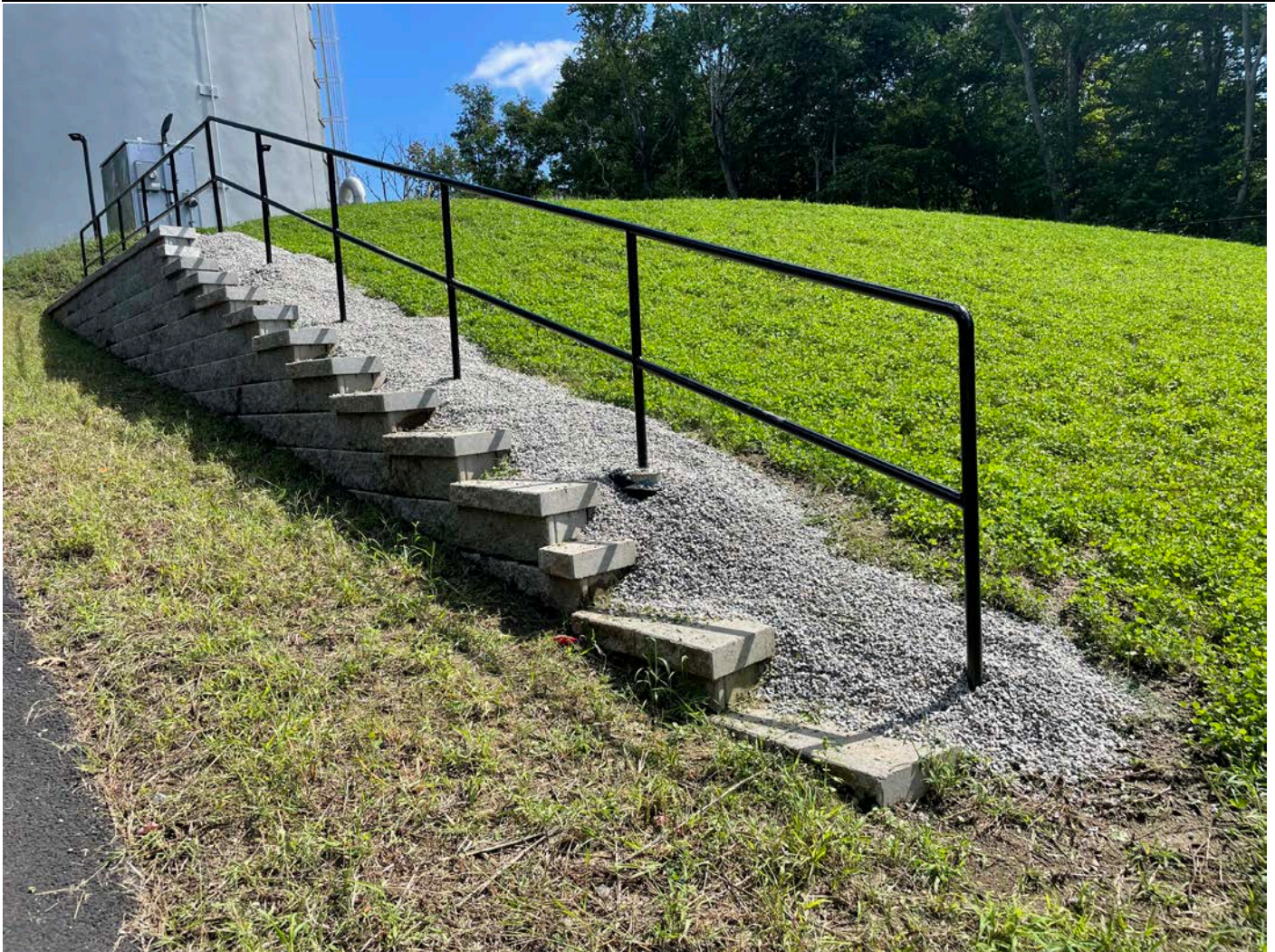
Picture 6: View of the ¾” stone that Ludlow placed at the base of the railing that was installed on the south side of the retaining wall located on the Shared Access Road in Middletown. View to the southeast.
