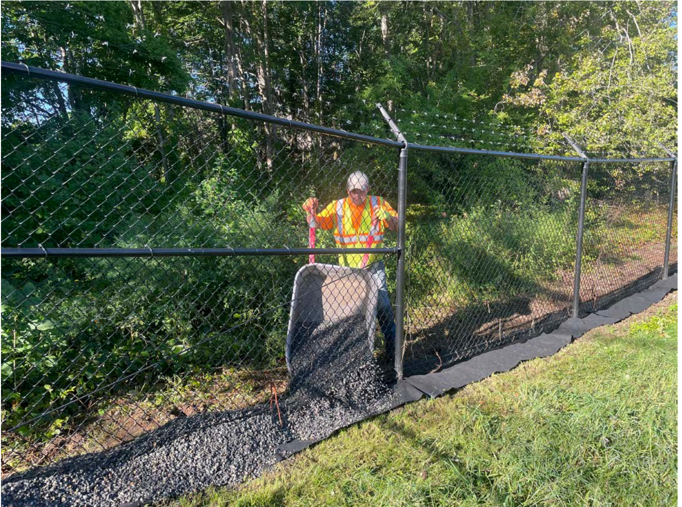
Picture 2: Ludlow placing 3/4" stone on top of the geofabric they placed at the base of the fence that surrounds the Booster Station located on S. Main Street in Middletown. View to the southwest.
