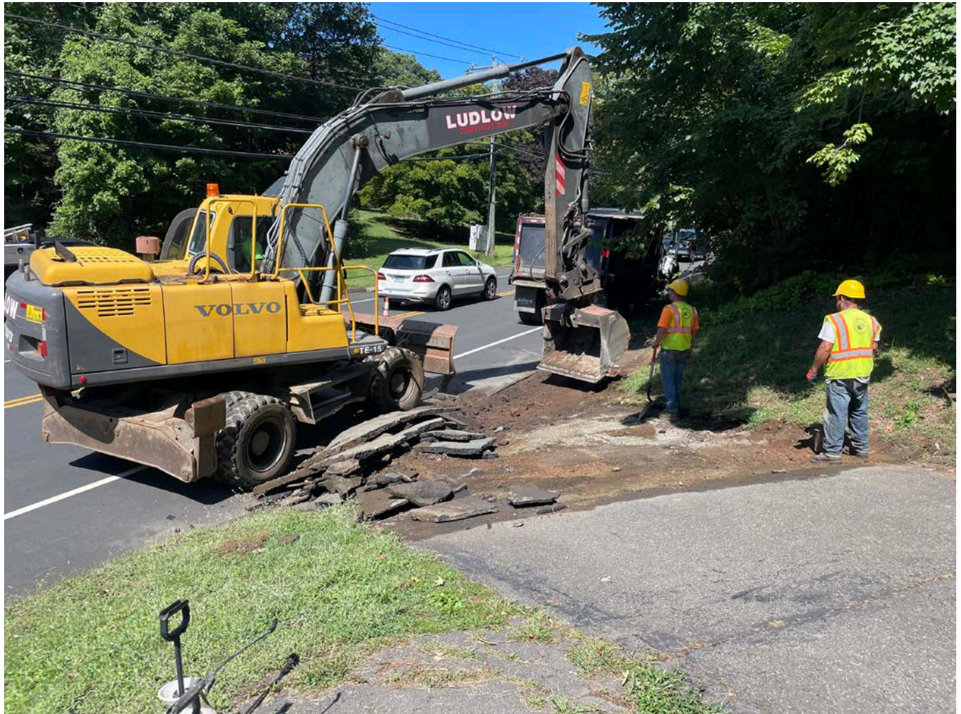
Picture 7: Ludlow stripping asphalt from the driveway apron of the 475 Main Street, Durham, property as they prepare to repave. View to the northwest.
