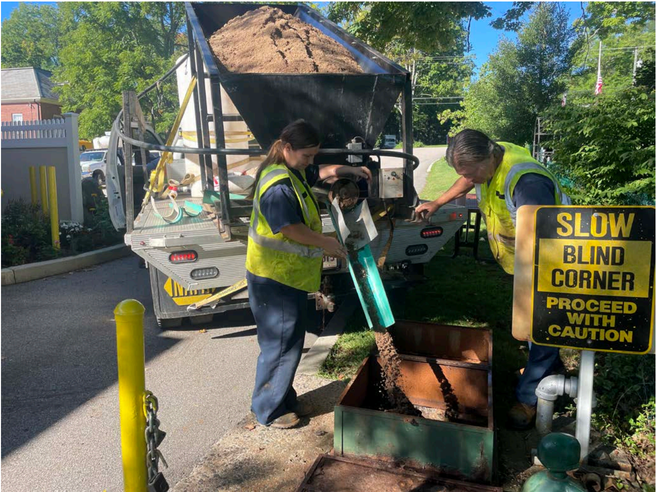
Picture 3: Grela placing sand into the well located to the north of the northwest corner of the Durham Manufacturing facility located on 201-203 Main Street in Durham as part of well decommissioning activities. View to the west.
