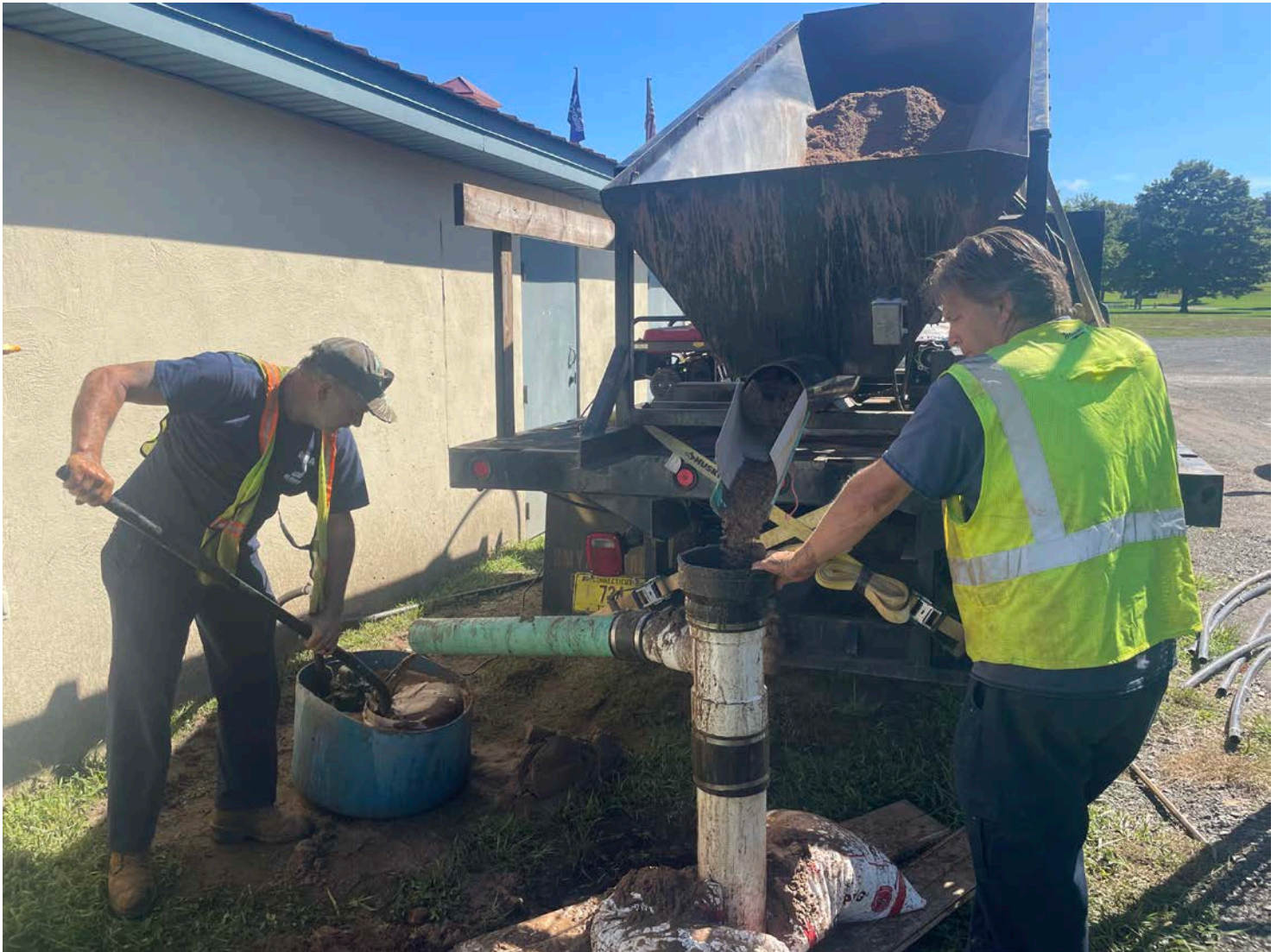
Picture 5: Grela placing sand into the well located to the south side of the recreation center next to the pickleball courts on the north side of Pickett Lane. View to the east.
