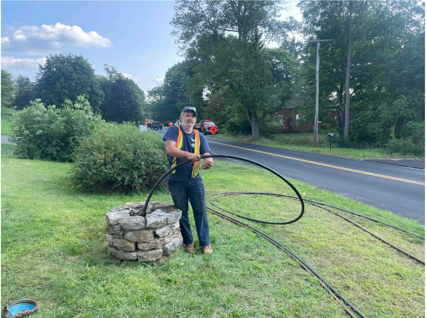
Picture 10: Grela pulling the pump from the well located on the west side of the 133 Maple Avenue, Durham, residence. View to the south.
