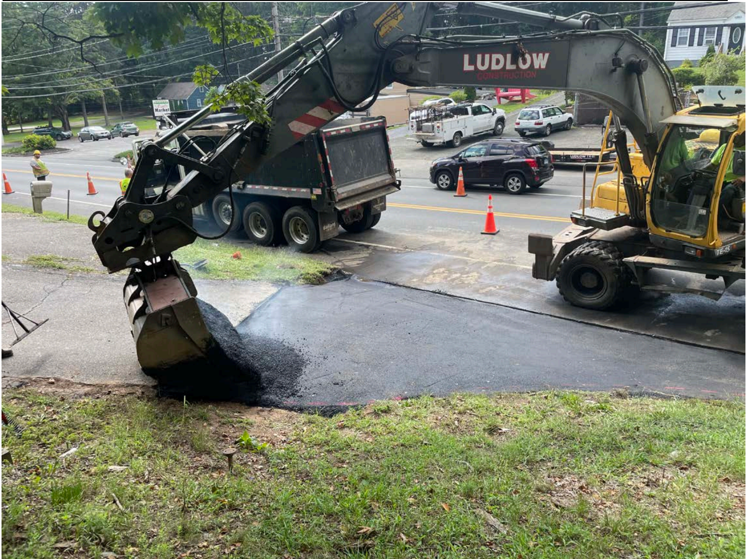
Picture 9: Ludlow placing a second lift of asphalt onto the footprint of the driveway apron at the 475 Main Street, Durham, property. View to the southwest.
