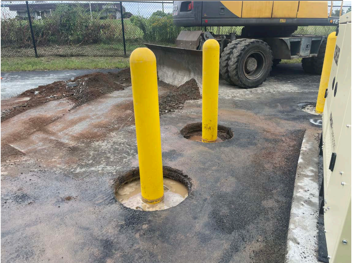
Picture 10: Bollards placed around the generator located on the west side of the Booster Station that Ludlow has cemented into place. View to the north.
