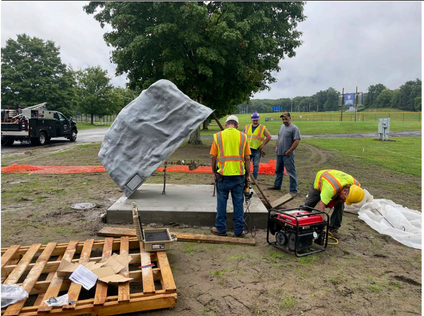
Picture 1: Ludlow placing a cover over the backflow preventer located on the south side of Pickett Lane, Durham, at Station 517+73. View to the east.
