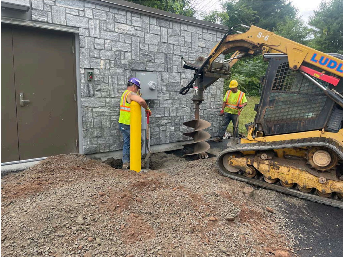
Picture 4: Ludlow auguring a hole for the placement of a bollard on the west side of the Water Meter Building located on S. Main Street in Middletown. View to the southeast.
