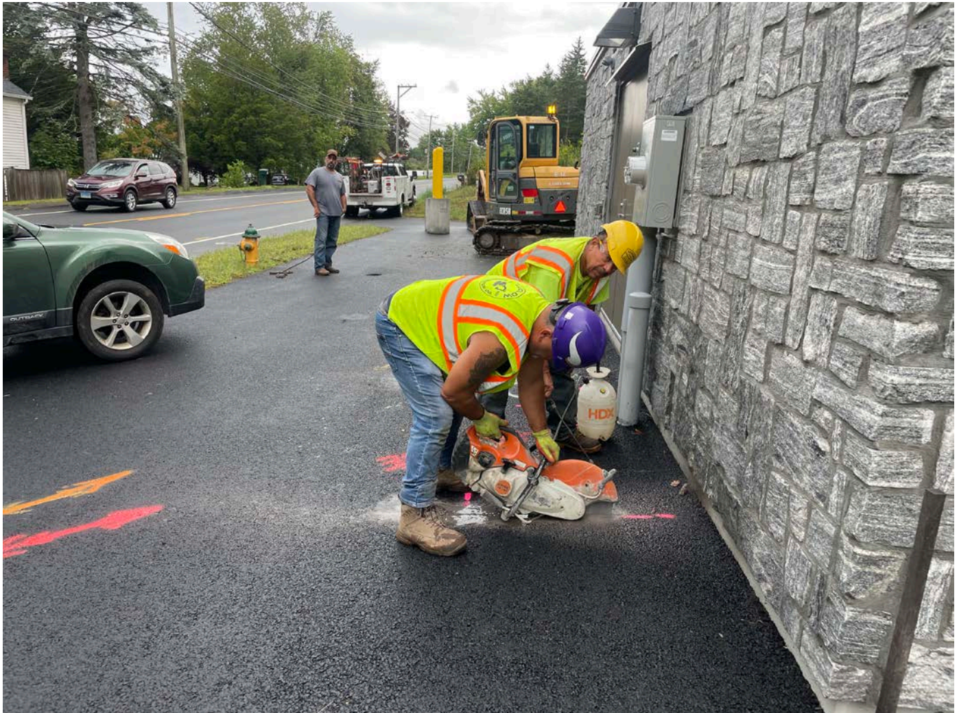
Picture 2: Ludlow saw-cutting asphalt on the west side of the Water Meter Building as they prepare to install two bollards. View to the north.
