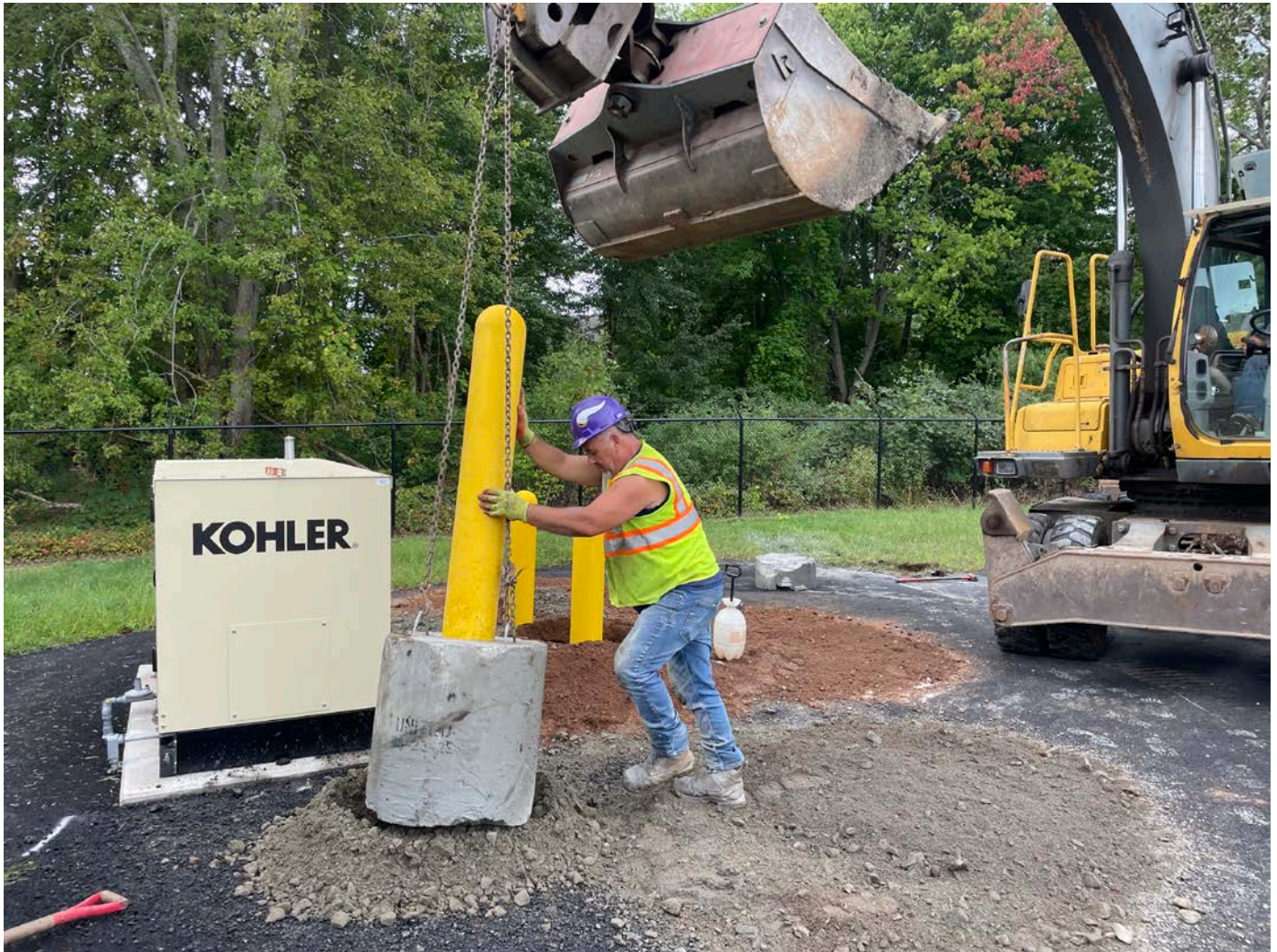
Picture 8: Ludlow placing a third bollard on the north side of the generator located on the west side of the Booster Station in Middletown. Ludlow cut 1' off the bottom of the bollard base due to the presence of concrete ~2' below surface grade associated with subsurface electrical conduits. View to the southwest.
