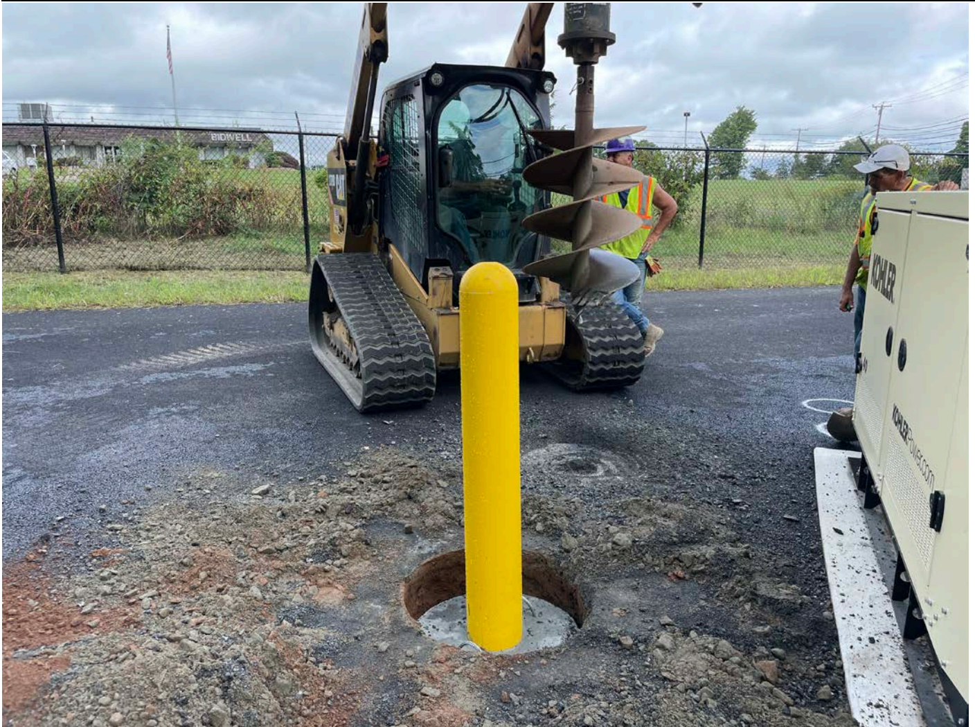
Picture 7: Ludlow preparing to auger a hole for the placement of a second bollard on the west side of the generator located on the west side of the Booster Station in Middletown. View to the north.
