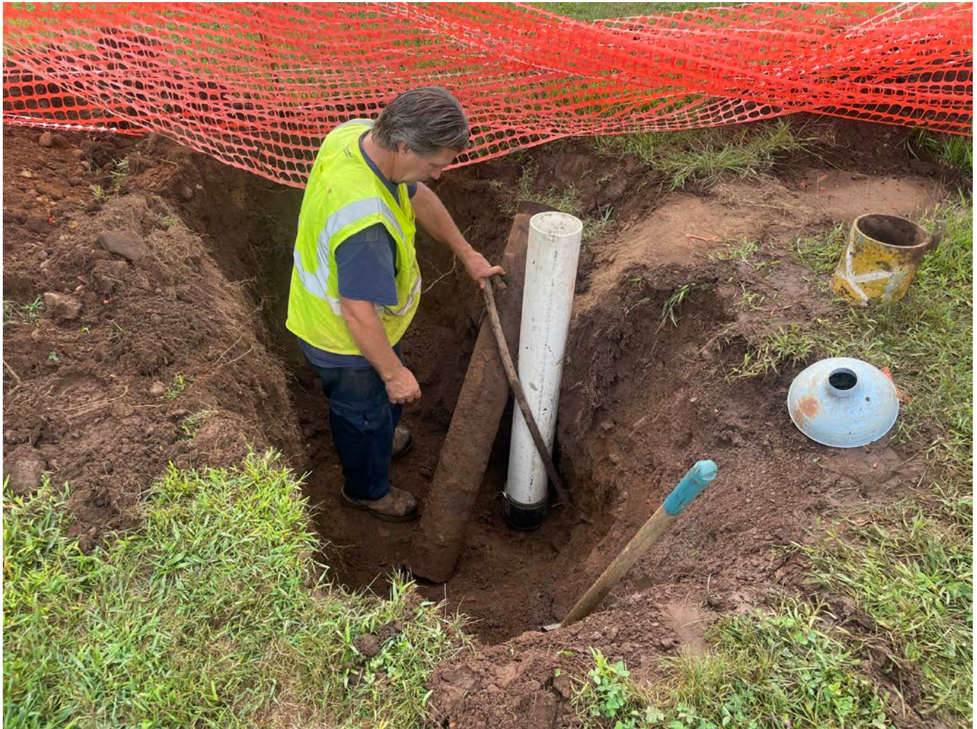
Picture 3: Grela working to decommission the well located at Station 518+50 on the north side of Pickett Lane in Durham. View to the south.
