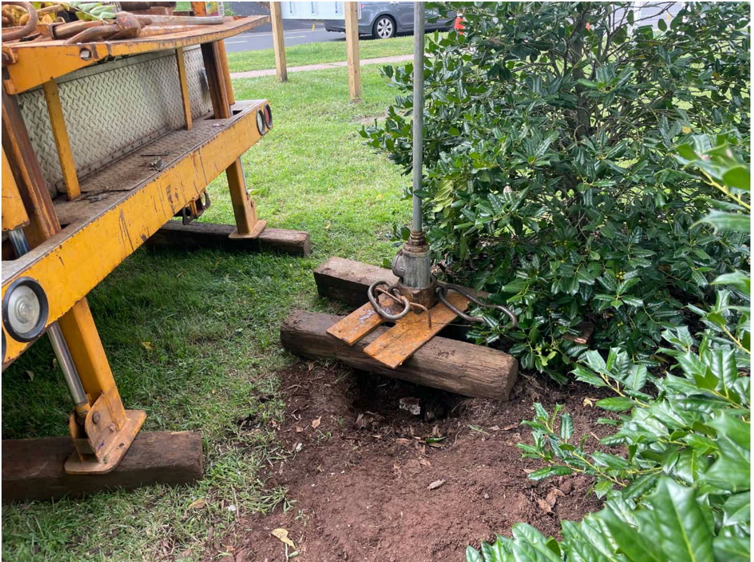
Picture 11: Grela set up to pull the pump from the well located in the southwest corner of the vault that is located on the west side of the Durham Manufacturing facility. View to the west.
