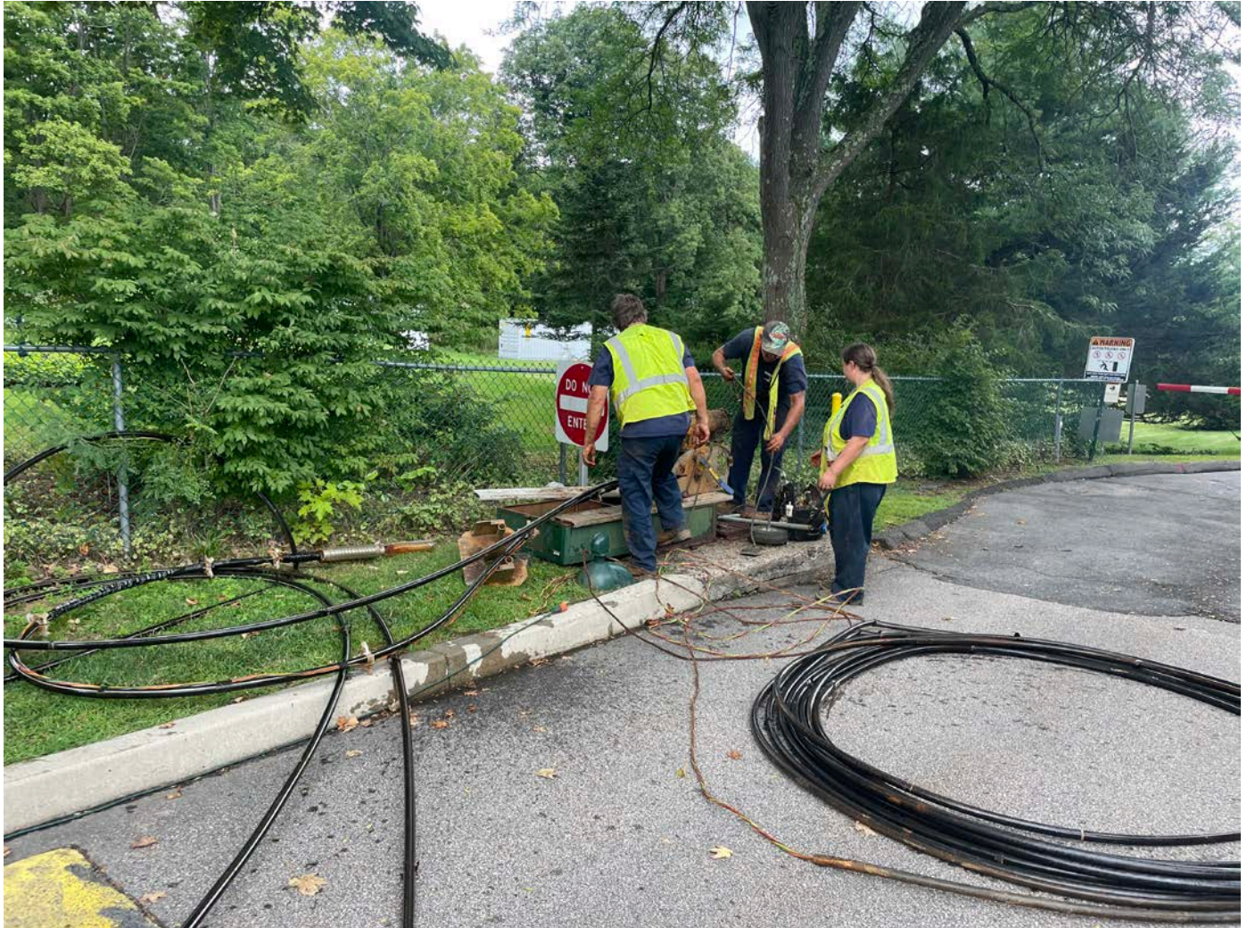
Picture 12: Grela preparing to pull the pump from the well located on the north side of the Durham Manufacturing facility. View to the northeast.
