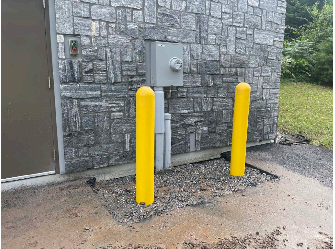
Picture 5: Bollards installed at the electrical service to the water meter building on South Main Street in Middletown. View to the southeast.
