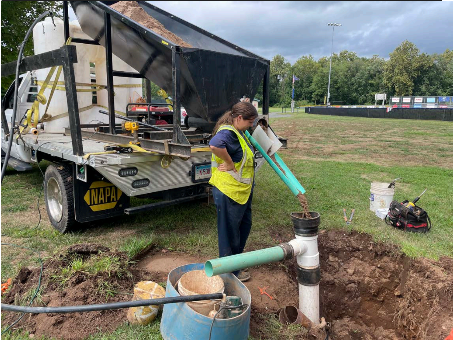
Picture 9: Grela placing sand into the well located at Station 518+50 on Pickett Lane as part of well decommissioning activities. View to the southwest.
