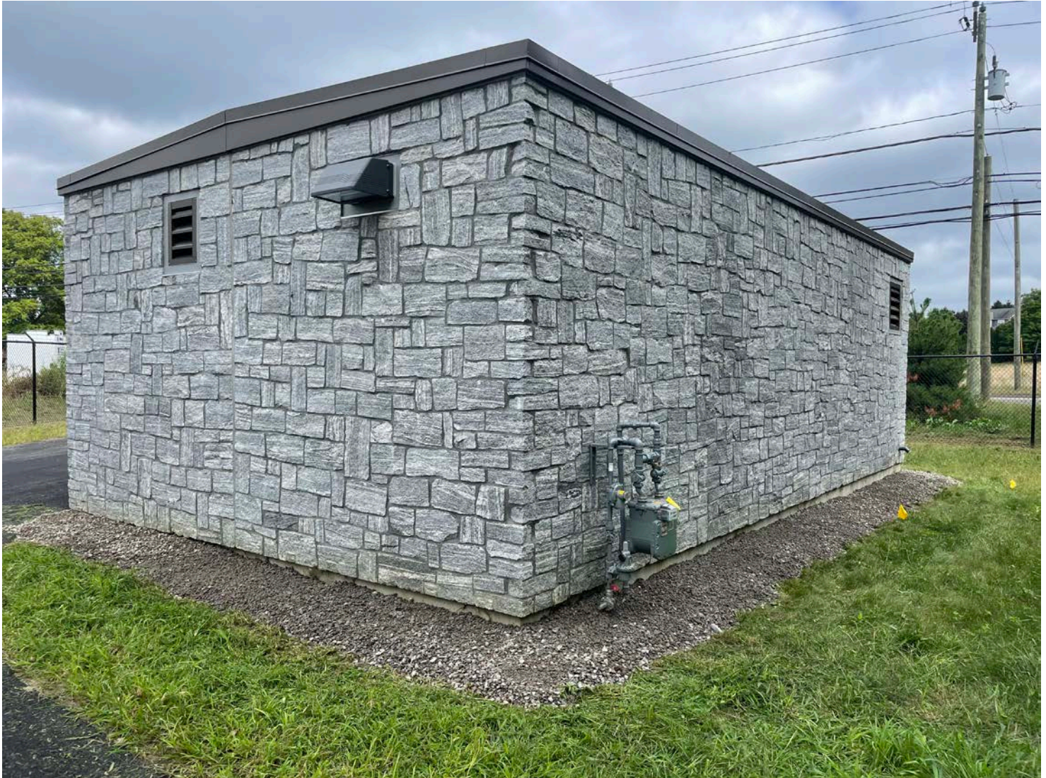
Picture 15: View of the Booster Station located on S. Main Street in Middletown where Ludlow placed geofabric and 3/4" stone along the perimeter of the building. View to the northeast.
