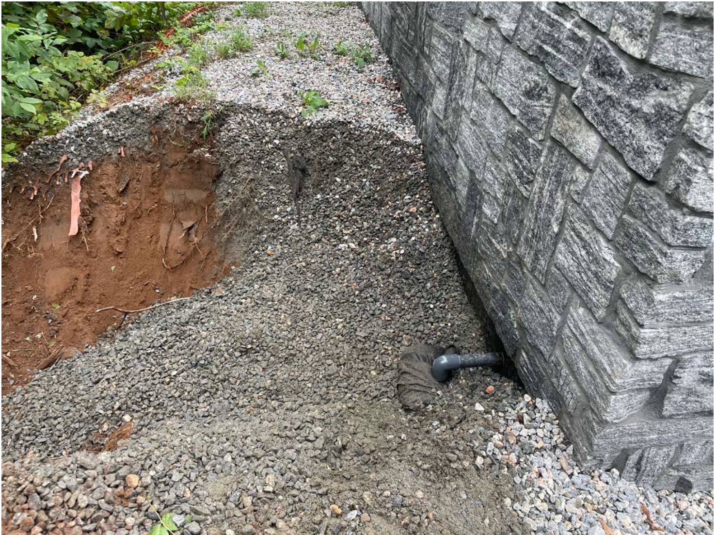
Picture 13: Sump pump discharge pipe that Ludlow daylighted on the northeast corner of the Water Meter Building located on S. Main Street in Durham. View to the south.
