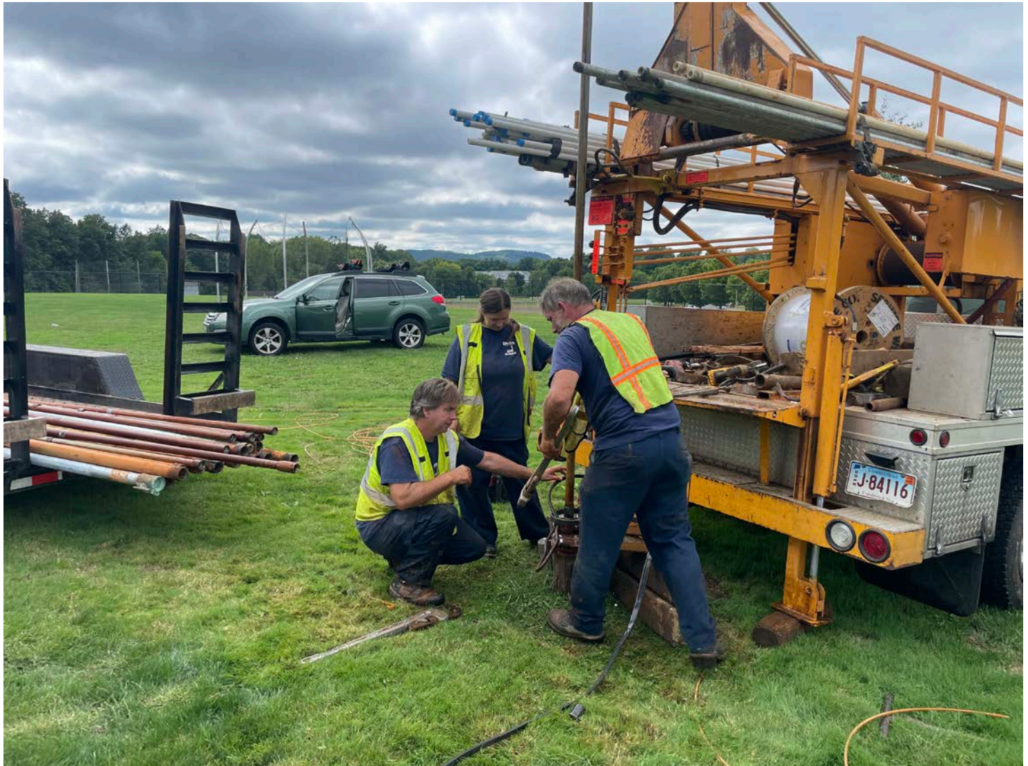
Picture 14: Grela preparing to pull the pump from the well located on the west side of the Coginchaug Regional High School soccer field on the south side of Pickett Lane, Durham. View to the west.
