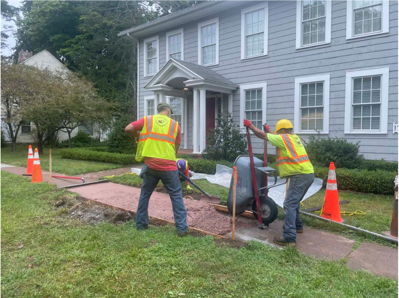
Picture 4: Ludlow placing 4000 PSI concrete on a section of the sidewalk located in front of the 293 Main Street residence in Durham. View to the northeast.
