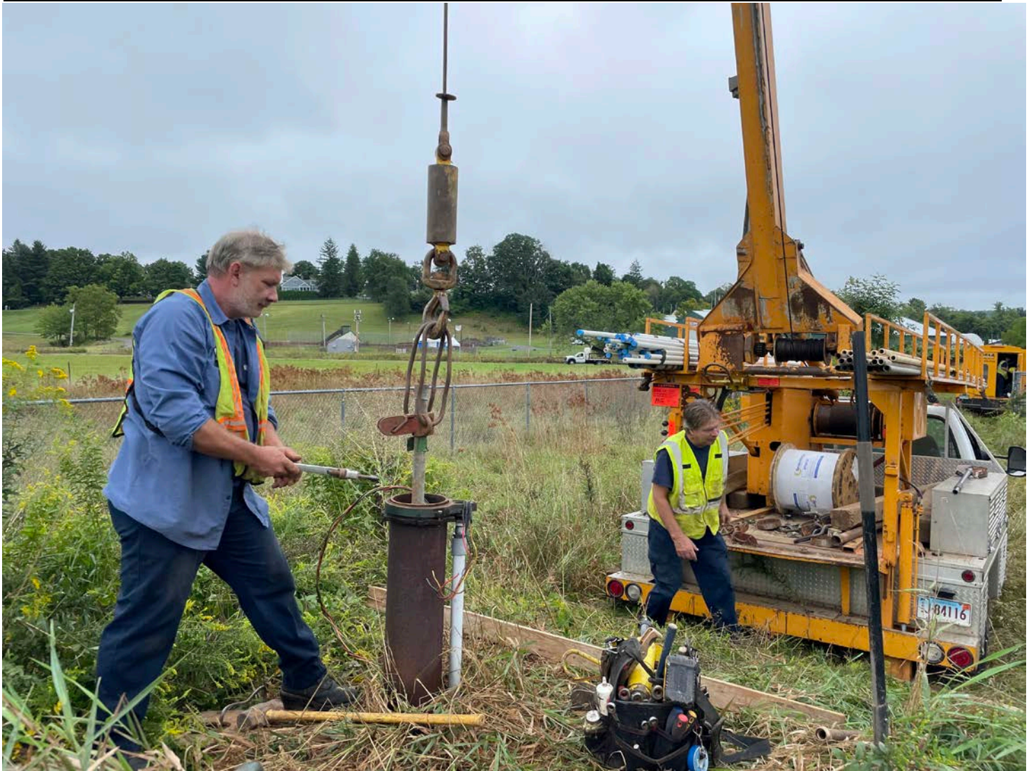
Picture 9: Grela attempting to pull the pump from the easternmost of the two Durham Fairground wells. View to the east.
