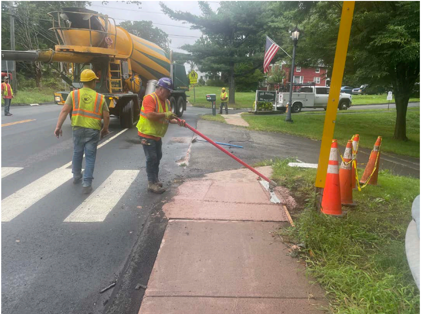
Picture 8: Ludlow leveling 4000 PSI concrete that they placed on a section of the sidewalk located in front of the 153 Main Street residence in Durham. View to the north.
