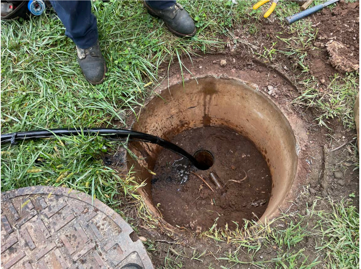
Picture 11: Well located on the west side of the recreation center located on the north side of Pickett Lane, Durham, next to the pickleball courts where Grela is pulling the pump from the well. View to the west.
