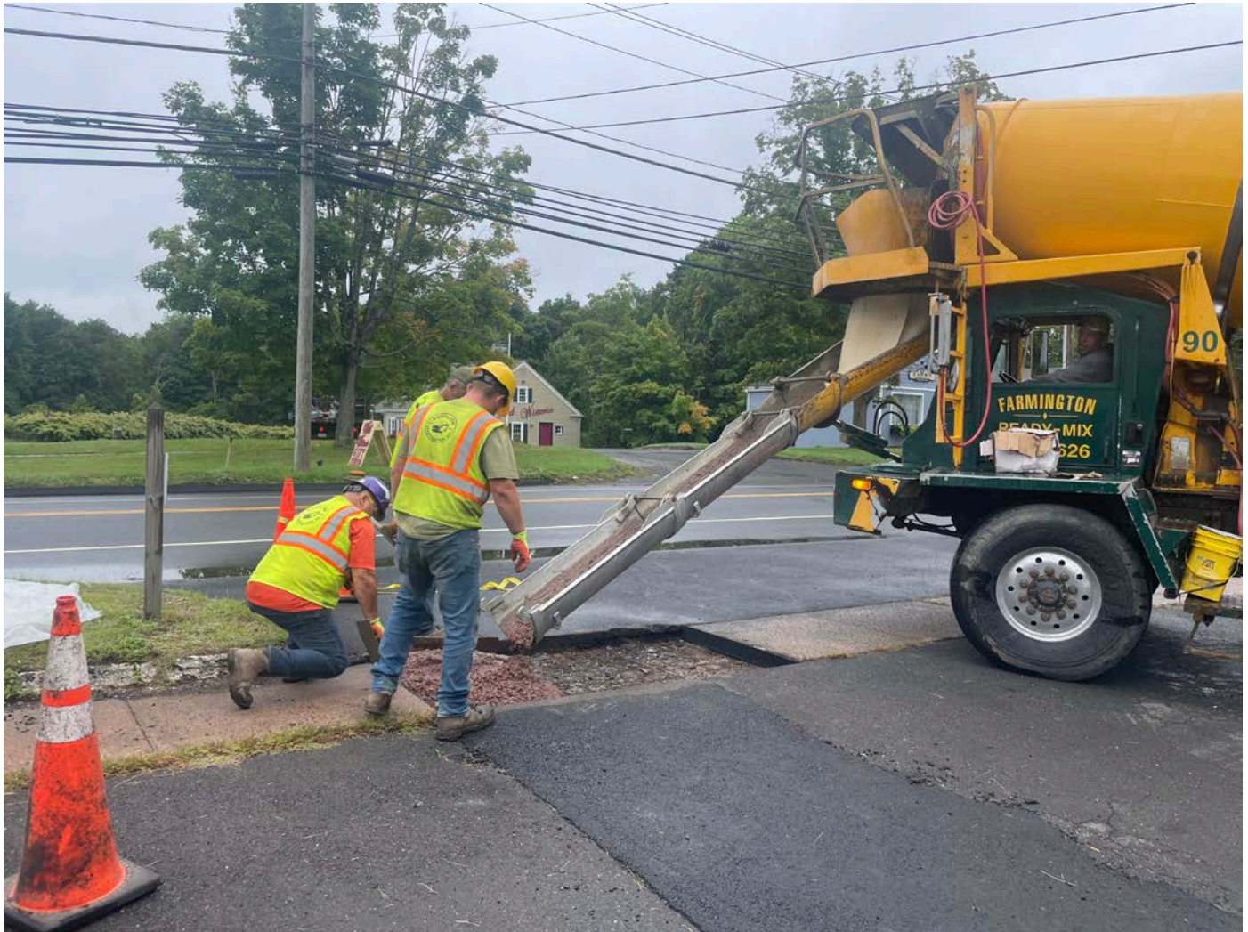
Picture 3: 4000 PSI concrete being placed on a section of the sidewalk located in front of 336 Main Street in Durham. View to the southeast.
