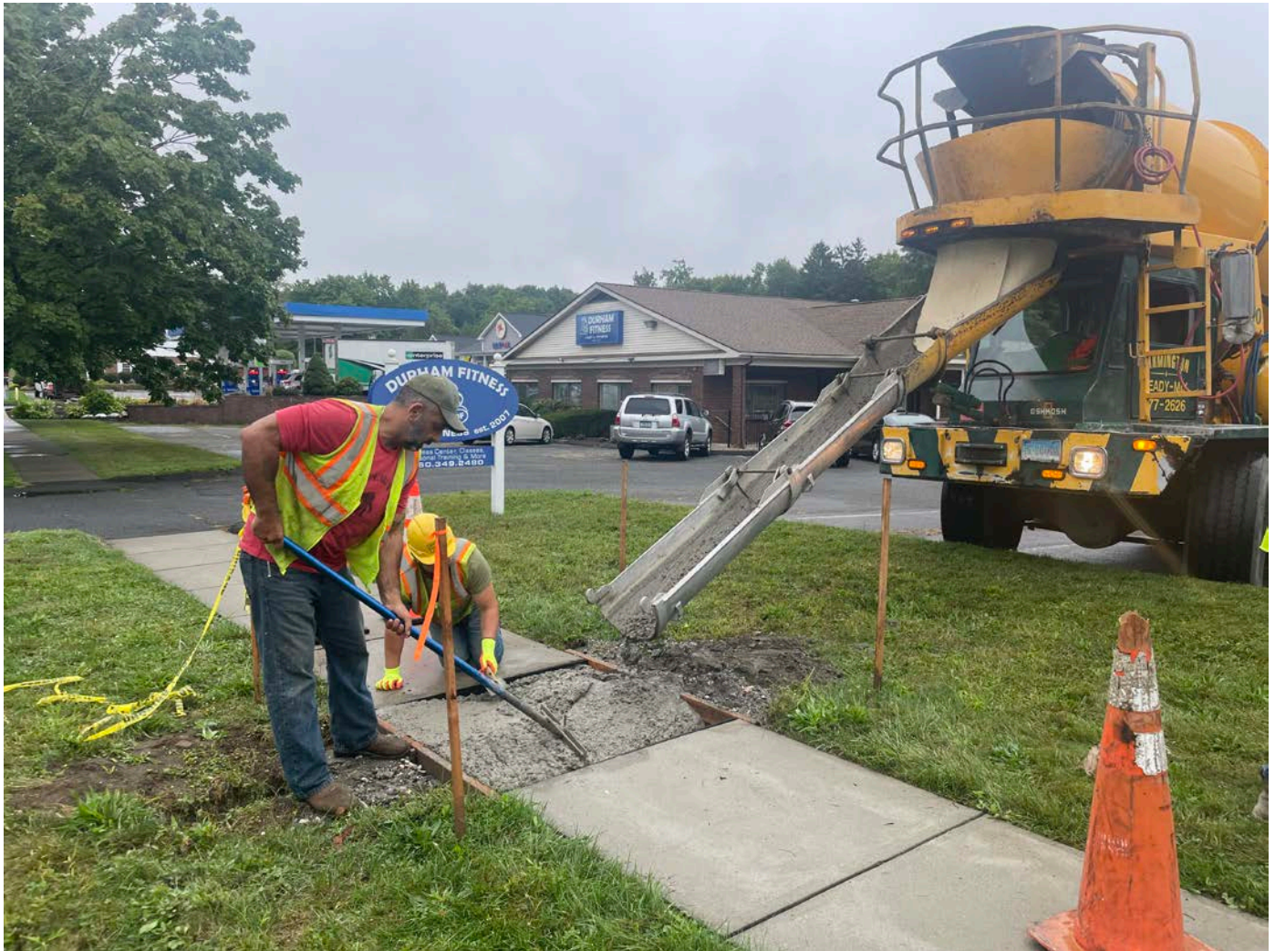
Picture 2: 4000 PSI concrete being placed on a section of the sidewalk located between 331 and 339 Main Street in Durham. View to the southwest.
