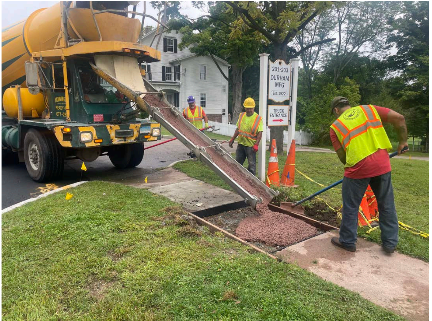
Picture 7: Ludlow placing 4000 PSI concrete on a section of the sidewalk located in front of the 201-203 Main Street property in Durham. View to the northeast.
