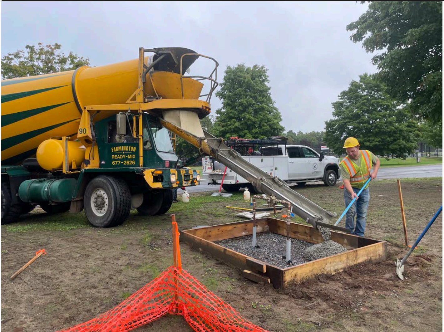
Picture 1: Farmington Ready Mix placing 4000 PSI concrete into a form that was built around the backflow preventer located on the south side of Pickett Lane, Durham, at Station 517+73. View to the northeast.
