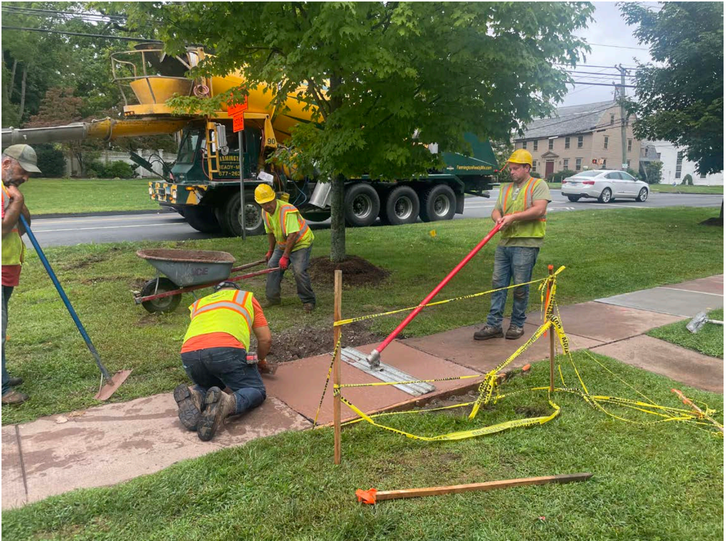
Picture 6: Ludlow leveling 4000 PSI concrete that they placed on a section of the sidewalk located in front of the 215 Main Street residence in Durham. View to the northwest.
