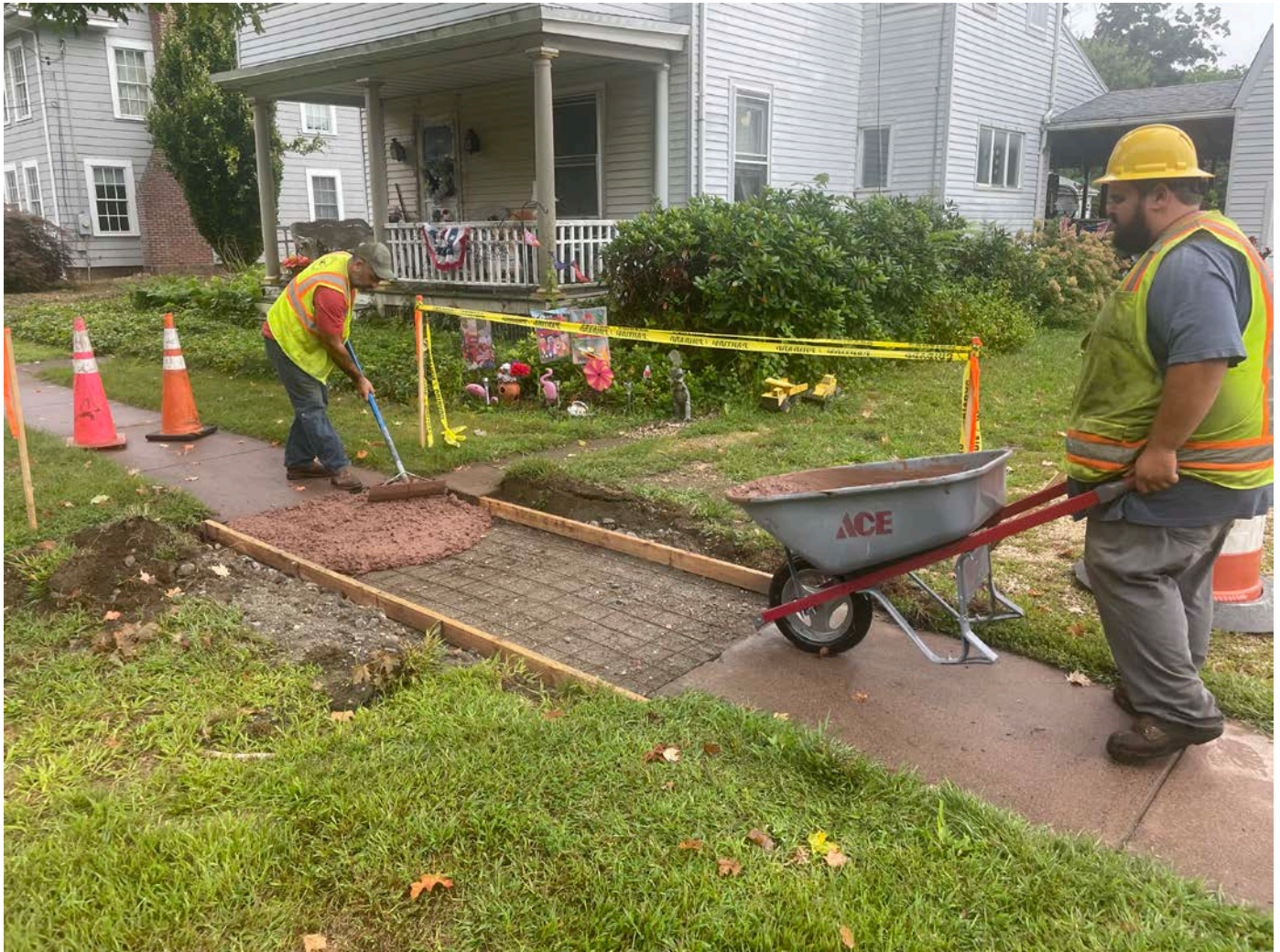
Picture 5: Ludlow placing 4000 PSI concrete on a section of the sidewalk located in front of the 289 Main Street residence in Durham. View to the northeast.
