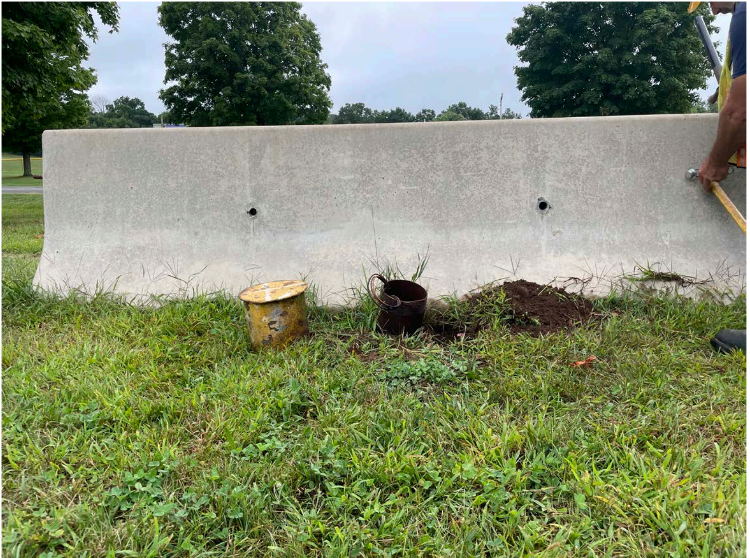
Picture 10: Well casing located 45' north of Pickett Lane, Durham, at Station 518_50. Grela was unable to pull the pump from this well as the casing had been previously damaged. View to the west.
