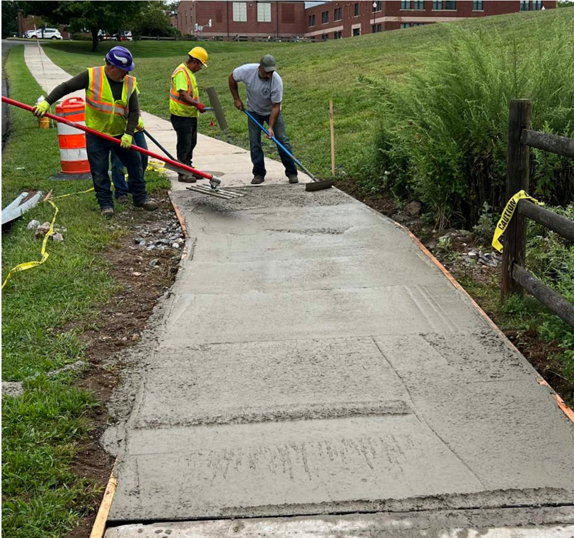
Picture 4: Ludlow Construction is using concrete screeds, rakes, and floats to adjust the recently placed concrete located between Cuginchaug Regional High School and Frank Ward Strong School on the north side of Pickett Lane.
