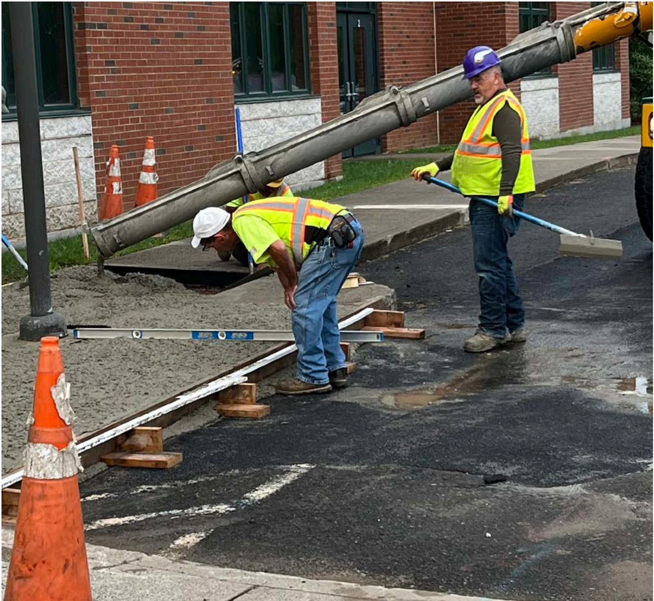
Picture 2: Ludlow Construction is checking the level of the wooden forms to the existing light pole base to confirm that the concrete will be at the desired grade.
