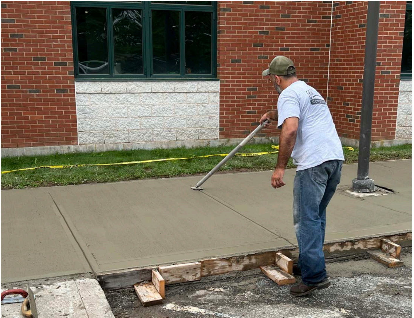
Picture 5: Ludlow construction is tooling the joints in the concrete sidewalk near Coginchaug Regional High School.
