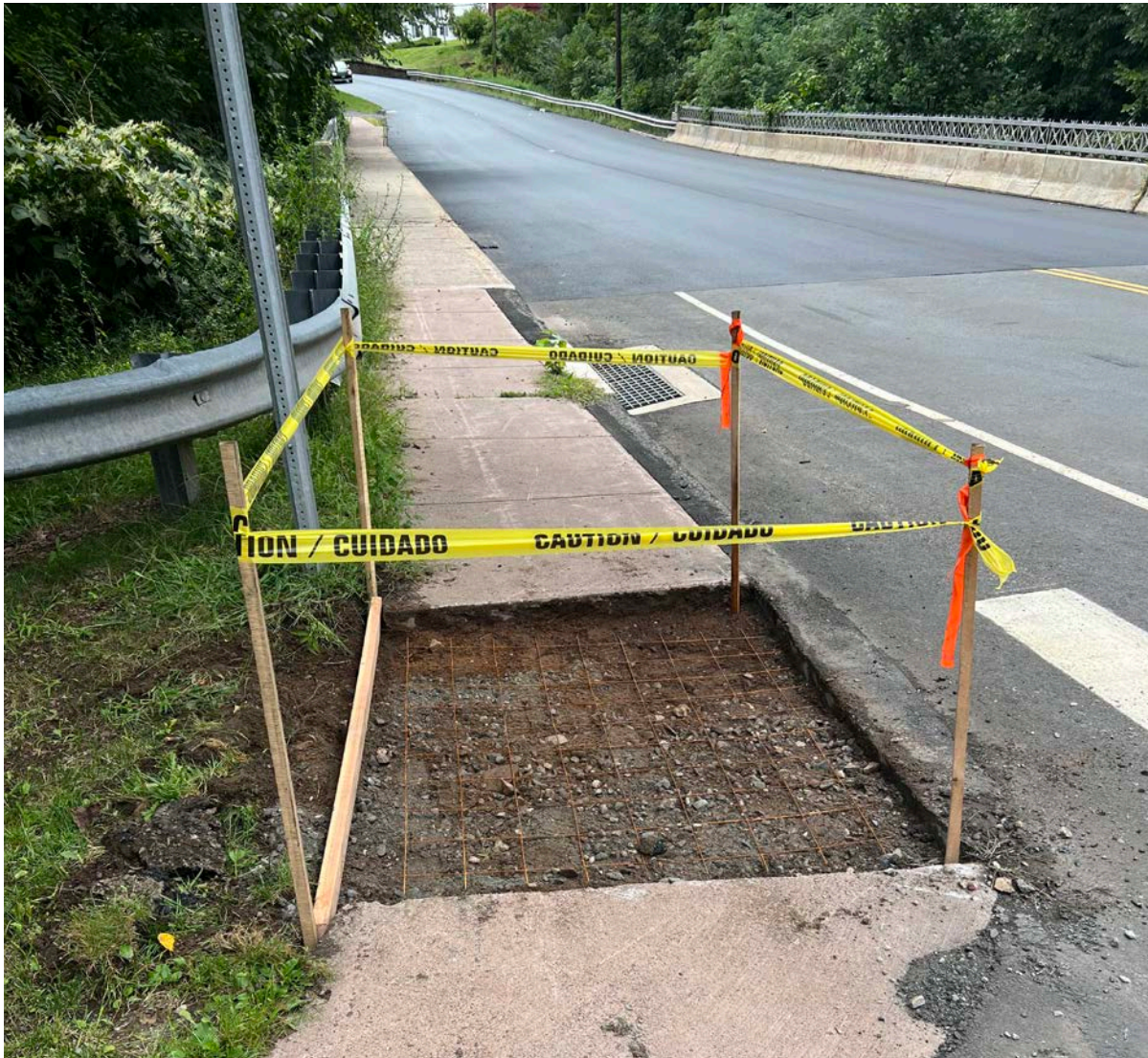
Picture 7: Ludlow Construction has finished forming a section of removed sidewalk located at 153 Main Street Durham. View to the south.
