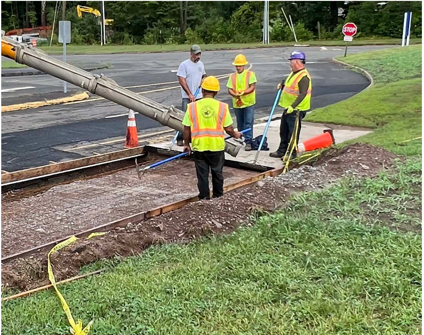
Picture 3: Ludlow Construction is placing concrete in another section of removed sidewalk located near Coginchaug Regional High School.
