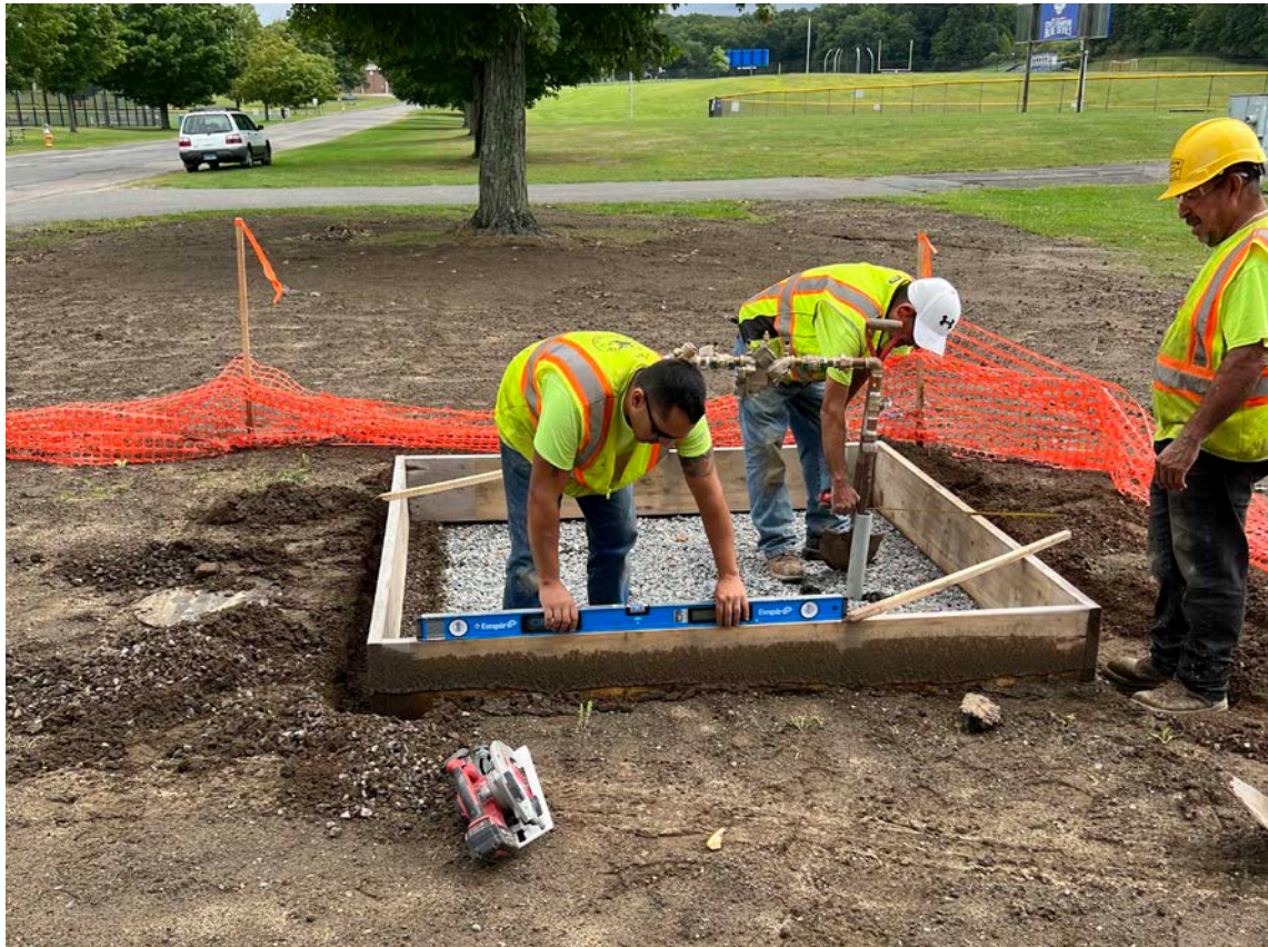
Picture 6: Ludlow Construction begins to adjust the forms for the backflow preventer enclosure base on the south side of Pickett Lane.
