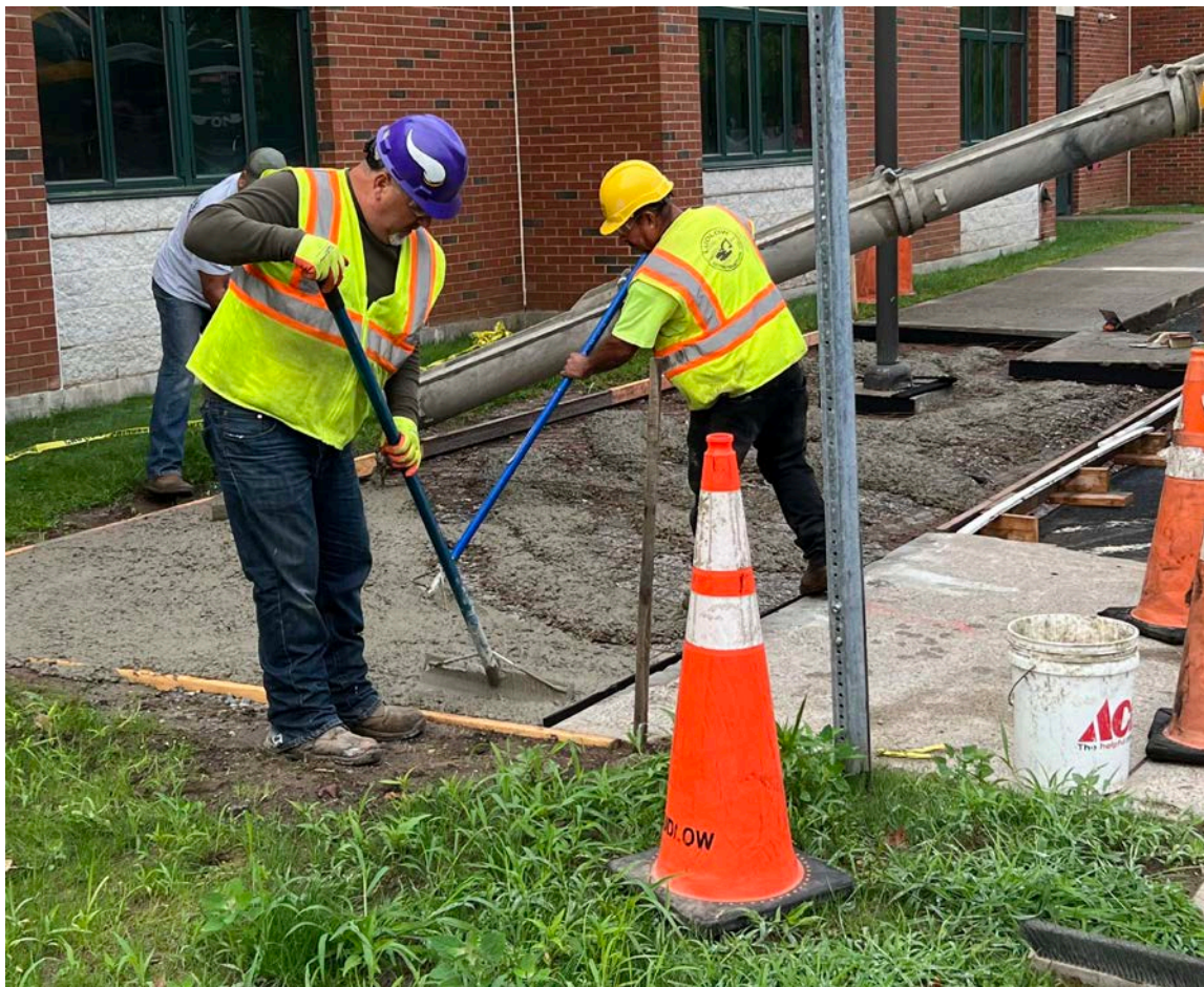
Picture 1: Ludlow Construction is placing concrete onto a section of removed sidewalk located near Coghinchaug Regional High School that has been prepped for concrete placement.
