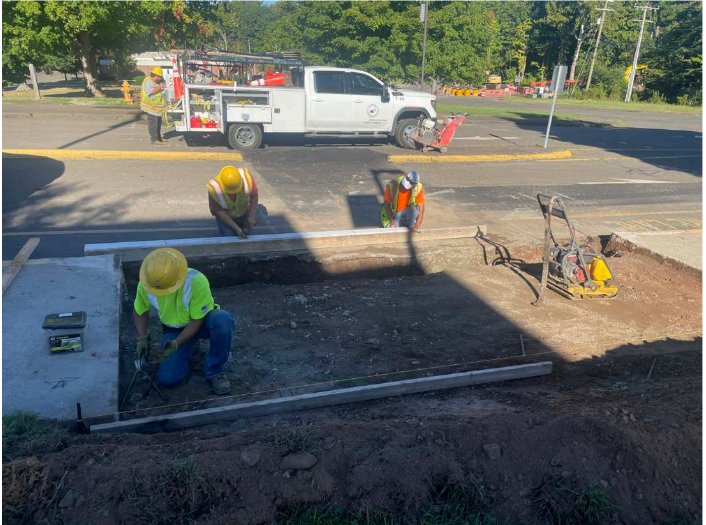
Picture 5: Ludlow constructing a concrete form on the sidewalk located on the west side of the Coginchuag Regional High School, Durham, as they prepare to repair the sidewalk. View to the west.
