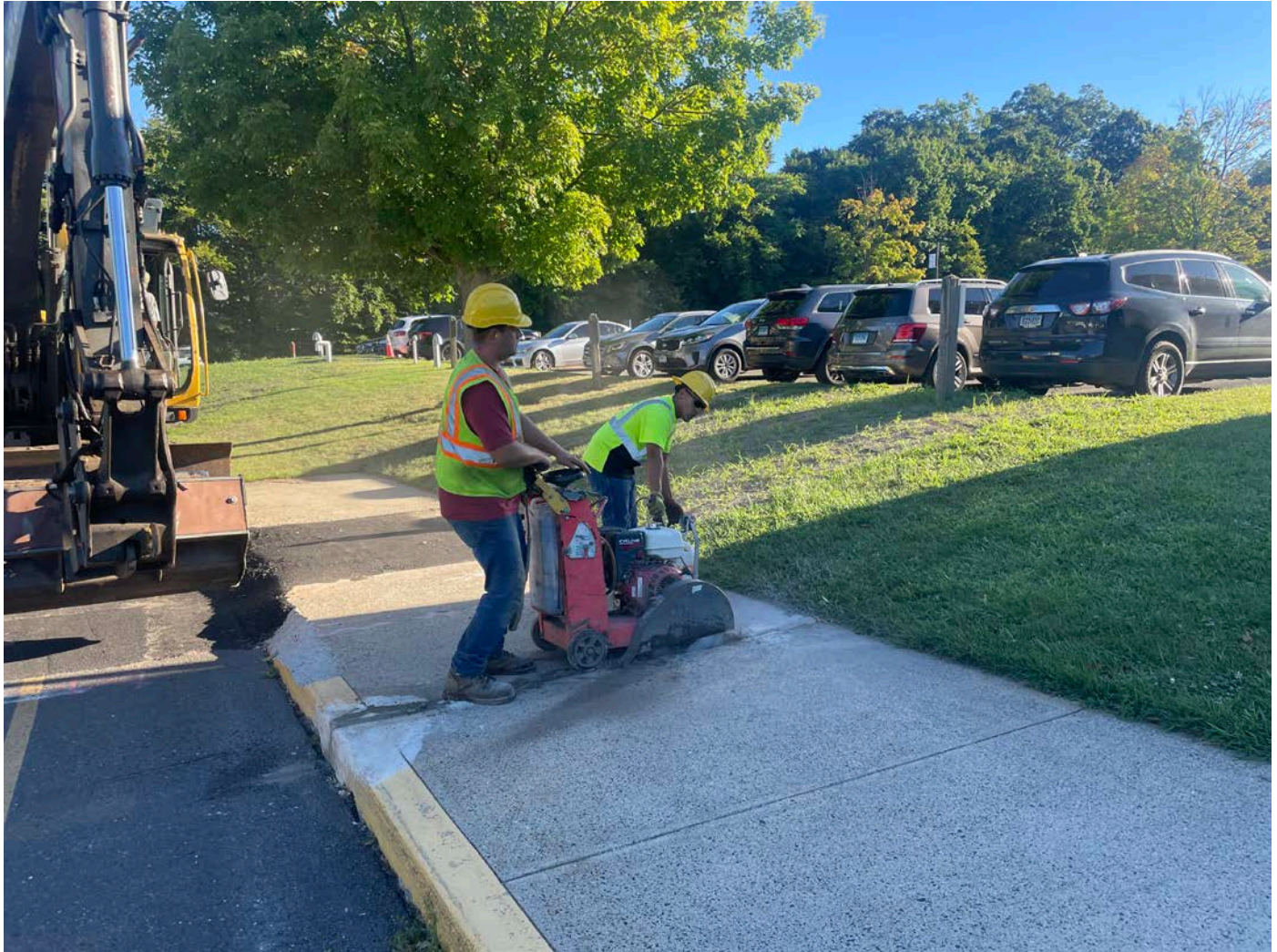
Picture 3: Ludlow saw-cutting a damaged sidewalk panel located on the west side of the Coginchuag Regional High School, Durham, as they prepare to repair the sidewalk. View to the north.
