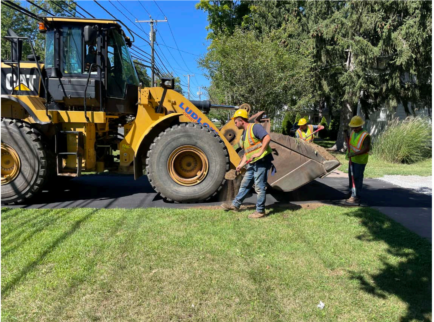
Picture 11: Ludlow placing loam and grass seed on both sides of the paved portion of the driveway located at the 303/305R Main Street, Durham, property. View to the north.
