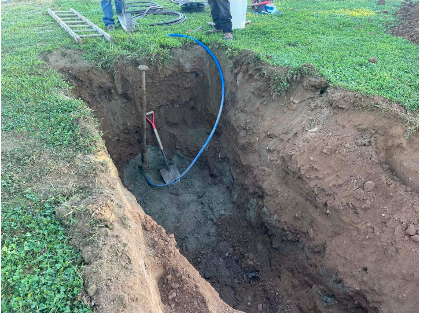
Picture 2: Curb stop located at Station 517+73 that Ludlow daylighted. View to the northeast.
