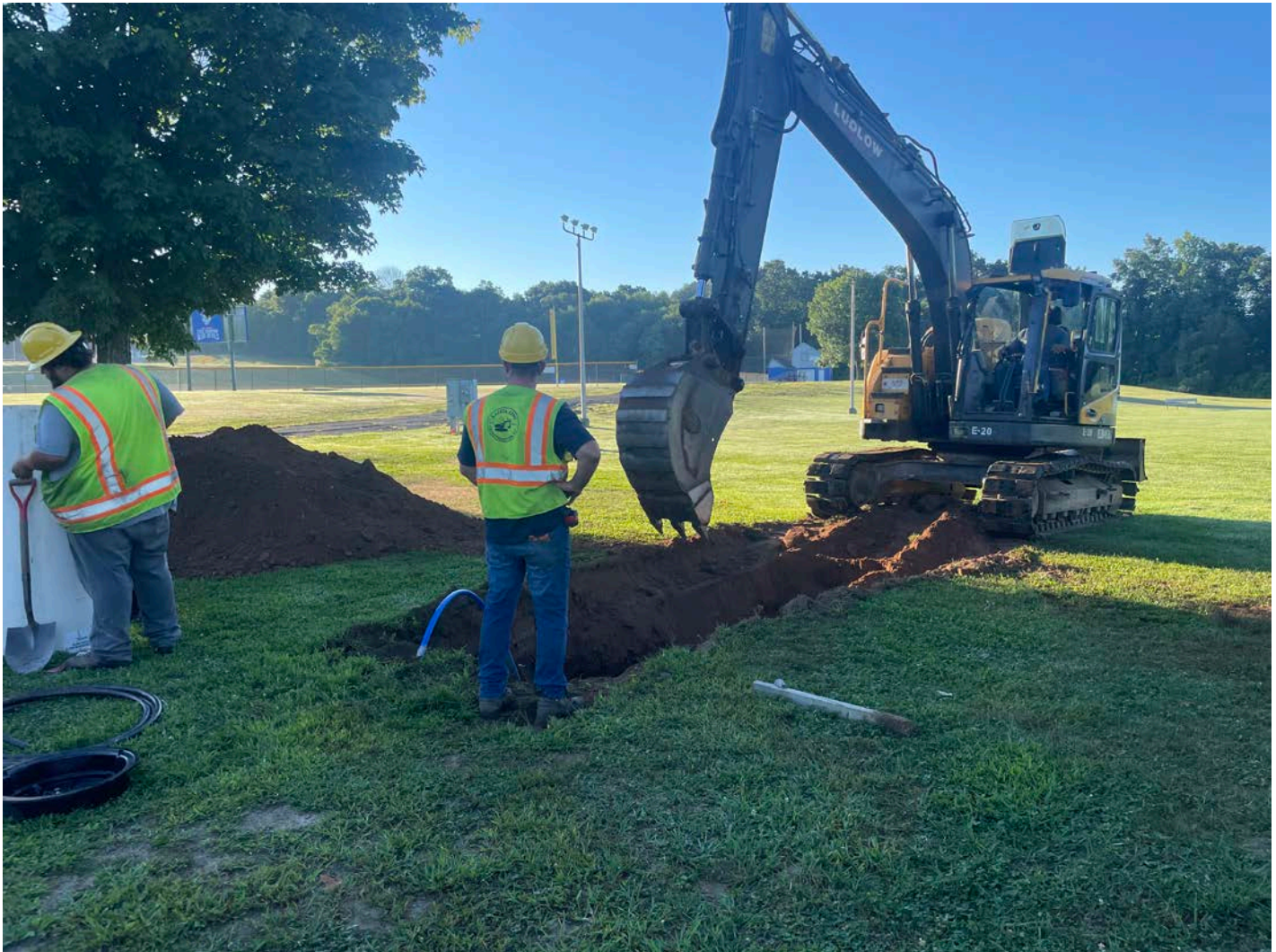
Picture 1: Ludlow excavating at Station 517+73 for the installation of a 1" copper water service line. View to the southeast.
