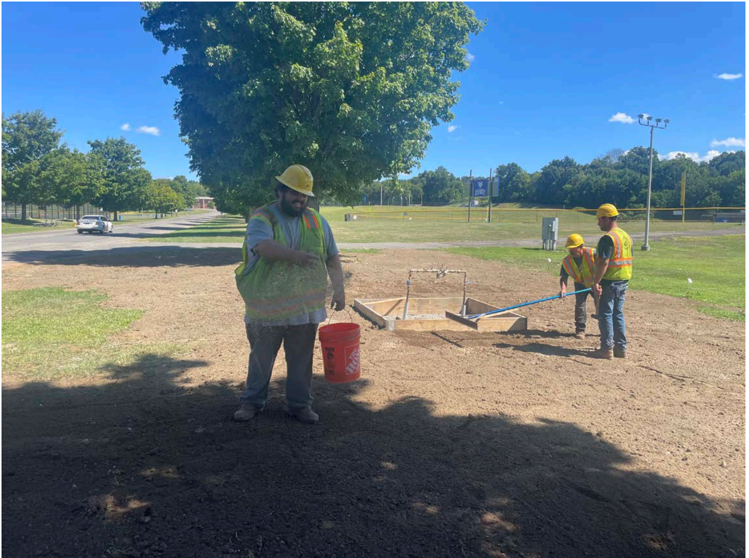
Picture 9: Ludlow grading loam and spreading grass seed on the areas that were disturbed when they installed a meter pit, backflow preventer, and copper water service line starting at the curb stop located at Station 517+73. View to the west.
