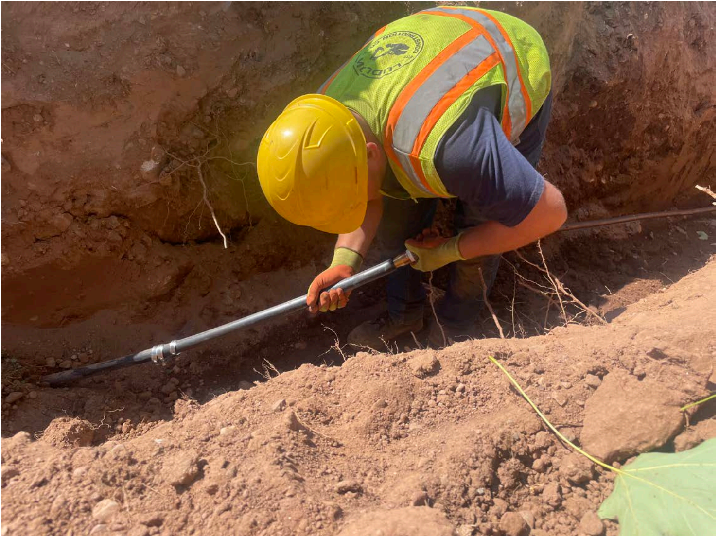
Picture 6: Ludlow connecting the 1" copper water service line that they ran from Station 517+73 to the south and then to the east to the existing HDPE water line.
