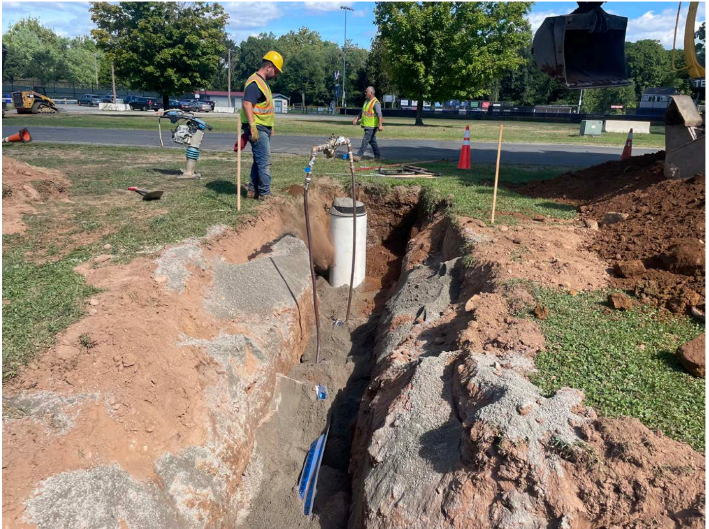
Picture 5: Backflow preventer and meter pit that Ludlow installed at Station 517+73. View to the north.
