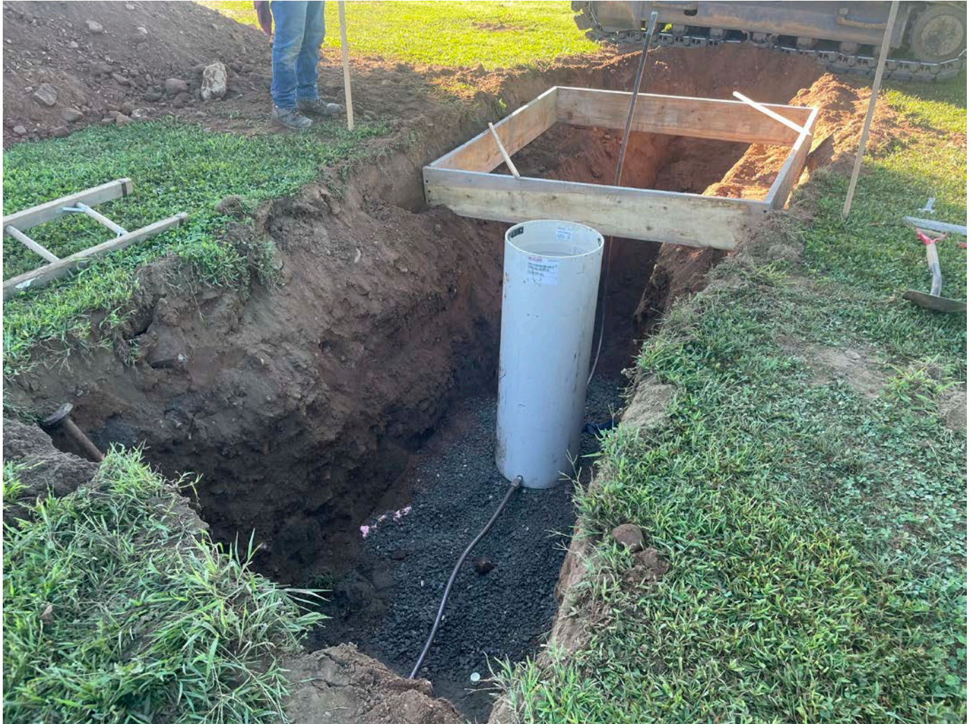
Picture 3: Meter pit that Ludlow installed at Station 517+73, with a section of 1" copper water service line that was run between the curb stop and the meter pit. View to the southeast.
