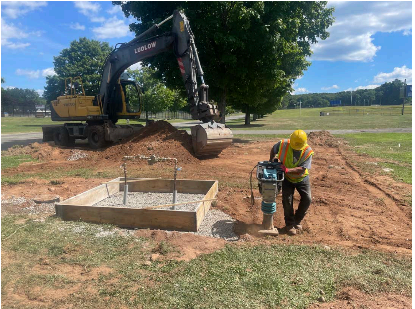
Picture 7: Ludlow compacting backfill on the north side of a concrete form they placed around the backflow preventer at Station 517+73. View to the east.
