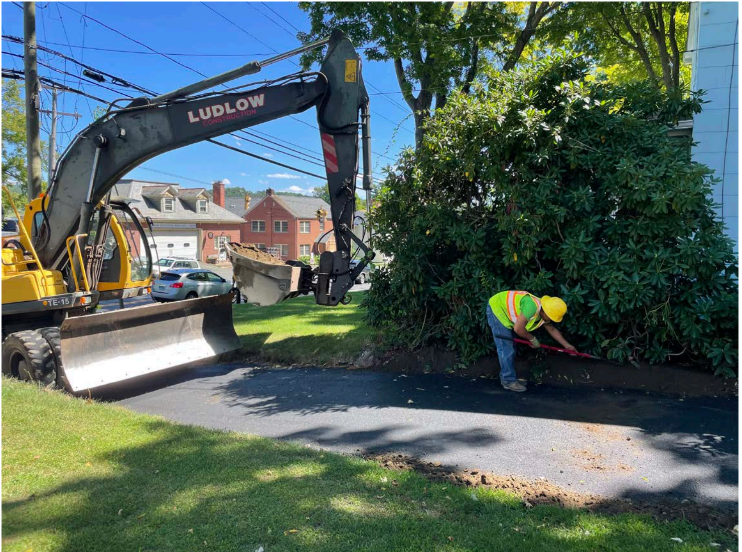
Picture 10: Ludlow placing loam and grass seed on both sides of the paved portion of the driveway located at the 208 Main Street, Durham, property. View to the southeast.
