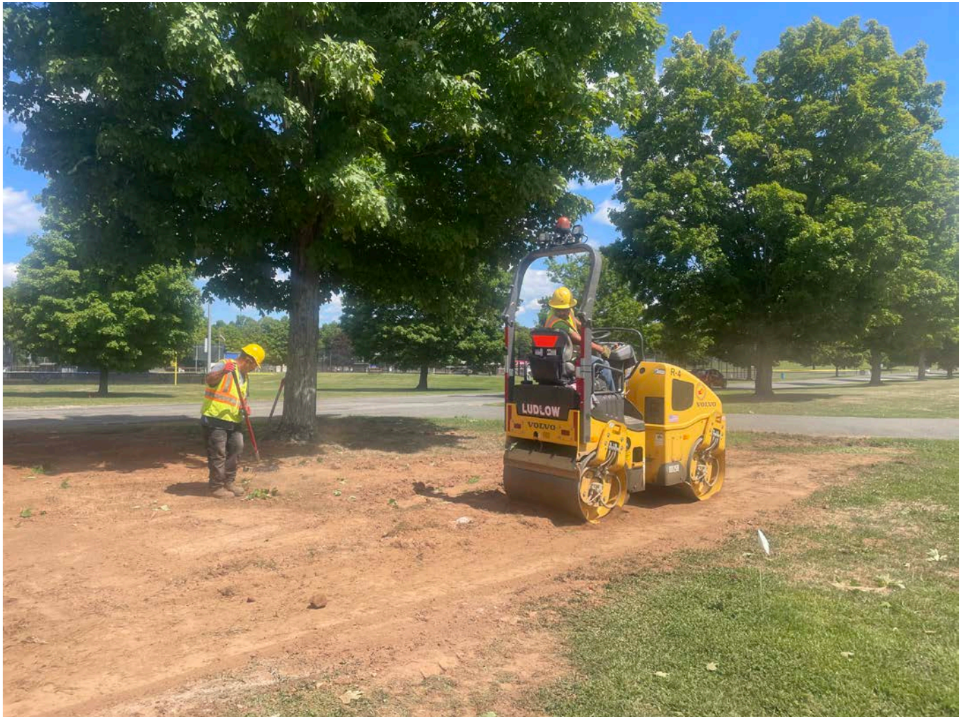
Picture 8: Ludlow using a rolling compactor on the native fill they backfilled over the 1" copper water service line they installed starting at the curb stop located at Station 517+73. View to the northeast.
