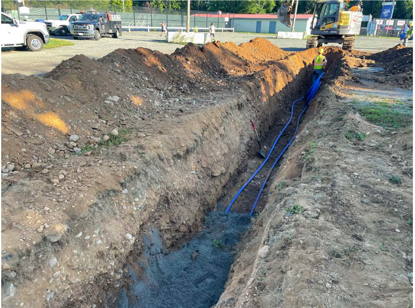
Picture 2: Ludlow installing two 1.5" polyethylene water lines to the north of the two meter vaults they installed at Station ~516+55. View to the north.
