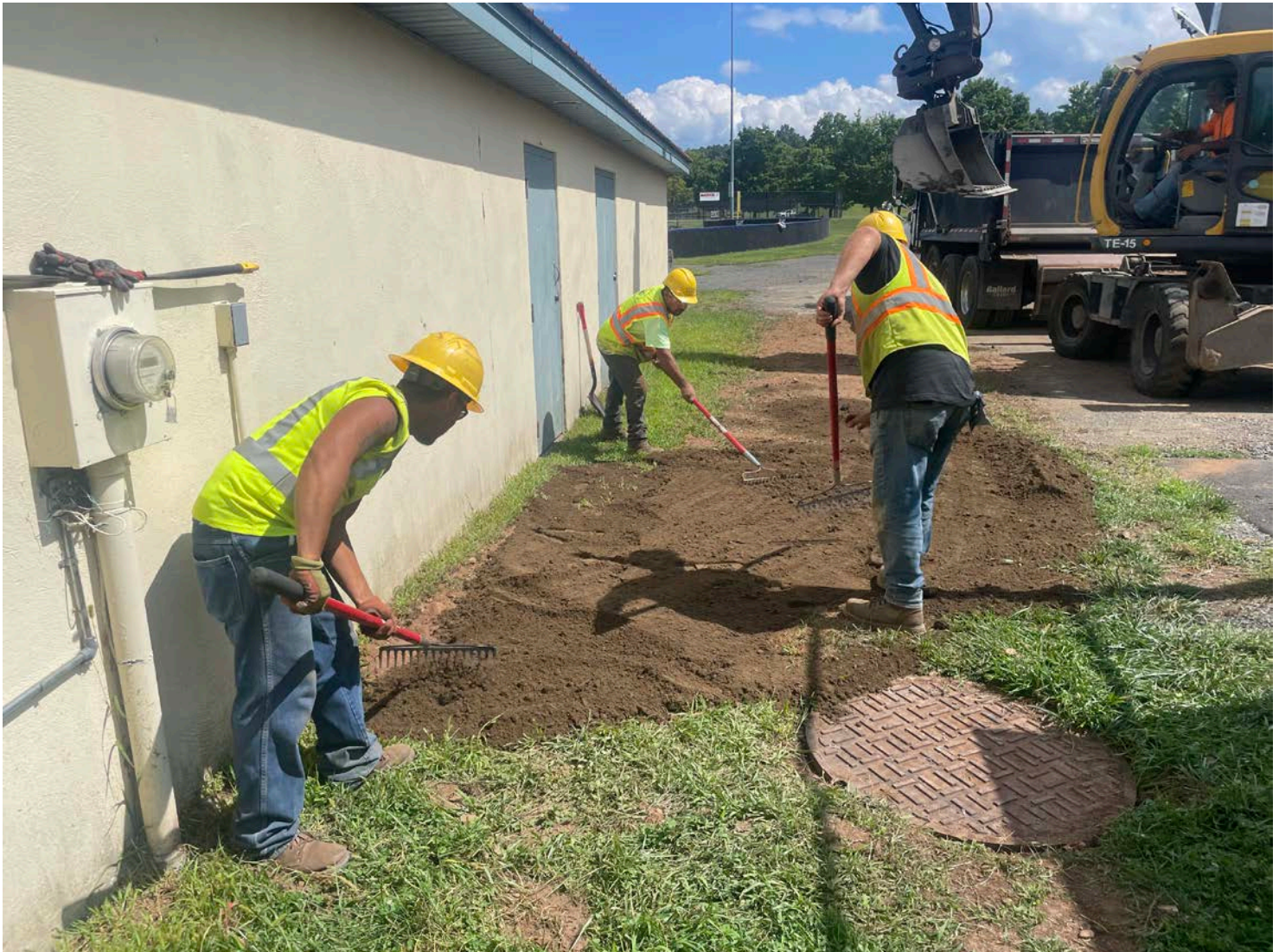
Picture 11: Ludlow placing loam and grass seed on the south side of the recreation center located on Pickett Lane after they installed two 1.5" polyethylene water lines. View to the east.
