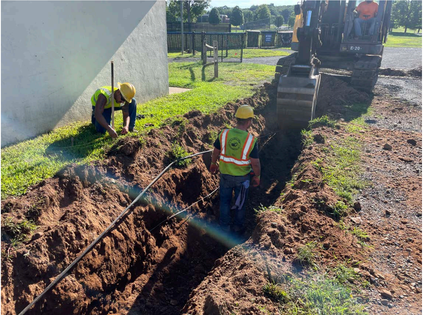
Picture 6: Ludlow excavating on the south side of the recreation center in order to install two 1.5” polyethylene water lines at the recreation center. View to the east.
