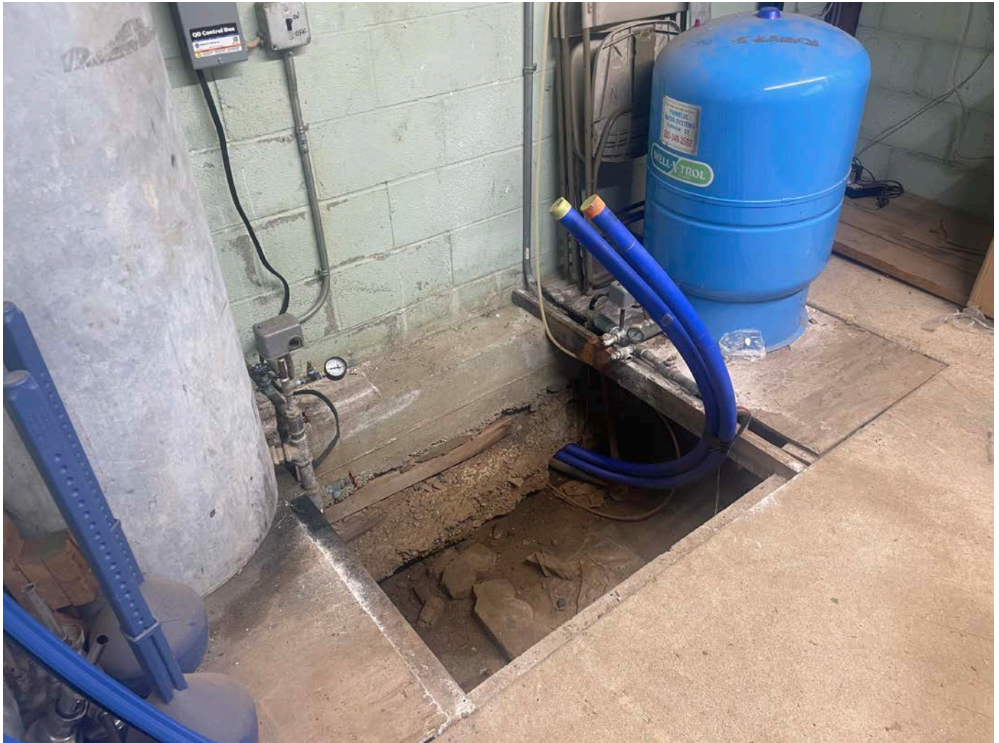
Picture 8: View from the inside of the recreation center where Ludlow ran two 1.5" polyethylene waters. View to the southwest.
