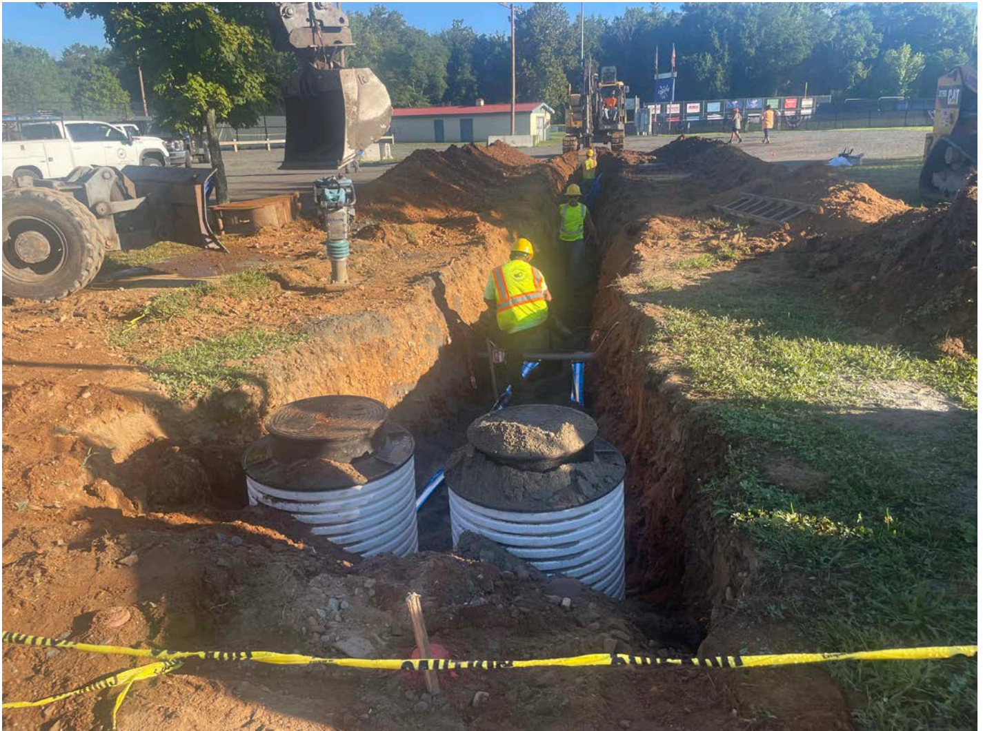
Picture 1: Ludlow installing two 1.5" polyethylene water lines to the north of the two meter vaults they installed at Station ~516+55. View to the north.
