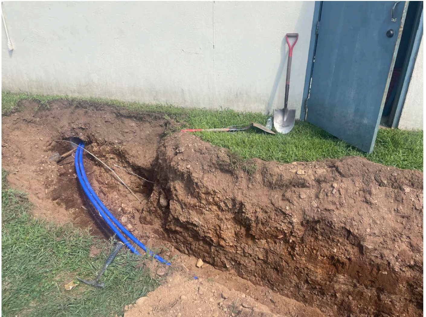
Picture 7: View of the two 1.5" polyethylene water lines that Ludlow installed, where it was run into the south side of the recreation center located on Pickett Lane. View to the northwest.
