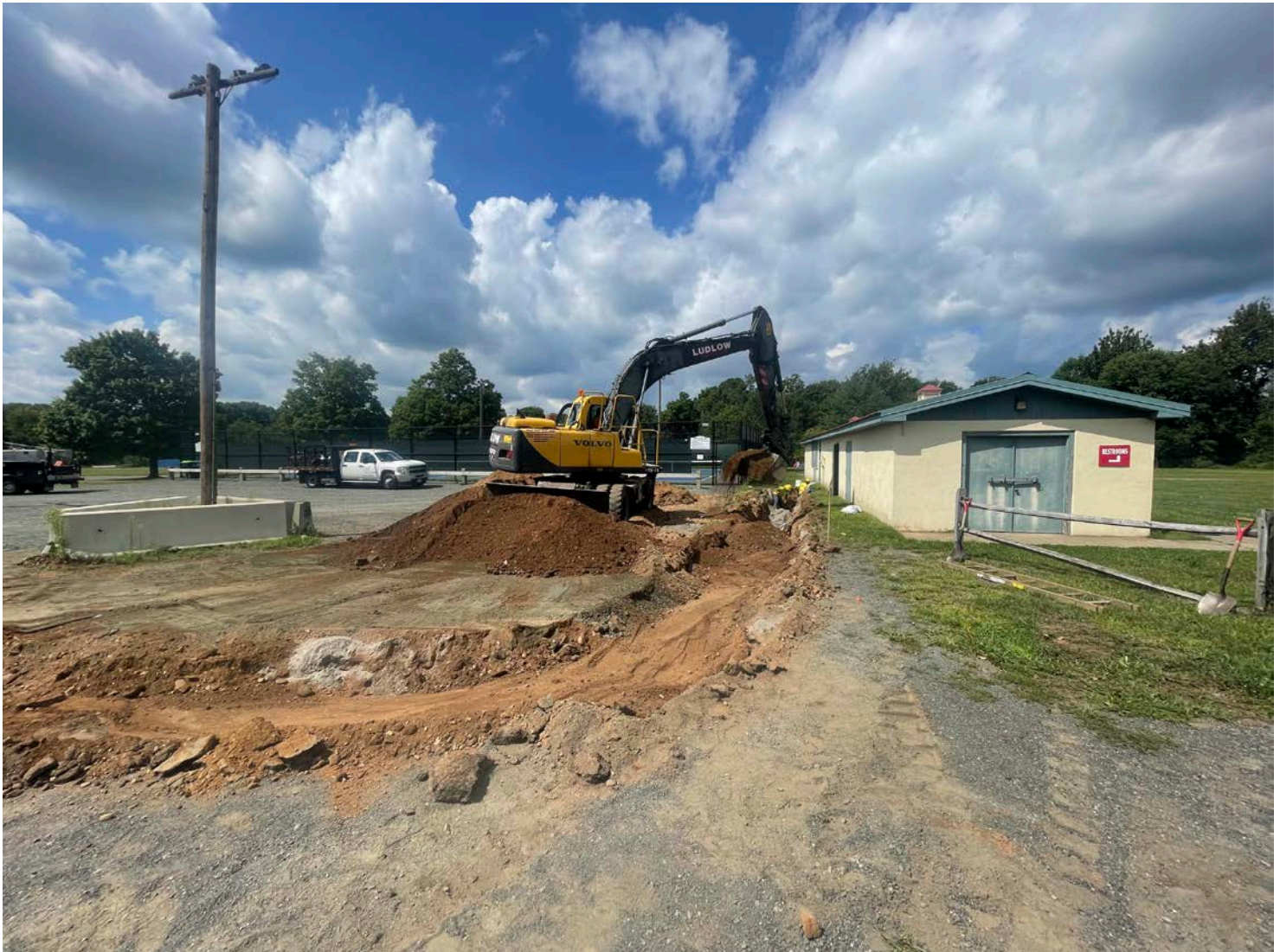
Picture 9: Ludlow placing native fill over the sand they placed over the two 1.5” polyethylene water lines that they Ludlow installed on the south side of the recreation center located on Pickett Lane. View to the west.
