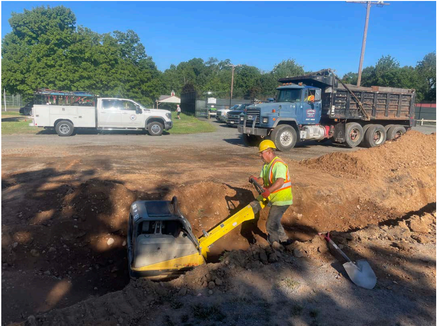
Picture 5: Ludlow compacting fill that was placed over the caution tape and sand they placed on top of the two 1.5" polyethylene water lines that Ludlow installed to the north of the two meter vaults they installed at Station ~516+55. View to the west.
