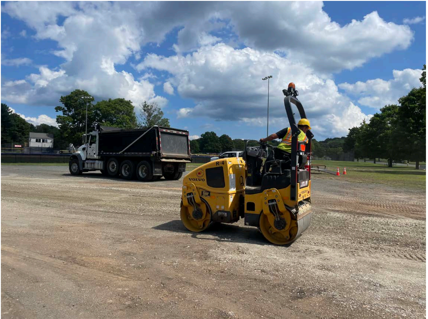
Picture 10: Ludlow compacting the fill they backfilled over the sand and caution tape that was placed over the two 1.5" polyethylene water lines that they installed today. View to the east.
