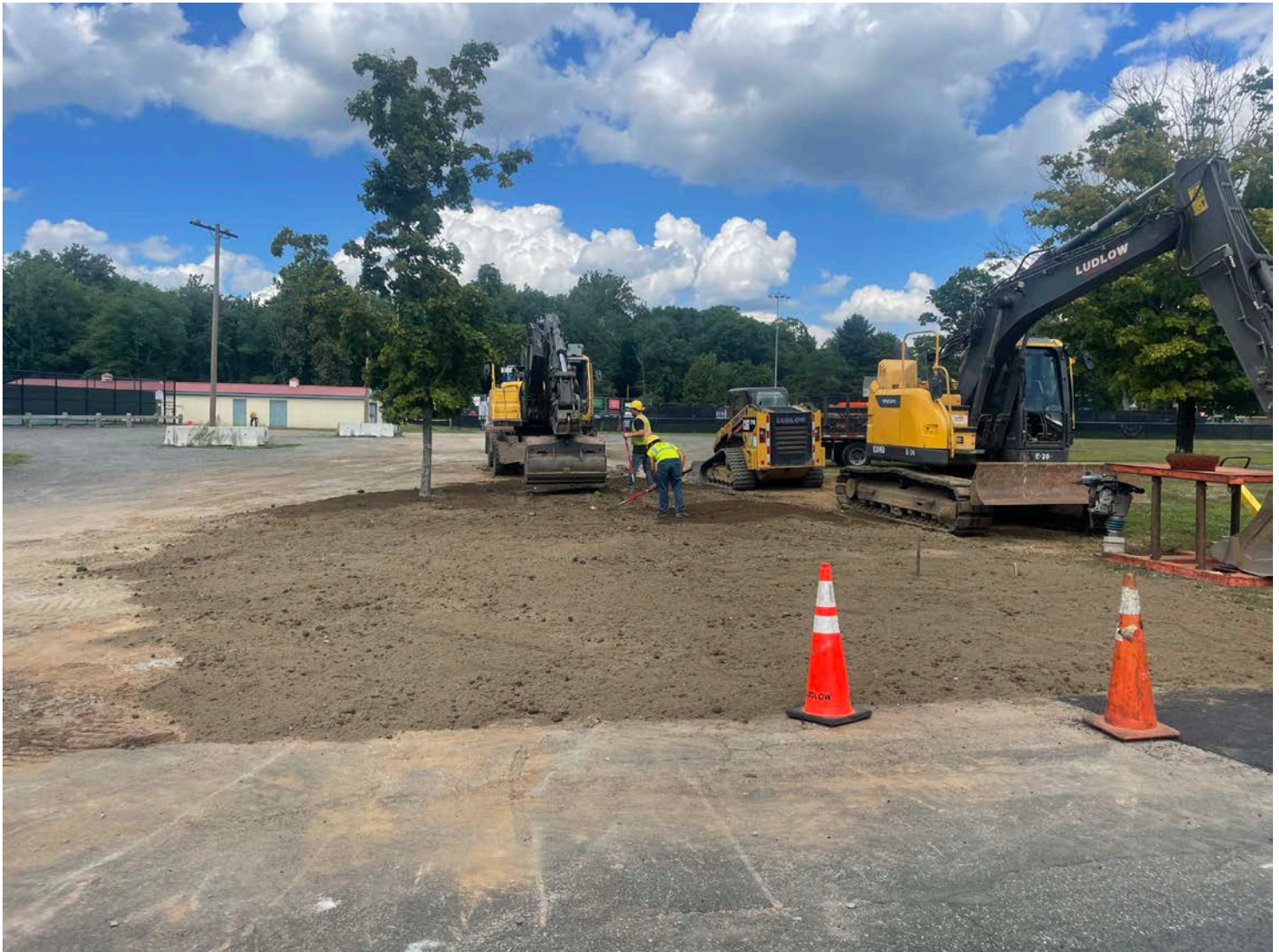
Picture 12: Ludlow placing loam and grass seed on the north side of Pickett Lane after they installed two 1.5” polyethylene water lines. View to the north.
