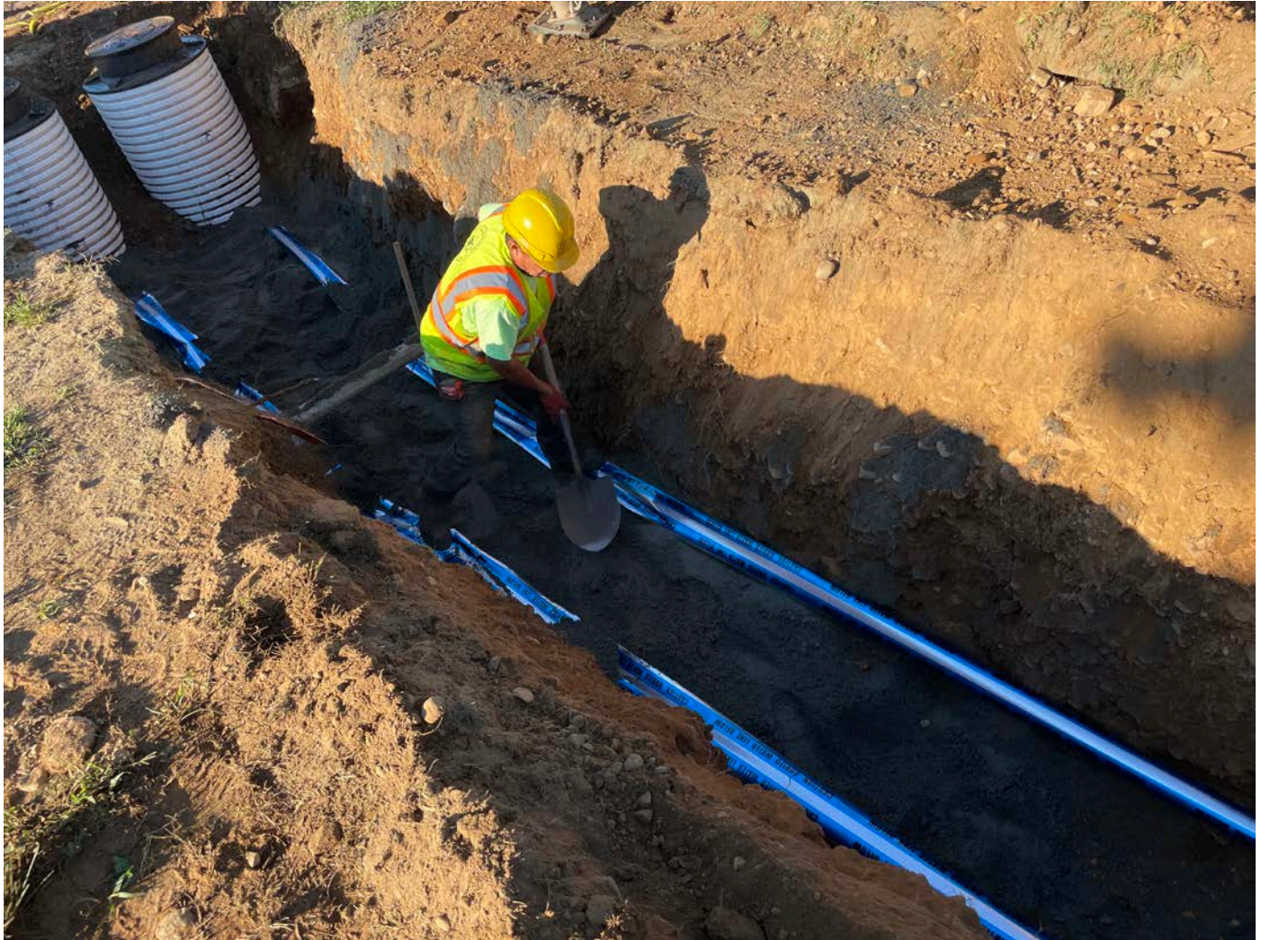
Picture 3: Ludlow placing sand followed by caution tape over the two 1.5" polyethylene water lines they are installing to the north of the two meter vaults they installed at Station ~516+55. View to the southwest.
