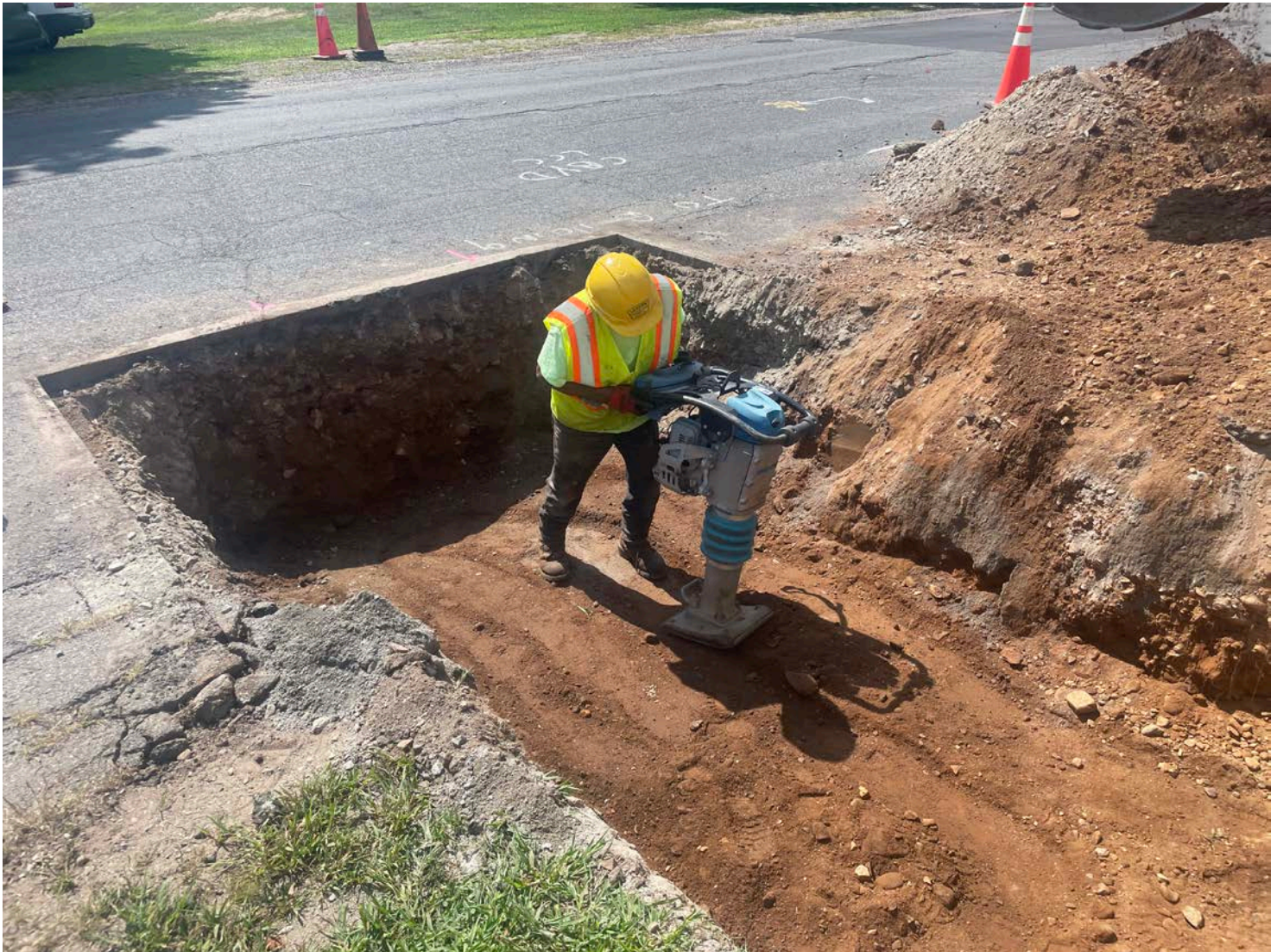
Picture 10: Ludlow using a jumping jack to compact the fill they placed over the two 1.5" copper water service lines they installed at Station ~516+55. View to the southwest.
