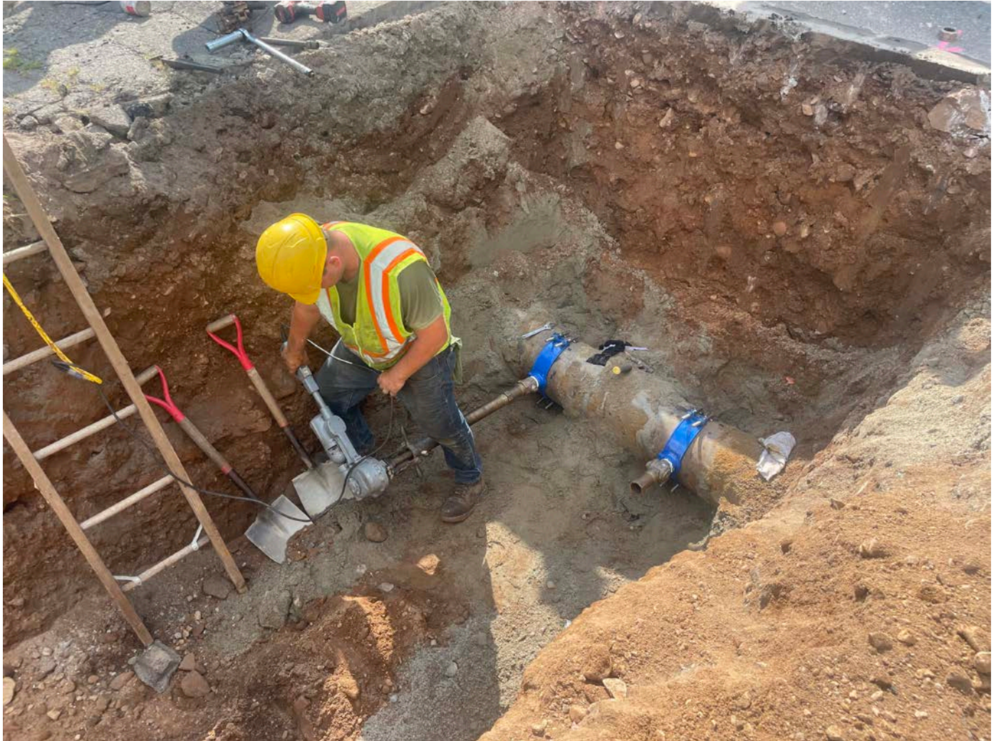
Picture 5: Ludlow tapping the 12" DIP water line they previously installed on the north side of Pickett Lane at Station ~516+55 to install the second of two corporation stops. View to the southeast.
