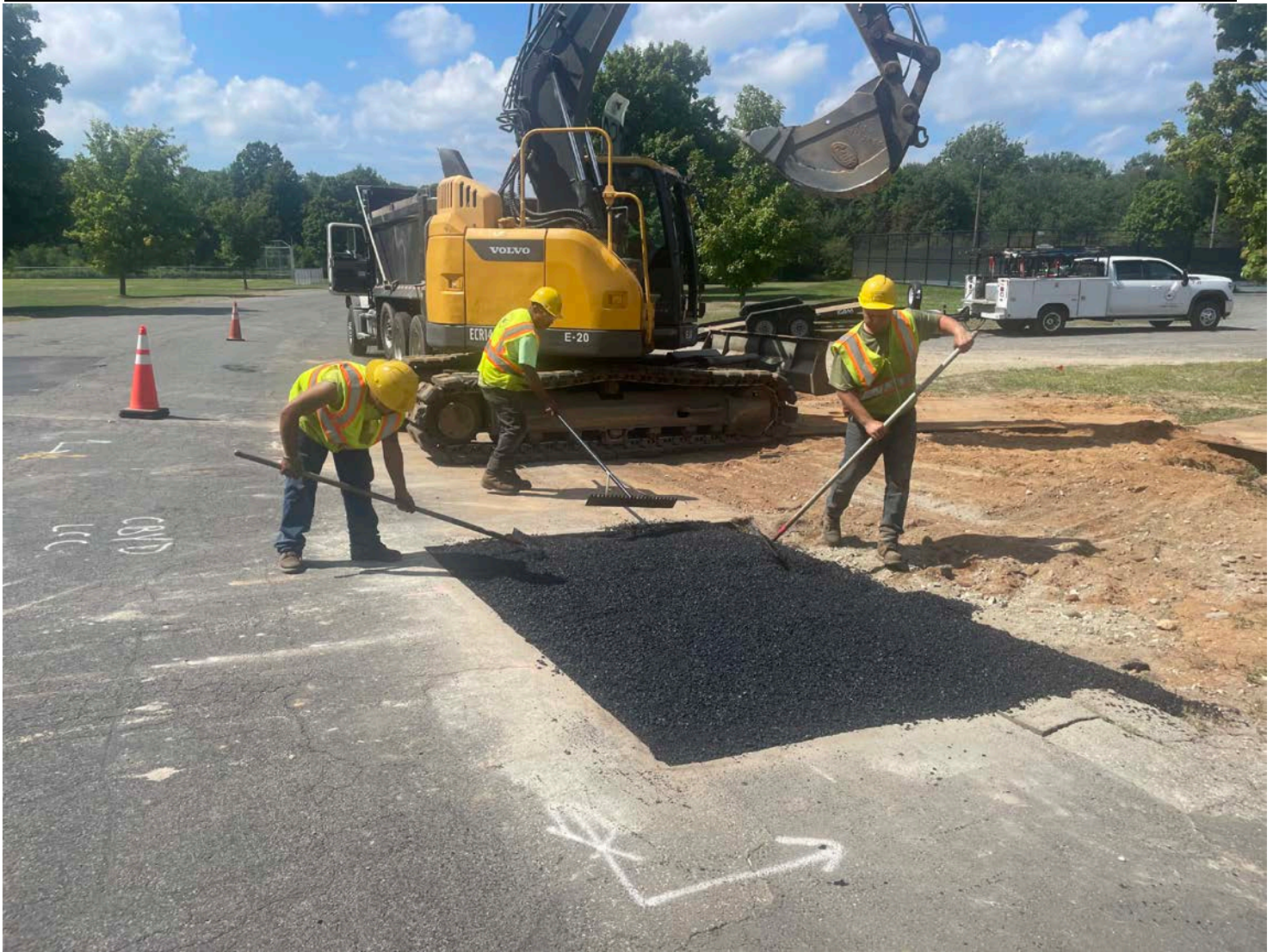
Picture 11: Ludlow placing the first of two lifts of temporary pavement at Station ~516+55 on Pickett Lane. View to the west.
