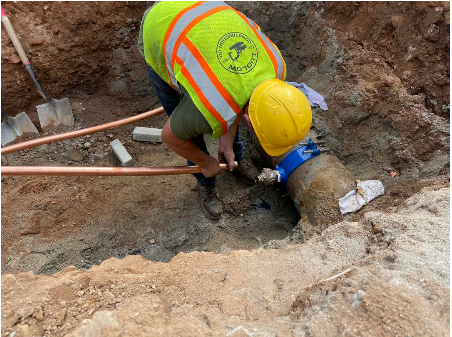
Picture 6: Ludlow connecting 1.5” copper water service line one of the two corporation stops they installed this morning on the 12” DIP water line they previously installed on the north side of Pickett Lane at Station ~516+55. View to the southeast.
