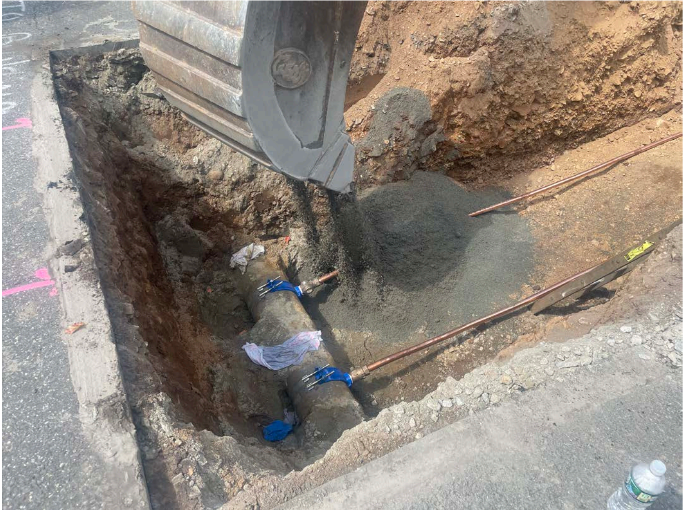
Picture 8: Ludlow placing sand above and below the two 1.5" copper water service lines they connected to the 12" DIP water line located on the north side of Pickett Lane at Station ~516+55. View to the west.
