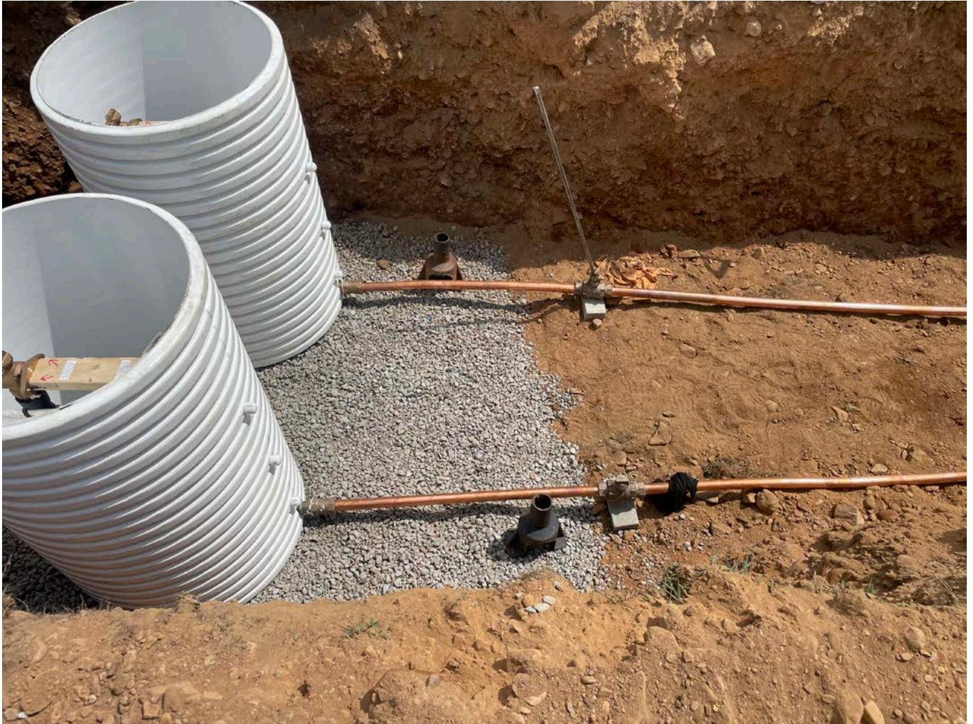
Picture 7: Two curb stops, meter pits and 1.5" copper water service lines that Ludlow has installed at Station ~516+55. View to the east.
