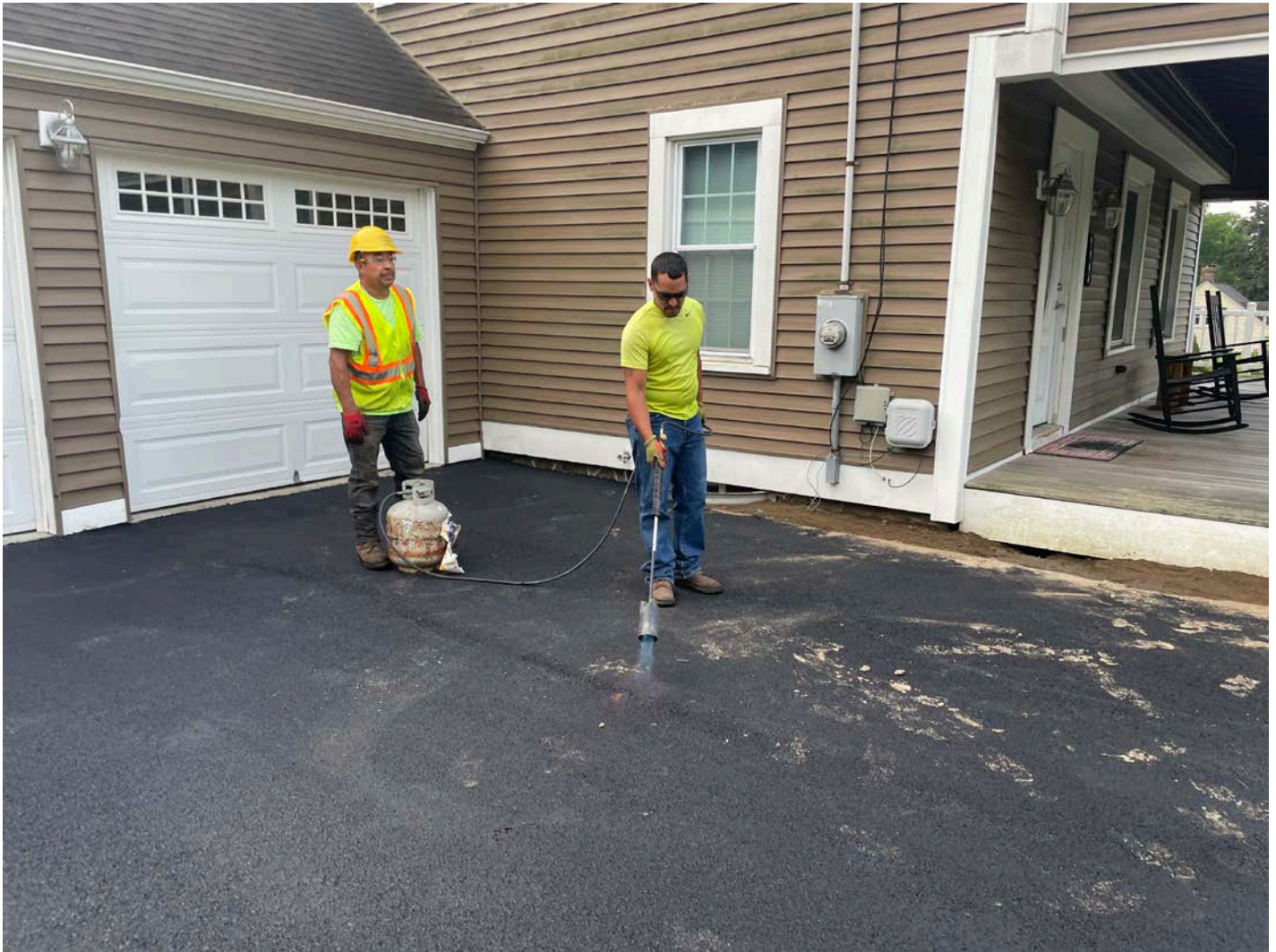
Picture 1: Ludlow using a torch to heat a high spot on the driveway located on the north side of the 245 Maple Avenue, Durham, residence. View to the southeast.
