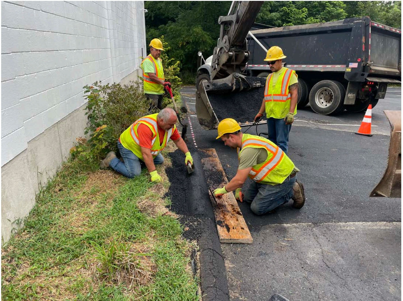
Picture 3: Ludlow repairing the asphalt curbing located on the south side of the 321 Main Street, Durham, building. View to the east.
