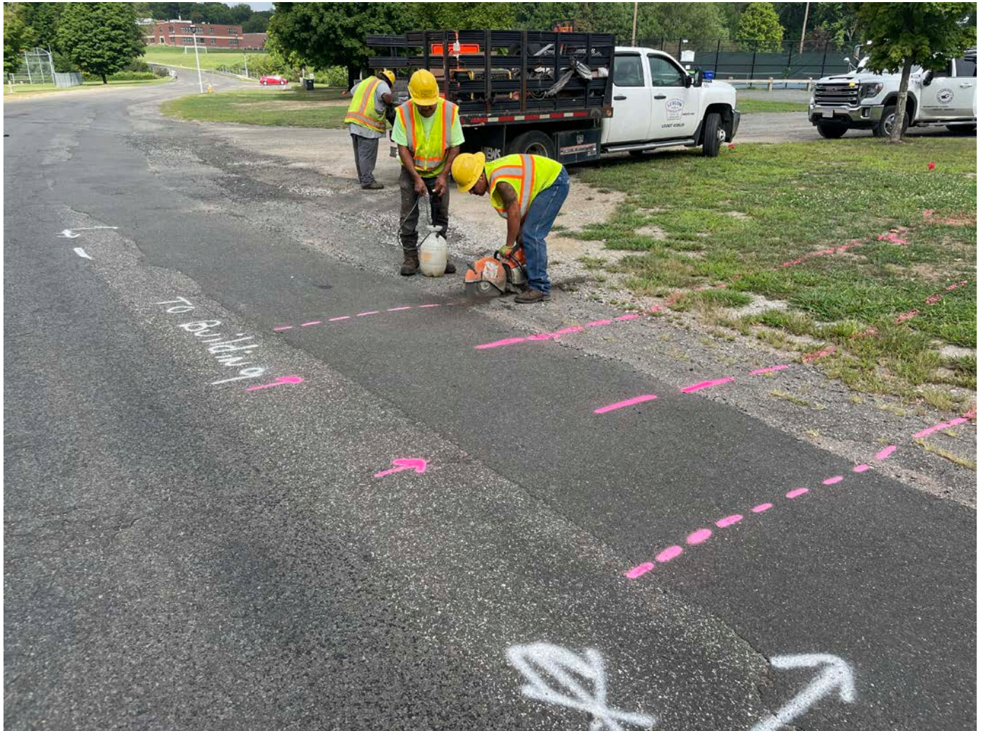
Picture 4: Ludlow saw-cutting pavement on Pickett Lane where they are preparing to install two 1.5" water service lines at Station ~516+50. View to the northwest.
