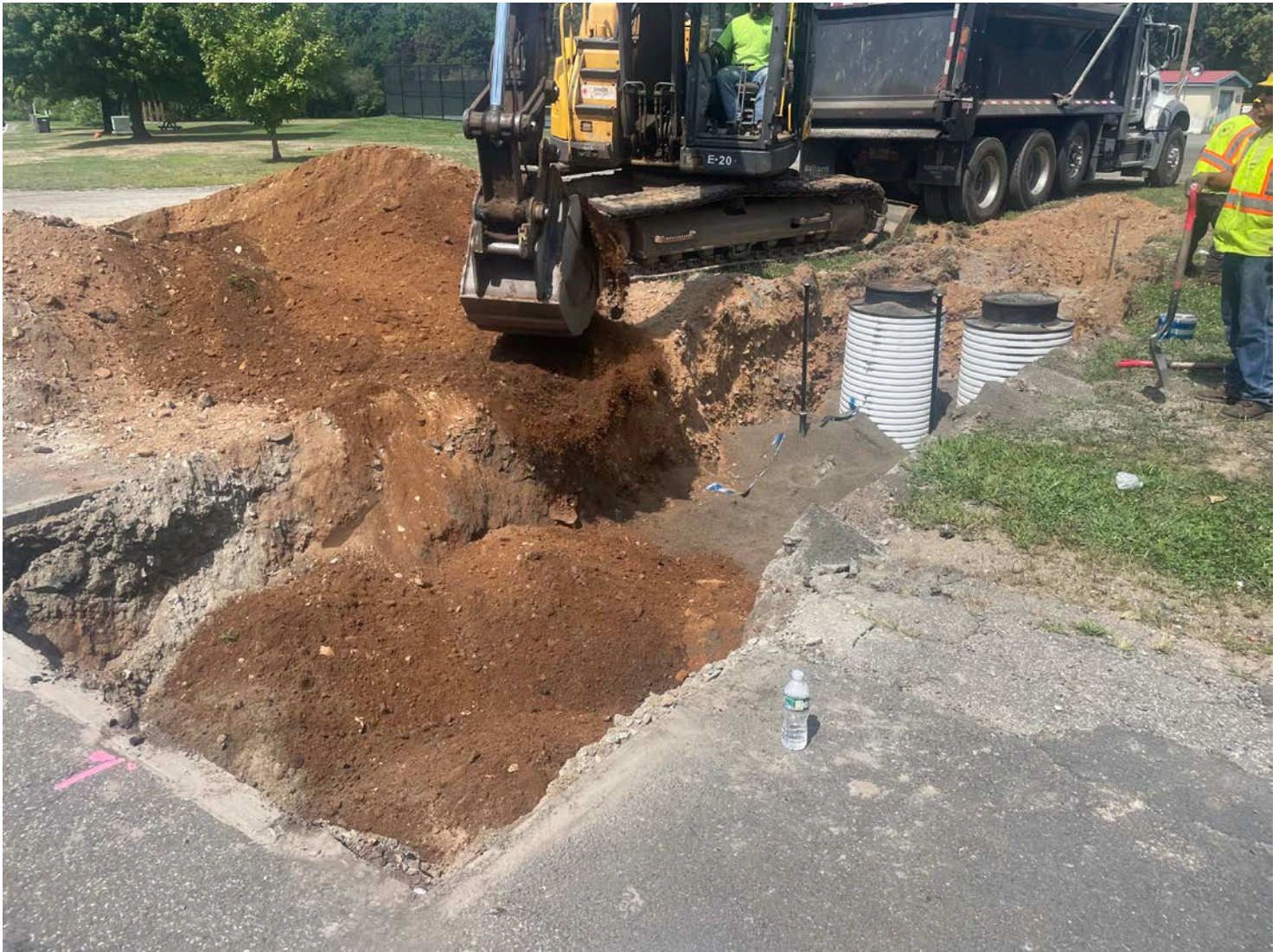
Picture 9: Ludlow placing native fill over the sand they placed over the two 1.5" copper water service lines that they installed between the 12" DIP water line located on the north side of Pickett Lane and the two curb stops and meter pits the placed to the north of the water line. View to the northwest.
