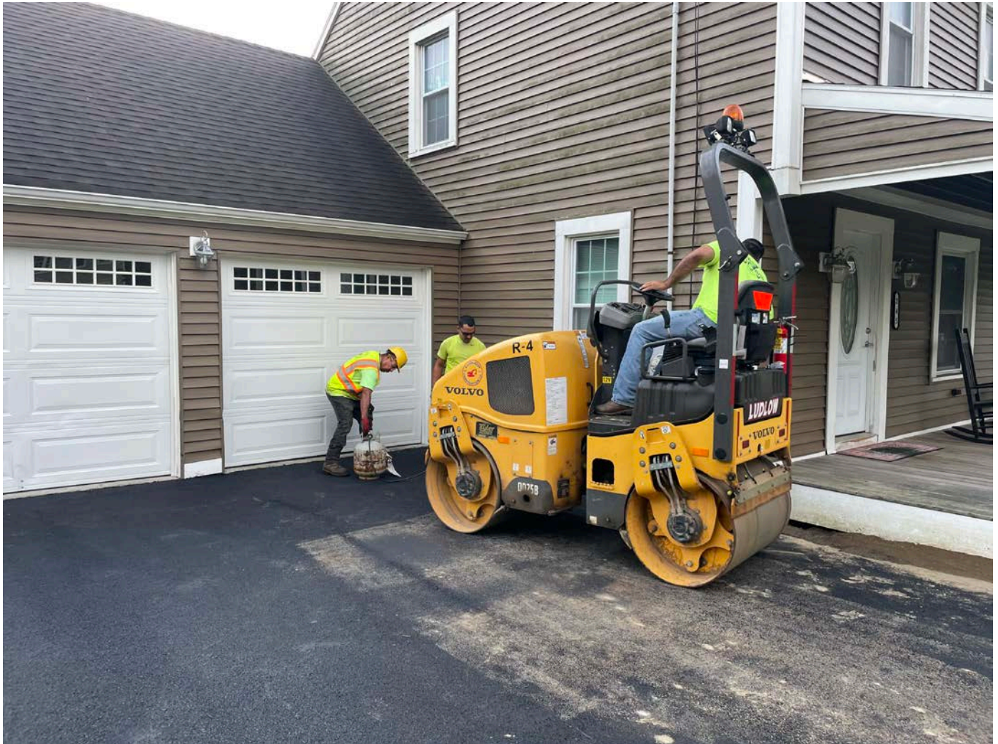
Picture 2: Ludlow rolling a high spot on the driveway located on the north side of the 245 Maple Avenue, Durham, residence after they heated the asphalt with a torch. View to the southeast.
