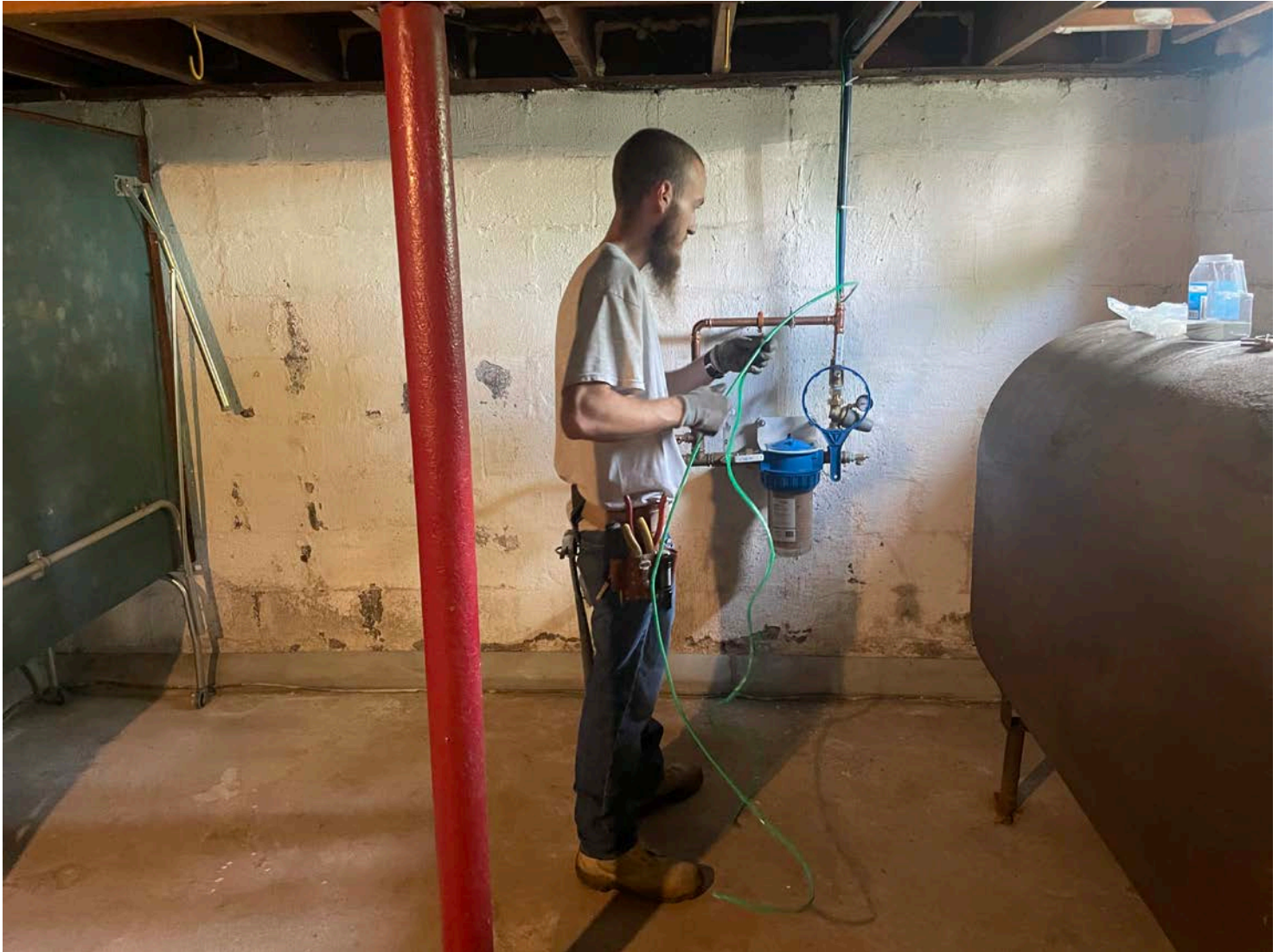
Picture 10: Apuzzo Electric preparing to install grounding lines onto the water system located at the 175R Main Street, Durham, residence.
