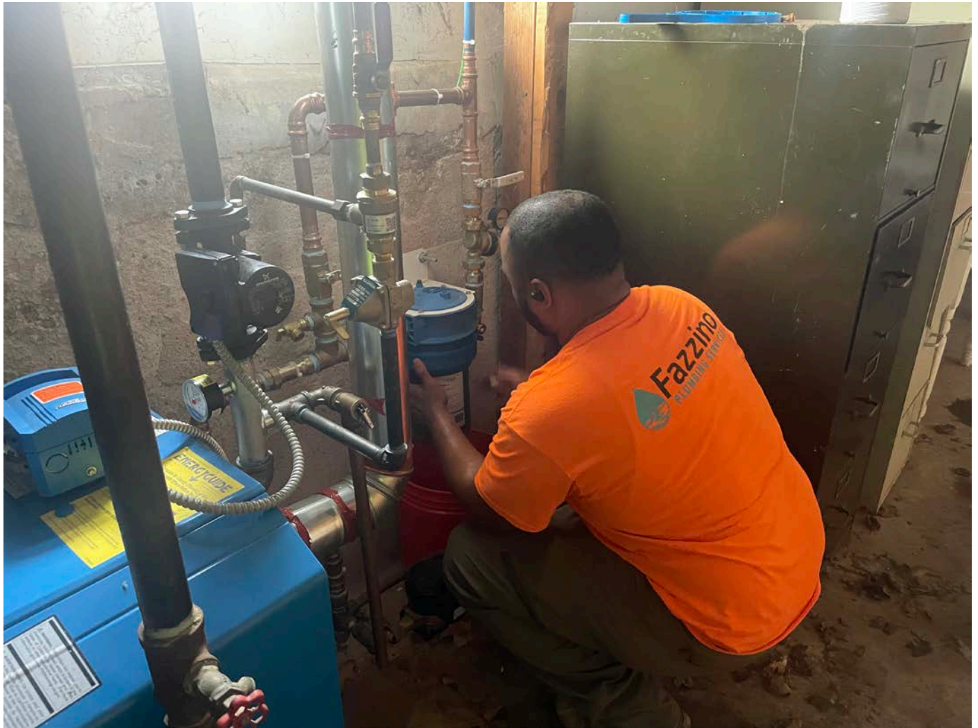
Picture 17: Fazzino Plumbing changing the filter on the water system they previously installed at the 253 Main Street, Durham, residence.
