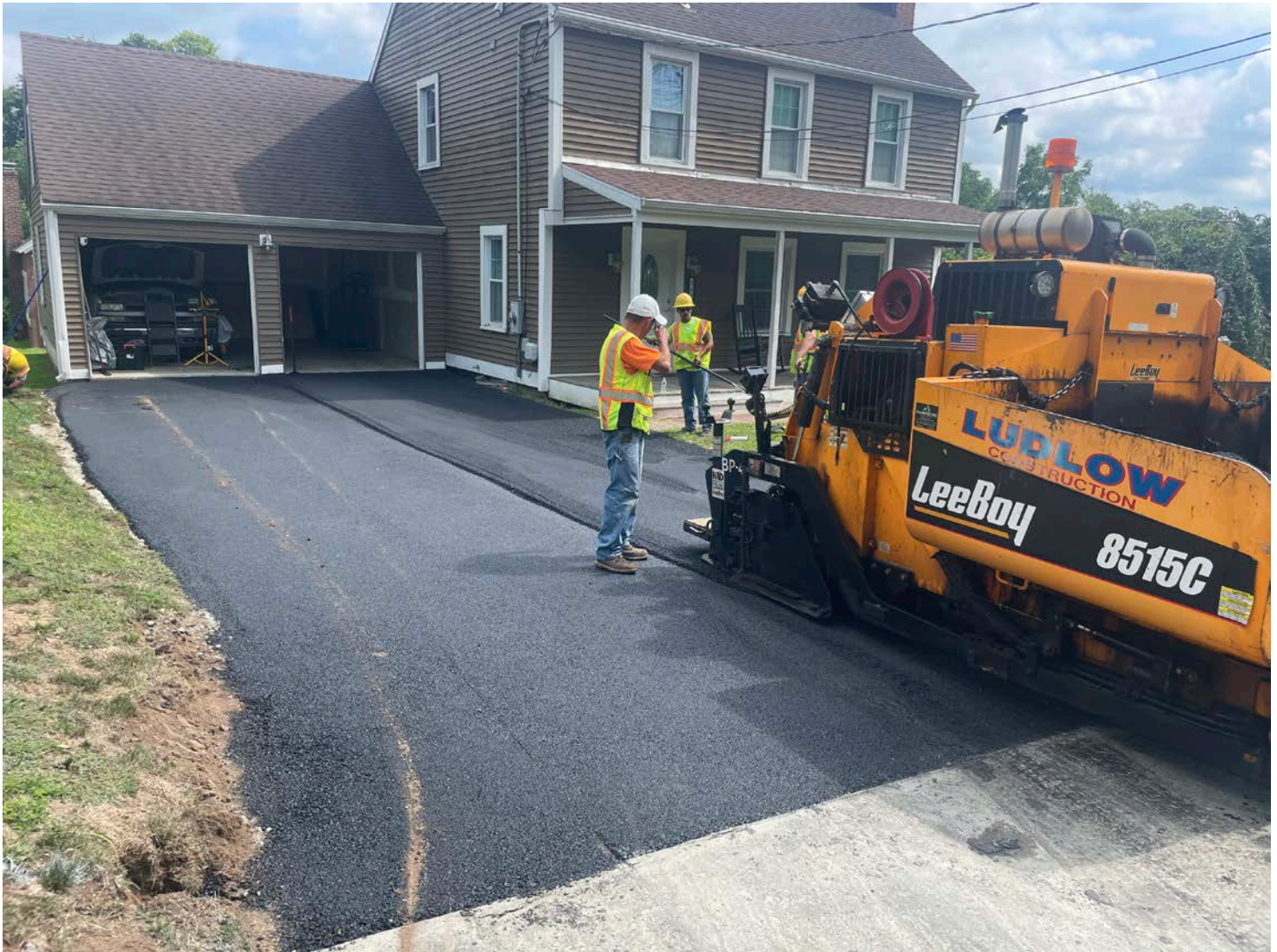
Picture 6: Ludlow starting to place the second of two lifts of asphalt onto the footprint of a portion of the driveway located on the north side of the 245 Maple Avenue property. View to the southeast.
