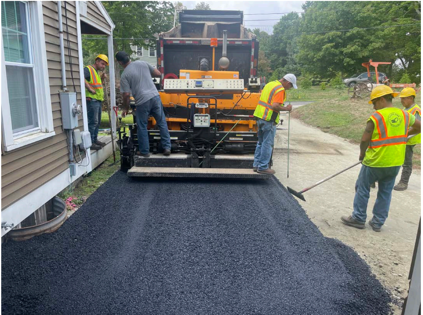
Picture 5: Ludlow starting to place the first of two lifts of asphalt onto the footprint of a portion of the driveway located on the north side of the 245 Maple Avenue property. View to the west.
