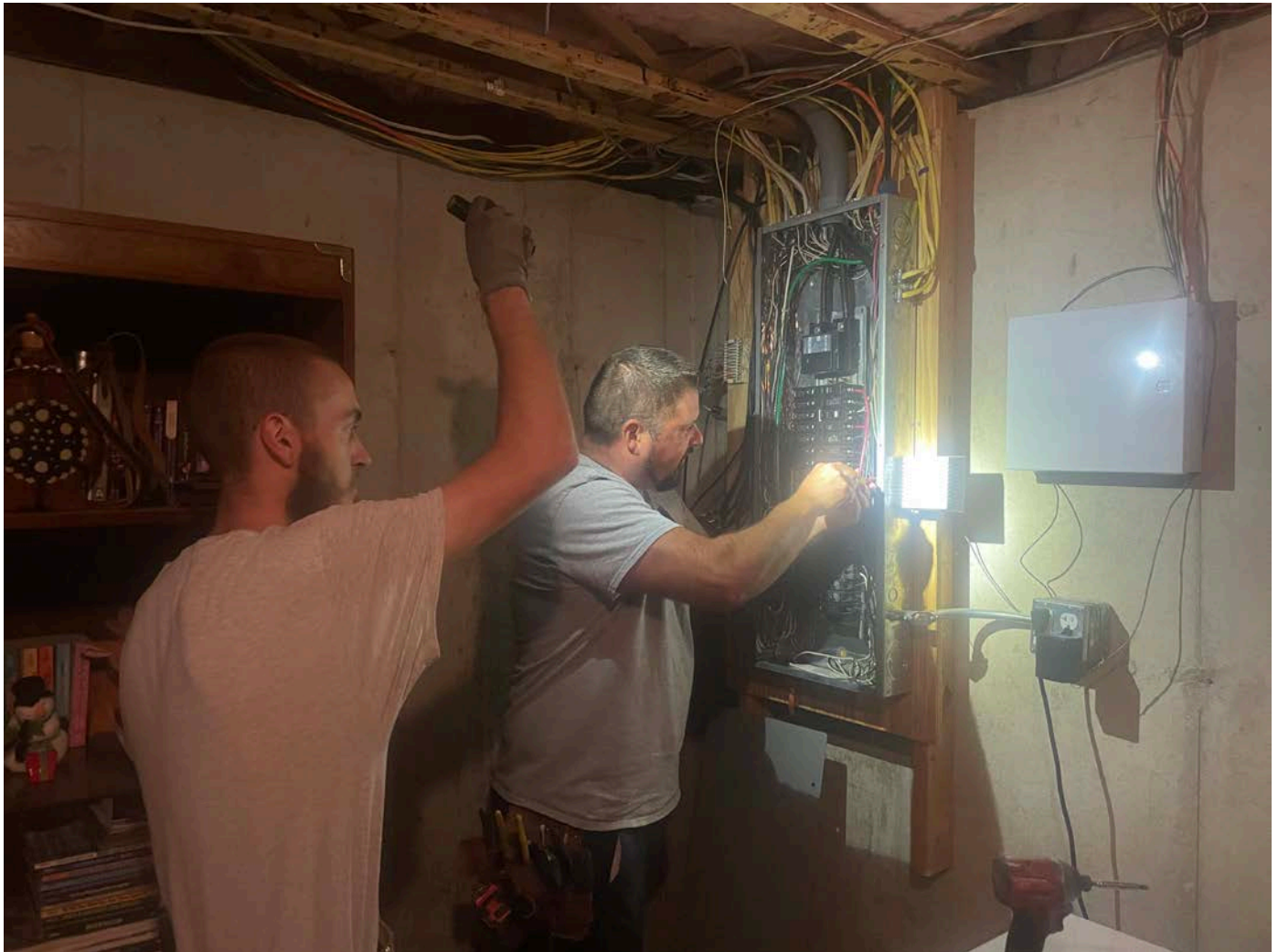
Picture 8: Apuzzo checking the wiring at the 166 Maple Avenue, Durham, residence. View to the northeast.
