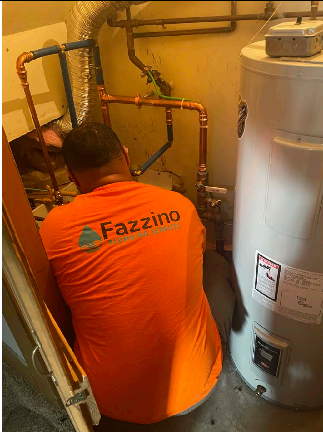
Picture 13: Fazzino Plumbing changing the filter on the water system they previously installed at the 305R Main Street, Durham, residence.
