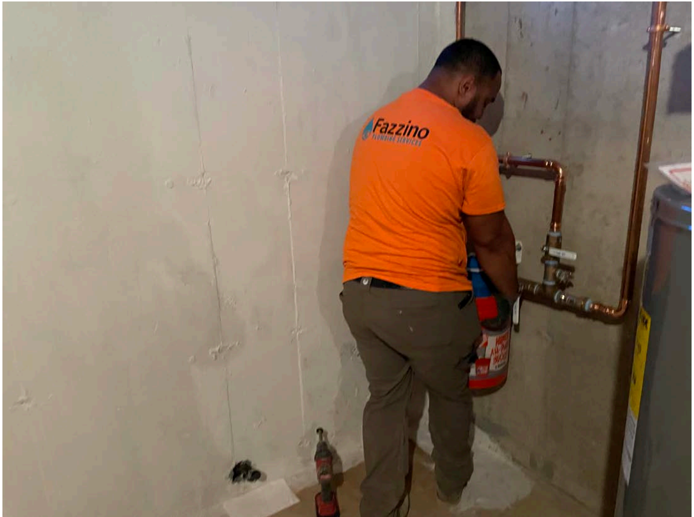
Picture 11: Fazzino Plumbing changing the filter on the water system they previously installed at the 166 Maple Avenue, Durham, residence. View to the northwest.
