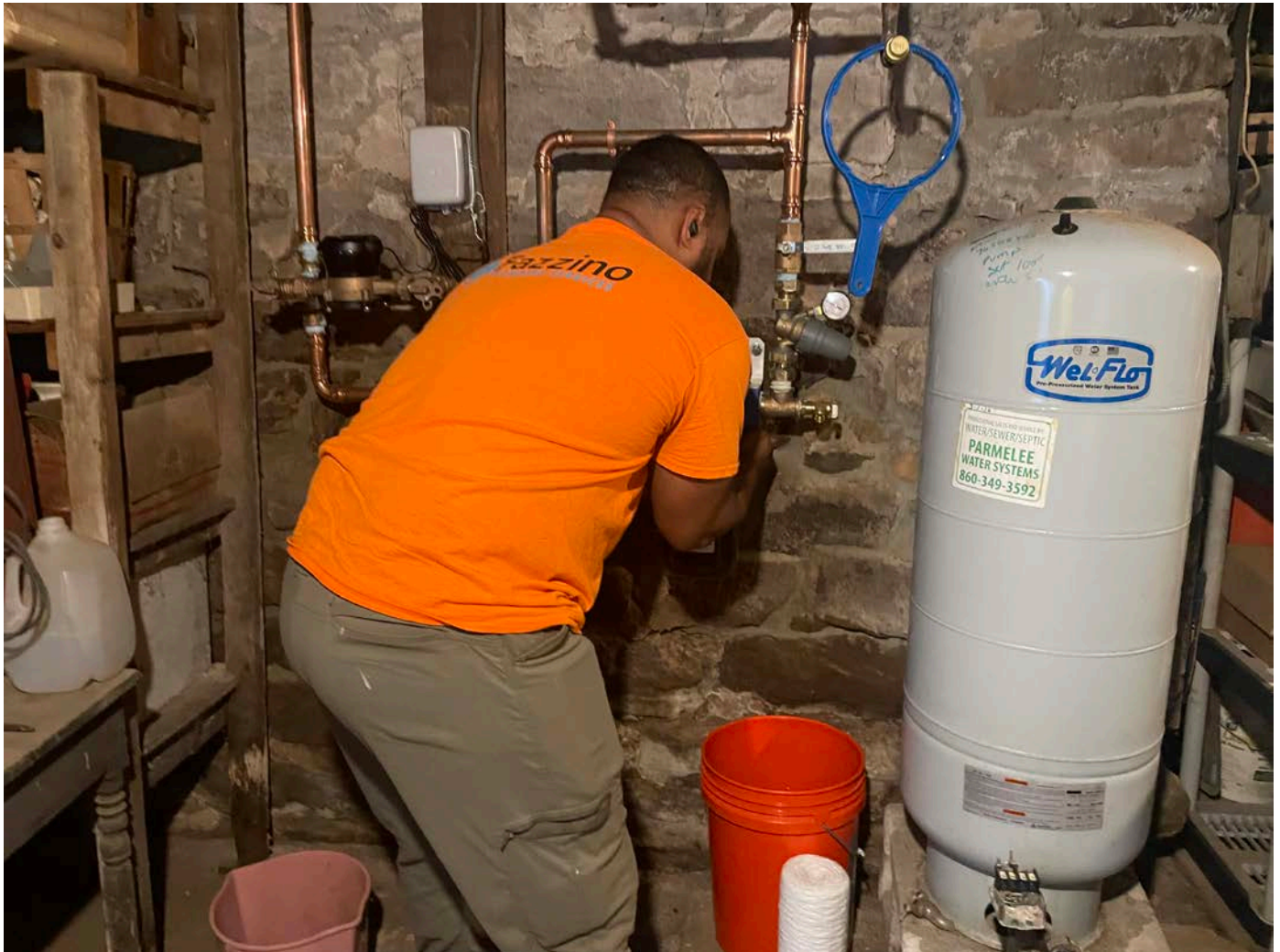
Picture 18: Fazzino Plumbing changing the filter on the water system they previously installed at the 110 Maple Avenue, Durham, residence.
