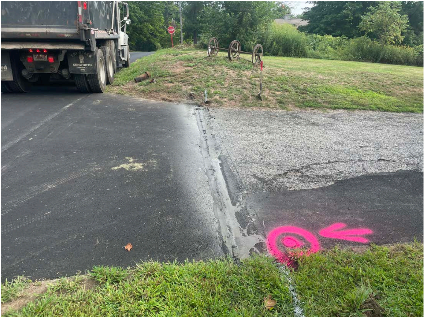
Picture 1: Driveway at 245 Maple Avenue, Durham, where Ludlow has saw-cut the pavement between the new apron that Laydon installed and the rest of the driveway. View to the north.
