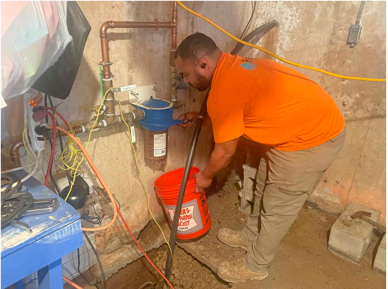
Picture 16: Fazzino Plumbing changing the filter on the water system they previously installed at the 187 Maple Avenue, Durham, residence.
