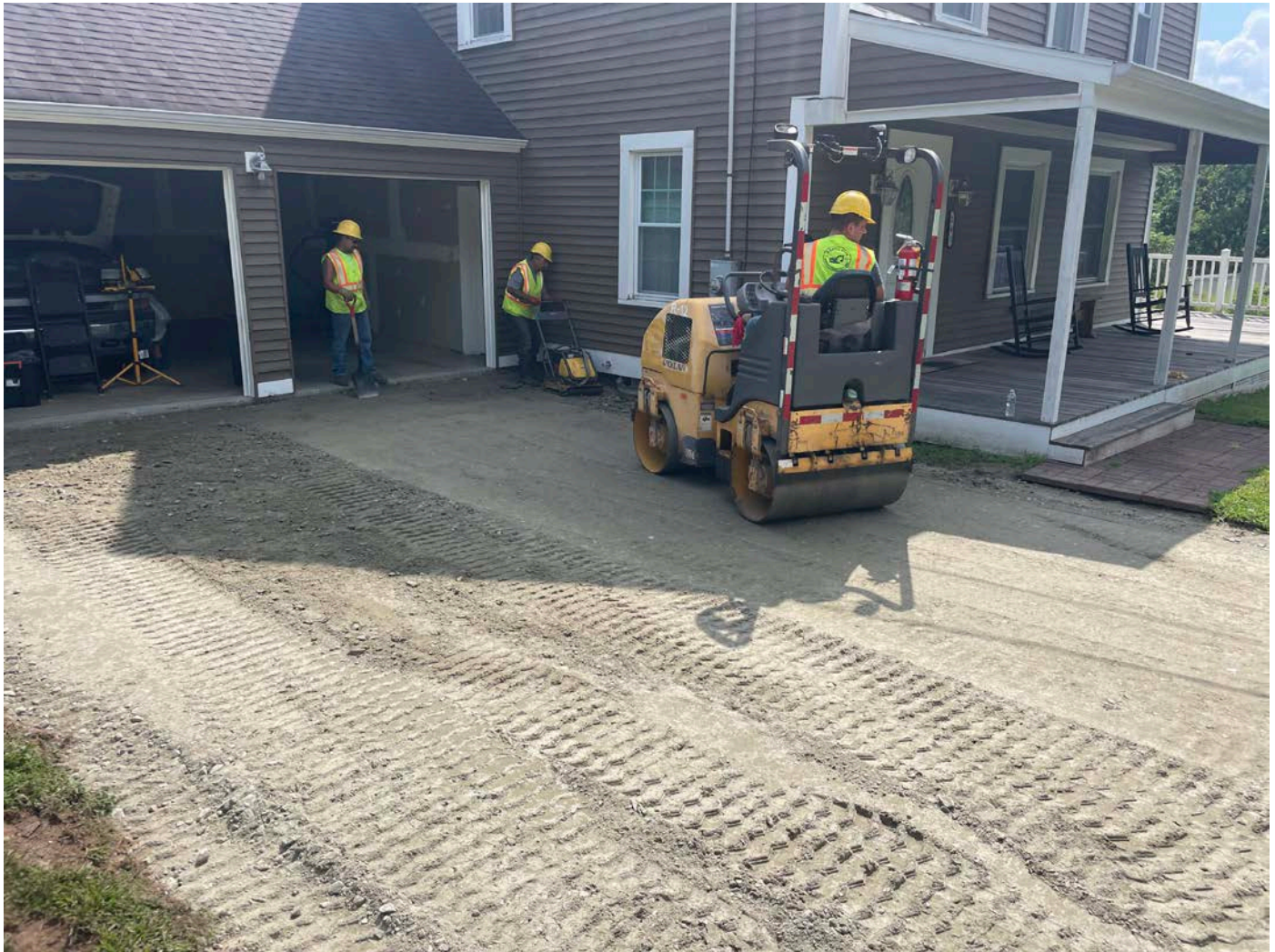
Picture 3: Ludlow using a plate compactor and a rolling compactor on 1.25” processed gravel that they placed within the footprint of a portion of the driveway located on the north side of the 245 Maple Avenue property. View to the southeast.
