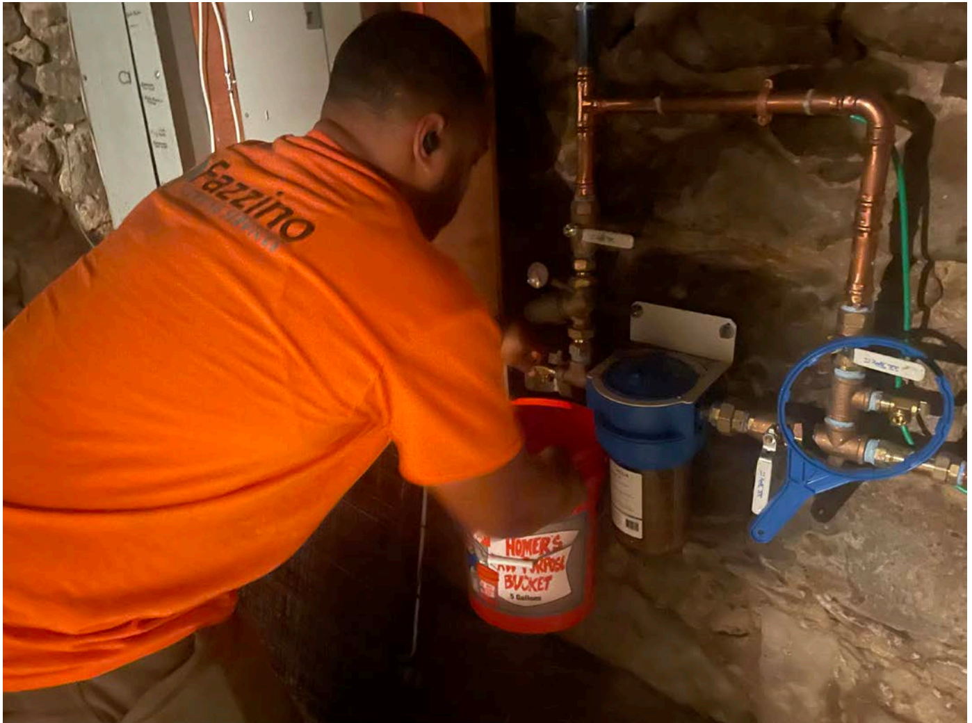
Picture 12: Fazzino Plumbing changing the filter on the water system they previously installed at the 303 Main Street, Durham, residence.
