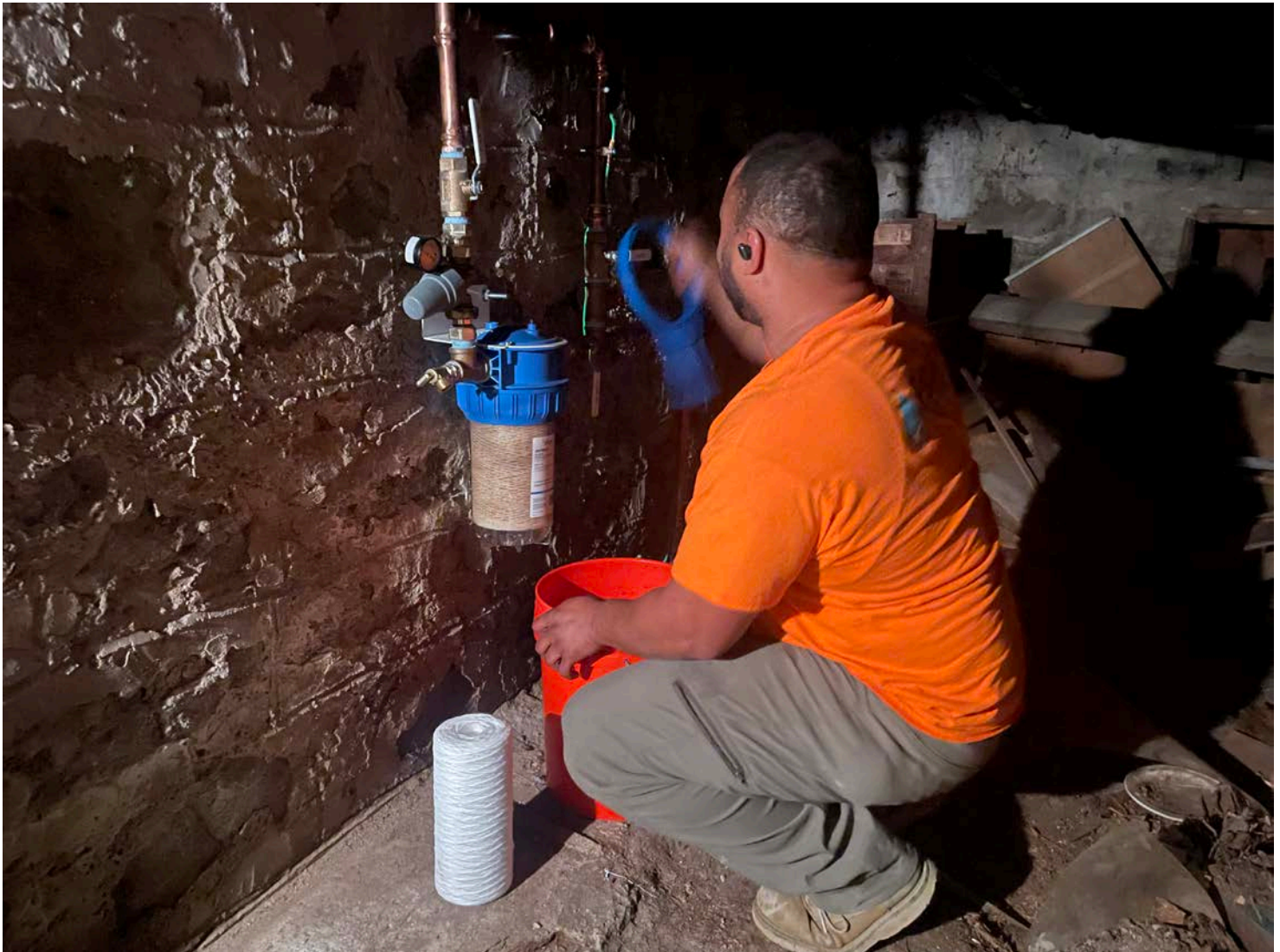
Picture 19: Fazzino Plumbing changing the filter on the water system they previously installed at the 289 Main Street, Durham, residence.
