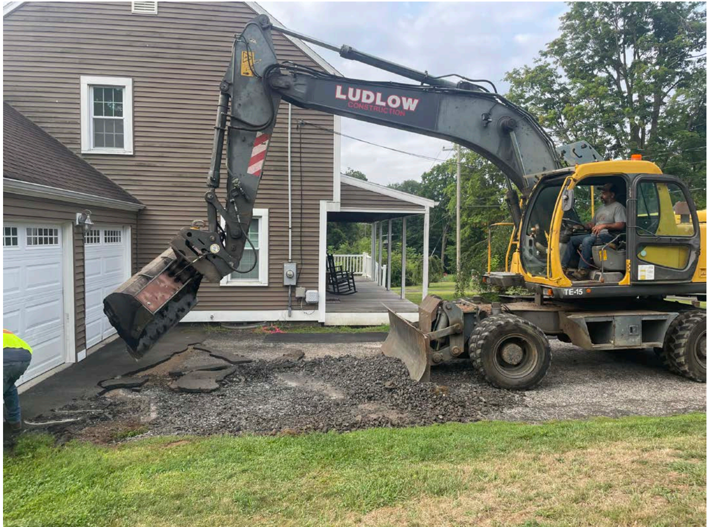
Picture 2: Ludlow removing pavement from the driveway located on the north side of the 245 Maple Avenue residence as they prepare to repave a portion of the driveway. View to the south.
