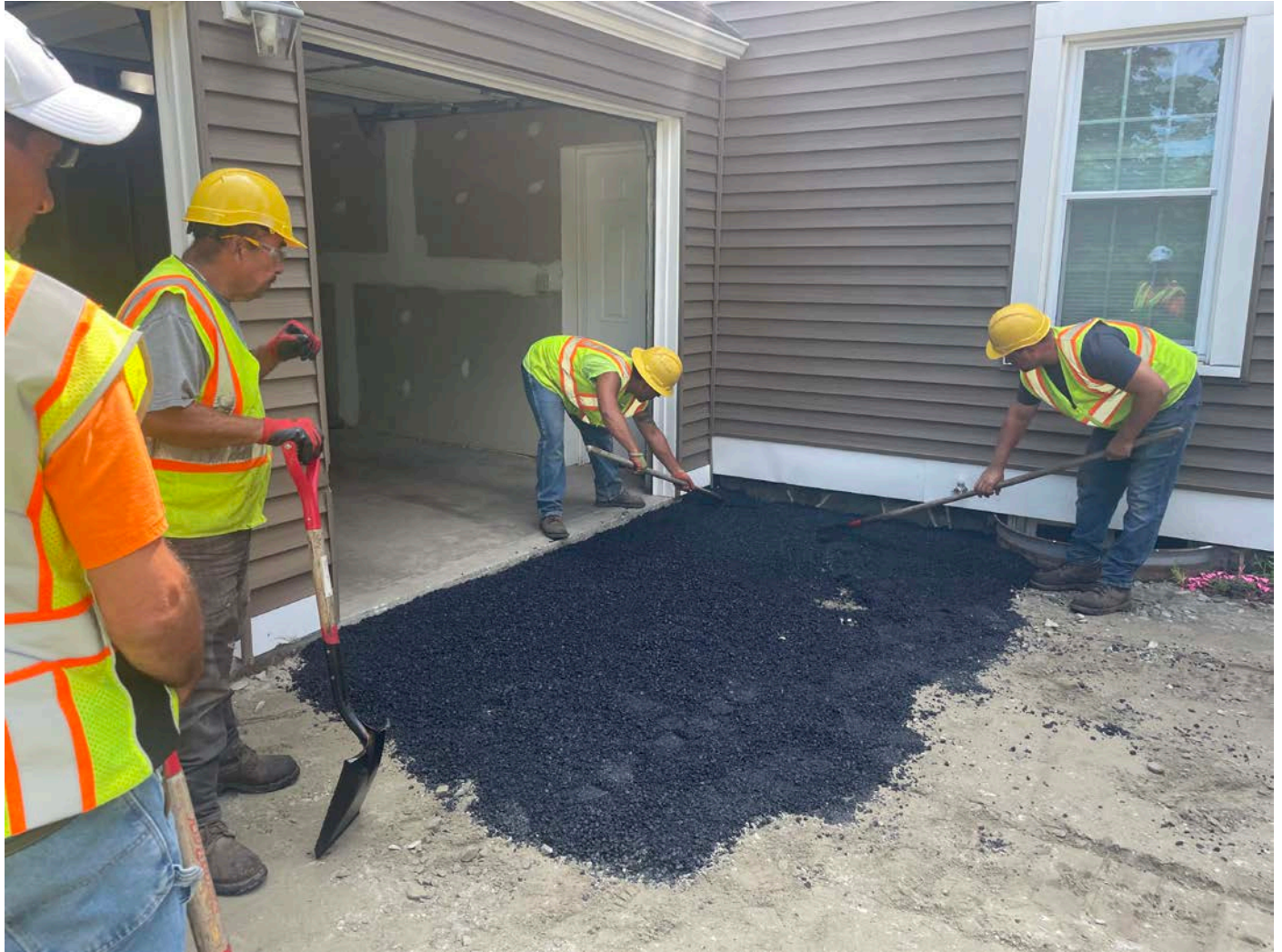
Picture 4: Ludlow starting to place the first of two lifts of asphalt onto the footprint of a portion of the driveway located on the north side of the 245 Maple Avenue property. View to the southeast.
