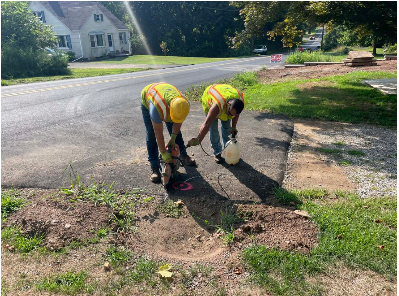
Picture 5: Ludlow saw-cutting the pavement on the 236 Maple Avenue property driveway in order to daylight and raise the curb stop. View to the south.
