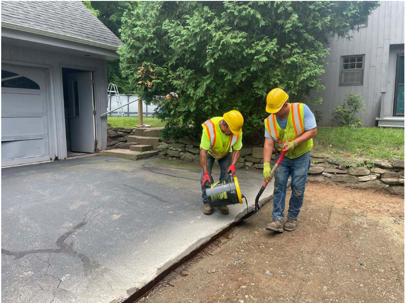
Picture 8: Ludlow applying tack coat to the cut edge of the pavement on the east side of the trench overcut on the footprint of the 119 Maple Avenue property driveway. View to the southeast.
