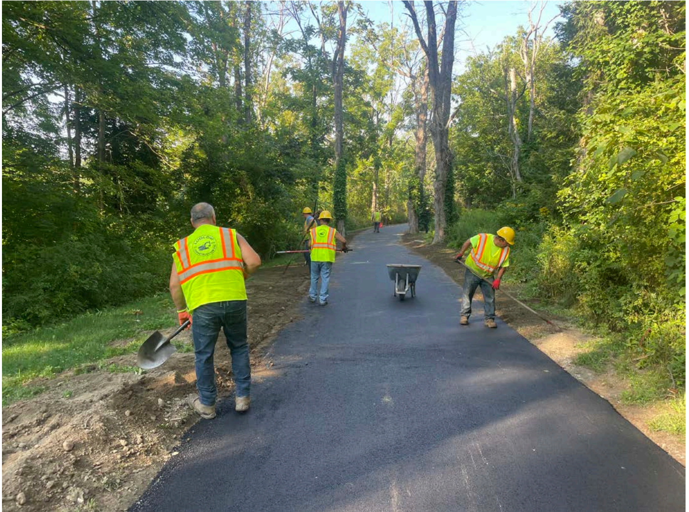
Picture 2: Ludlow grading loam that they placed on the sides of the driveway footprint of the 212R Maple Avenue, Durham, property. View to the west.
