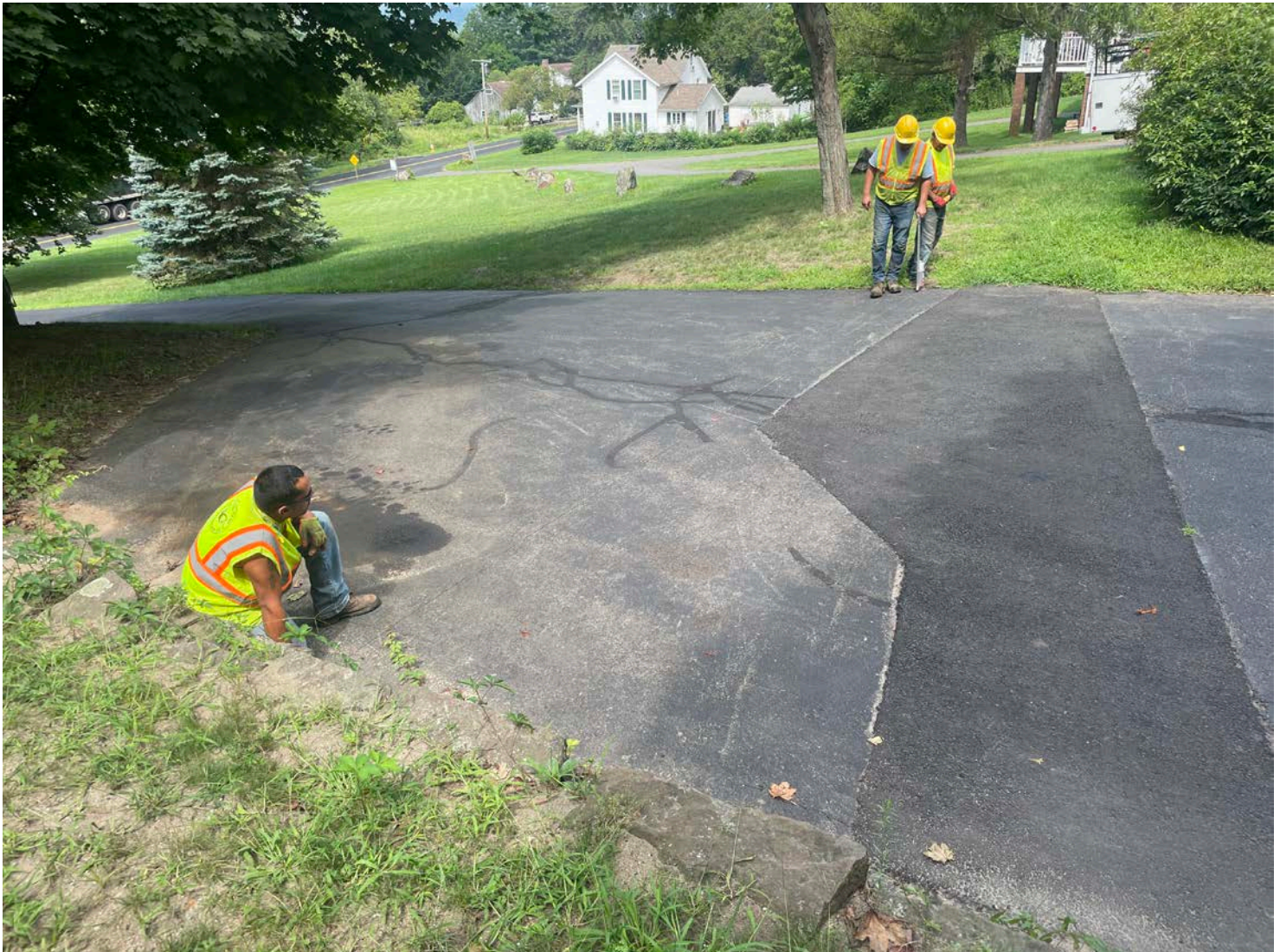
Picture 6: Ludlow marking out the cut lines on the trench overcut on the driveway of the 119 Maple Avenue property. View to the north.
