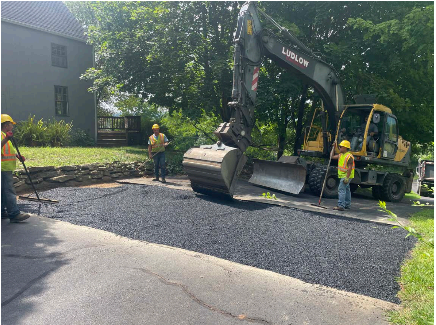
Picture 9: Ludlow placing the first of two lifts of asphalt on the footprint of the 119 Maple Avenue trench overcut. View to the southwest.
