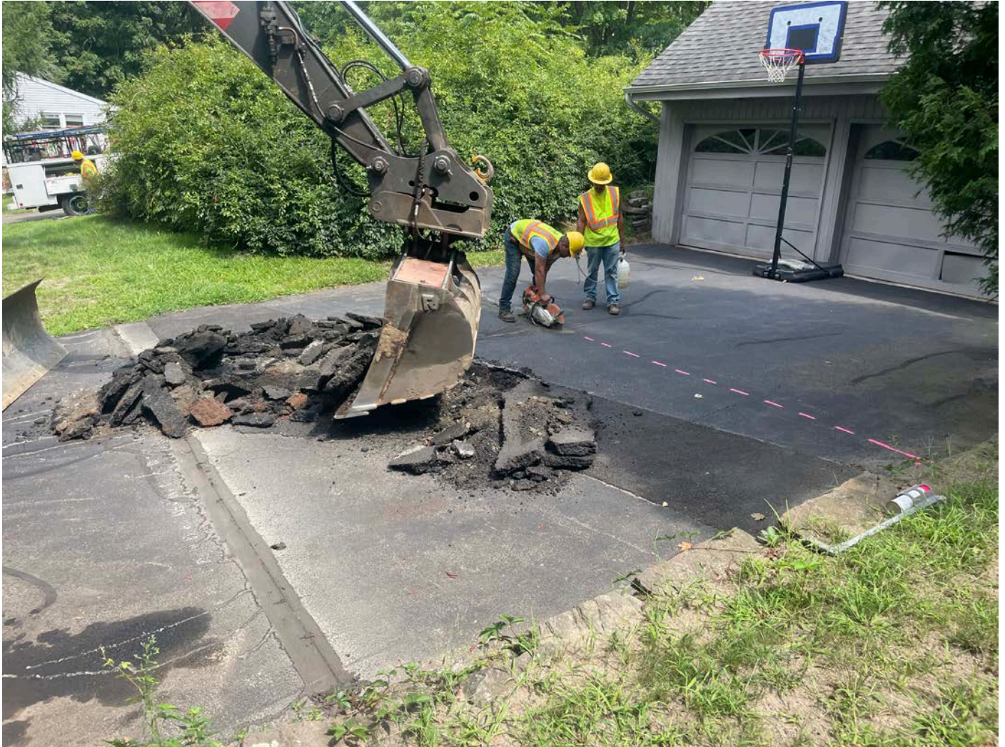
Picture 7: Ludlow saw-cutting the footprint of the trench overcut on the east side of the 119 Maple Avenue driveway. View to the northeast.
