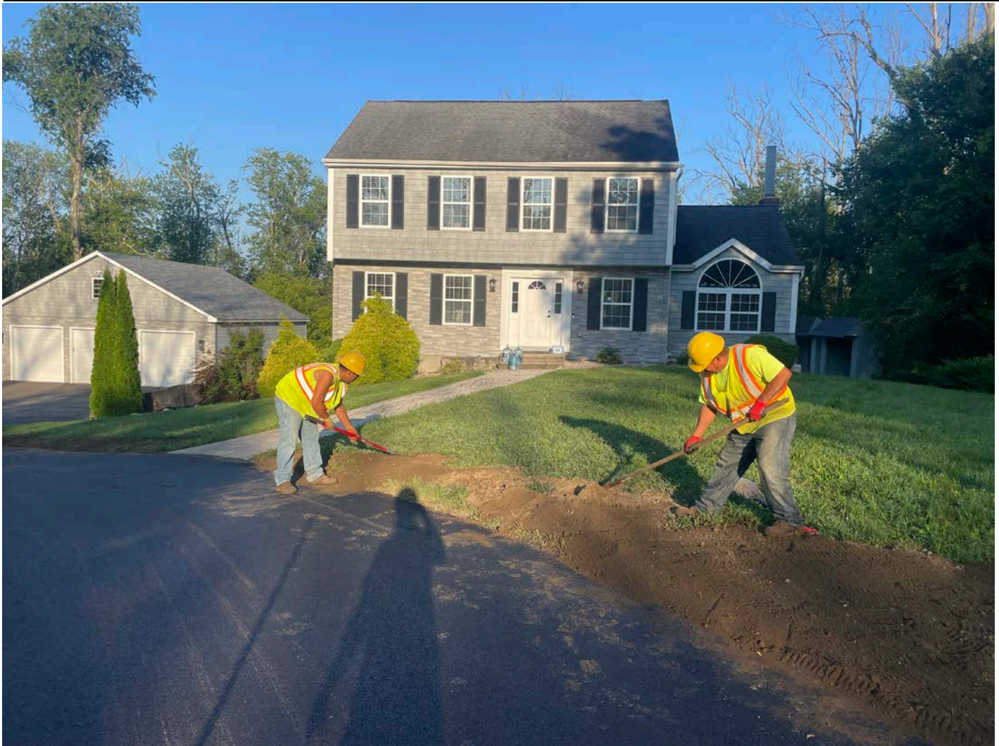
Picture 1: Ludlow grading loam that they placed on the sides of the driveway footprint of the 212R Maple Avenue, Durham, property. View to the west.
