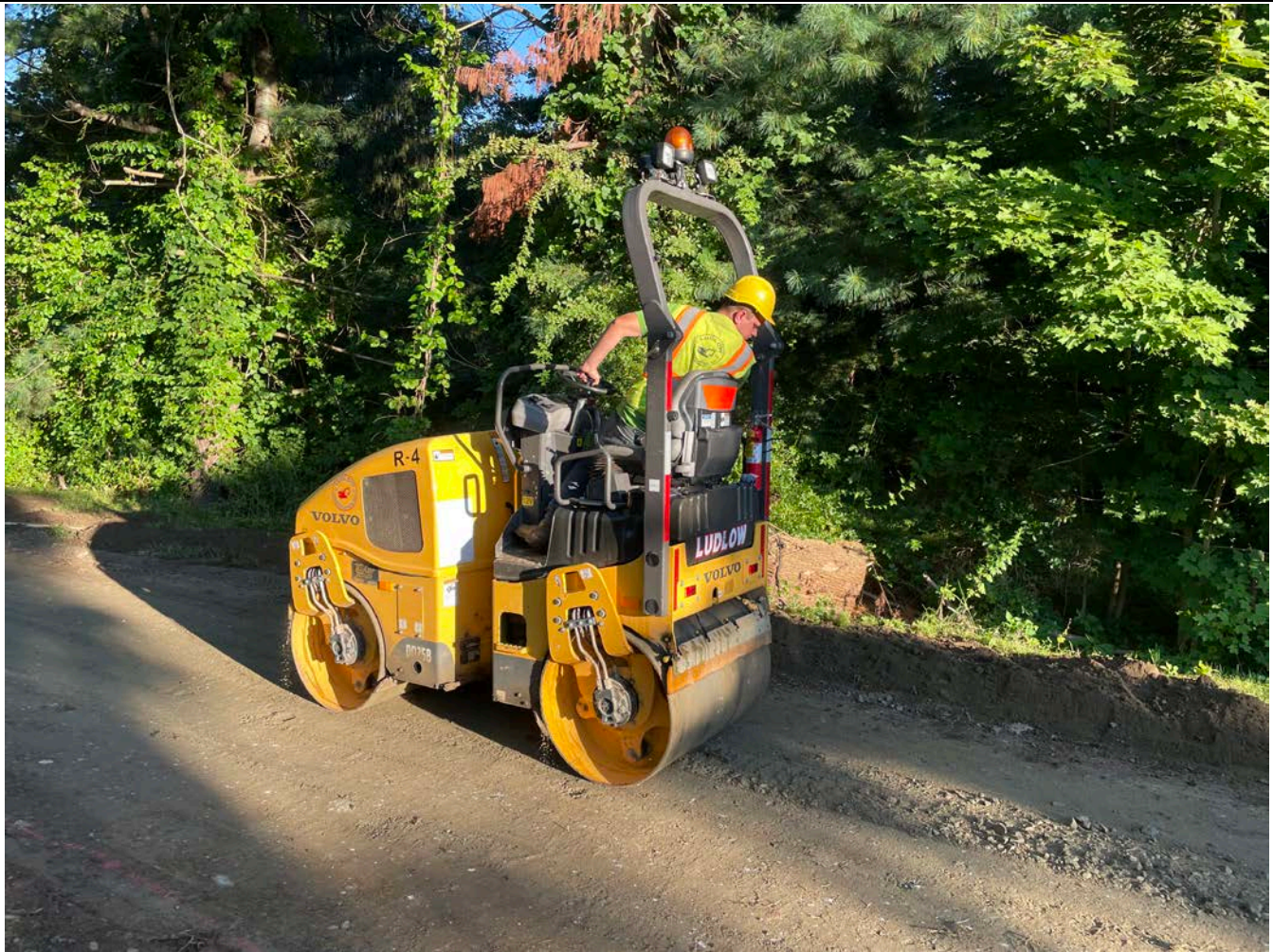
Picture 1: Ludlow compacting 1.25" processed gravel on the driveway footprint of the 212R Maple Avenue, Durham, property. View to the northwest.
