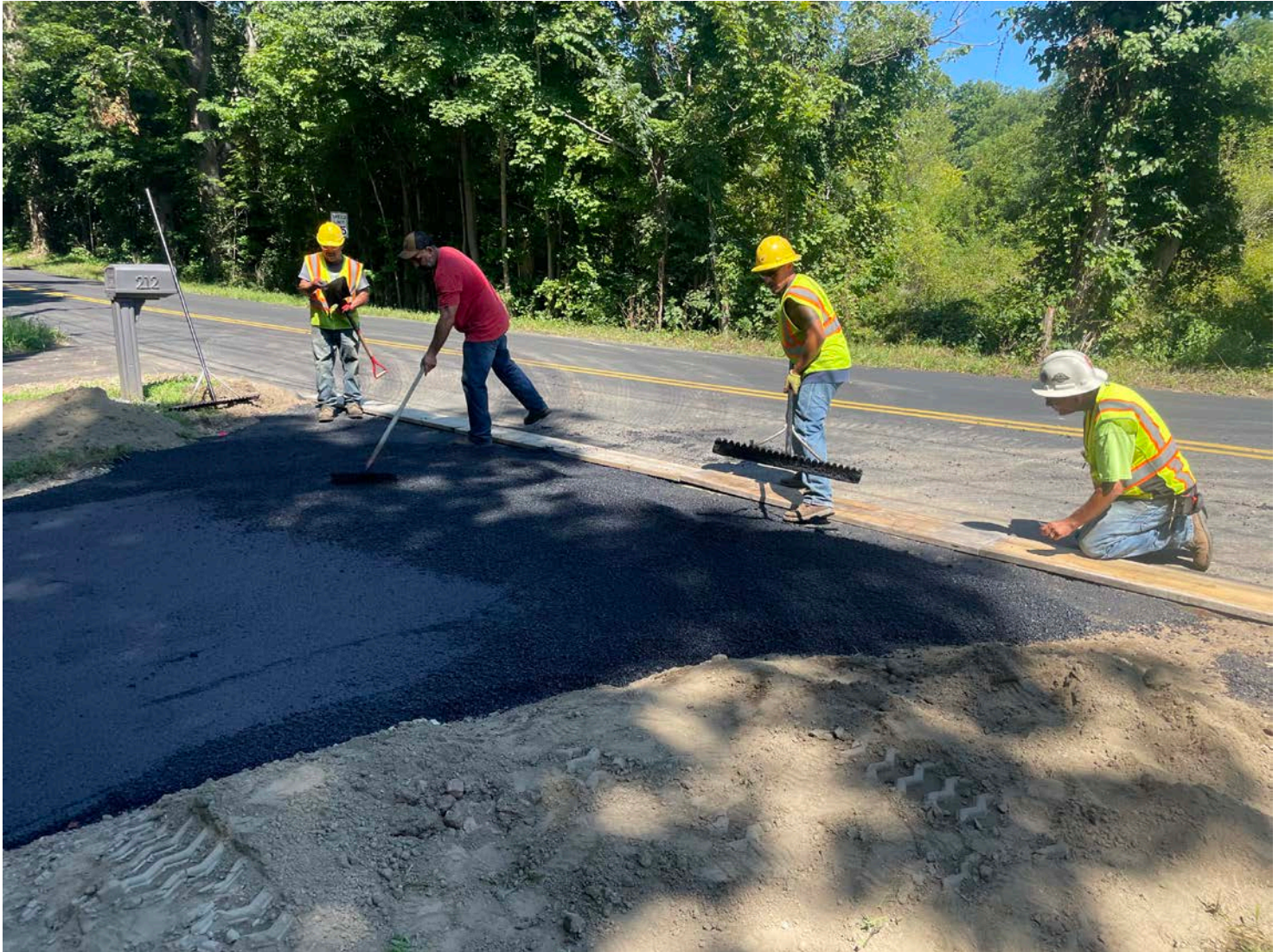
Picture 6: Ludlow placing the second of two lifts of asphalt on the footprint of the 212R Maple Avenue property driveway where it connects with Maple Avenue. View to the northeast.
