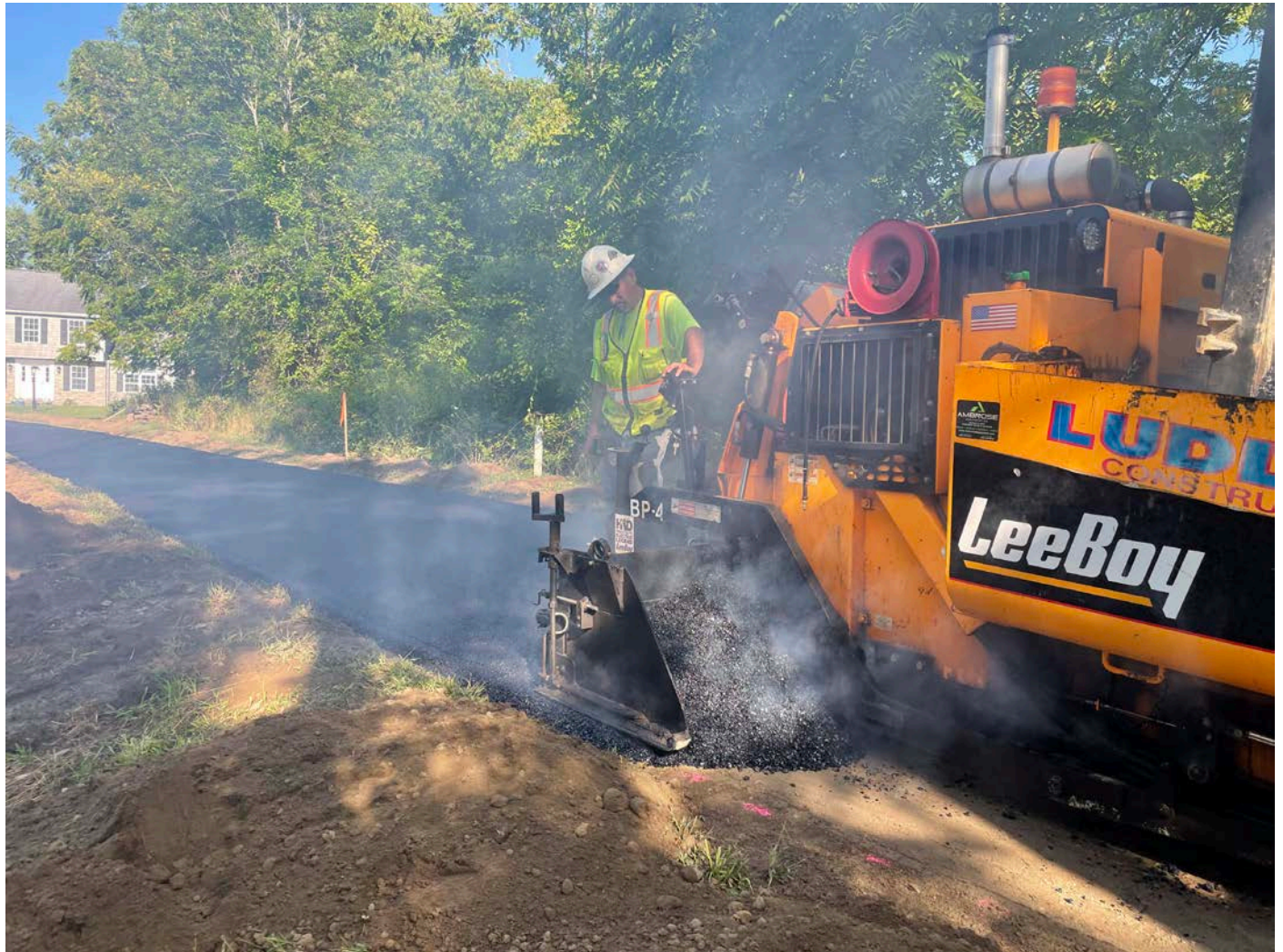
Picture 4: Ludlow placing the first of two lifts of asphalt on the footprint of the 212R Maple Avenue property driveway. View to the west.
