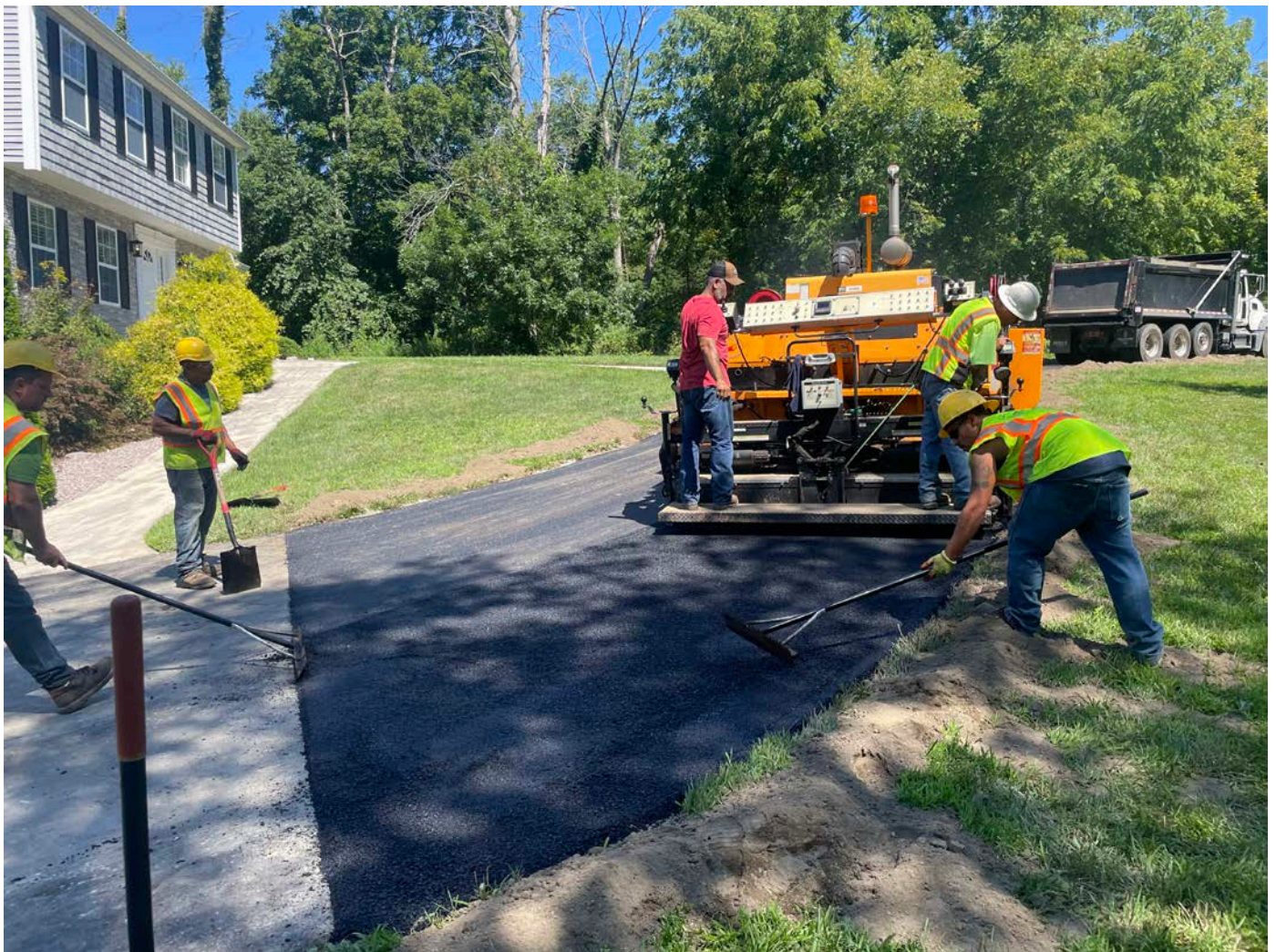
Picture 5: Ludlow placing the second of two lifts of asphalt on the footprint of the 212R Maple Avenue property driveway. View to the north.
