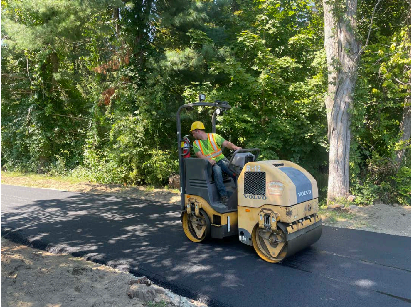
Picture 7: Ludlow using a rolling compactor on the second lift of asphalt they placed on the footprint of the driveway on the 212R Maple Avenue property. View to the northwest.
