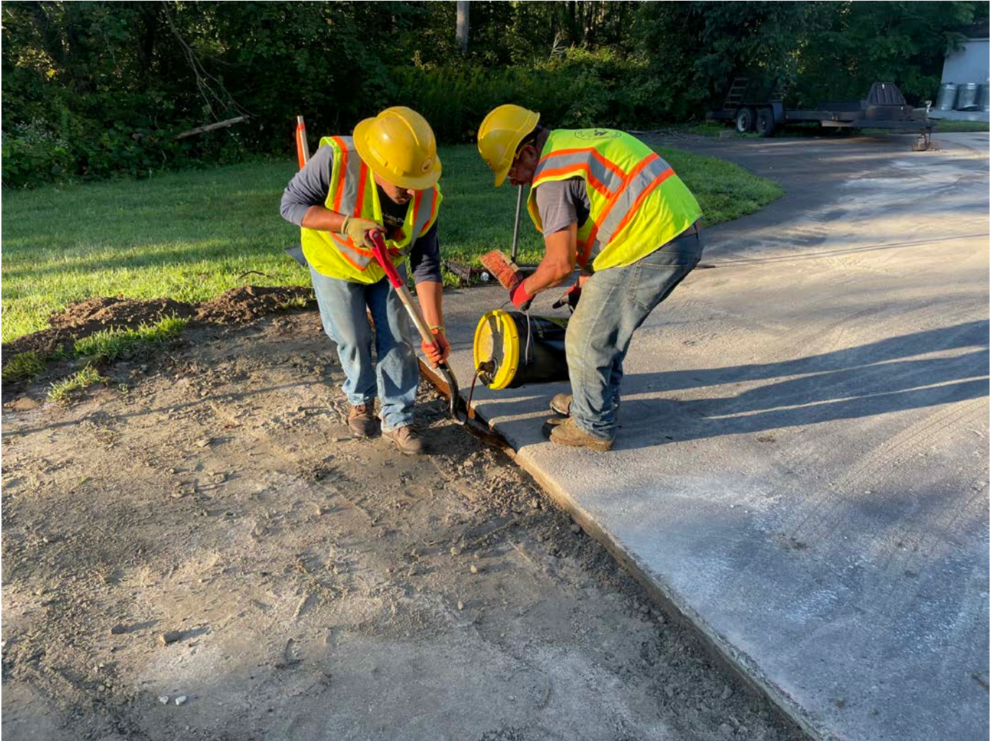
Picture 2: Ludlow applying tack coating to the cut edge of existing pavement on the west side of the driveway footprint of the 212R Maple Avenue property. View to the southwest.
