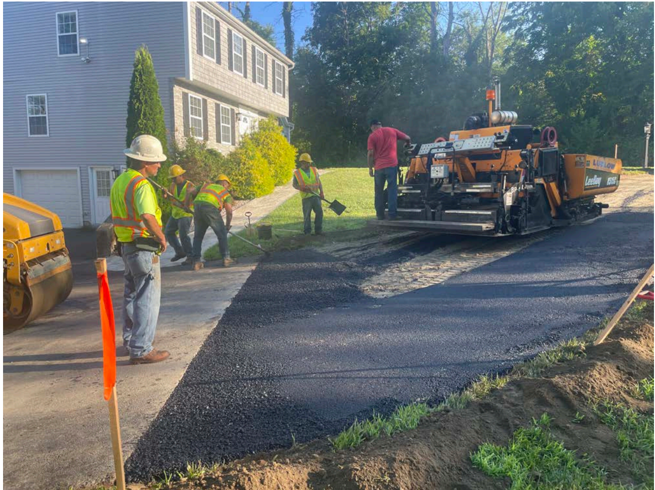
Picture 3: Ludlow placing the first of two lifts of asphalt on the footprint of the 212R Maple Avenue property driveway. View to the north.
