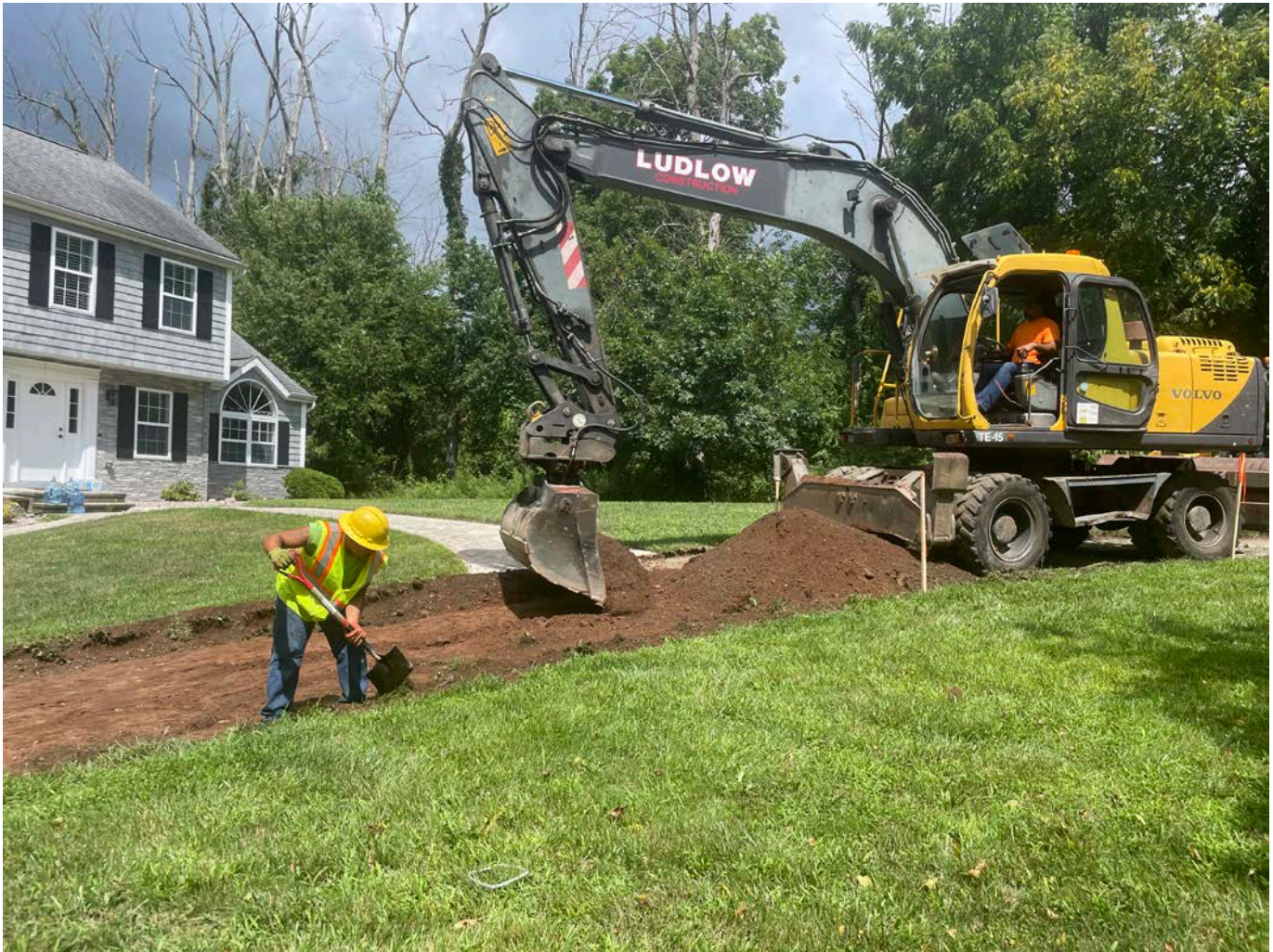
Picture 5: Ludlow excavating and grading the driveway at 212R Maple Avenue.
