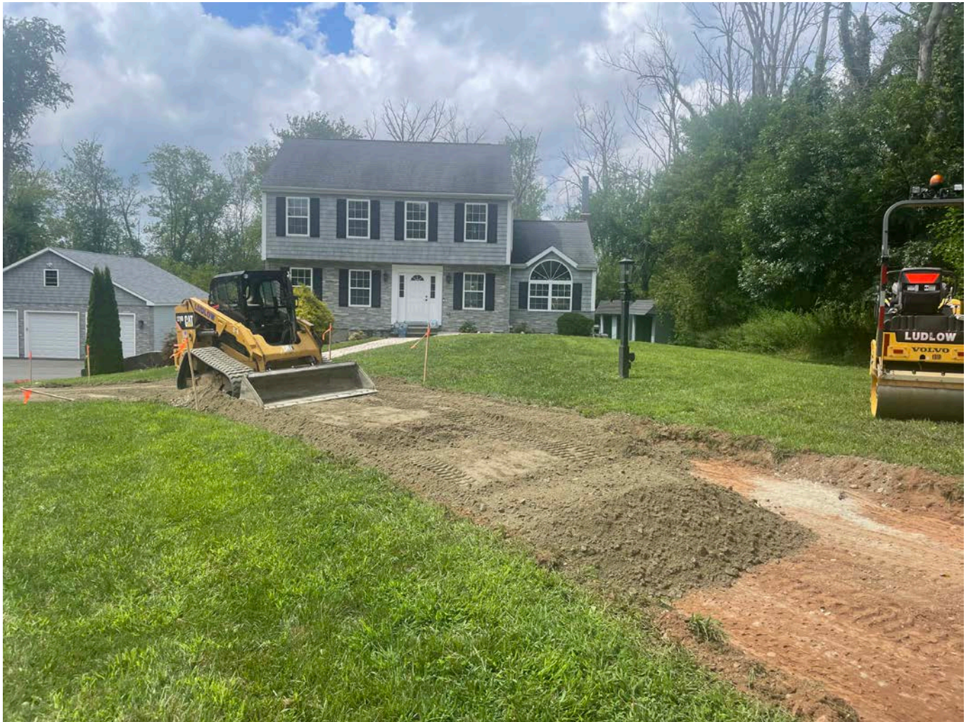
Picture 7: Ludlow placing processed stone in the driveway at 212R Maple Ave. View to the west.
