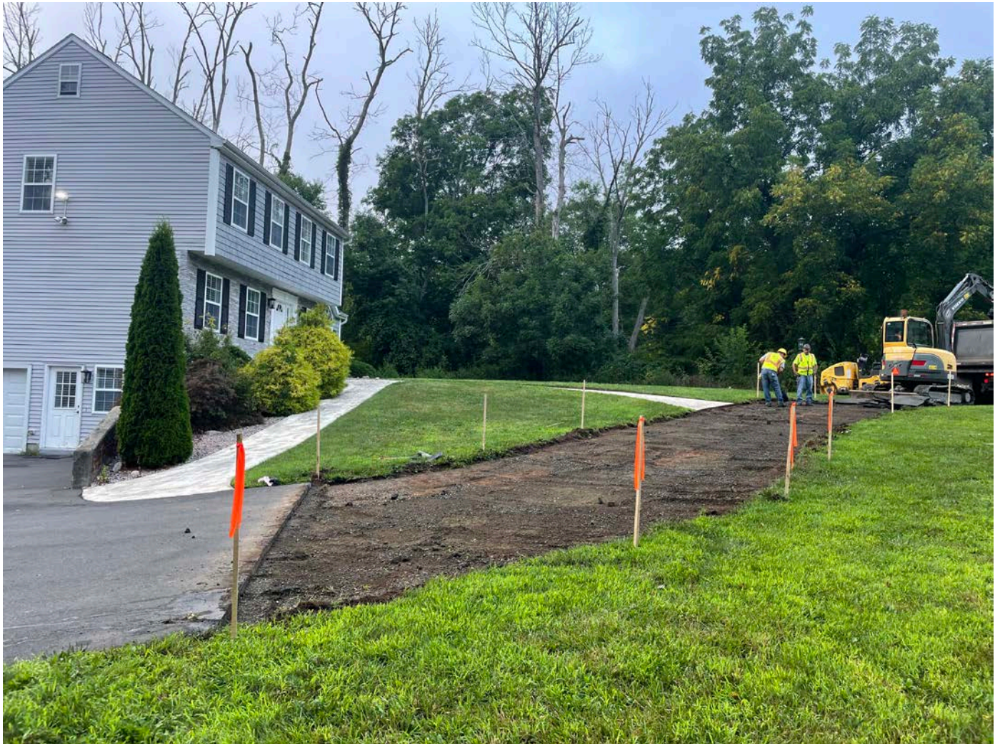
Picture 2: Ludlow staking the edge of the existing driveway and removing the existing asphalt pavement at 212R Maple Ave.
