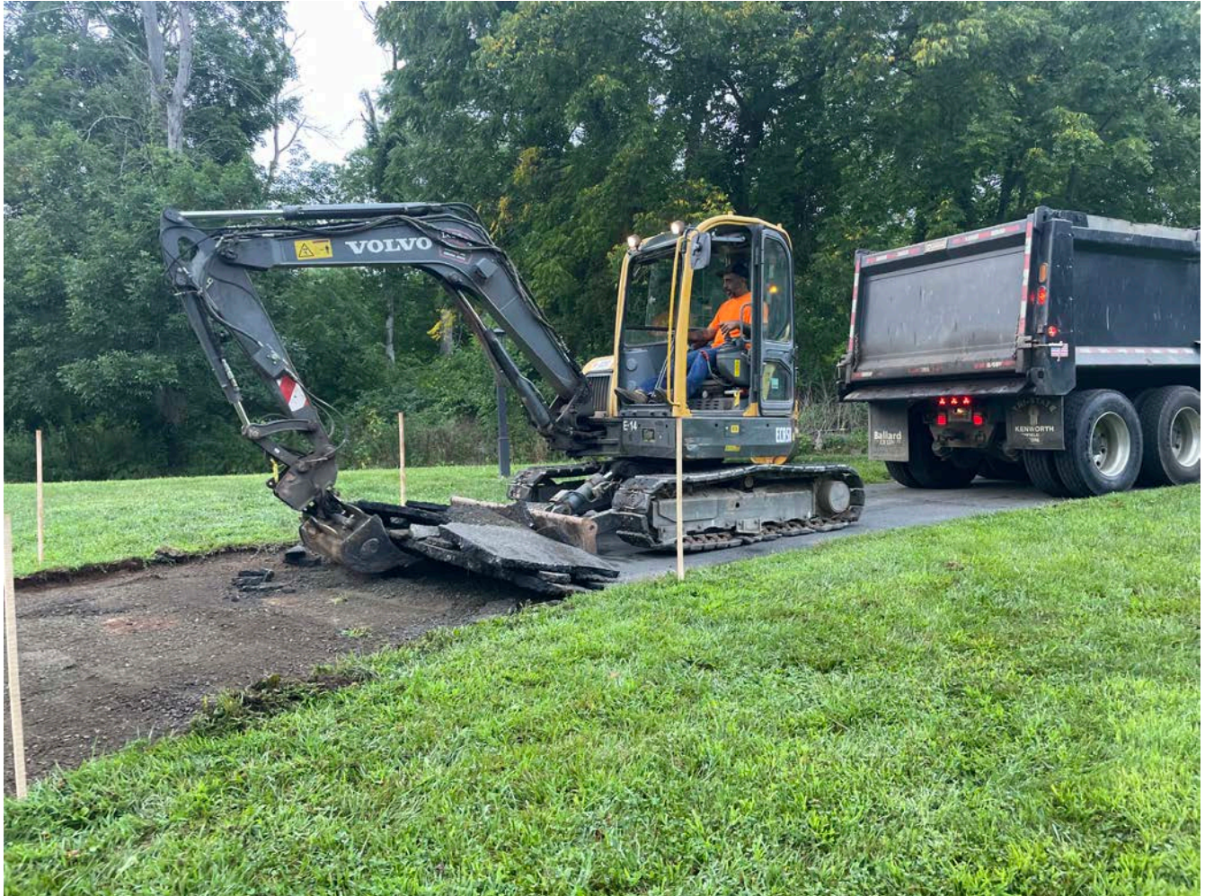
Picture 1: Ludlow removing pavement from the driveway at 212R Maple Ave. residence.
