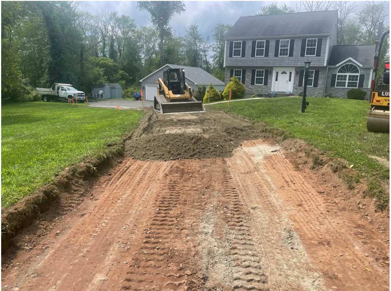
Picture 6: Ludlow placing processed stone in the driveway at 212R Maple Avenue.
