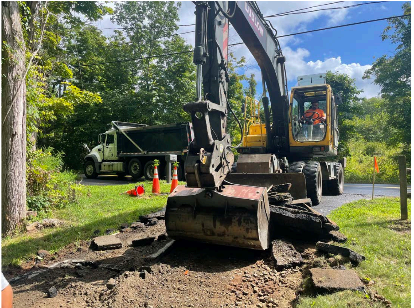
Picture 4: Ludlow removing pavement at the driveway entrance to 212R Maple Avenue. View to the east.
