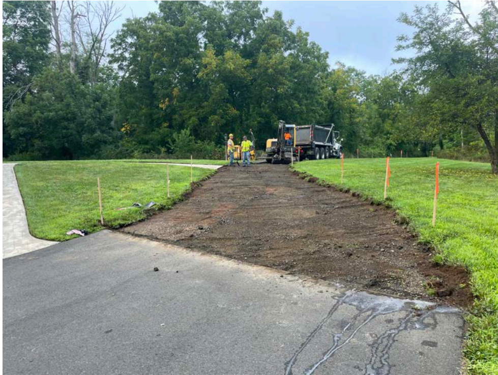
Picture 3: Ludlow removing existing pavement from the driveway at 212R Maple Avenue. View to the east.
