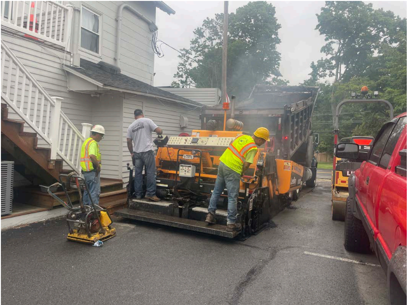
Picture 5: Ludlow placing the first lift of asphalt on the south side of the driveway of the 238 Main Street property. View to the east.
