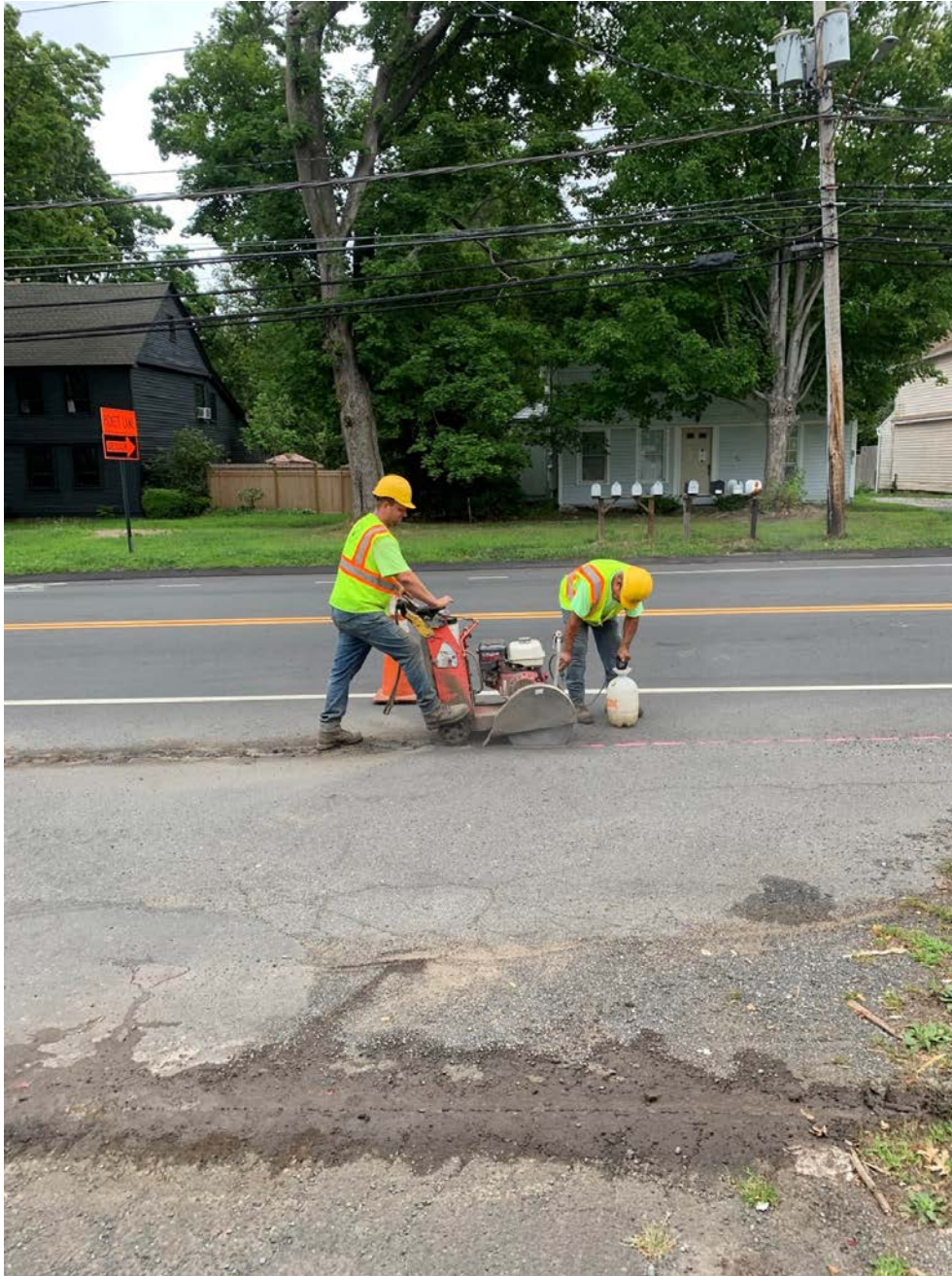
Picture 1: Ludlow saw cutting the pavement apron at 238 Main Street. View to the east.
