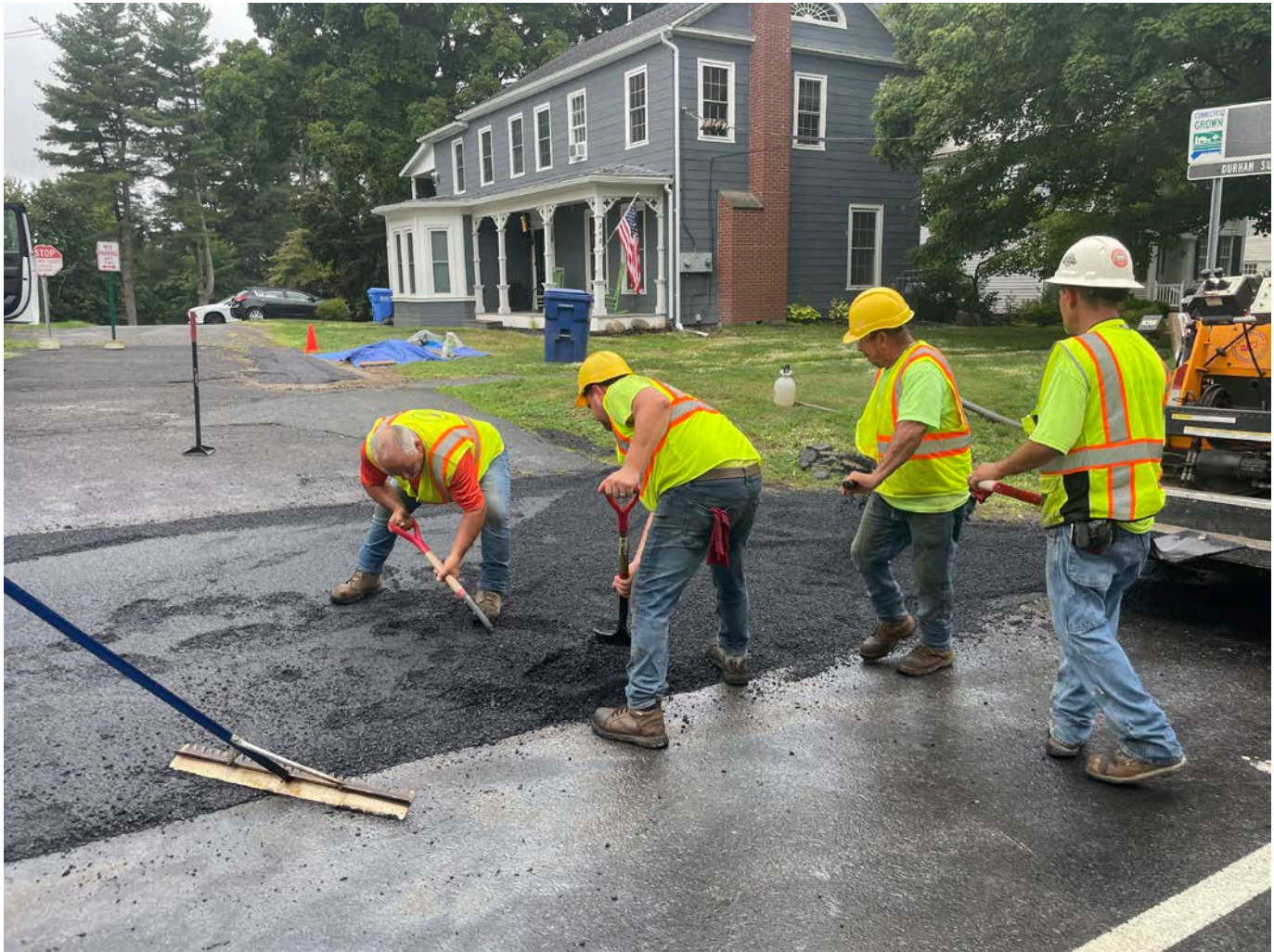
Picture 7: Ludlow grading the second lift of asphalt placed on the driveway footprint at the 238 Main Street property. View to the west.
