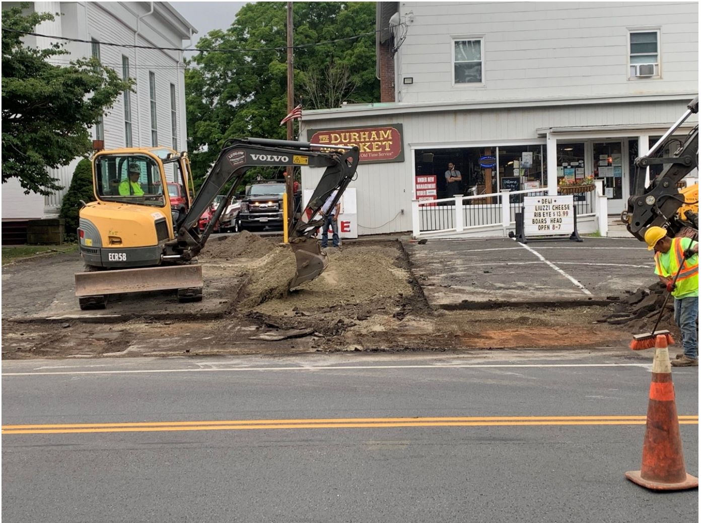
Picture 2: Ludlow removing the existing driveway pavement at the 238 Main Street property. View to the west.
