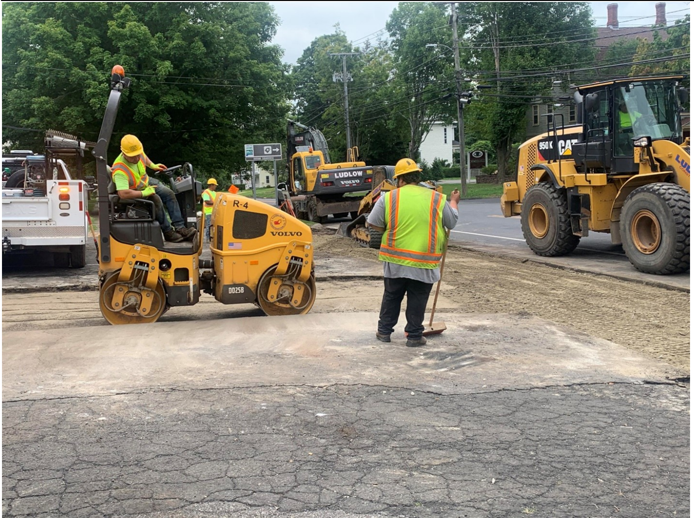
Picture 4: Ludlow compacting the processed stone base at 238 Main Street. View to the northeast.
