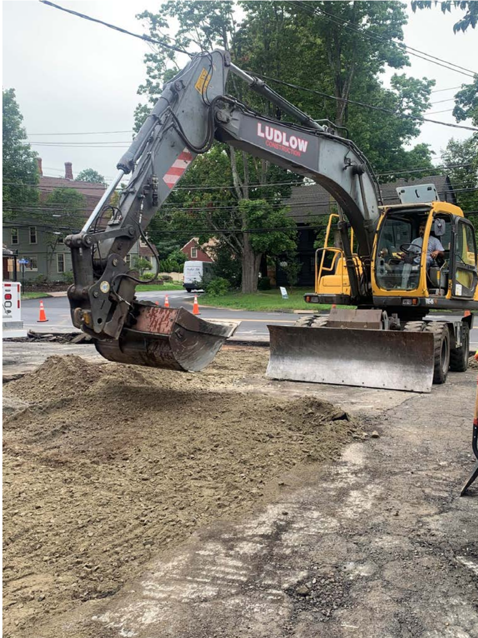
Picture 3: Ludlow grading the processed stone base on the driveway at 238 Main Street. View to the east.
