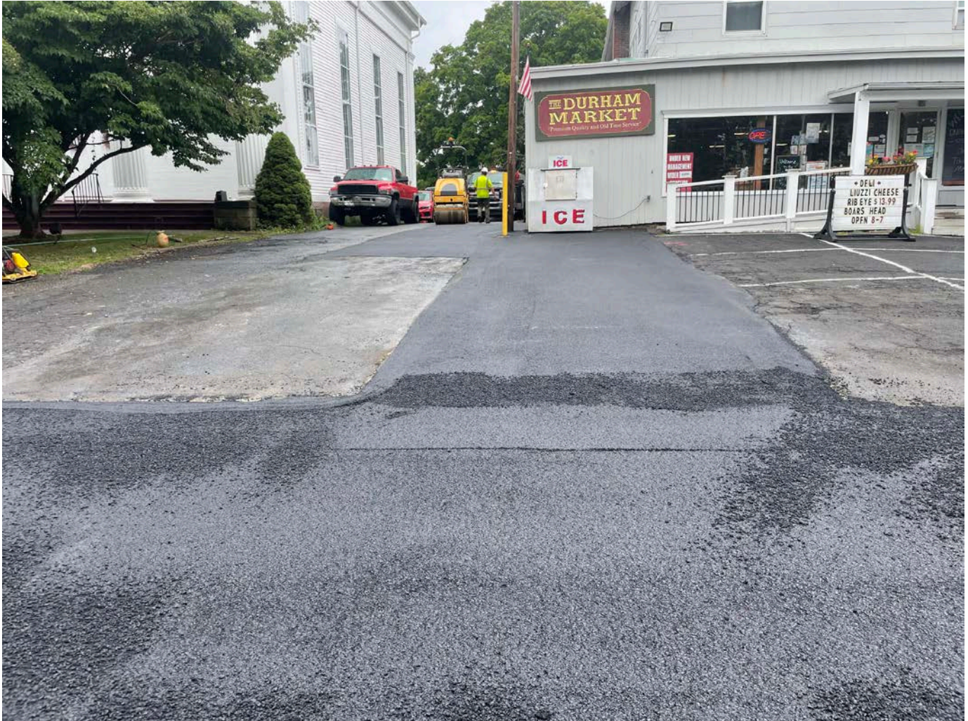
Picture 8: Ludlow compacting the second pavement course of the driveway at the 238 Main Street property. View to the west.
