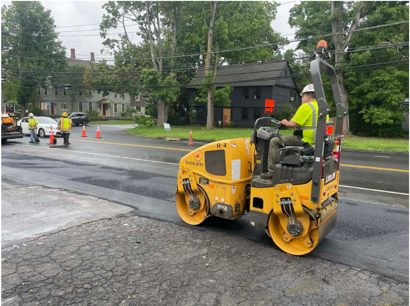
Picture 9: Ludlow rolling the driveway apron pavement at the 238 Main Street property. View to the northeast.
