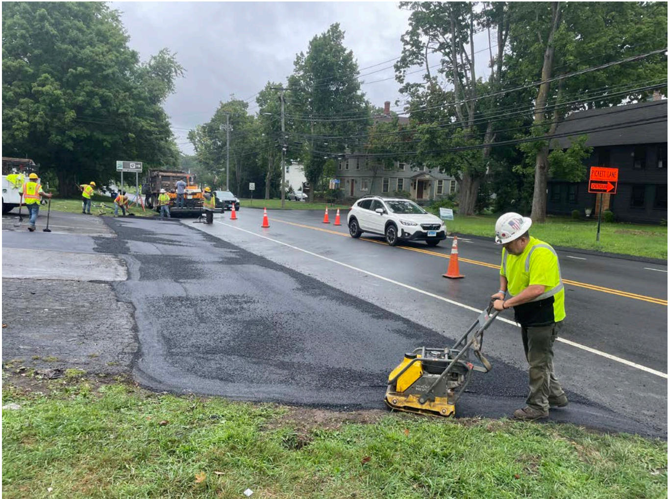
Picture 6: Ludlow compacting the first pavement layer for the driveway apron at 238 Main Street. View to the north.
