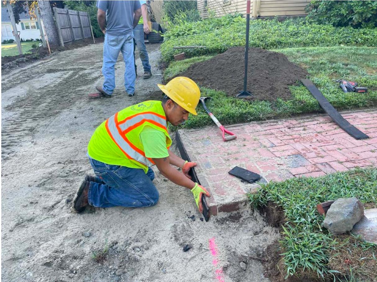
Picture 2: Ludlow placing an expansion joint on the north side of the brick sidewalk on the 257 Main Street property. View to the east.
