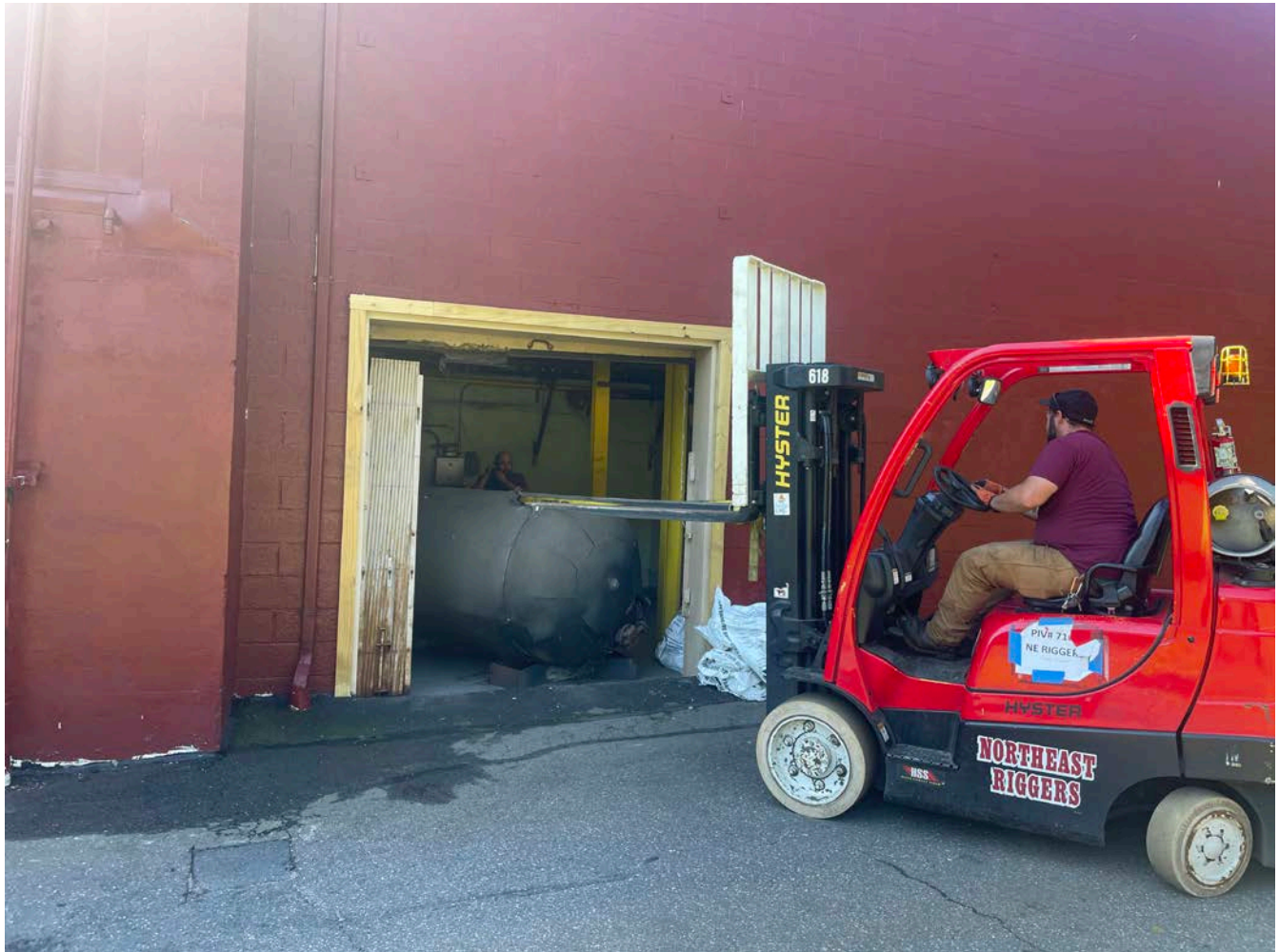
Picture 6: Northeast Rigging removing a water tank from the north side of the Durham Manufacturing facility. View to the south.
