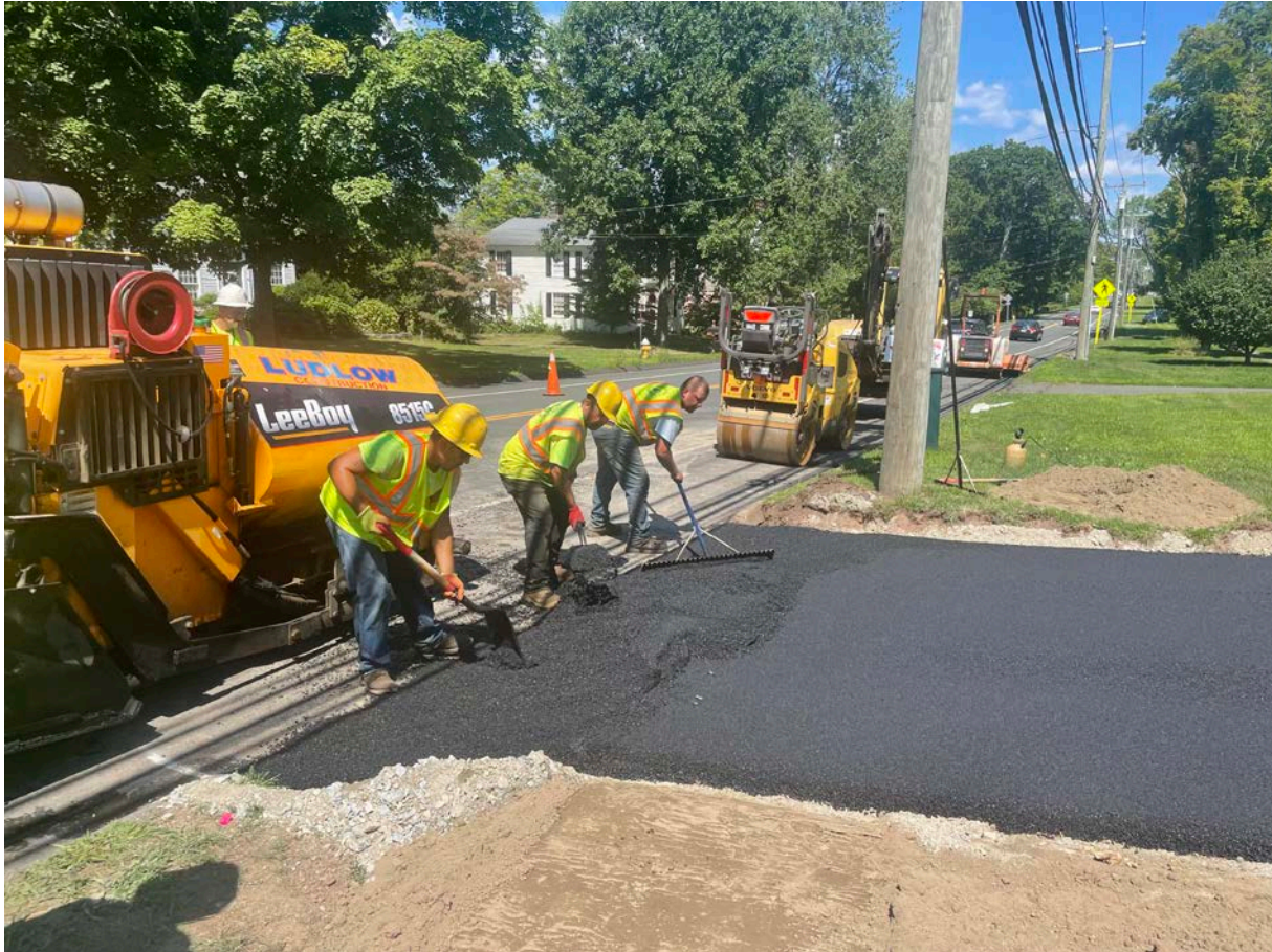
Picture 7: Ludlow grading the second lift of asphalt placed on the driveway footprint at the 257 Main Street property. View to the north.
