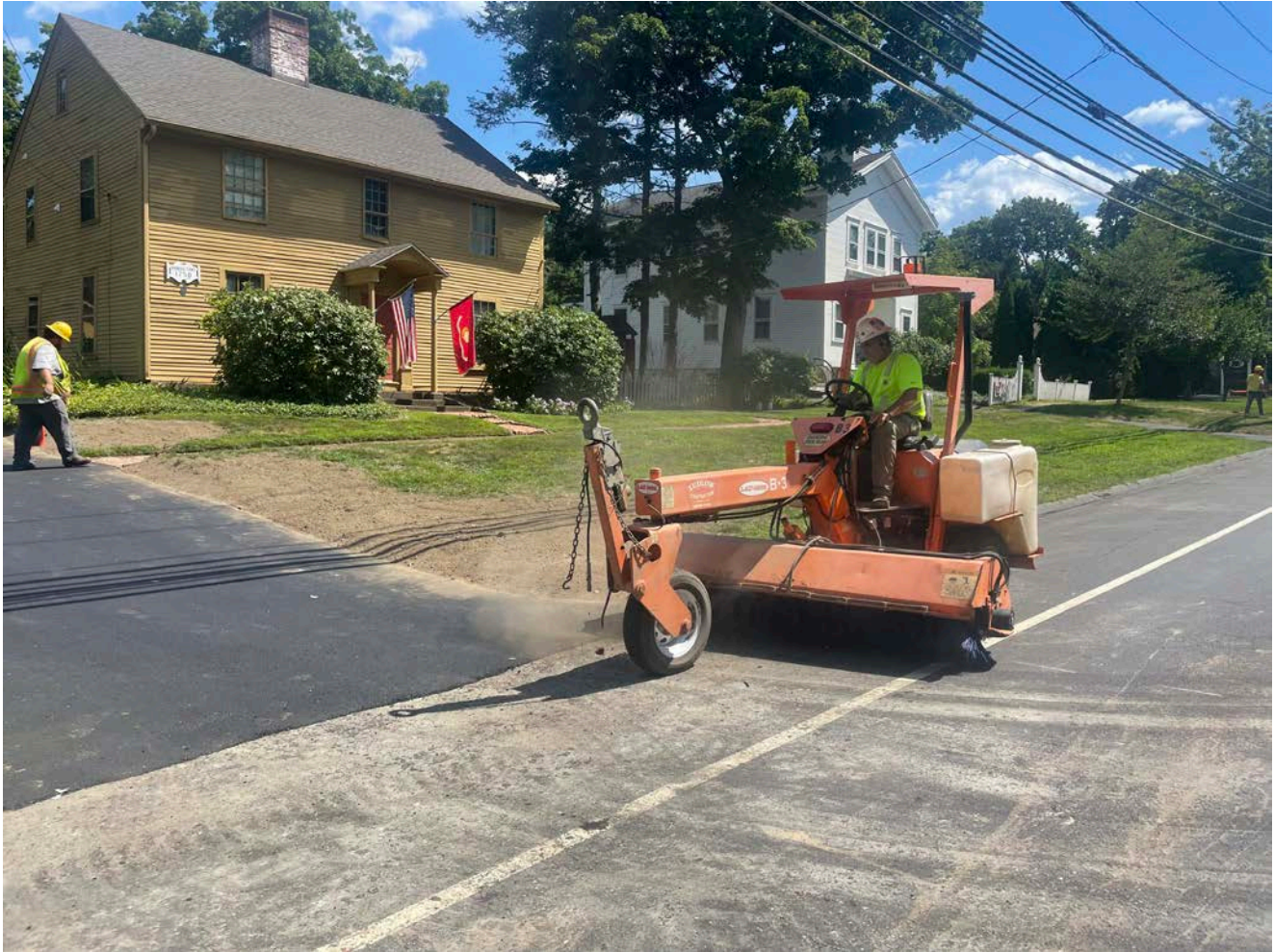
Picture 9: Ludlow using a Broce Broom to clean the street in front of the driveway at the 257 Main Street property. View to the southeast.
