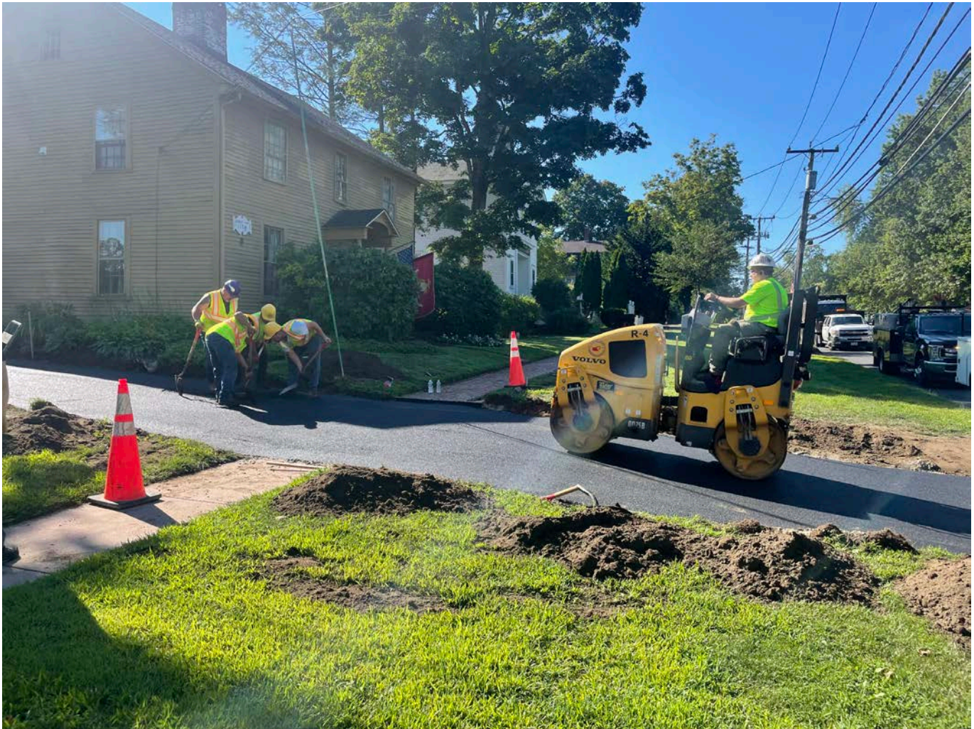
Picture 5: Ludlow compacting the first lift of asphalt on the west side of the driveway of the 257 Main Street property. View to the southeast.
