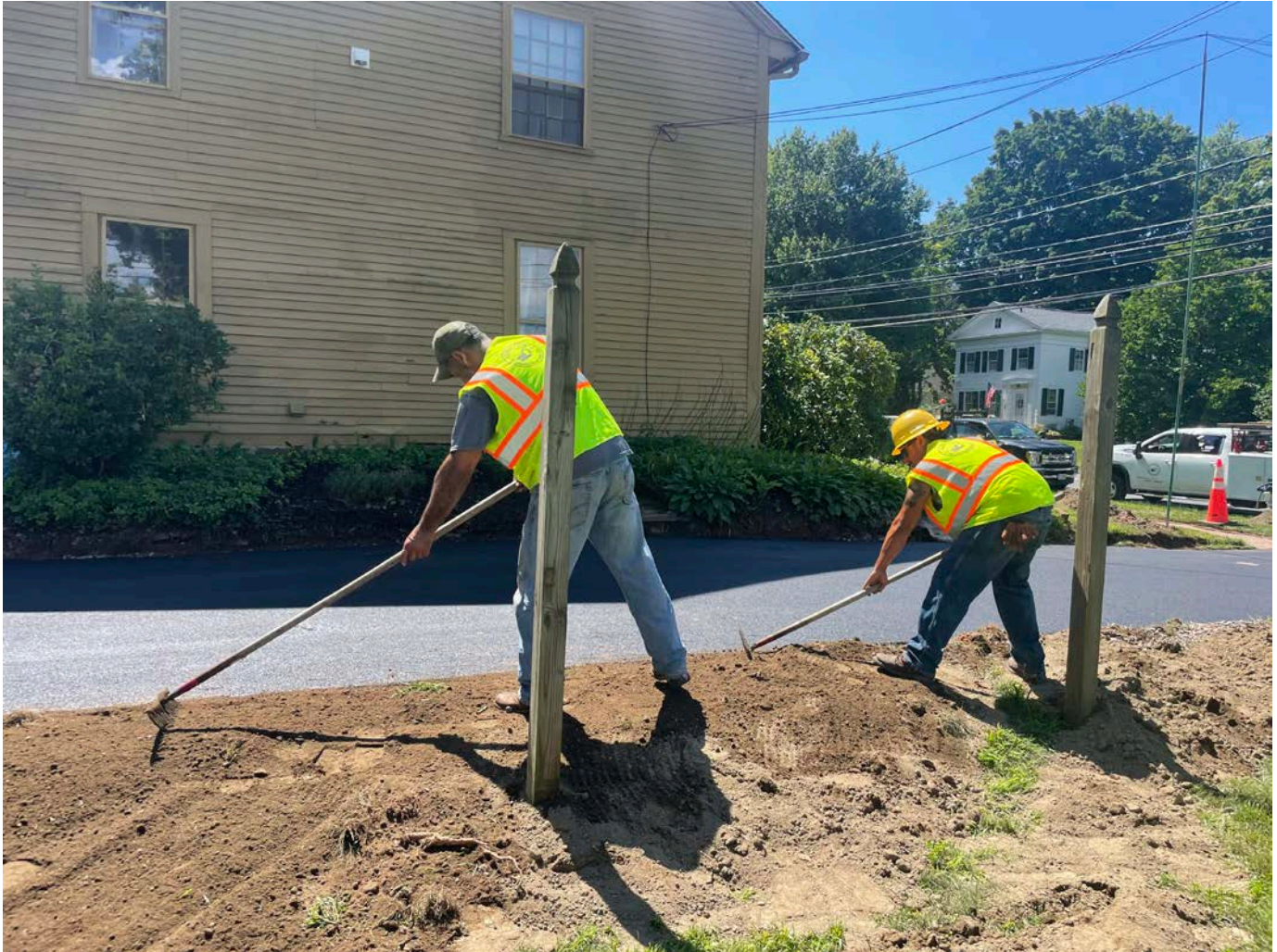
Picture 8: Ludlow grading loam on the north side of the driveway at the 257 Main Street property. View to the southwest.
