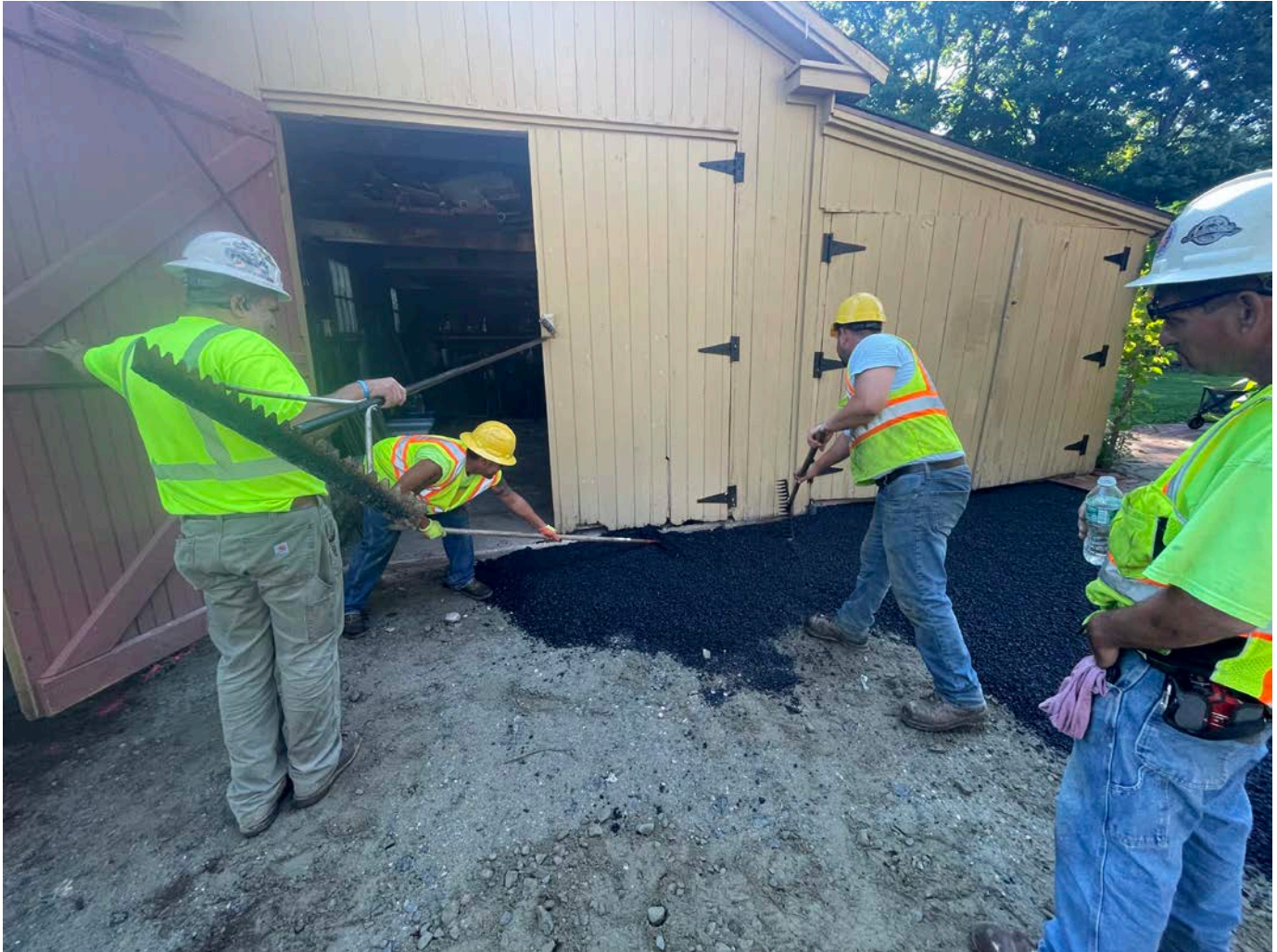
Picture 3: Ludlow placing the first lift of asphalt on the east side of the driveway of the 257 Main Street property. View to the east.
