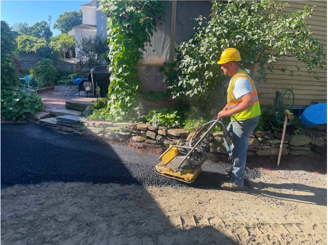
Picture 4: Ludlow compacting the first lift of asphalt on the east side of the driveway of the 257 Main Street property. View to the southeast.
