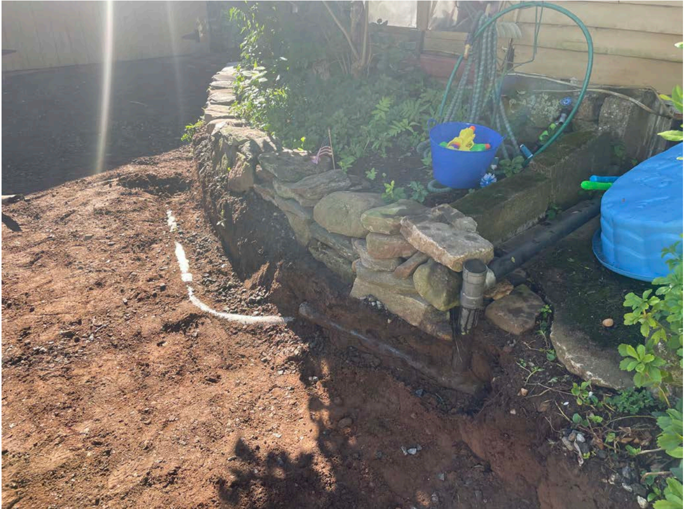
Picture 6: 2" PVC that Ludlow daylighted when preparing the subgrade of the driveway footprint at the 257 Main Street property for paving tomorrow. View to the southeast.
