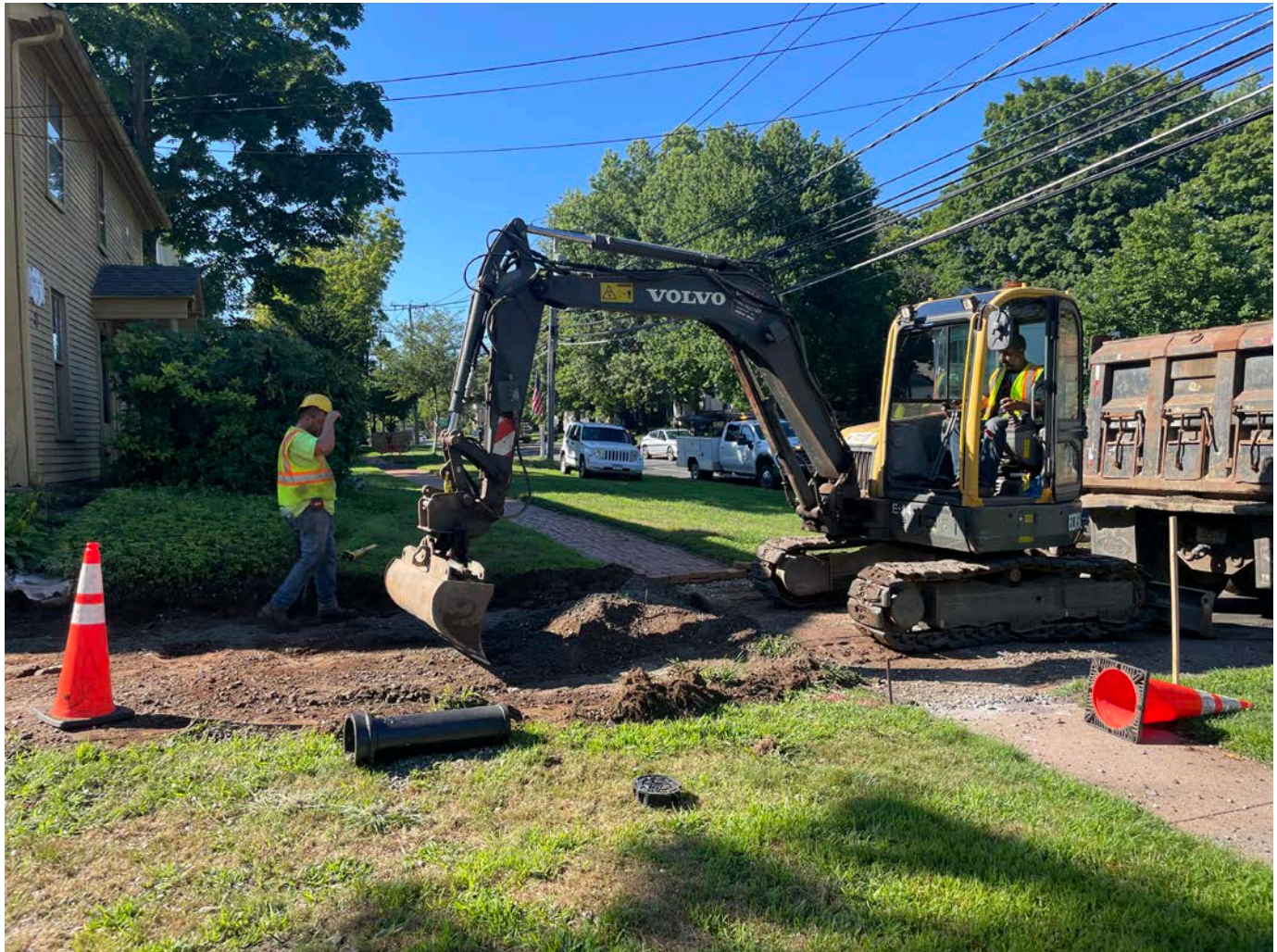
Picture 8: Ludlow placing and grading 1.25" processed gravel on the west side of the driveway at the 257 Main Street property as they prepare for paving tomorrow. View to the south.
