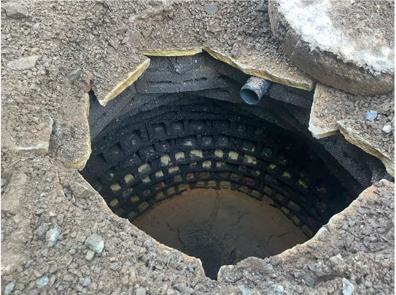
Picture 3: The interior of the dry well that Ludlow daylighted on the west side of the garage at the 257 Main Street property. View to the south.
