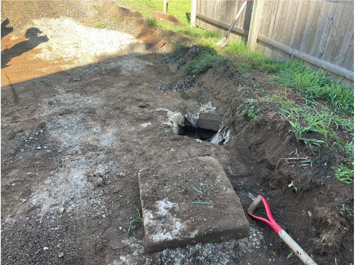
Picture 5: A second dry well that Ludlow daylighted when preparing the subgrade of the driveway footprint at the 257 Main Street property for paving tomorrow. View to the west.
