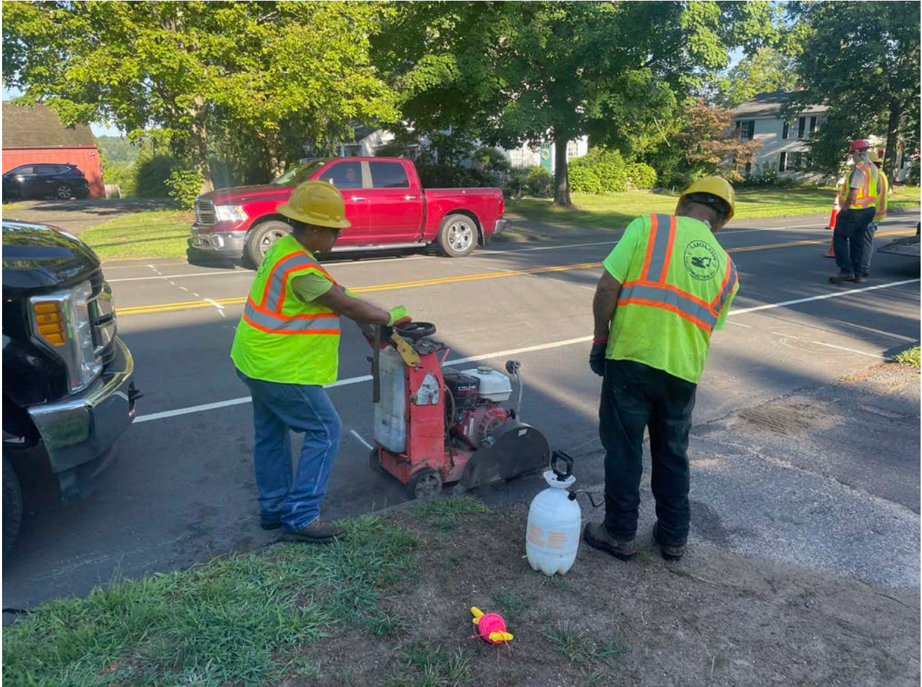
Picture 1: Ludlow saw cutting the edge of pavement where the driveway for the 257 Main Street residence meets Main Street in Durham. View to the northwest.
