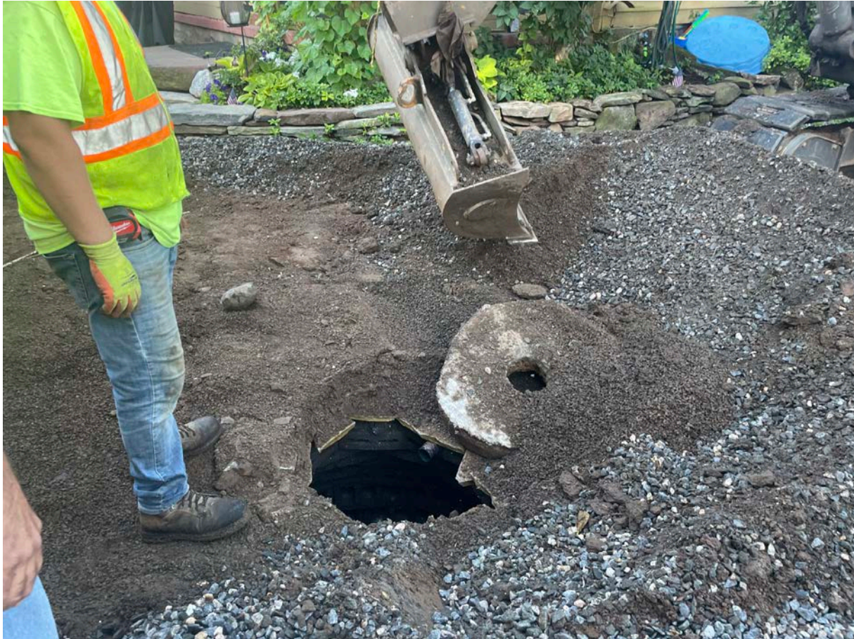
Picture 2: Ludlow uncovering a dry well located on the west side of the garage at the 257 Main Street property. View to the southeast.
