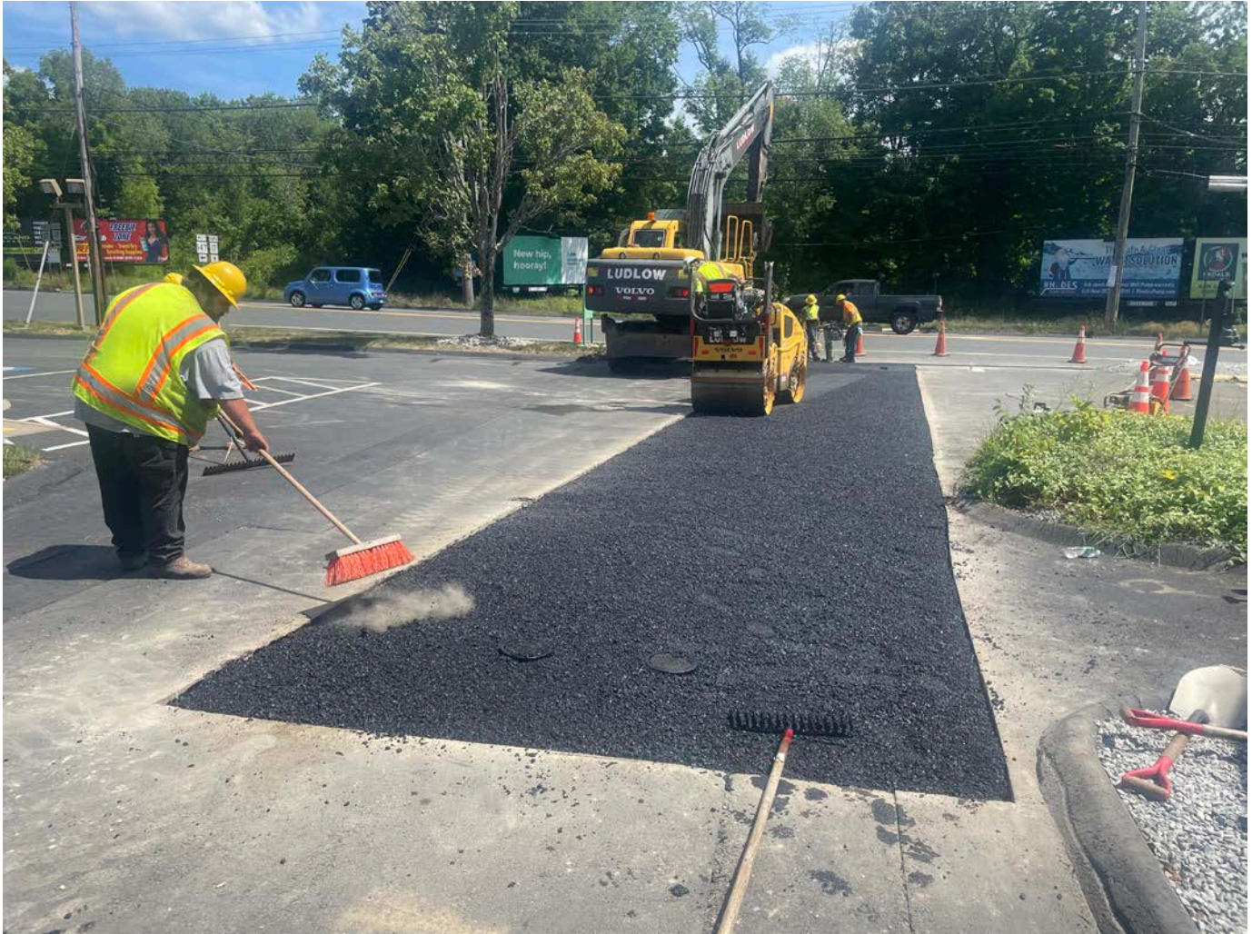
Picture 7: Ludlow compacting the first lift of asphalt that they placed within the footprint of the trench overcut and the shared driveway apron for the 370 and 376 Main Street, Durham, properties. View to the east.
