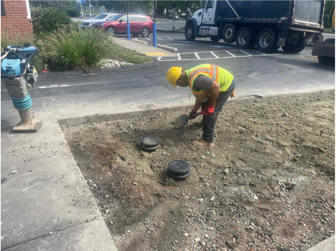
Picture 5: Ludlow backfilling around two road boxes they just installed over the curb stops for the 370 and 376 Main Street, Durham, properties. View to the northeast.
