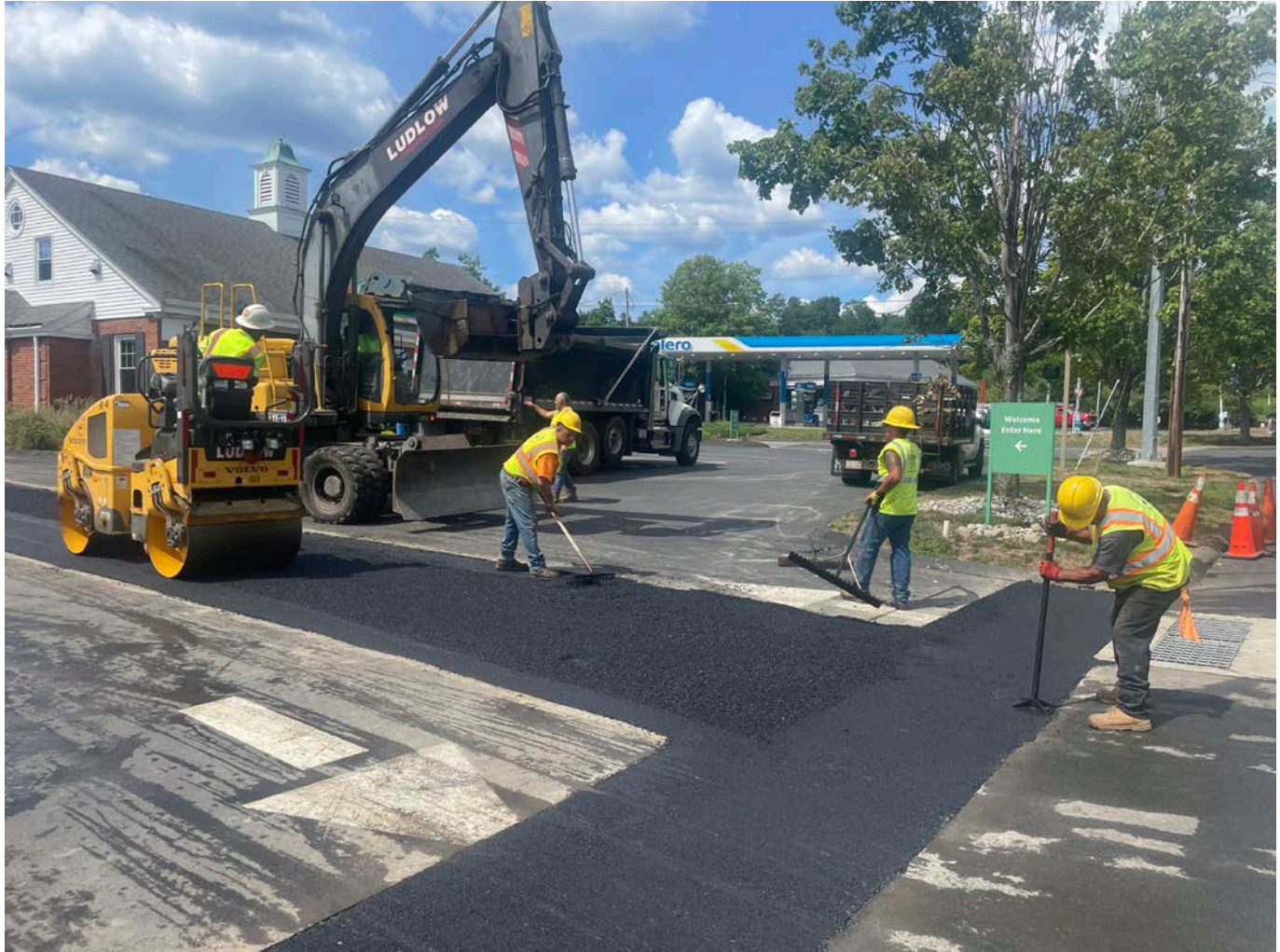
Picture 9: Ludlow grading and compacting the second lift of asphalt that they placed within the footprint of the trench overcut and the shared driveway apron for the 370 and 376 Main Street, Durham, properties with a jumping jack. View to the north.
