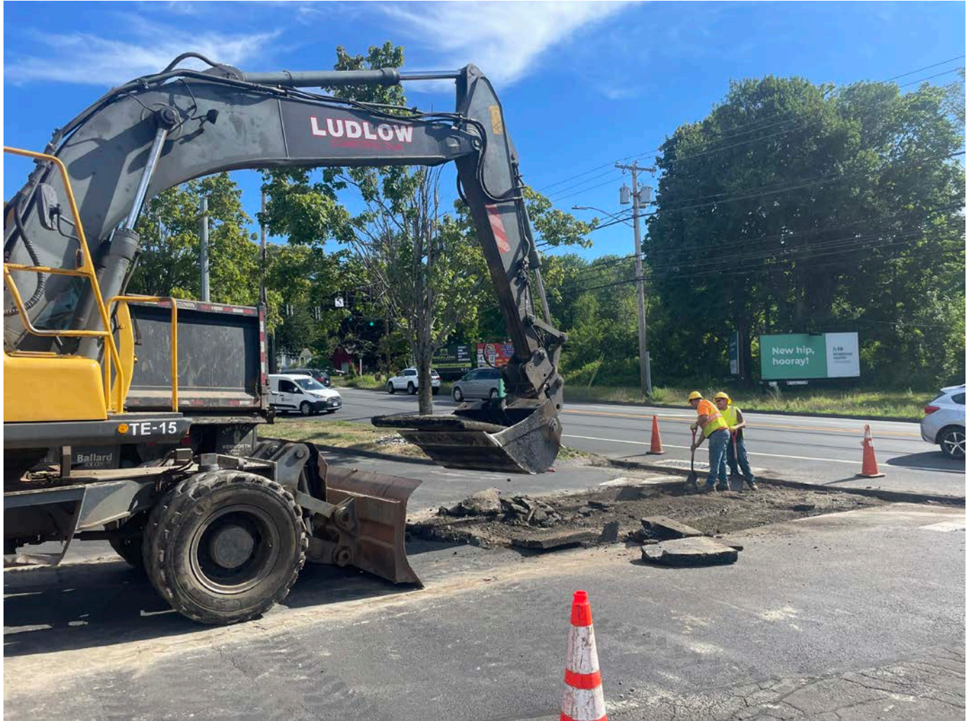
Picture 3: Ludlow removing old asphalt from within the footprint of the trench overcut and the shared driveway apron located between the 370 and 376 Main Street, Durham, properties. View to the northeast.
