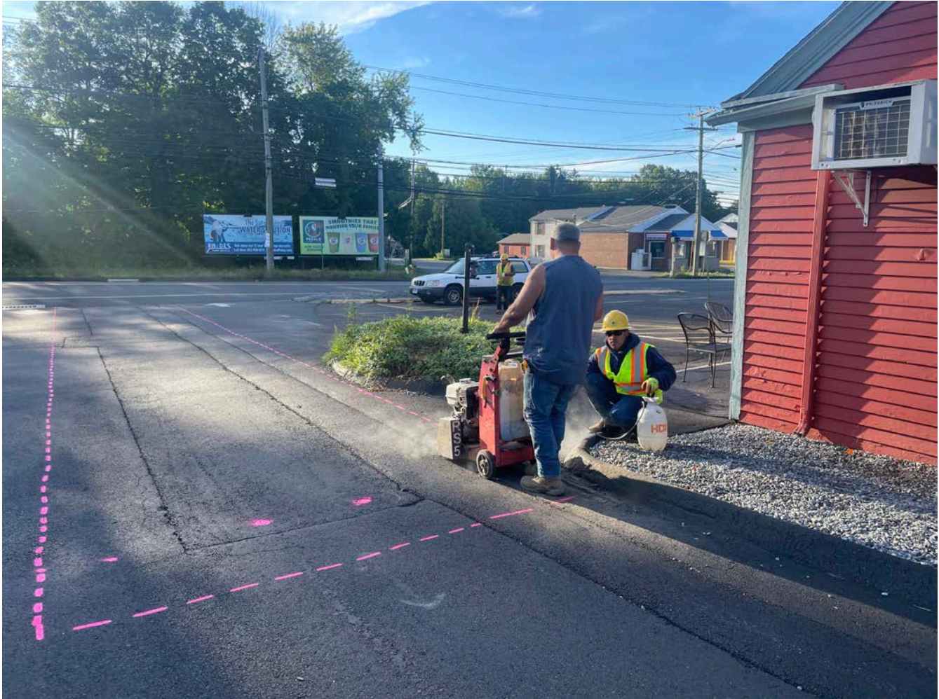
Picture 1: Ludlow saw cutting the footprint of a trench overcut located between 370 and 376 MainStreet in Durham. View to the east.
