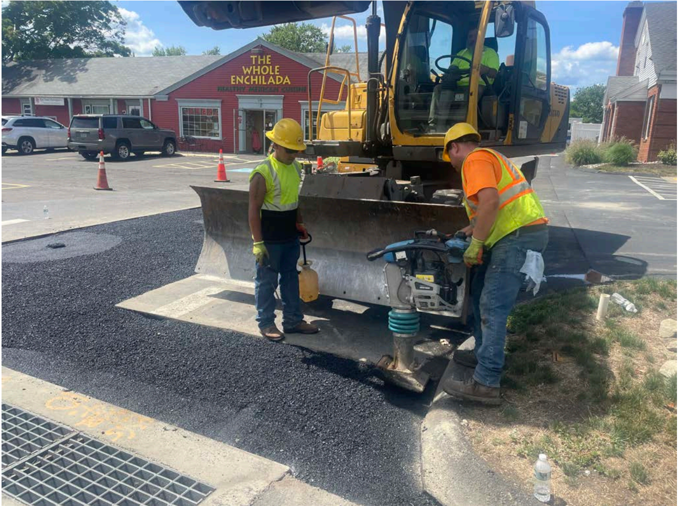
Picture 8: Ludlow compacting the first lift of asphalt that they placed within the footprint of the trench overcut and the shared driveway apron for the 370 and 376 Main Street, Durham, properties with a jumping jack. View to the west.
