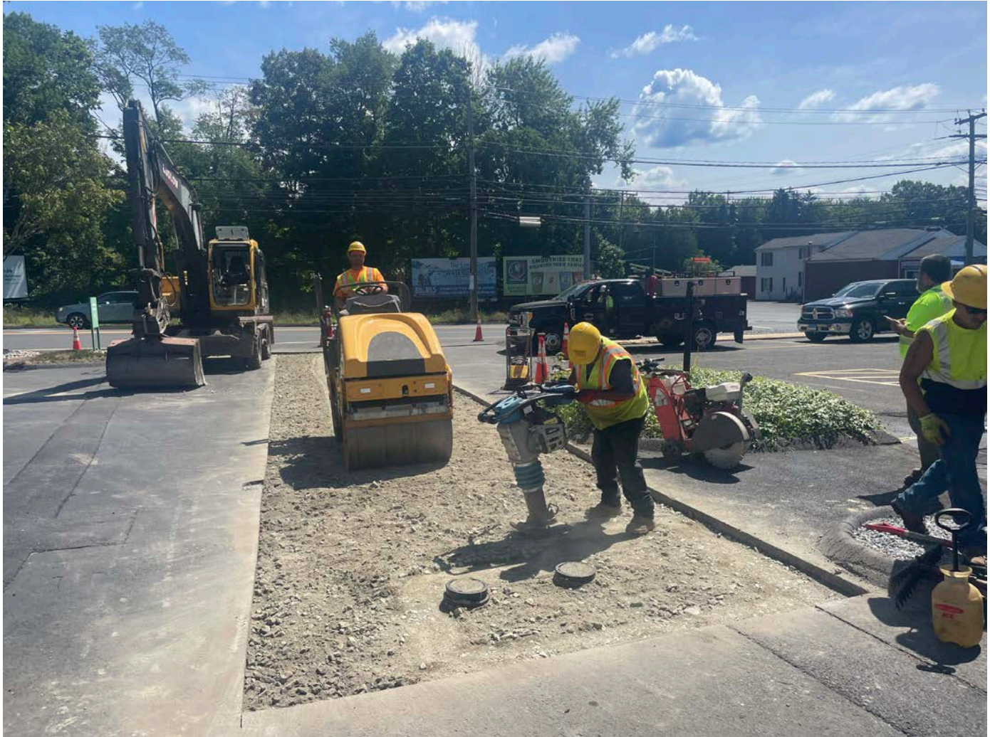
Picture 6: Ludlow compacting 1.25" processed gravel that they placed within the footprint of the trench overcut and the shared driveway apron for the 370 and 376 Main Street, Durham, properties. View to the east.
