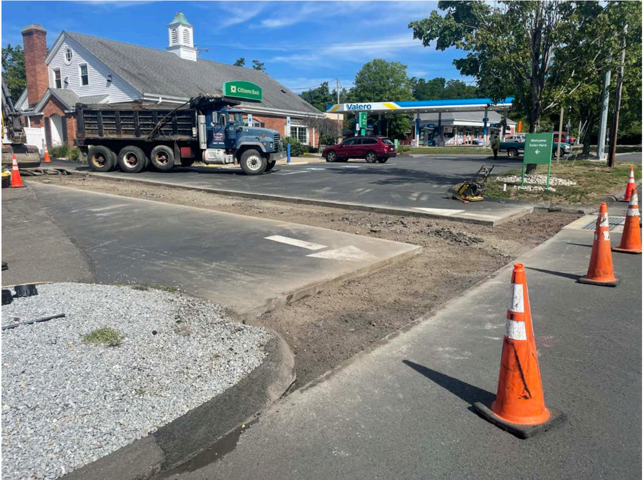
Picture 4: The footprint of the trench overcut and the shared driveway apron located between the 370 and 376 Main Street, Durham, properties after Ludlow removed the old asphalt from within the footprints. View to the northwest.
