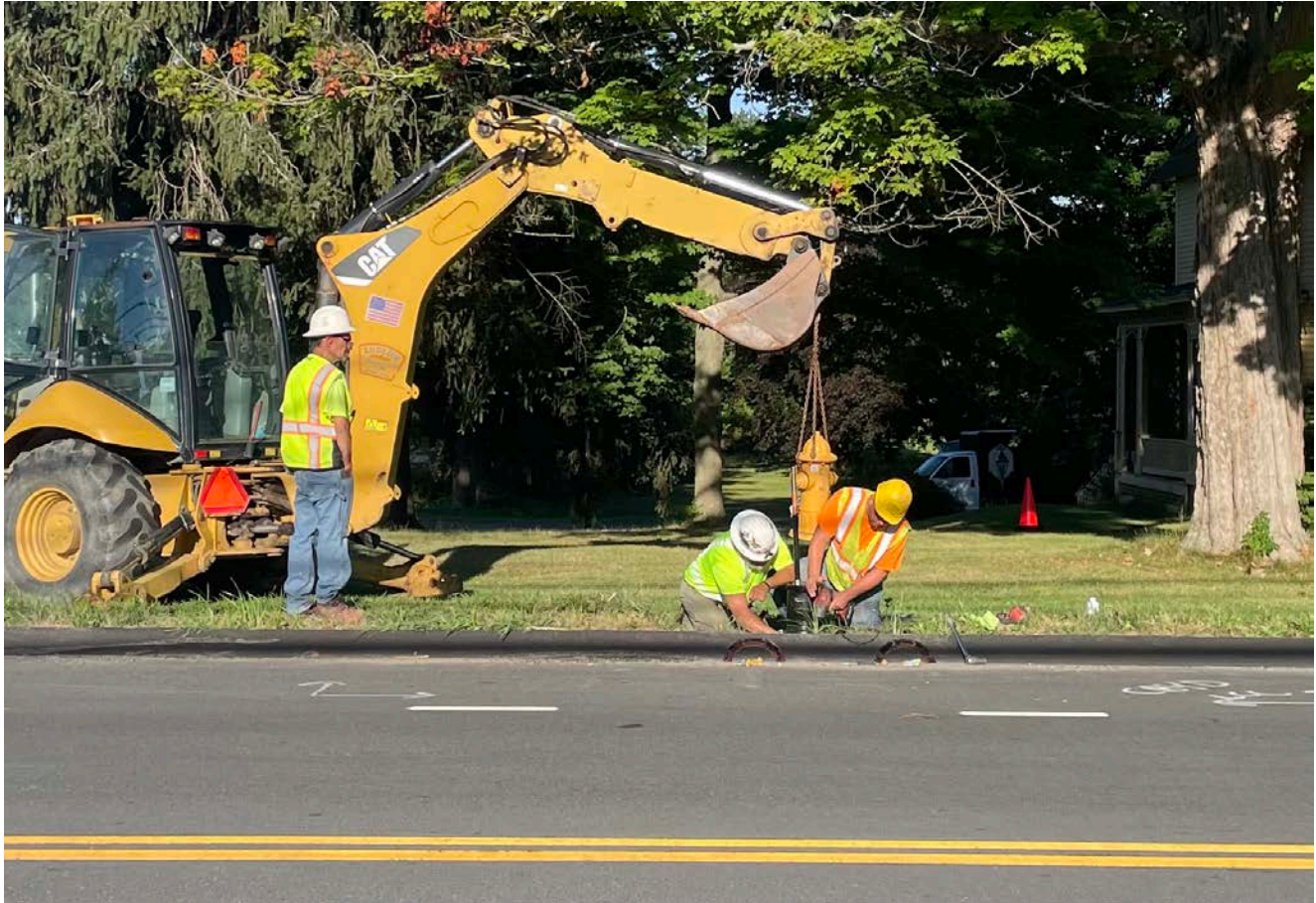
Picture 2: Ludlow installing a 1' extension on a hydrant located in front of 328 Main Street, Durham. View to the east.
