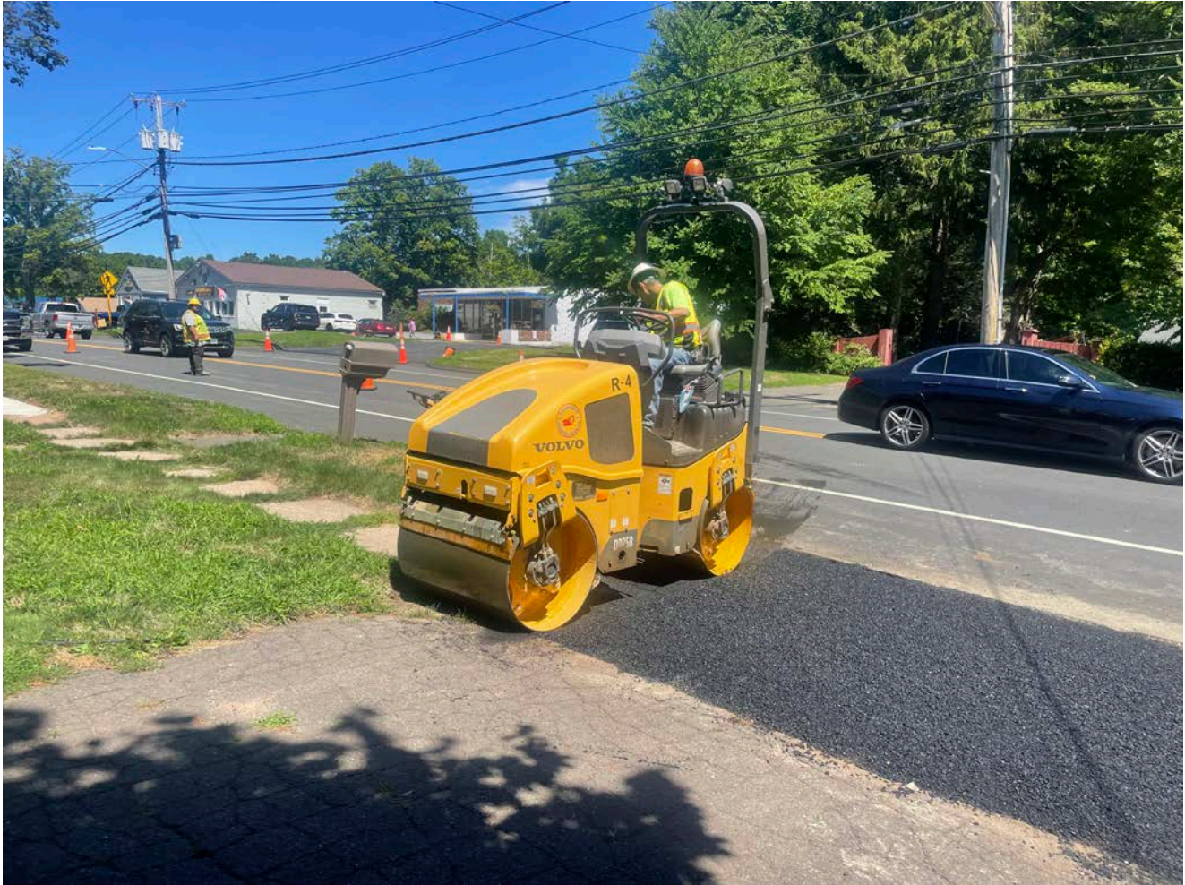
Picture 8: Ludlow using a rolling compactor on the first lift of asphalt that they placed within the footprint of the shared driveway apron for the 312 and 316 Main Street, Durham, properties. View to the northeast.
