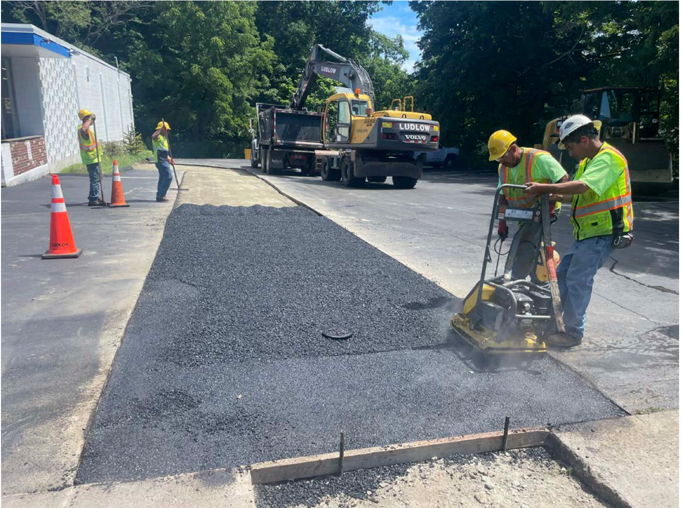
Picture 6: Ludlow compacting edges of the first lift of asphalt that they placed within the footprint of the trench overcut at the 321 Main Street, Durham, property. View to the east.
