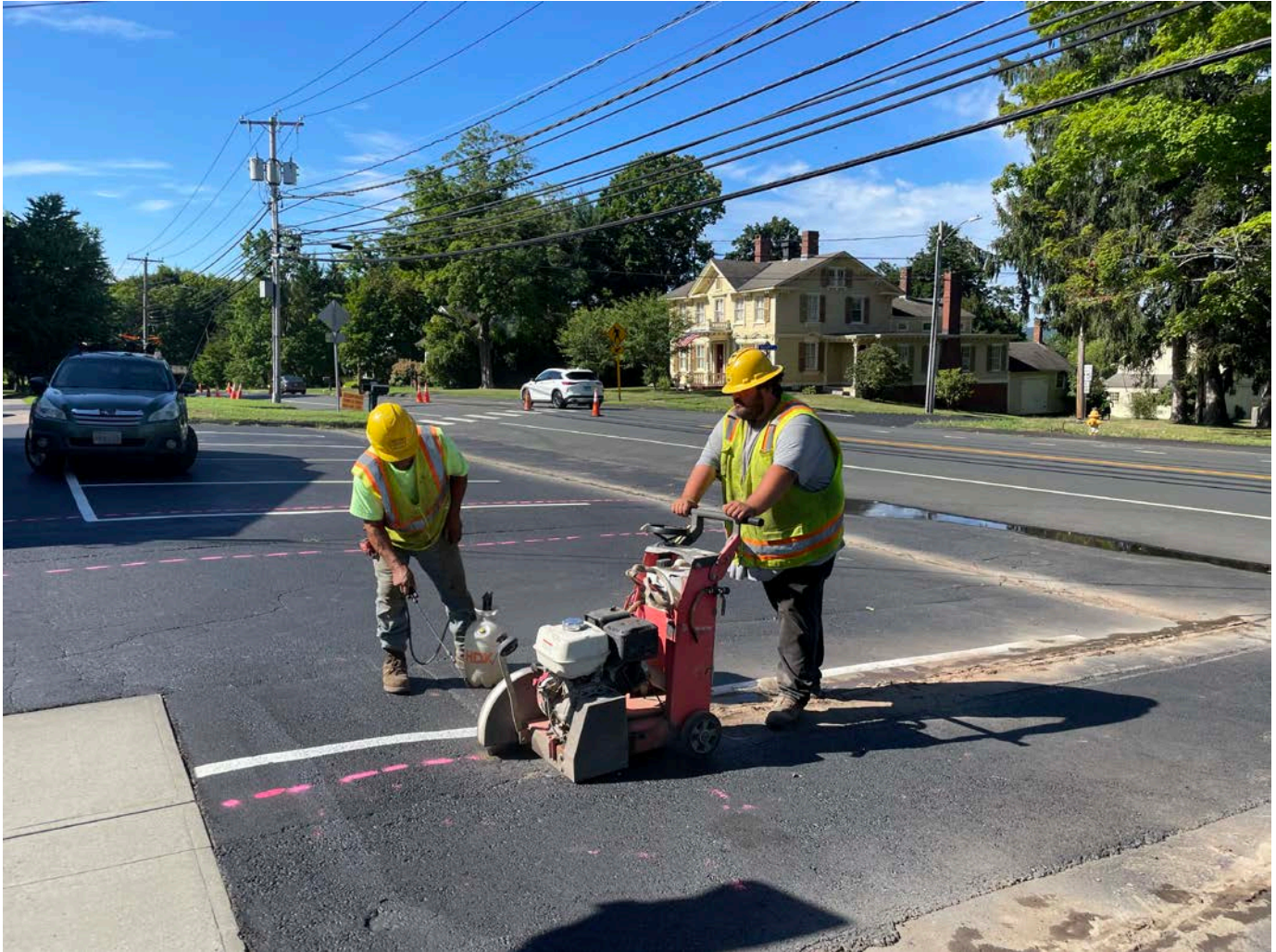
Picture 3: Ludlow saw-cutting the footprint of a trench overcut in order to place permanent pavement on the parking area of the 327 Main Street, Durham, property. View to the southwest.
