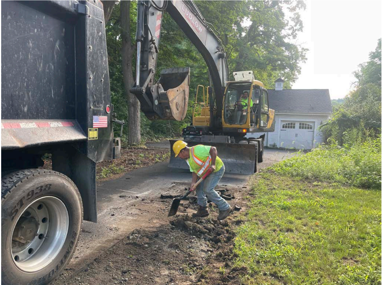
Picture 2: Ludlow excavating temporary paving on the south edge of the driveway of the 313 Main Street, Durham, property as they prepare to place permanent paving. View to the east.
