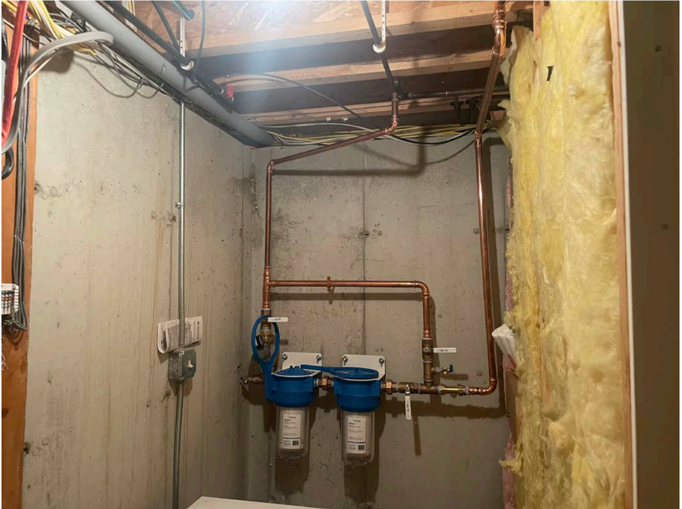
Picture 5: Final water service components that Fazzino installed at the 228R Maple Avenue, Durham, residence.
