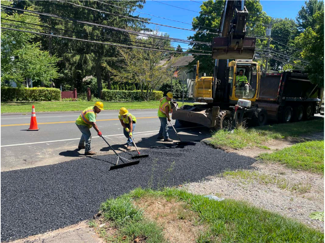
Picture 9: Ludlow grading the first lift of asphalt they placed within the footprint of the shared driveway apron for the 312 and 316 Main Street, Durham, properties. View to the northeast.
