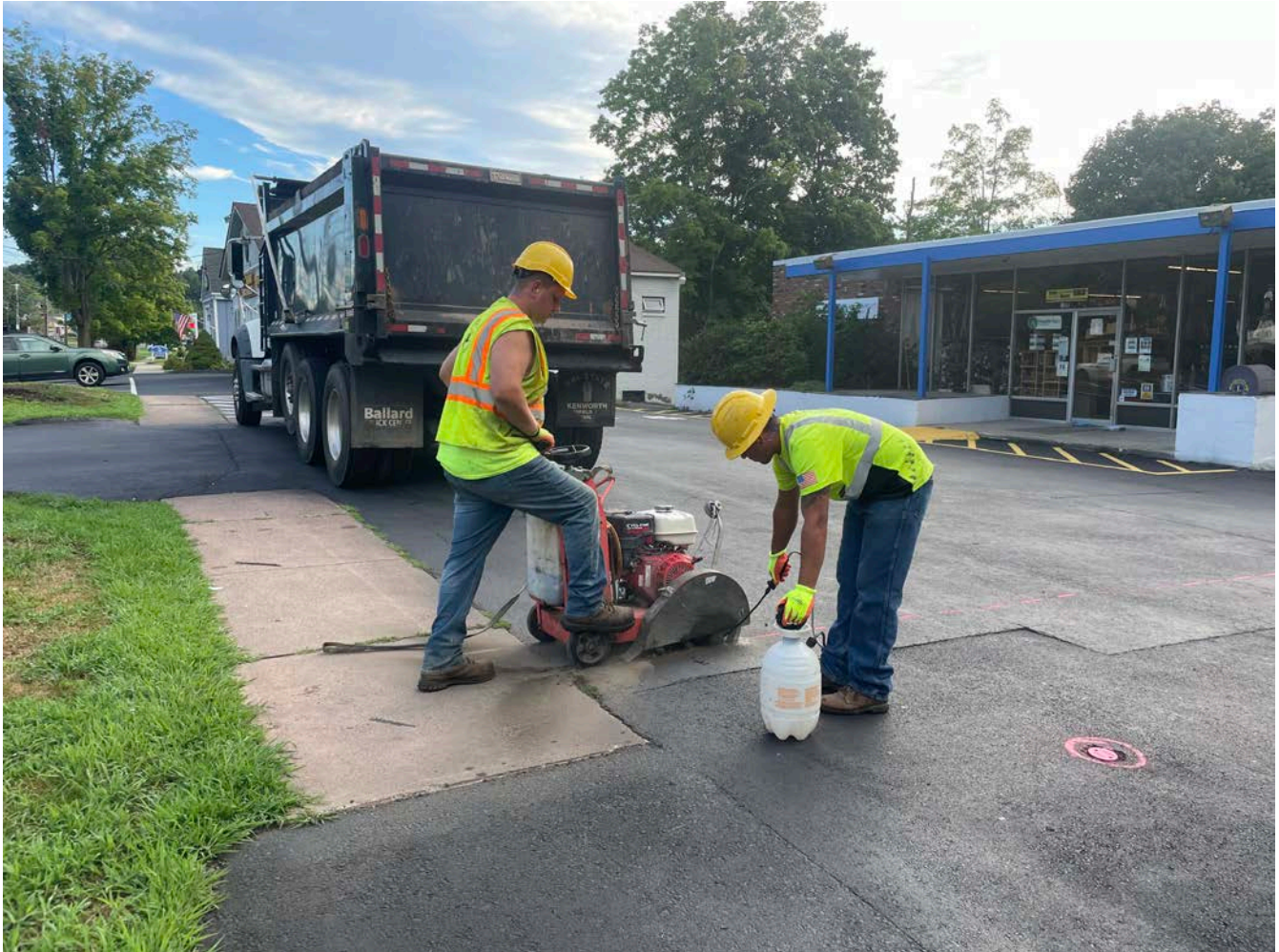
Picture 1: Ludlow saw-cutting the footprint of a trench overcut in order to place permanent pavement on the driveway of the 321 Main Street, Durham, property. View to the north.
