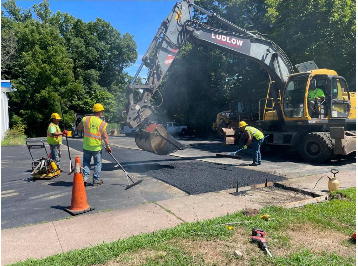
Picture 10: Ludlow placing the second lift of asphalt on the trench overcut footprint at the 321 Main Street, Durham, property. View to the southeast.
