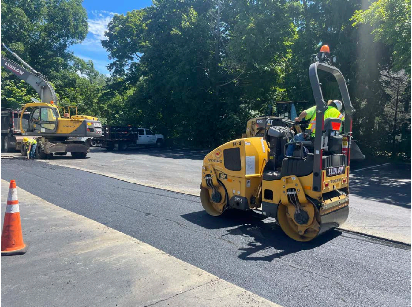
Picture 7: Ludlow using a rolling compactor on the first lift of asphalt that they placed within the footprint of the trench overcut at the 321 Main Street, Durham, property. View to the southeast.
