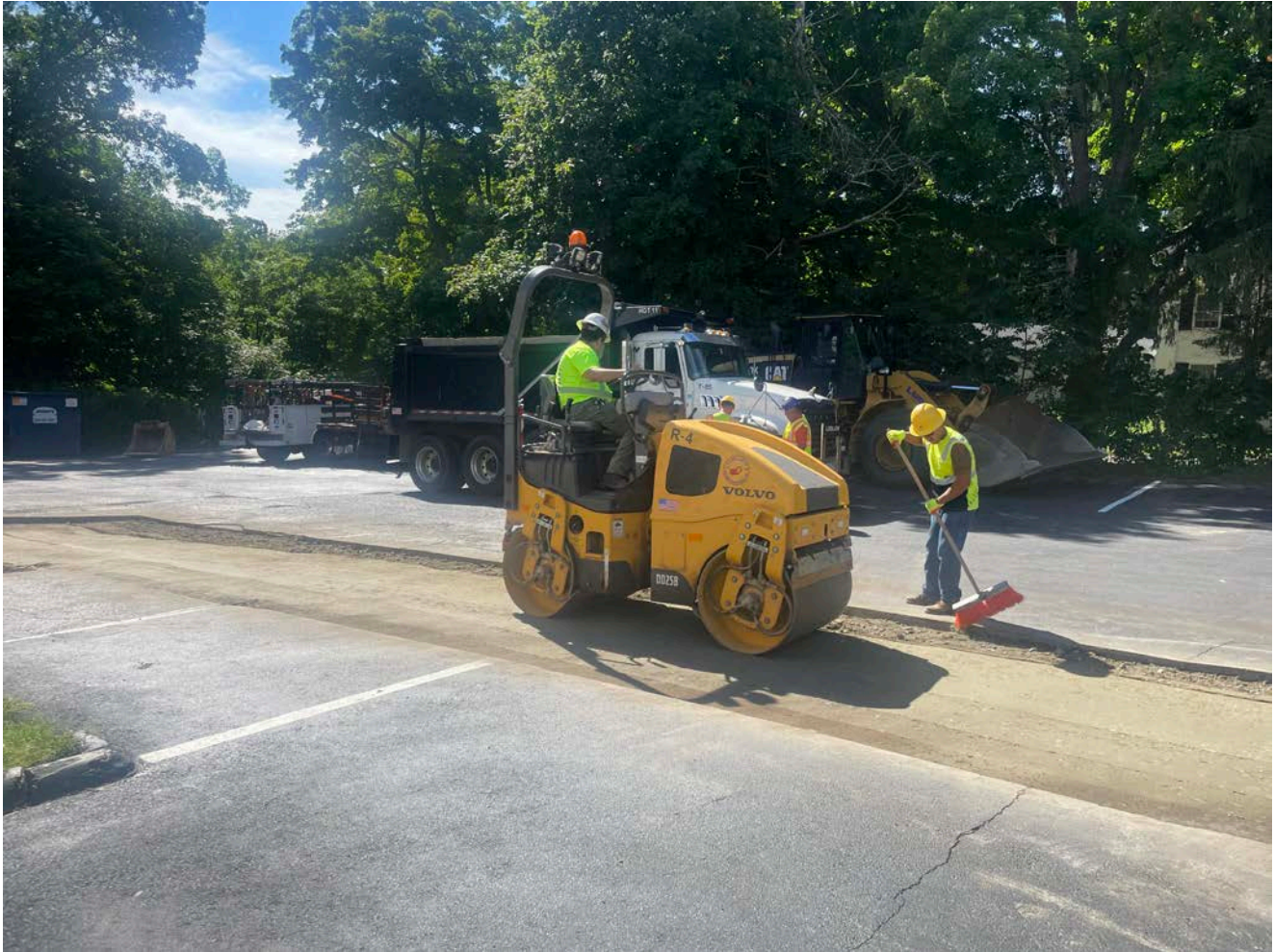
Picture 4: Ludlow compacting -1.25" processed gravel that they placed in the footprint of the trench overcut at the 321 Main Street, Durham, property. View to the southeast.
