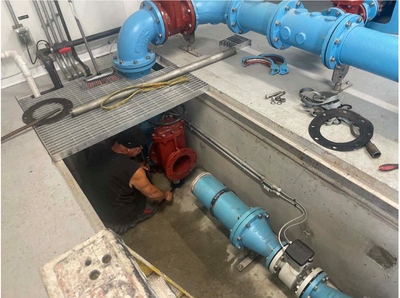
Picture 3: United concrete installing one of two 8" gate valves at the Booster Station located on S. Main Street in Middletown. View to the southeast.
