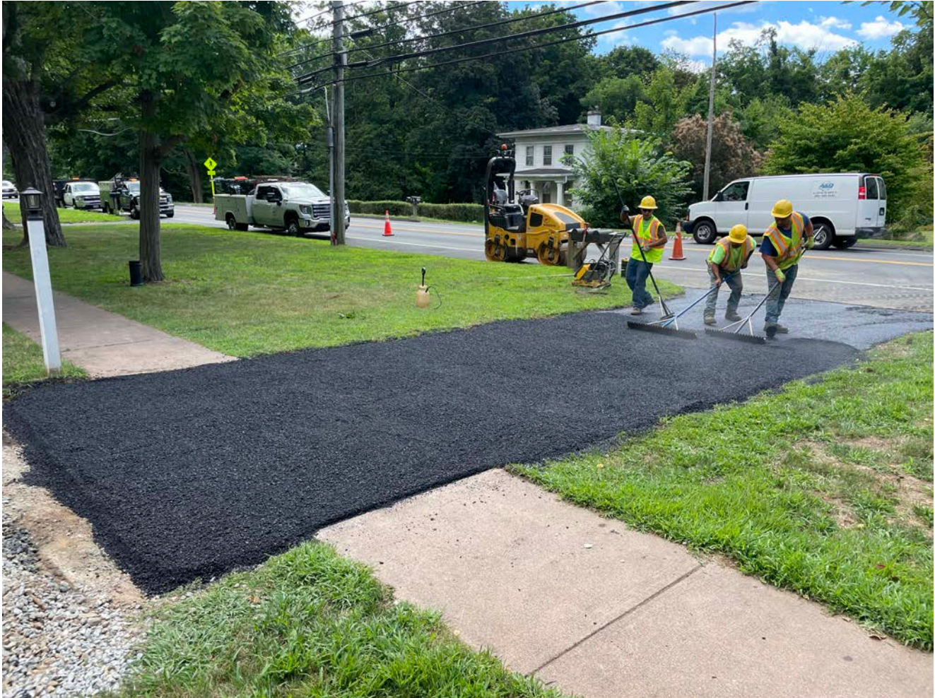
Picture 8: Ludlow grading the second lift of asphalt on the footprint of the driveway at the 303/305 Main Street, Durham, residences. View to the southwest.
