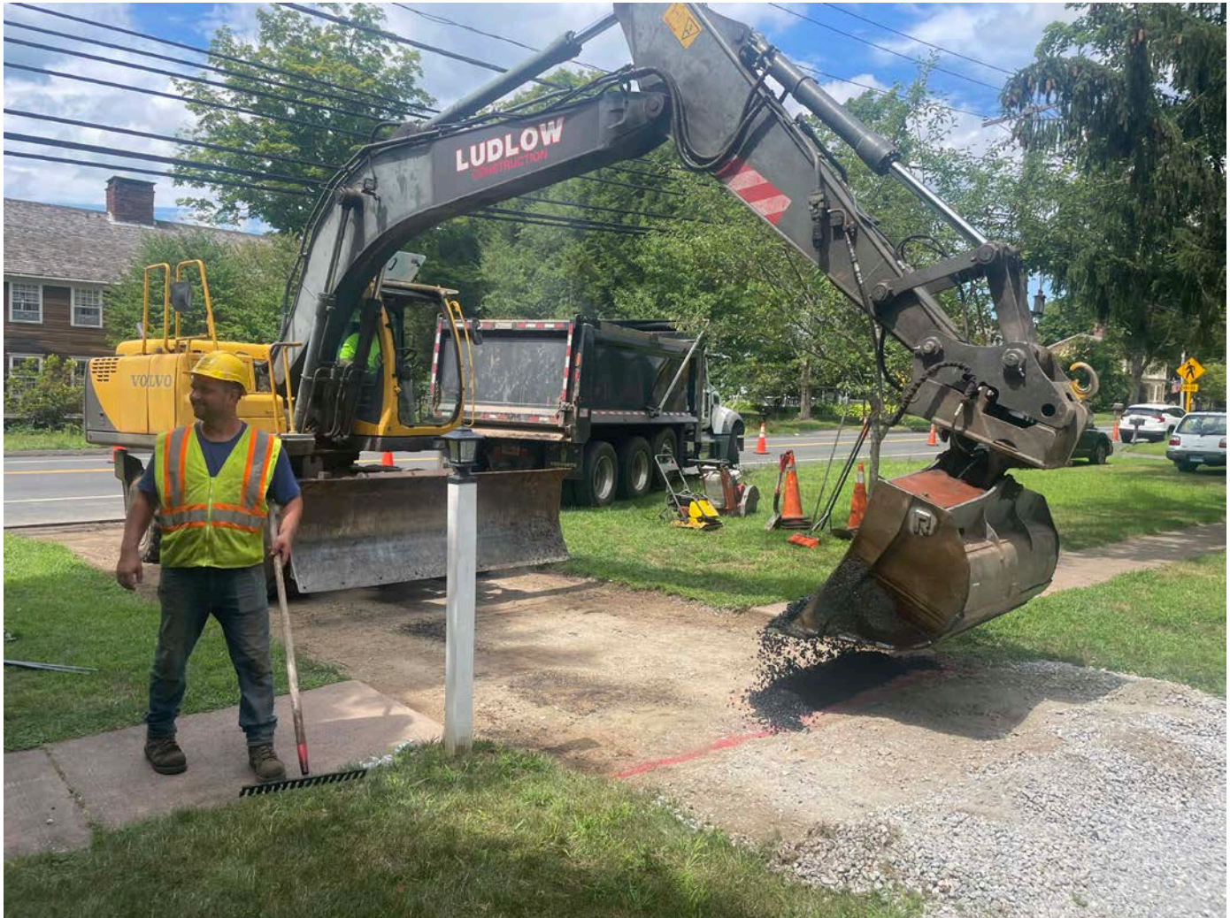
Picture 6: Ludlow placing the first lift of asphalt on the footprint of the driveway at the 303/305 Main Street, Durham, residences. View to the northwest.
