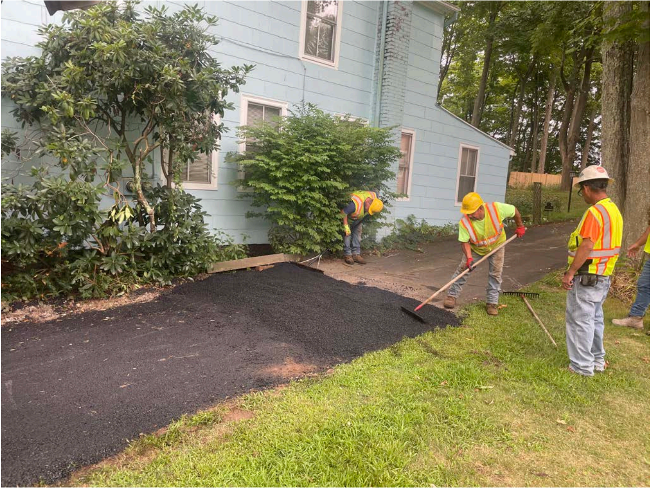
Picture 2: Ludlow grading the first lift of asphalt they are placing today on a portion of the driveway located on the 208 Main Street, Durham, property. View to the southwest.
