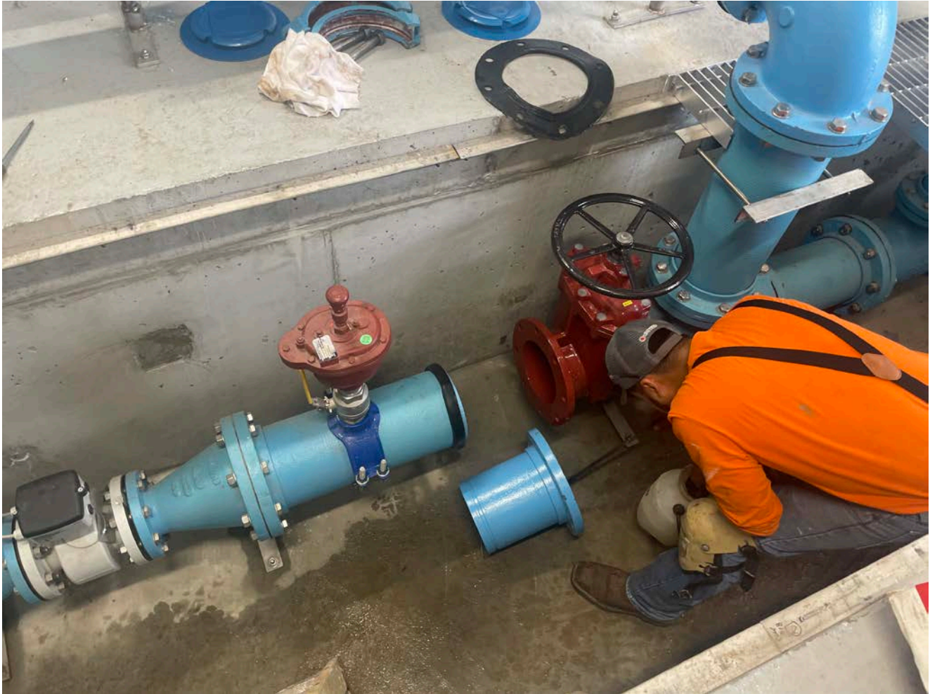
Picture 4: United concrete installing they second of two 8" gate valves at the Booster Station located on S. Main Street in Middletown. View to the south.
