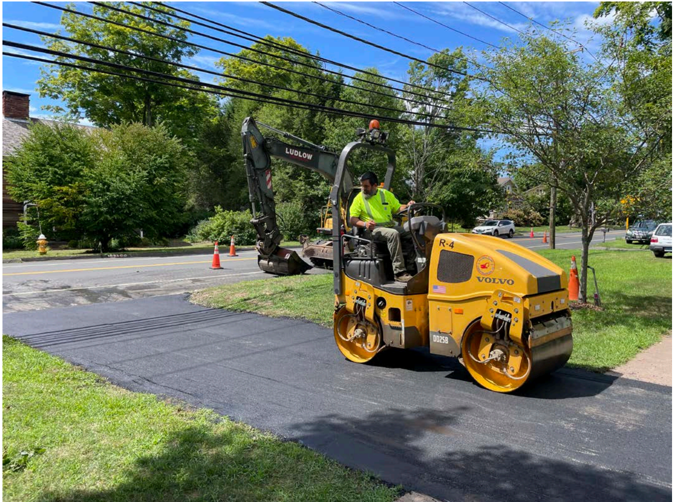
Picture 9: Ludlow compacting the second lift of asphalt they placed on the footprint of the driveway at the 303/305 Main Street, Durham, residences. View to the northwest.
