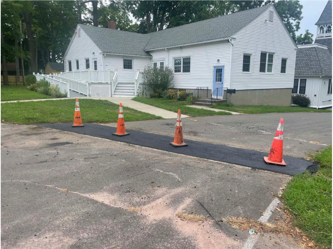
Picture 5: Permanent paving that Ludlow placed on the footprint of the trench they made when they previously installed a copper water service at the 196 Main Street, Durham, property. View to the northwest.
