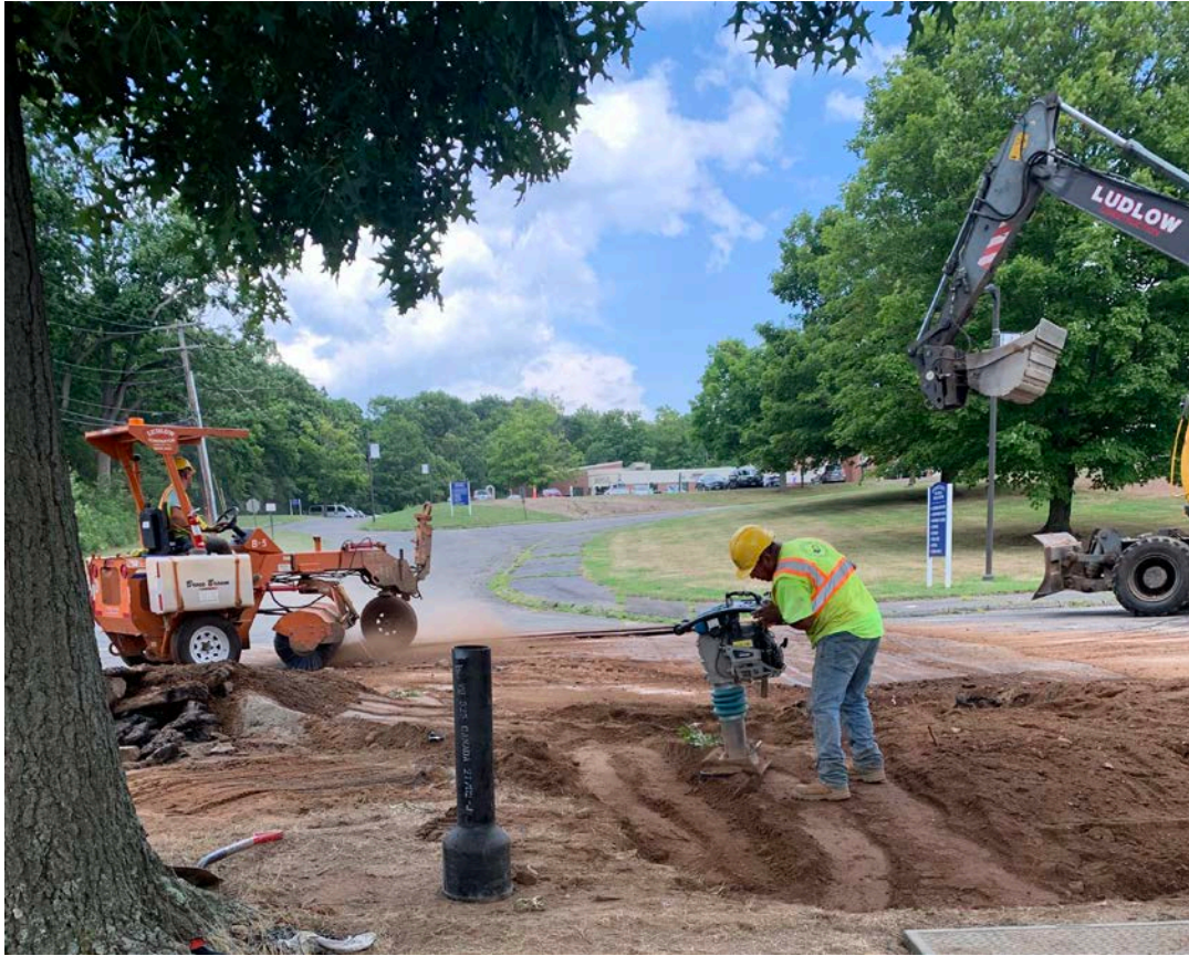
Photo 6: Ludlow Construction finishes the backfilling of the excavated trench at the former Korn School by compacting the ground with a compactor and prepping it for loam.
