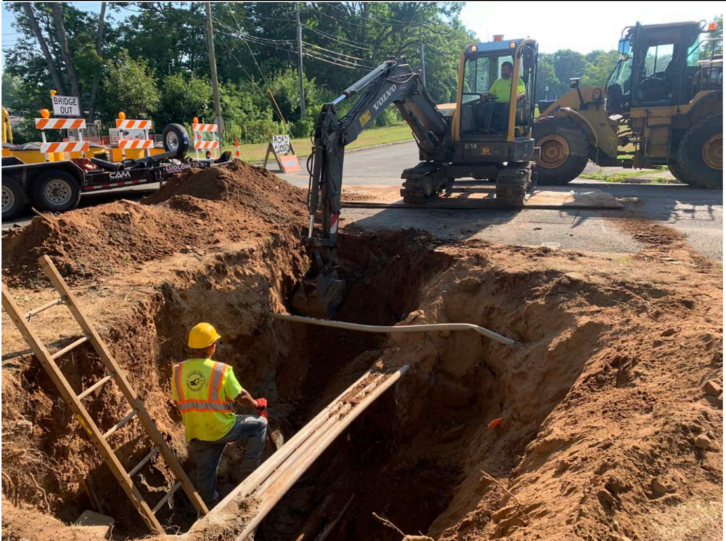
Photo 1: Ludlow Construction begins to excavate on Pickett Lane to access the fire service and domestic water service connections to the former Korn School.
