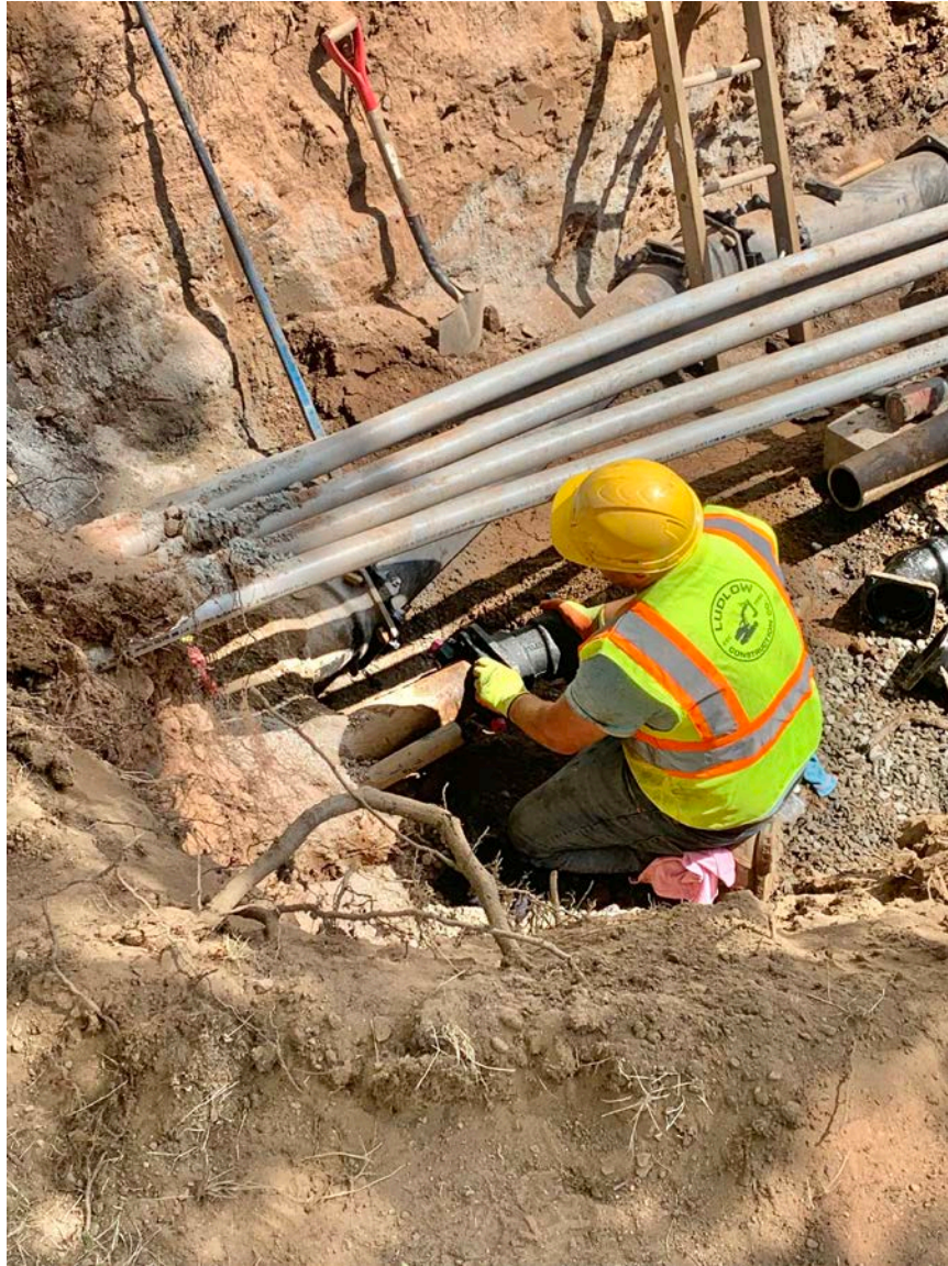
Photo 3: Ludlow Construction is connecting the 4" domestic water service at the former Korn School.
