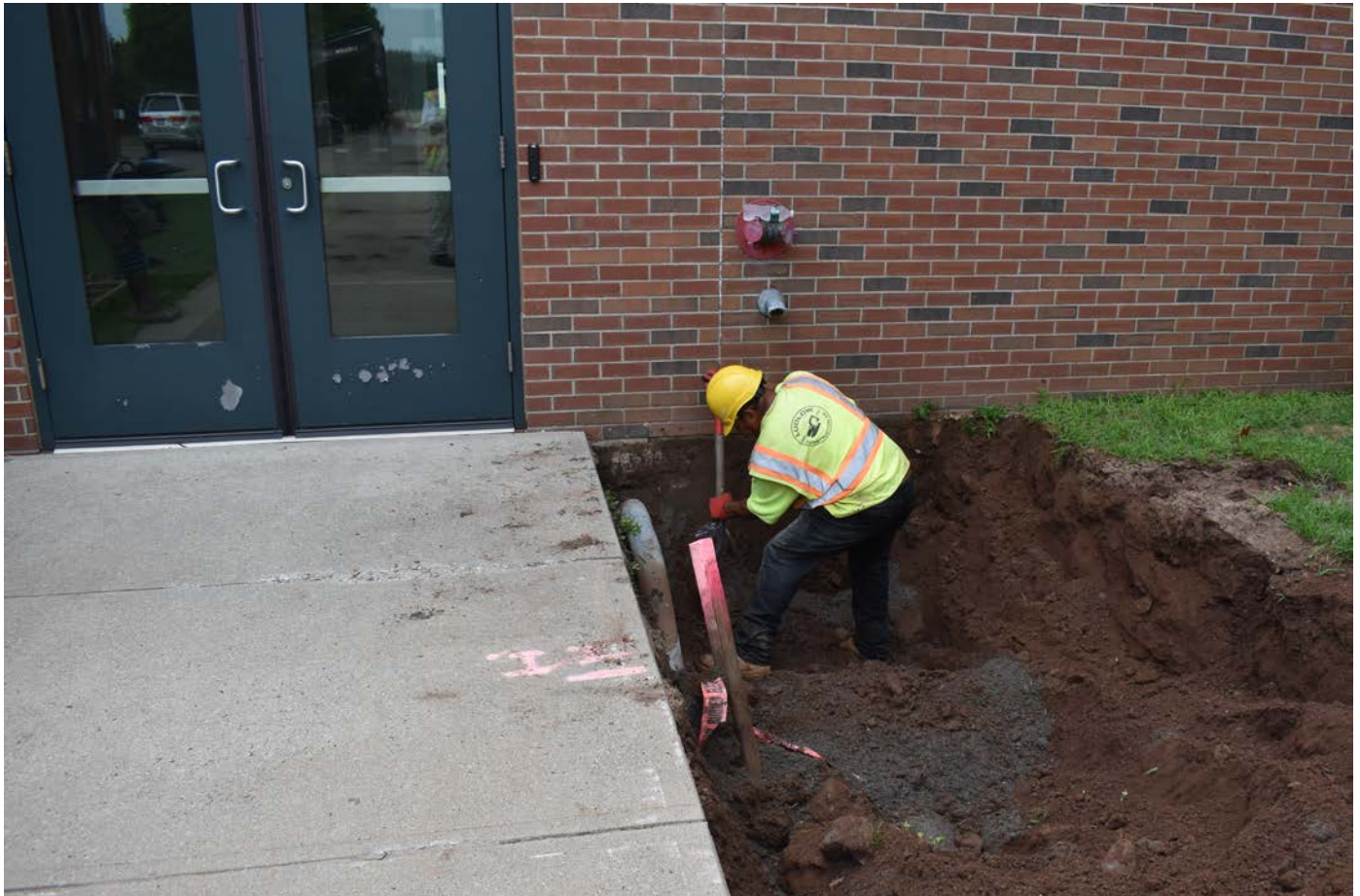
Photo 1: Ludlow laborer beginning excavation of supply line at school building wall. Electrical conduits visible adjacent to sidewalk. View to the east.
