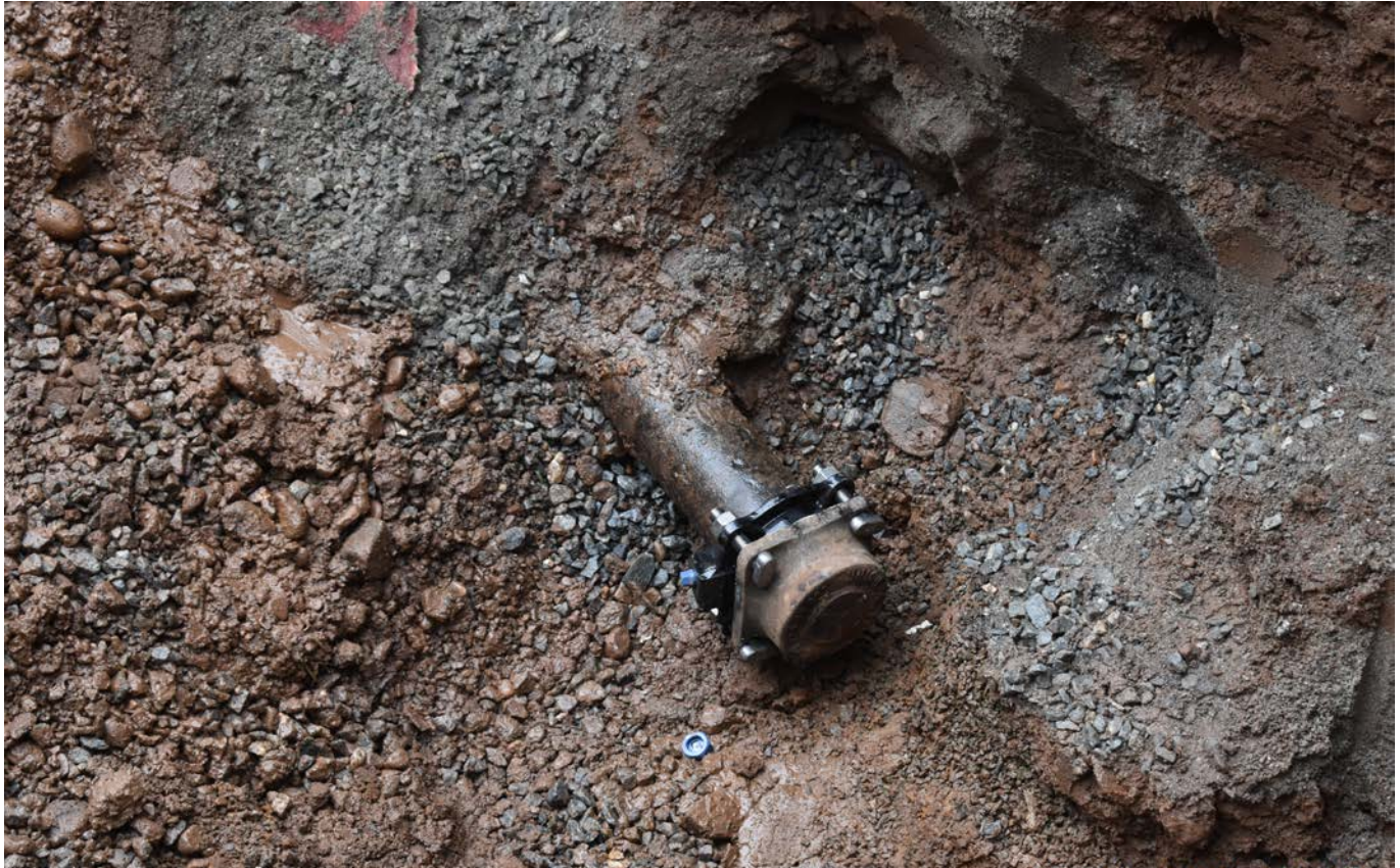
Photo 4: Capping completed at end of existing supply pipe adjacent to school. View to the northwest.
