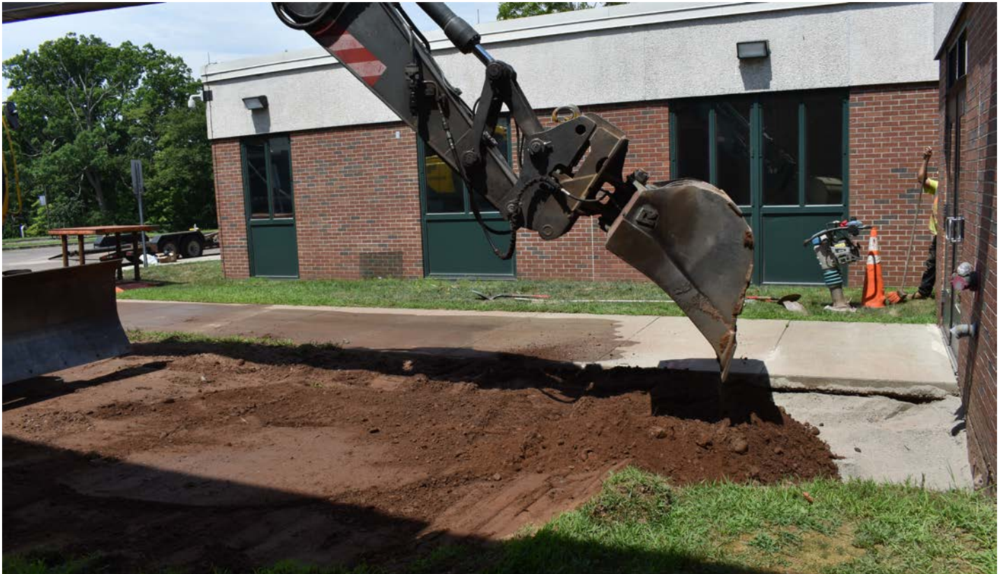
Photo 7: Ludlow placing backfill over pipe trench. View to the north.
