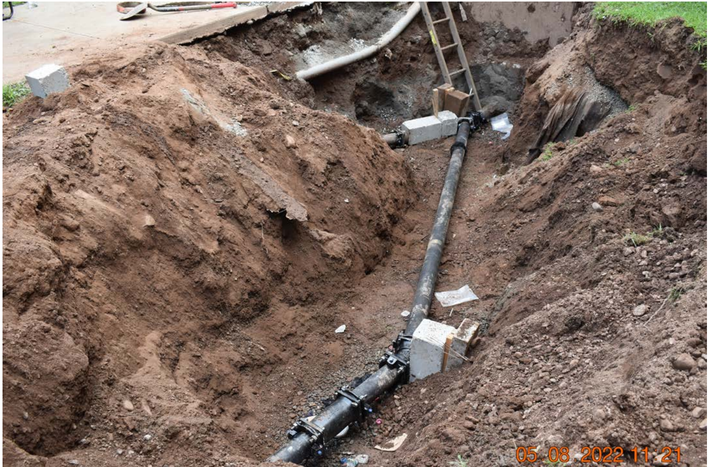
Photo 5: Completed pipe connection to new supply line at school wall, with thrust blocks added. View to the east.
