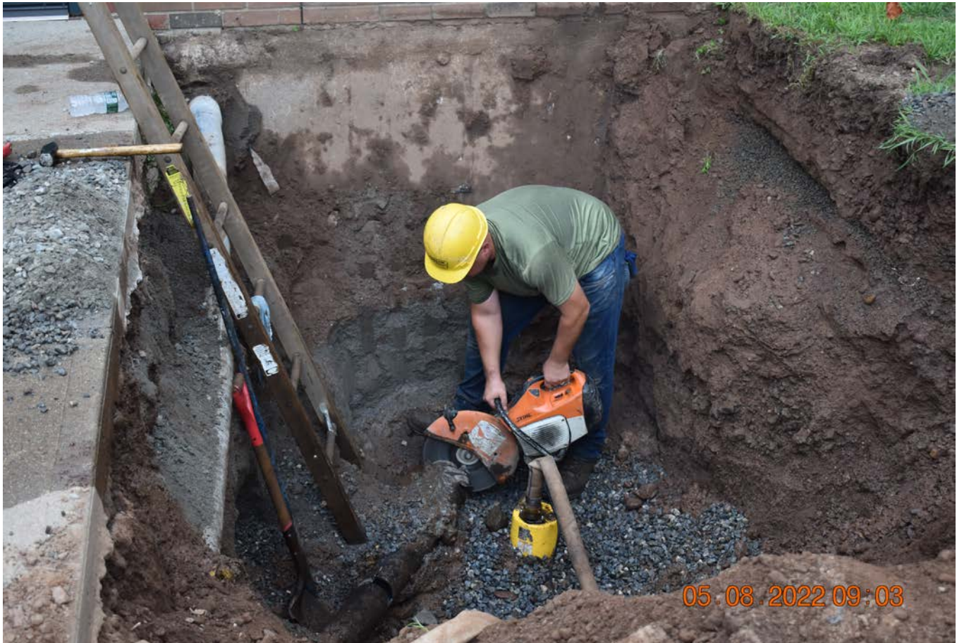
Photo 3: Ludlow making second cut to remove section of existing supply pipe at school wall. View to the east.
