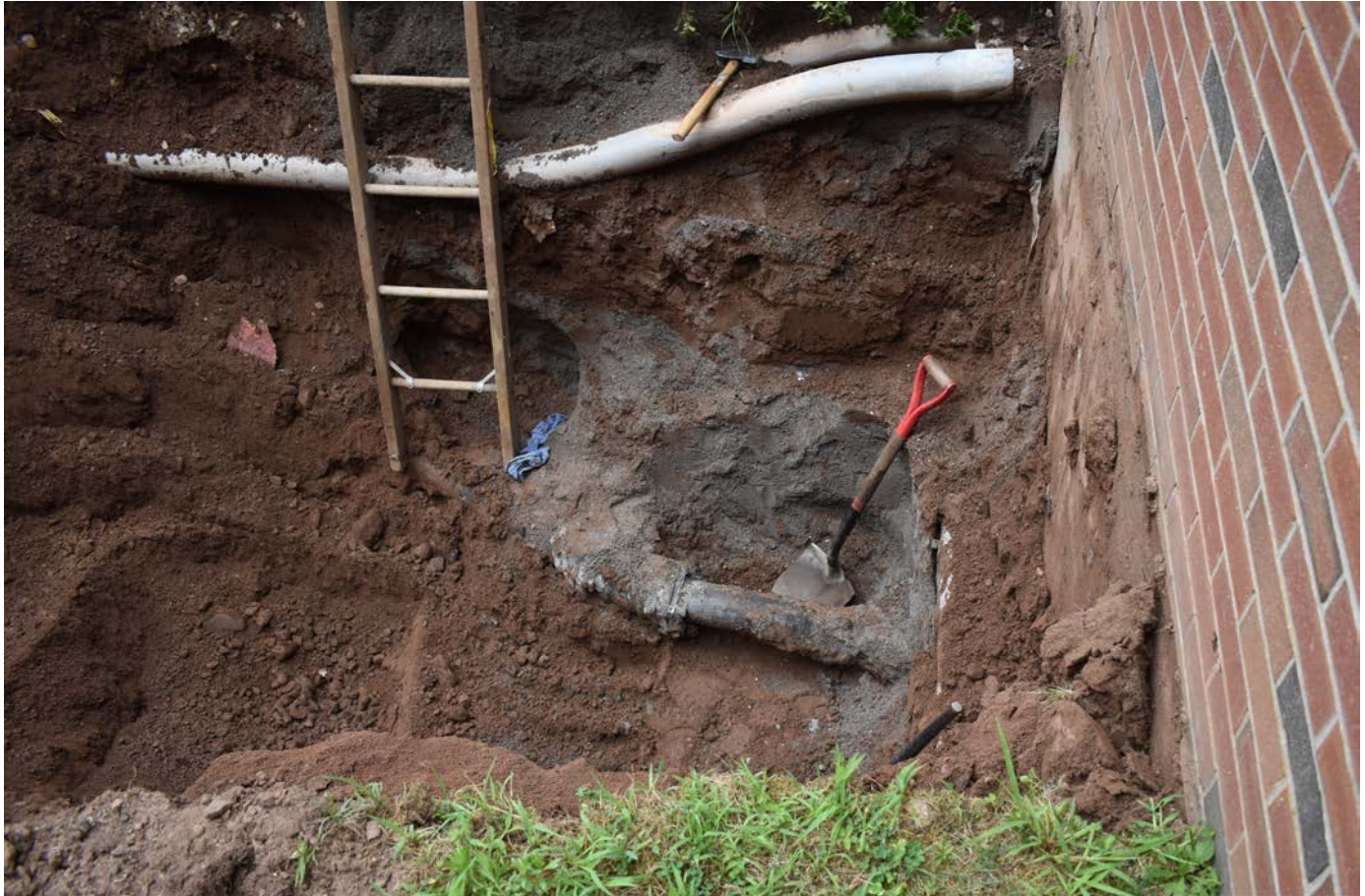
Photo 2: 4-inch existing supply pipe exposed. View to the north.
