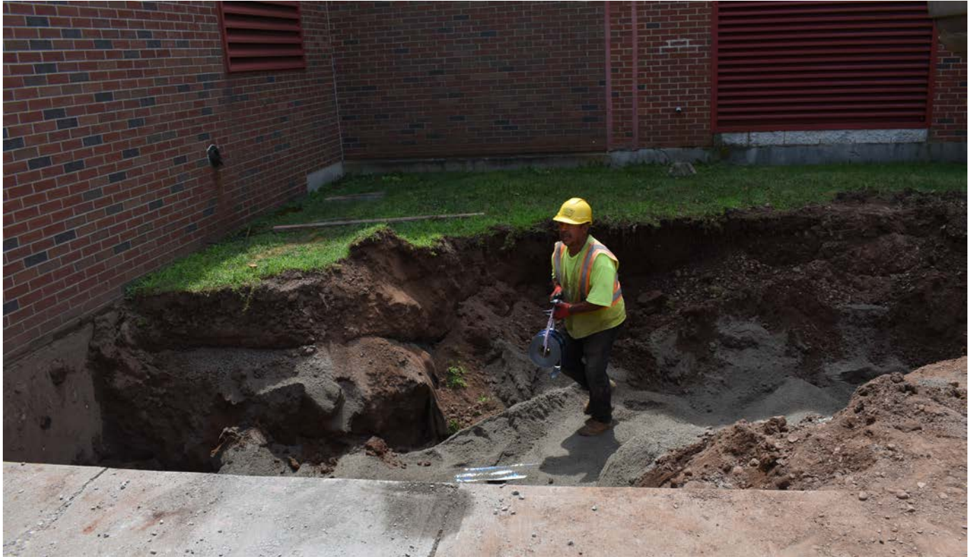
Photo 6: Ludlow laborer placing marker tape over new supply line. View to the south.
