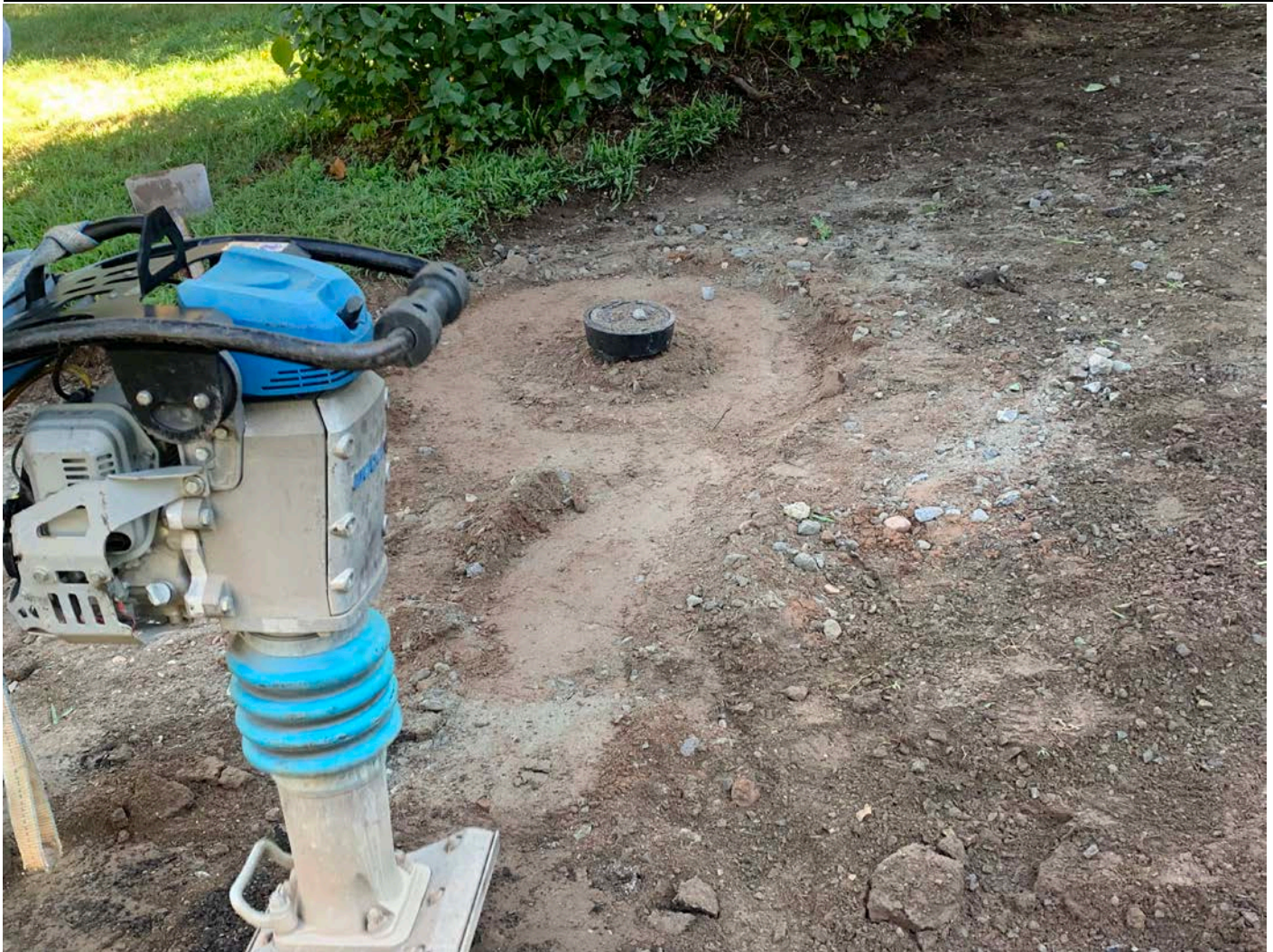
Picture 3: Ludlow Construction is at 253 Main St resetting a curb stop located in the driveway. A compactor is being used to compact around the curb stop.
