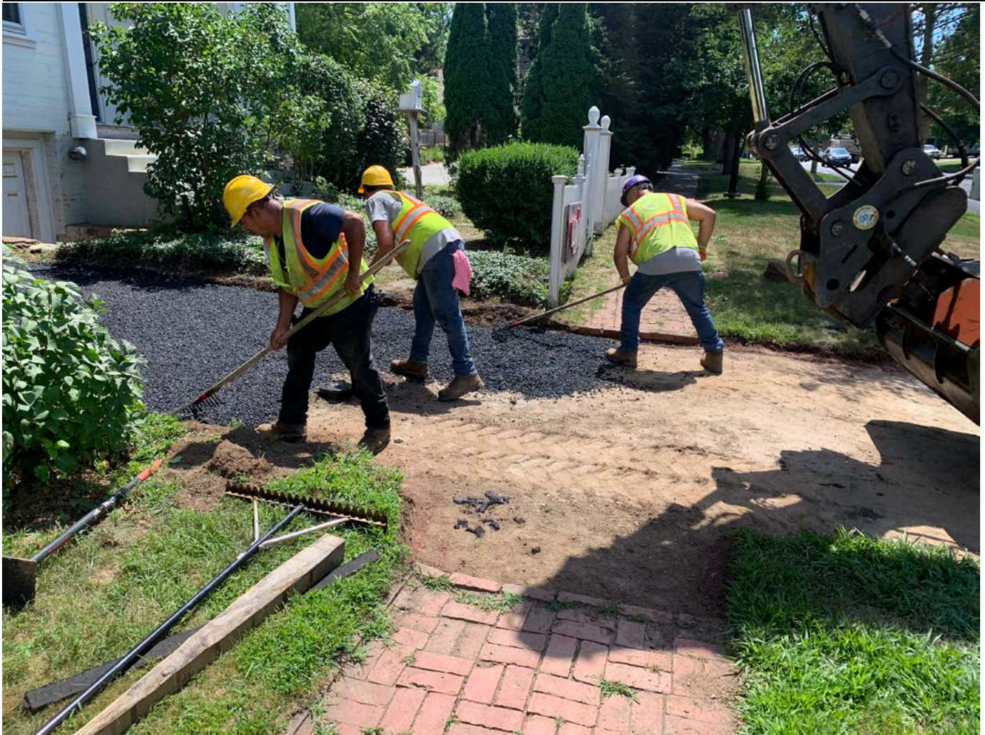
Picture 5: Ludlow Construction is laying the first layer asphalt at 253 Main St. (2 inches of 0.5 inch of aggregate of asphalt).
