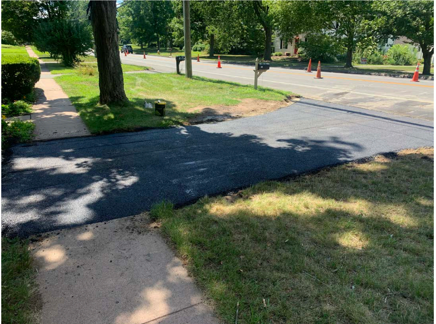
Picture 4: Ludlow Construction is at 271 Main St laying the first layer of asphalt (2 inches of 0.5 inch of aggregate of asphalt).
