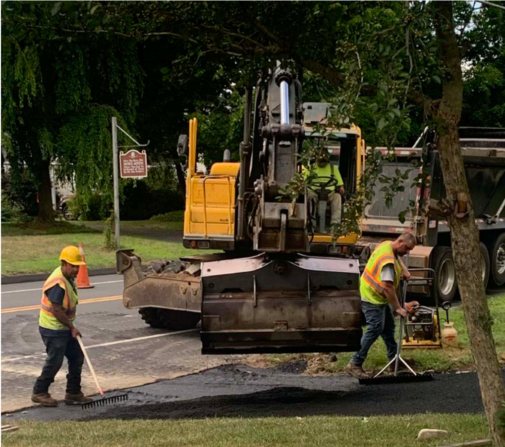
Picture 6: Ludlow Construction is at 253 Main St laying the second layer of asphalt (1 inch of 0.35-inch asphalt aggregate).
