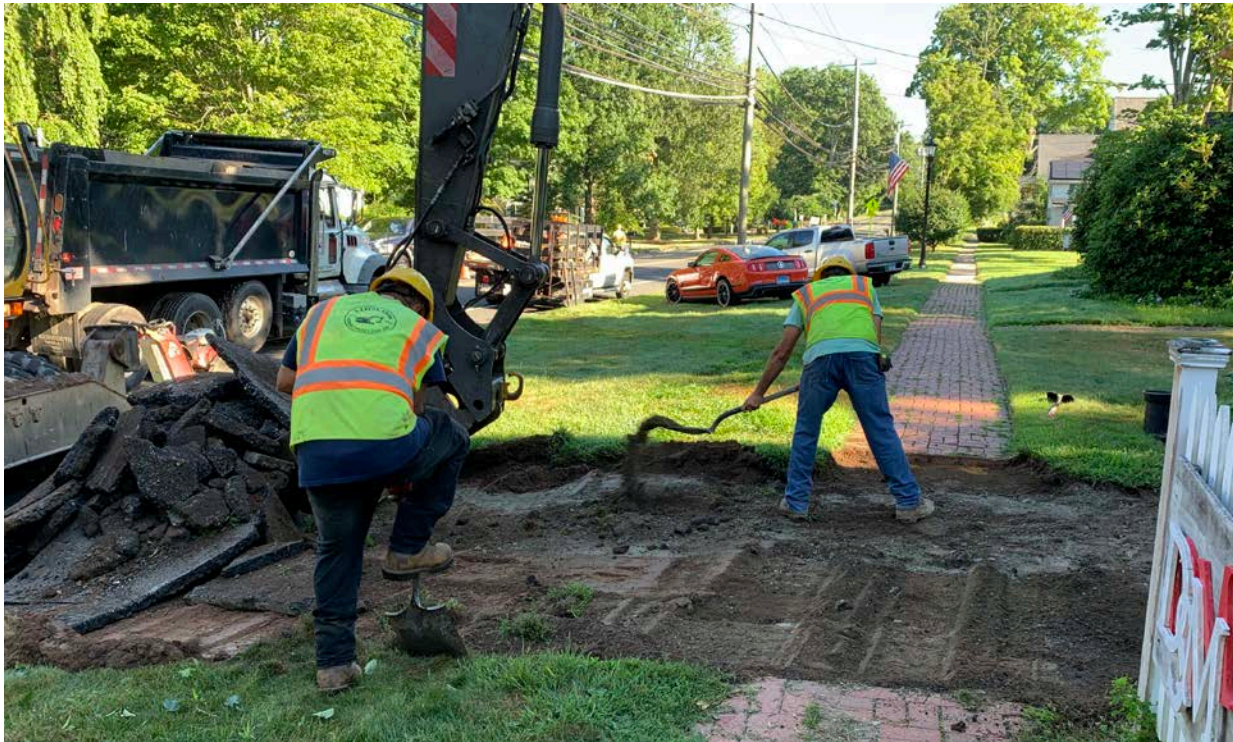
Picture 1: Ludlow Construction is at 253 Main St removing the existing blacktop of the entrance of the driveway using excavator and Ludlow Construction personnel.
