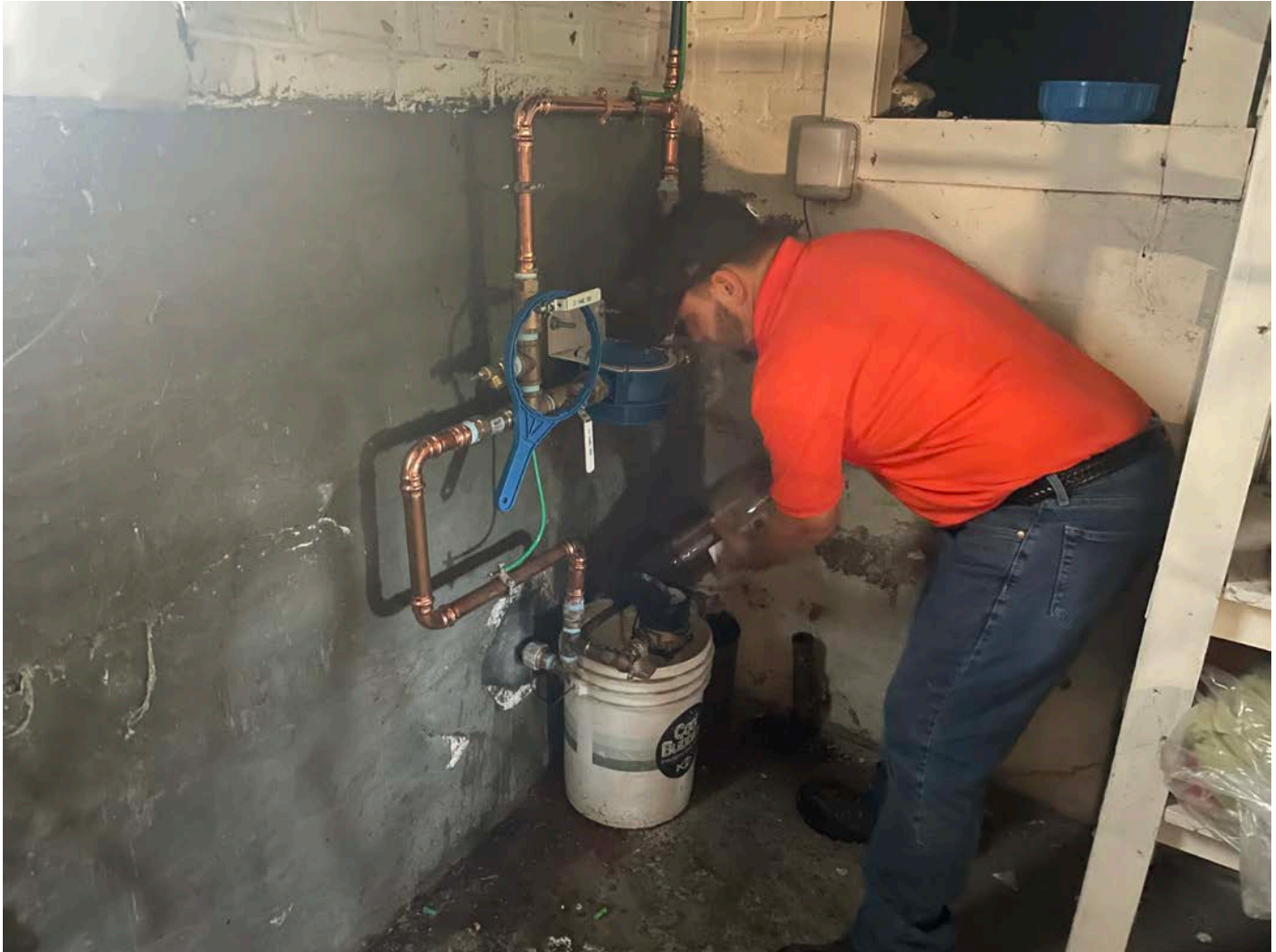
Picture 5: Fazzino changing the filter on the water system they recently installed at the 175 Maple Avenue, Durham, residence.
