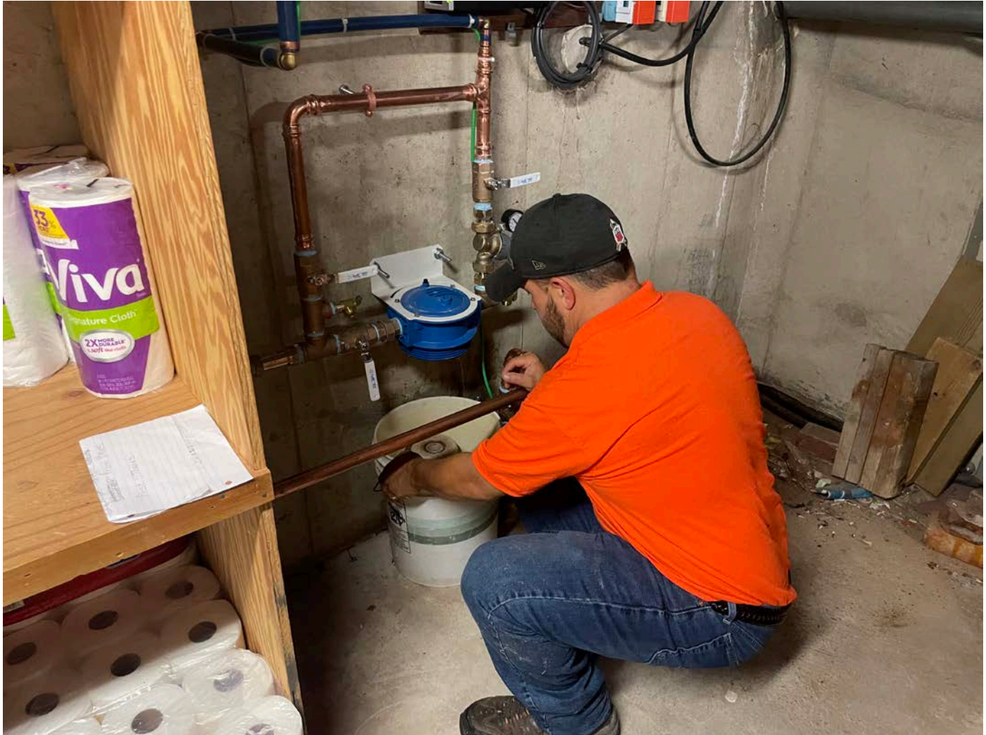
Picture 10: Fazzino changing the filter on the water system they recently installed at the 321 Main Street, Durham, residence.
