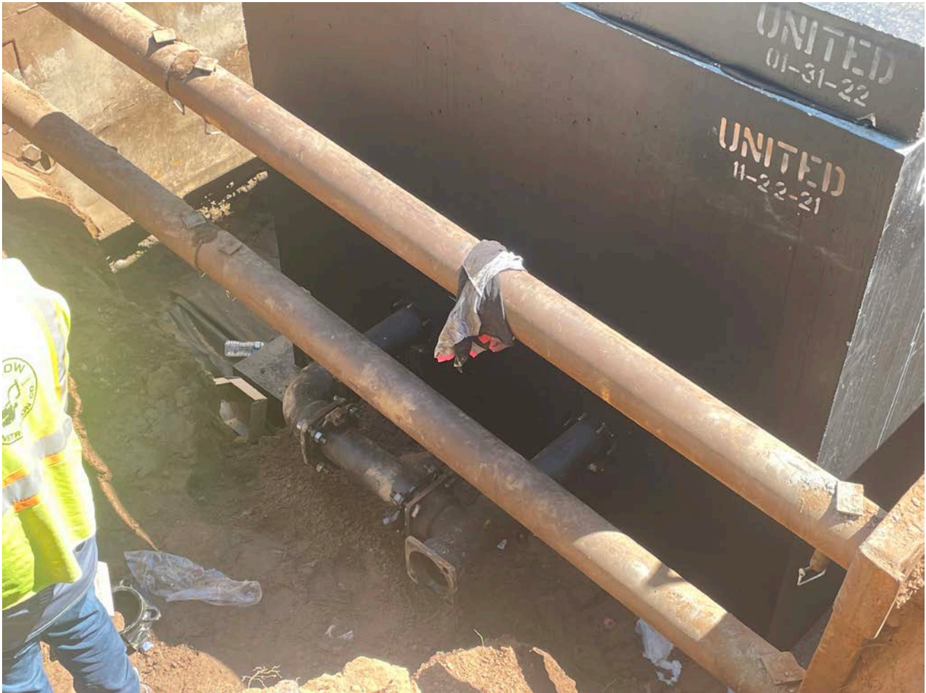
Picture 14: 4" DIP pipe and fittings that Ludlow has installed on the west side of the vault they are installing at Station 525+75. View to the northeast.
