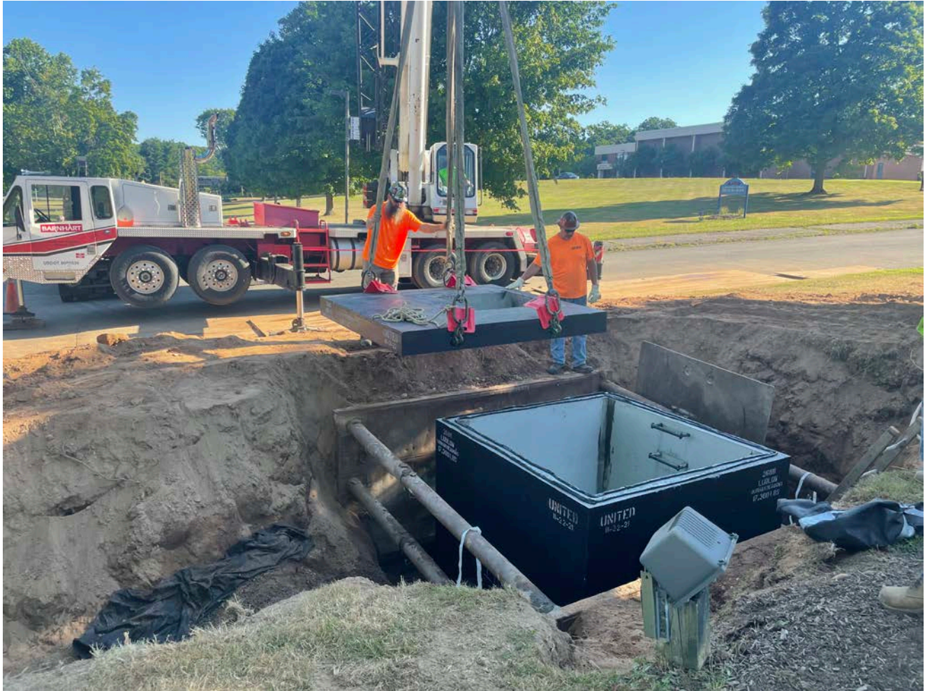
Picture 12: Barnhart and Ludlow placing the top section of the vault they are installing at Station 525+75 on Pickett Lane, Durham. View to the northeast.
