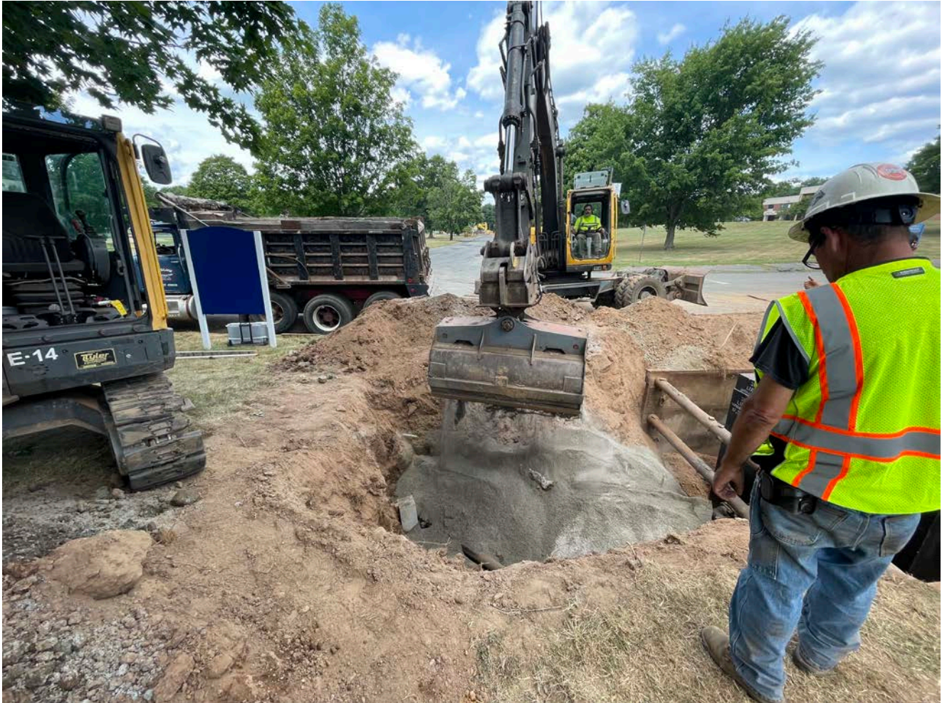
Picture 18: Ludlow placing sand over the 4" DIP they installed on the west side of the vault they installed at Station 525+75. View to the north.
