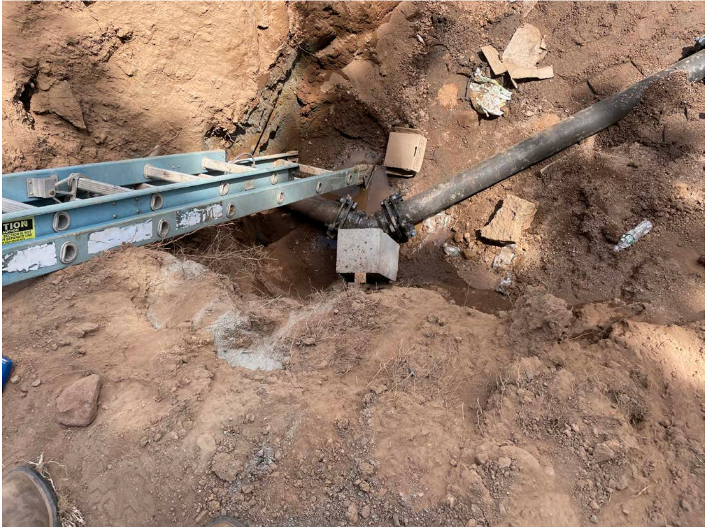
Picture 16: 4" DIP pipe and associated thrust blocks that Ludlow installed to the west of the vault they are installing at Station 525+75.
