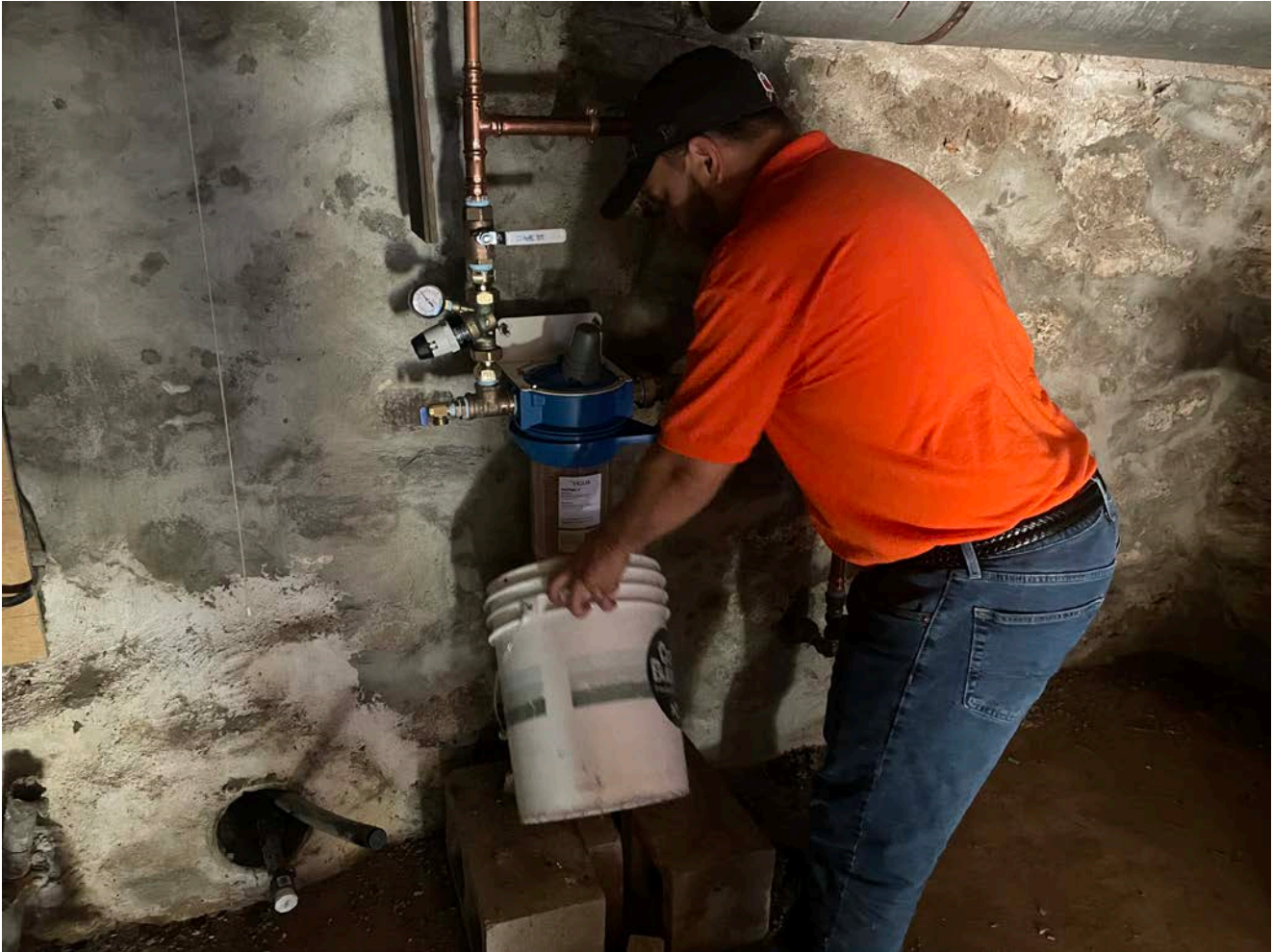
Picture 2: Fazzino changing the filter on the water system they recently installed at the 25 Talcott Lane, Durham, residence.
