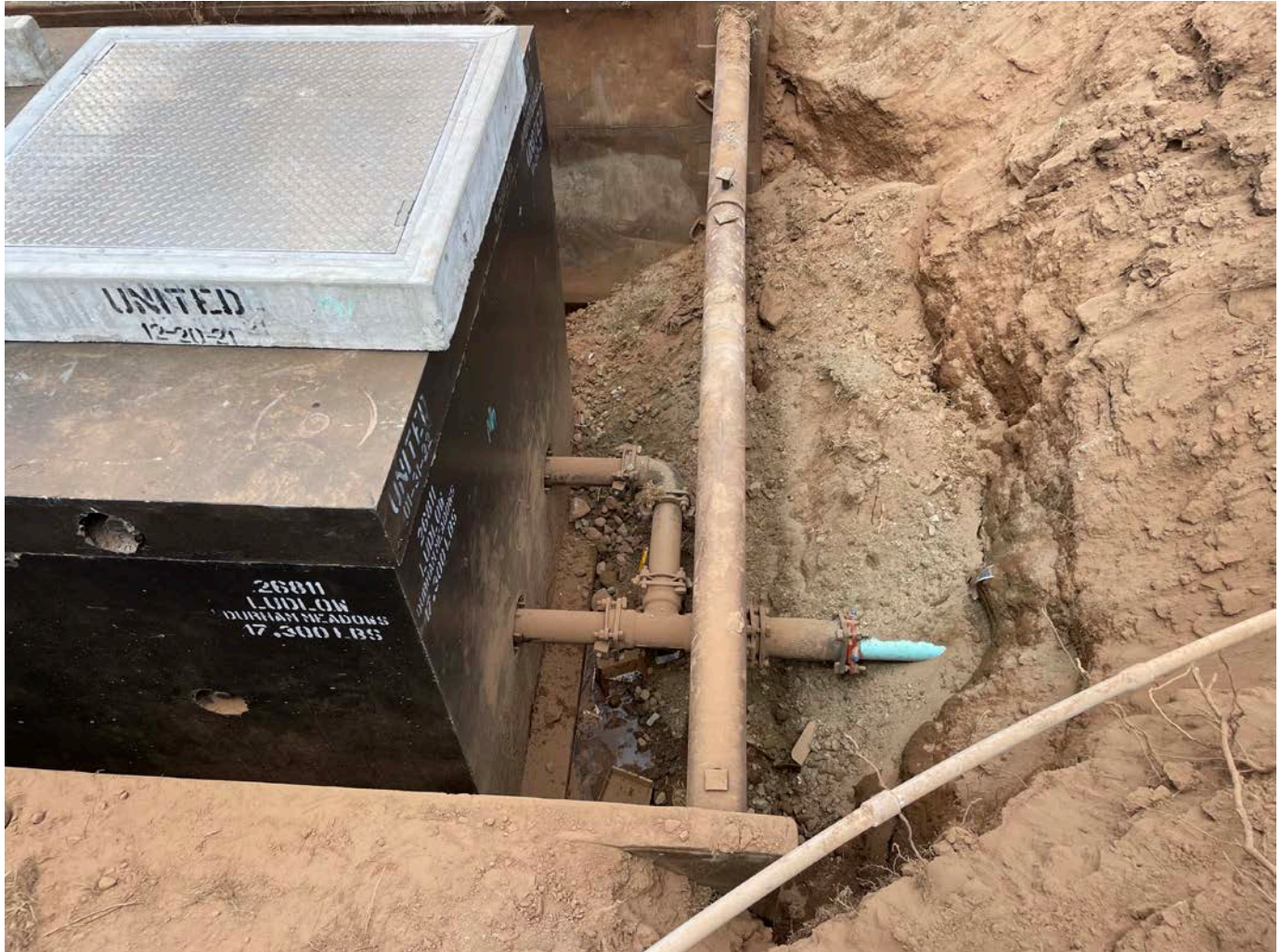
Picture 17: 4" DIP pipe and fittings that Ludlow has installed on the east side of the vault they are installing at Station 525+75. Note where the 4" DIP ties into the existing 4" PVC water line. View to the north.
