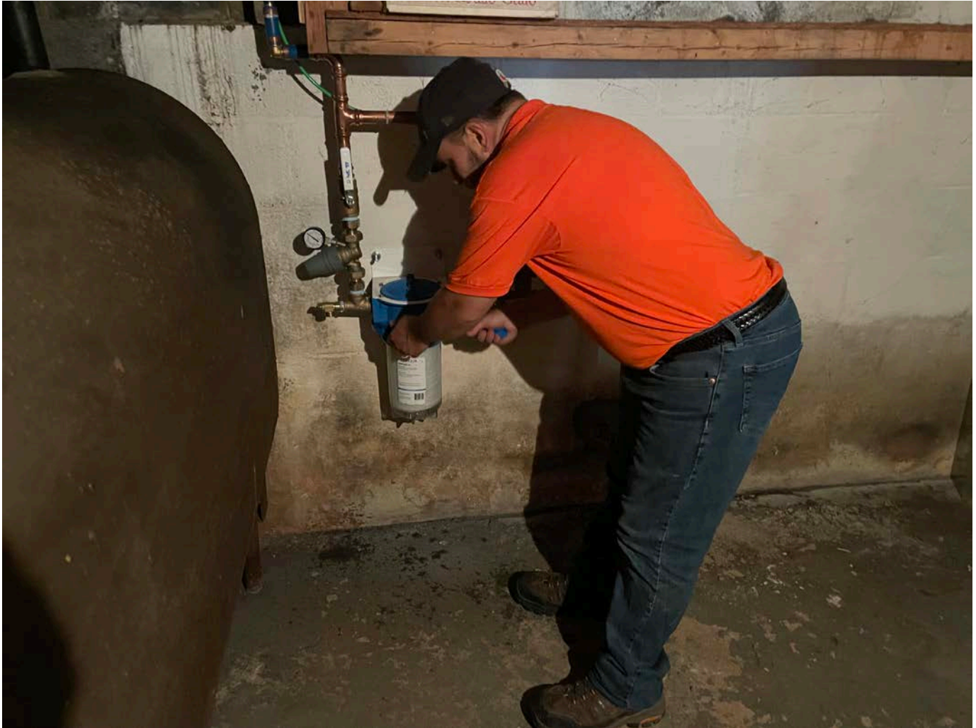
Picture 7: Fazzino changing the filter on the water system they recently installed at the 177R Main Street, Durham, residence.
