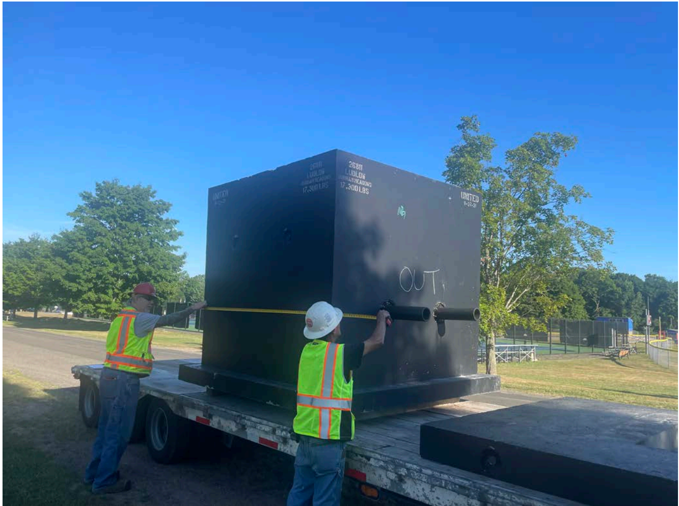
Picture 11: Ludlow measuring the vault delivered to the work zone by United Concrete that Ludlow will be installing at Station 525+75. View to the northwest.
