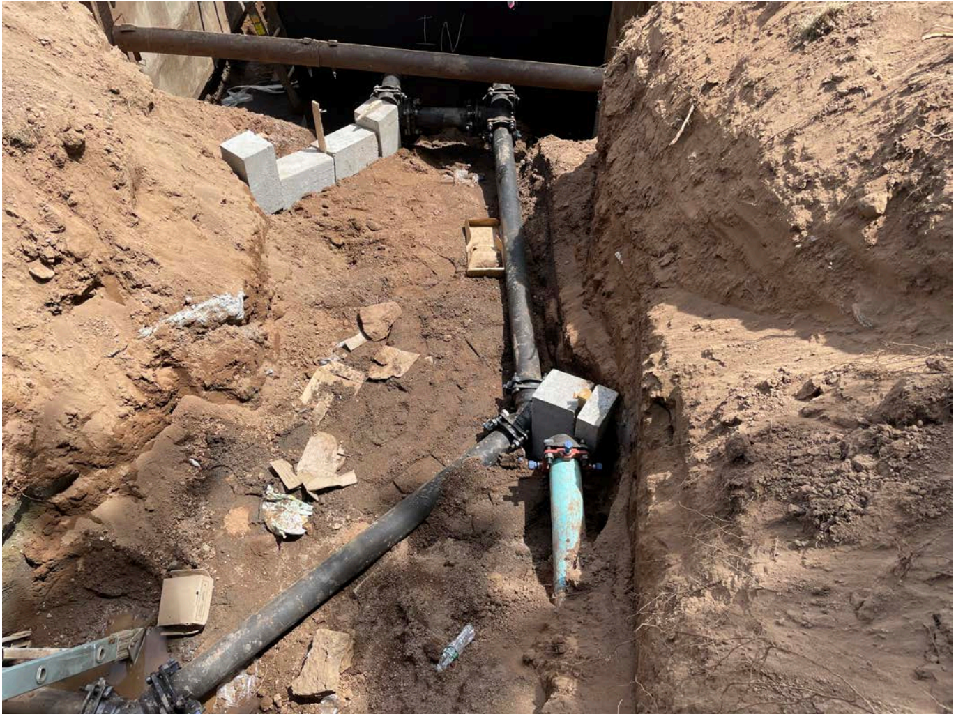
Picture 15: View of piping and thrust blocks that Ludlow installed on the west side of the vault they are installing at Station 525+75. Note the DIP cap that Ludlow placed on the blue 4" PVC water line that they cut. View to the east.
