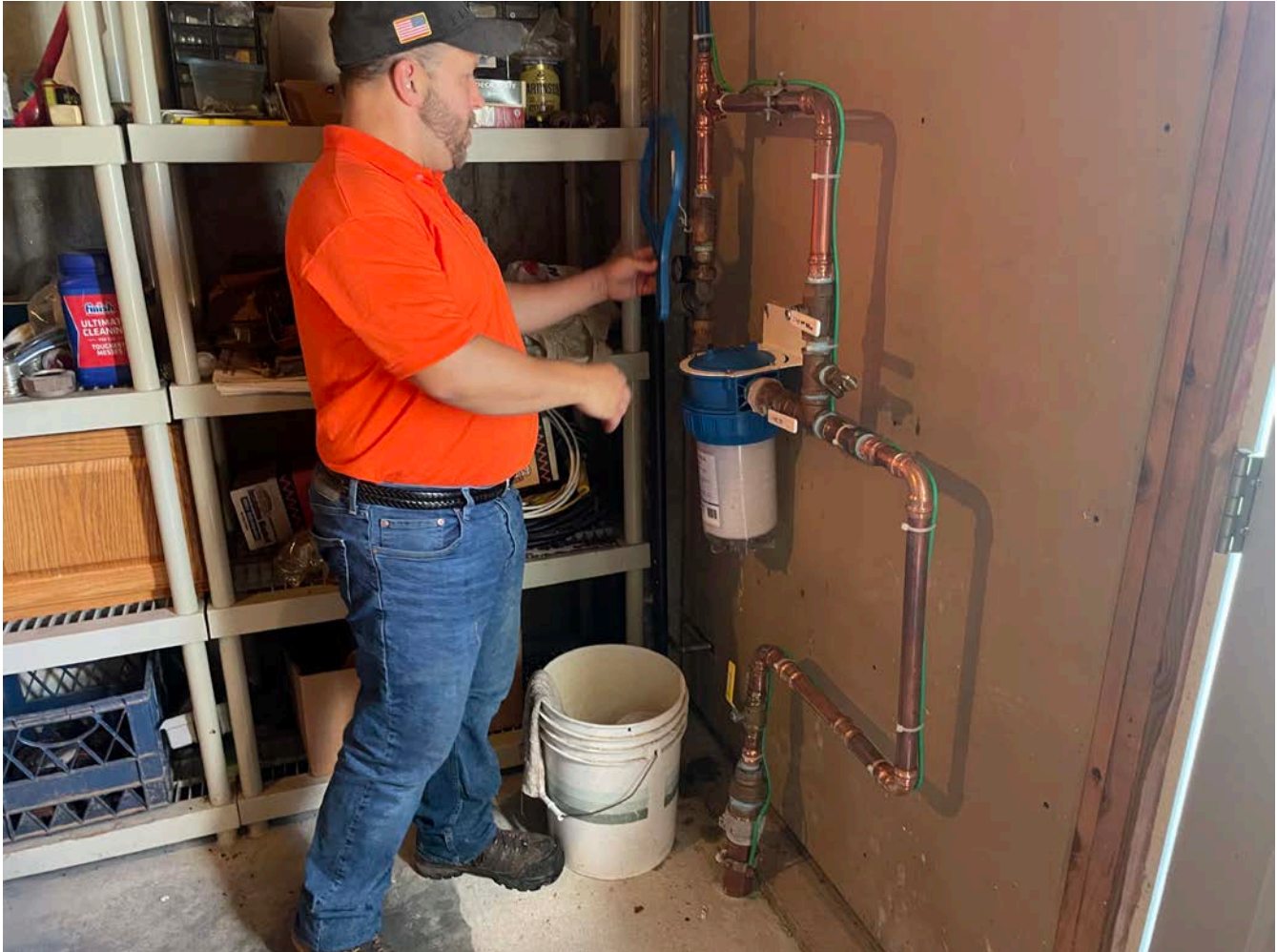
Picture 1: Fazzino changing the filter on the water system they recently installed at the 14 Talcott Lane, Durham, residence.
