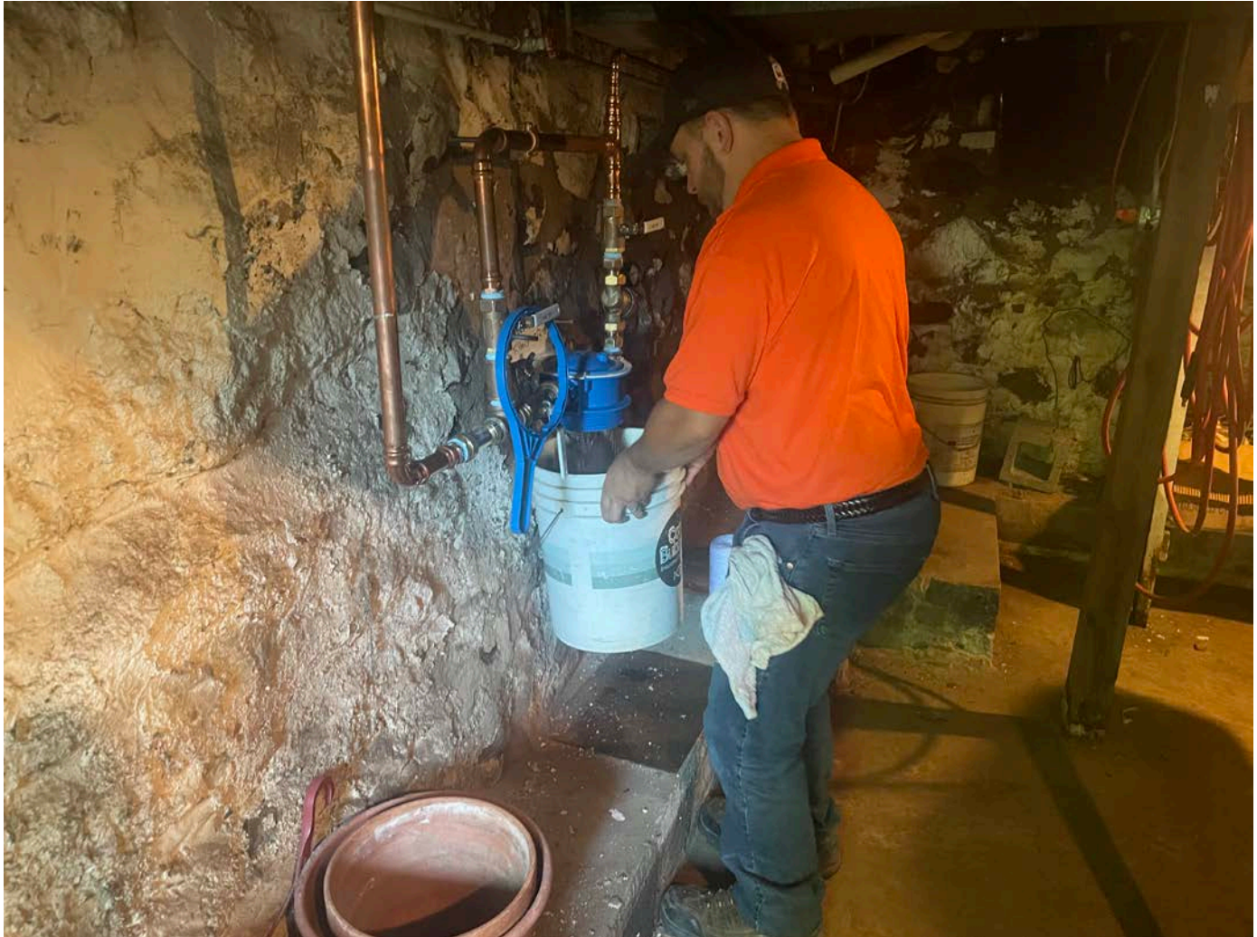
Picture 6: Fazzino changing the filter on the water system they recently installed at the 176 Maple Avenue, Durham, residence.
