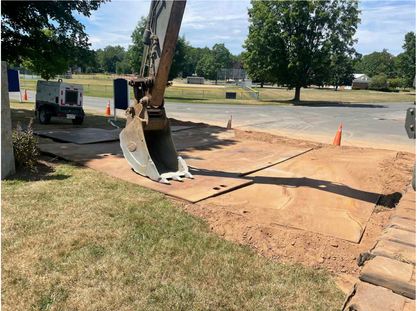
Picture 9: The excavation located at Station 525+75 on Pickett Lane that Ludlow has secured for the day after they finished work for the day.
