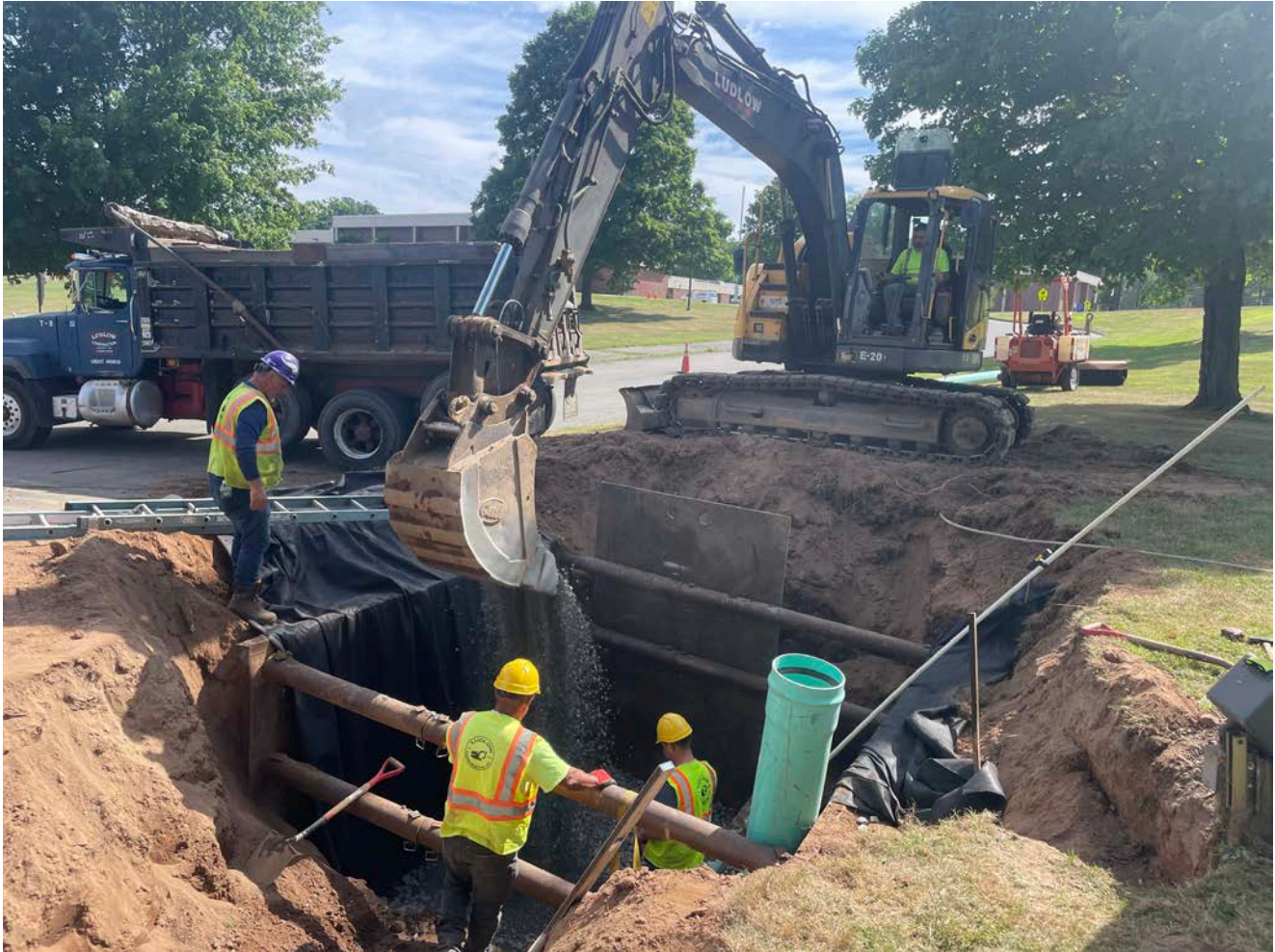
Picture 4: Ludlow placing 8" of \frac{3}{4} stone on top of the 4" of -2" stone that they placed on the bottom of the excavation where Ludlow will be installing a vault at Station 525+75.
