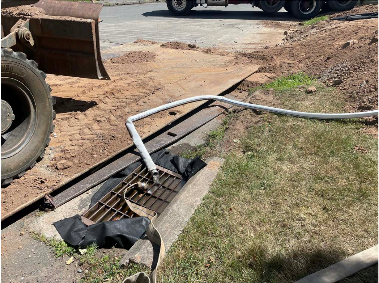
Picture 8: Water that Ludlow is pumping from the bottom of the excavation at Station 525+75 into the catch basin located at Station 525+49.
