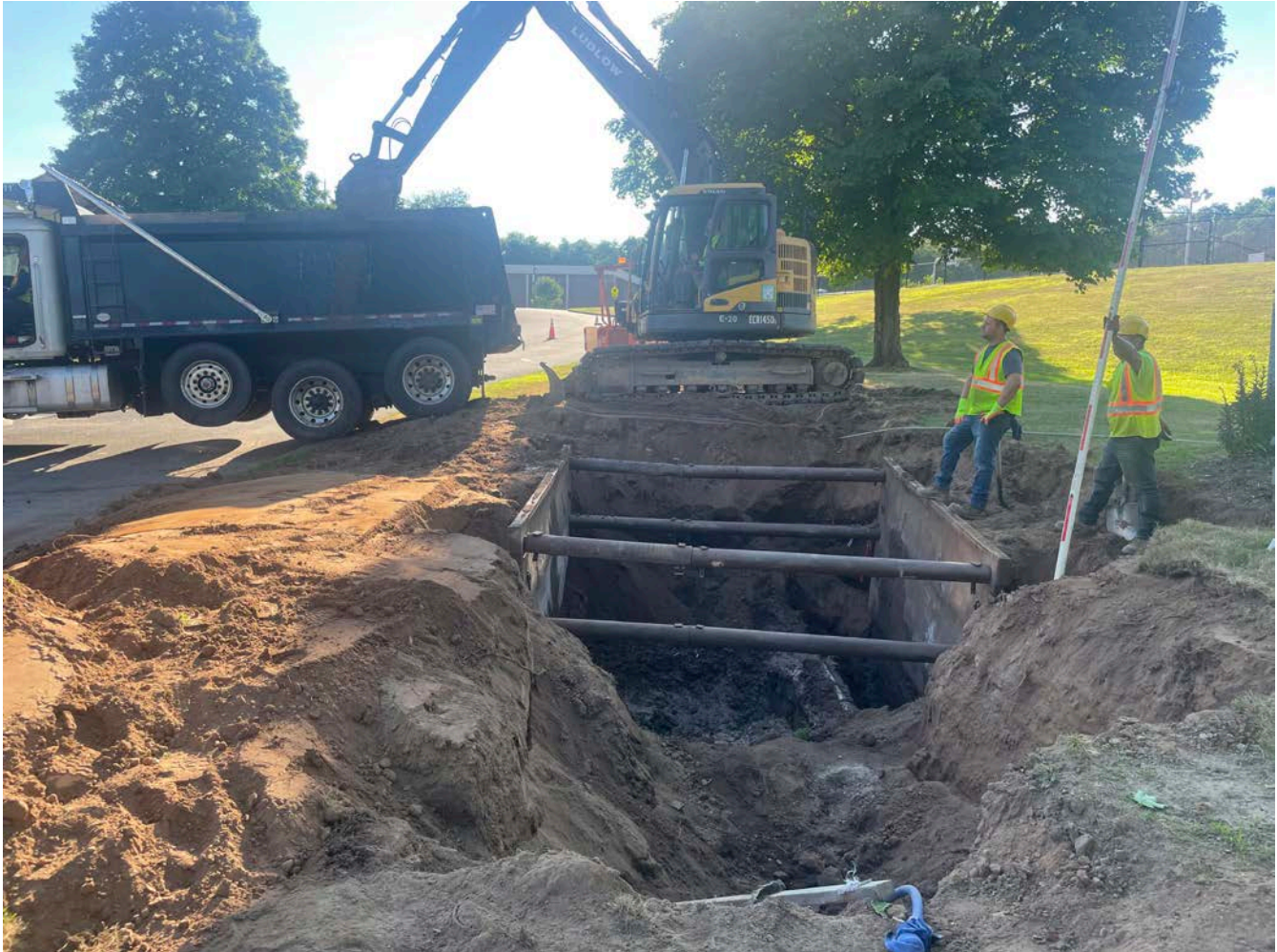
Picture 1: View of the excavation that Ludlow making for the placement of a vault at Station 525+75. View to the east.
