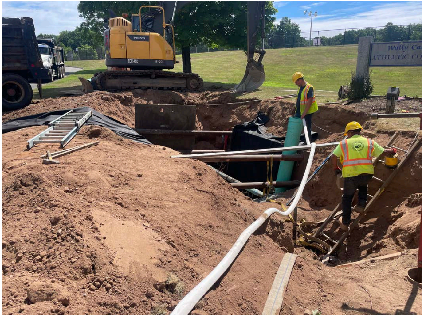
Picture 7: Ludlow in the process of pumping water from the bottom of the excavation at Station 525+75 into the catch basin located at Station 525+49.
