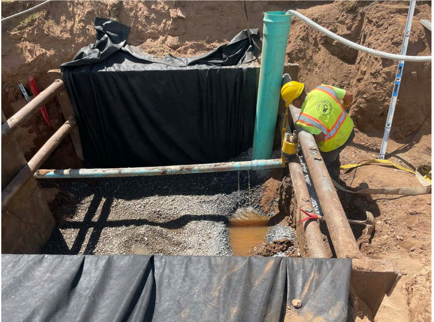
Picture 6: 4" PVC water line that Ludlow has cut on the bottom to drain the line. Ludlow is in the process of setting up a pump to move the water from the bottom of the excavation into the catch basin located at Station 525+49.
