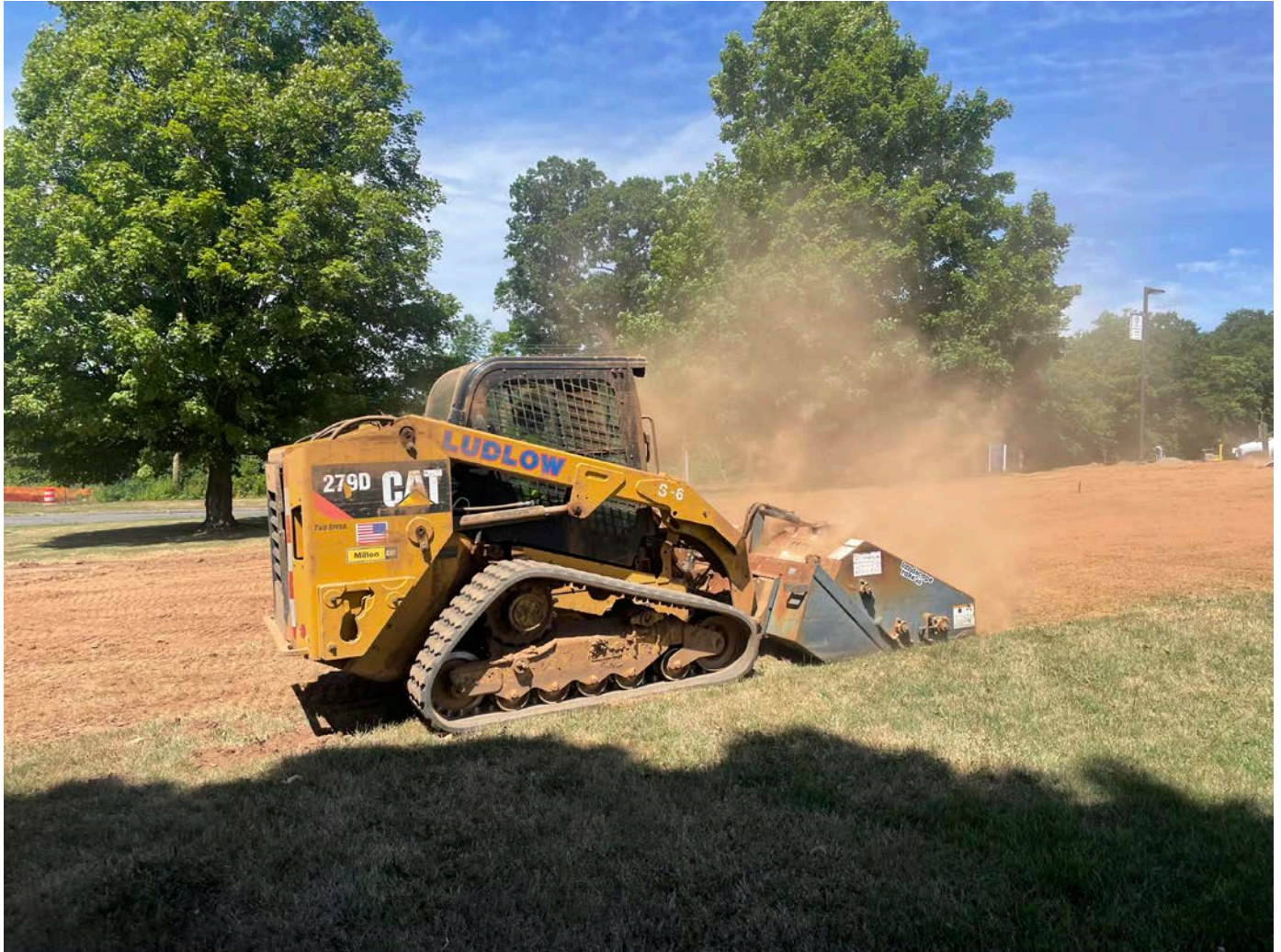
Picture 10: Ludlow is using a harley rake on a CAT 279D to grade the areas located between Pickett Lane and the access road located on the west side of the Coginchaug Regional High School that were disturbed during the installation of 4" and 8" DIP.
