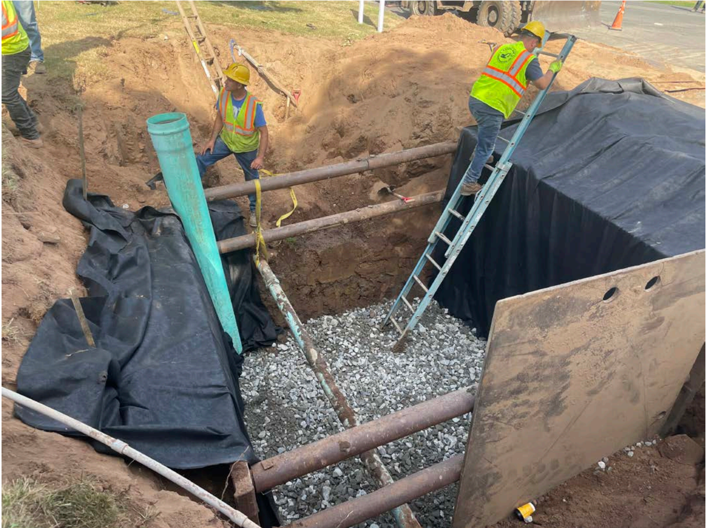
Picture 3: -2" rock that Ludlow has placed over black geofabric on the bottom of the excavation where Ludlow will be installing a vault at Station 525+75.
