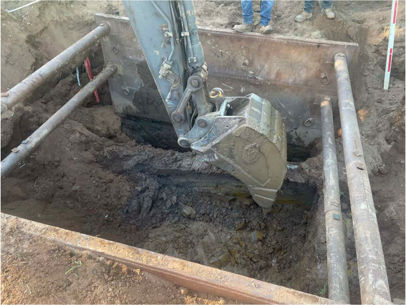
Picture 2: Ludlow excavating on the north side of a 4" water line that runs through the footprint of the vault they are installing at Station 525+75 on Pickett Lane, Durham. View to the south.
