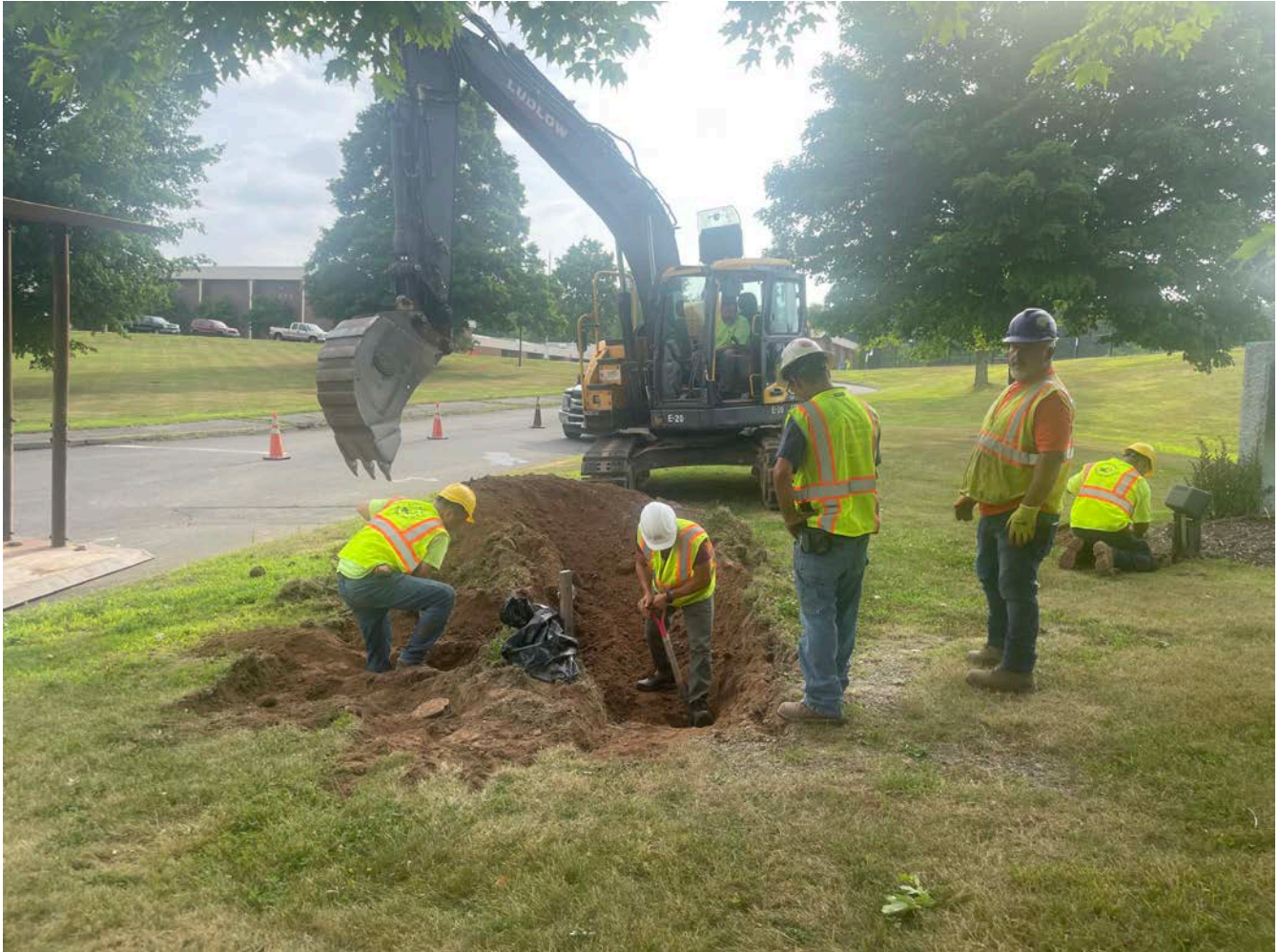
Picture 1: Ludlow using an excavator and hand tools to locate subsurface utilities located within the footprint of where they are working to install a vault at Station 525+75. View to the east.
