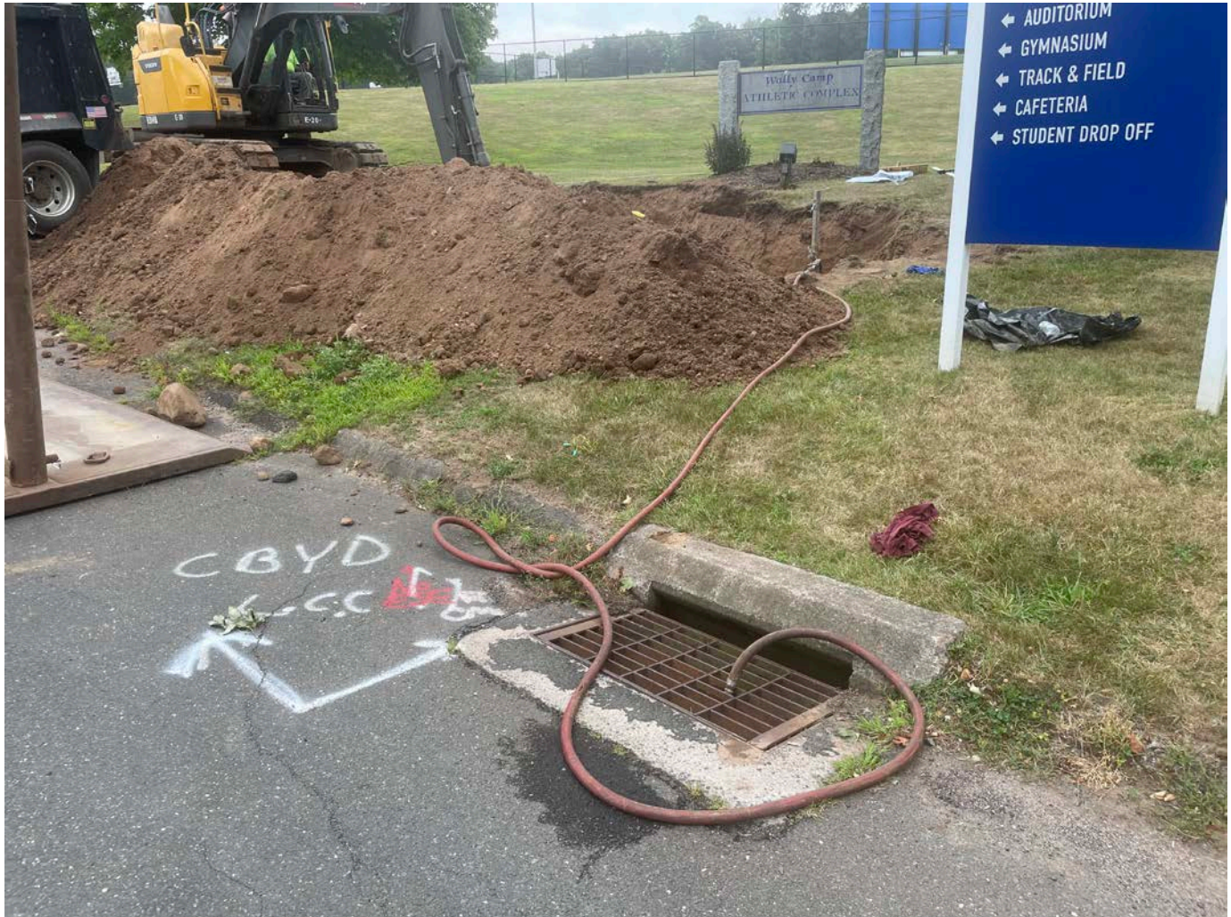
Picture 3: Ludlow draining the 50' of 4" DIP they previously installed at Station 525+75 through a 1" blowoff that they are directing to a catch basin located at Station ~525+49.
