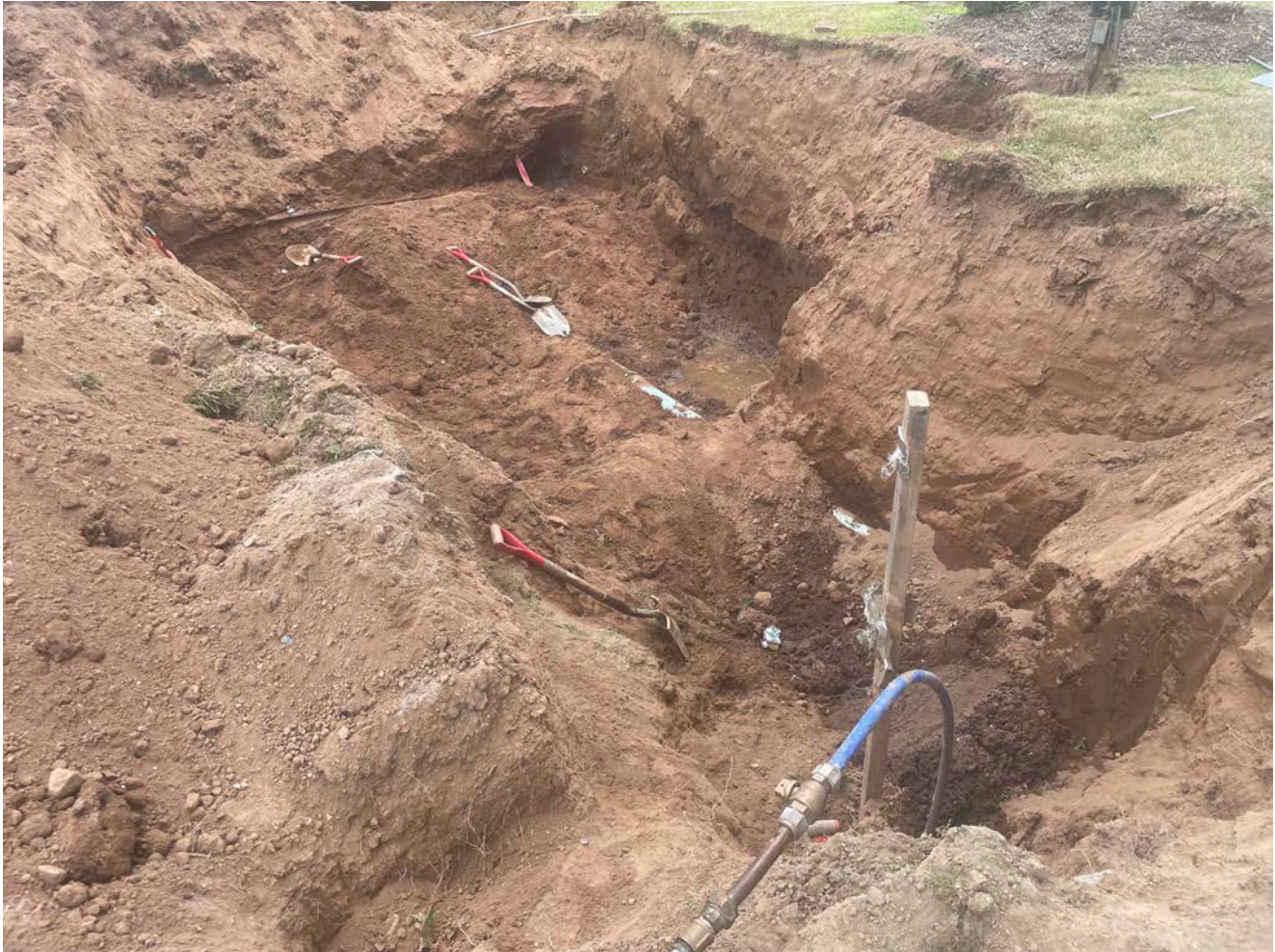
Picture 4: View of the excavation that Ludlow has made for the installation of a vault at Station 525+75. Note the 4" PVC water line that Ludlow has daylighted. View to the southeast.
