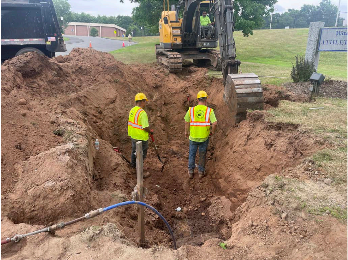
Picture 2: Ludlow excavating the footprint of the vault they are installing at Station 525+75 on Pickett Lane, Durham. View to the east.
