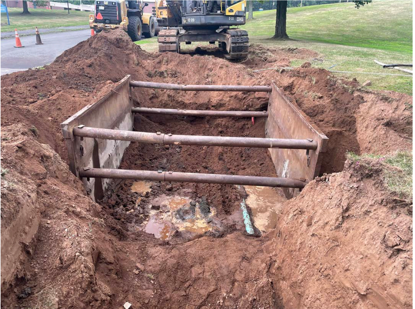
Picture 6: Trench box that Ludlow has set in the excavation they made for the installation of a vault at Station 525+75.
