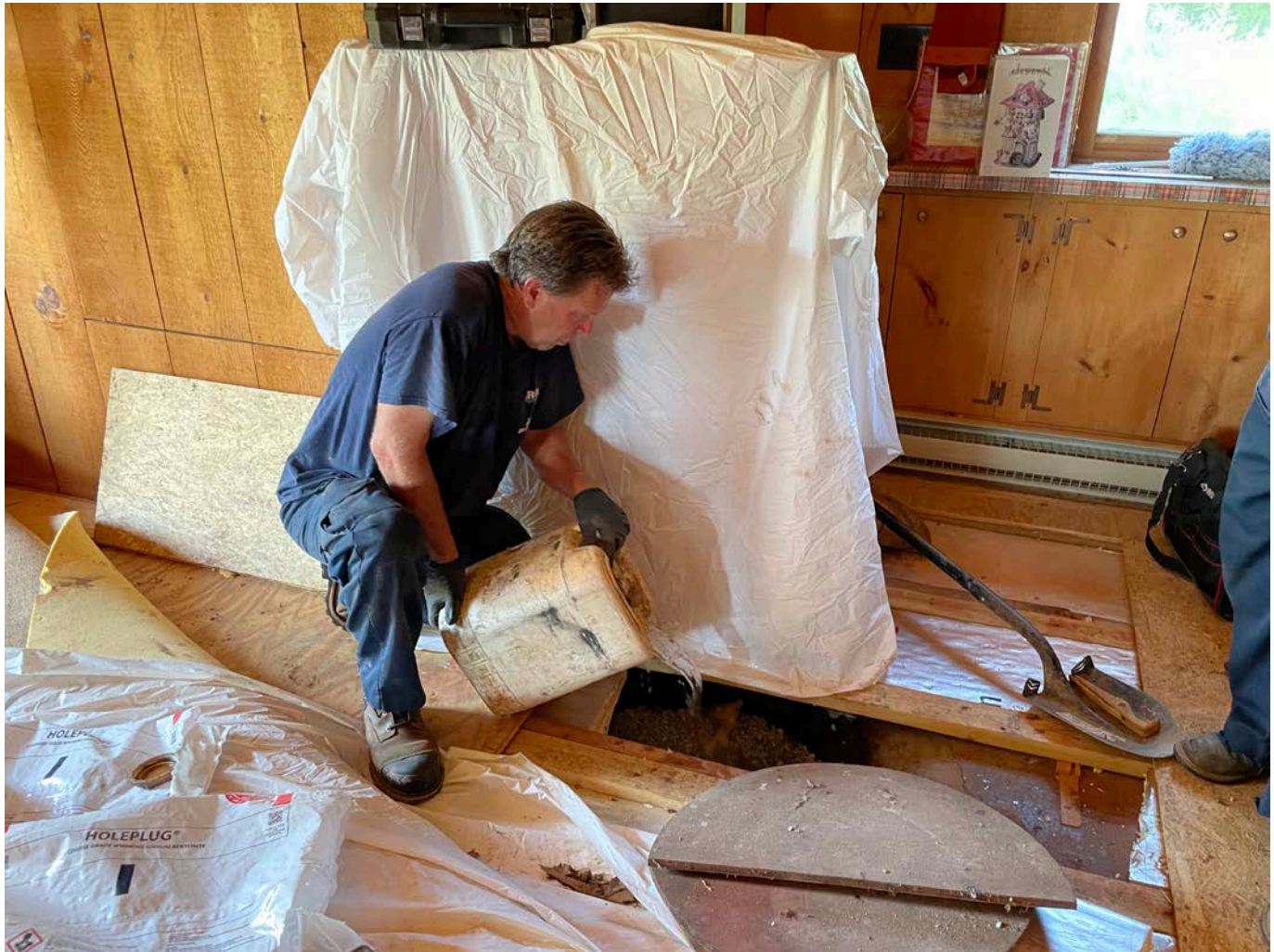
Picture 5: Grela hydrating the bentonite chips they placed the well tile located below the floor of the 289 Main Street residence as part of well decommissioning activities. View to the west.
