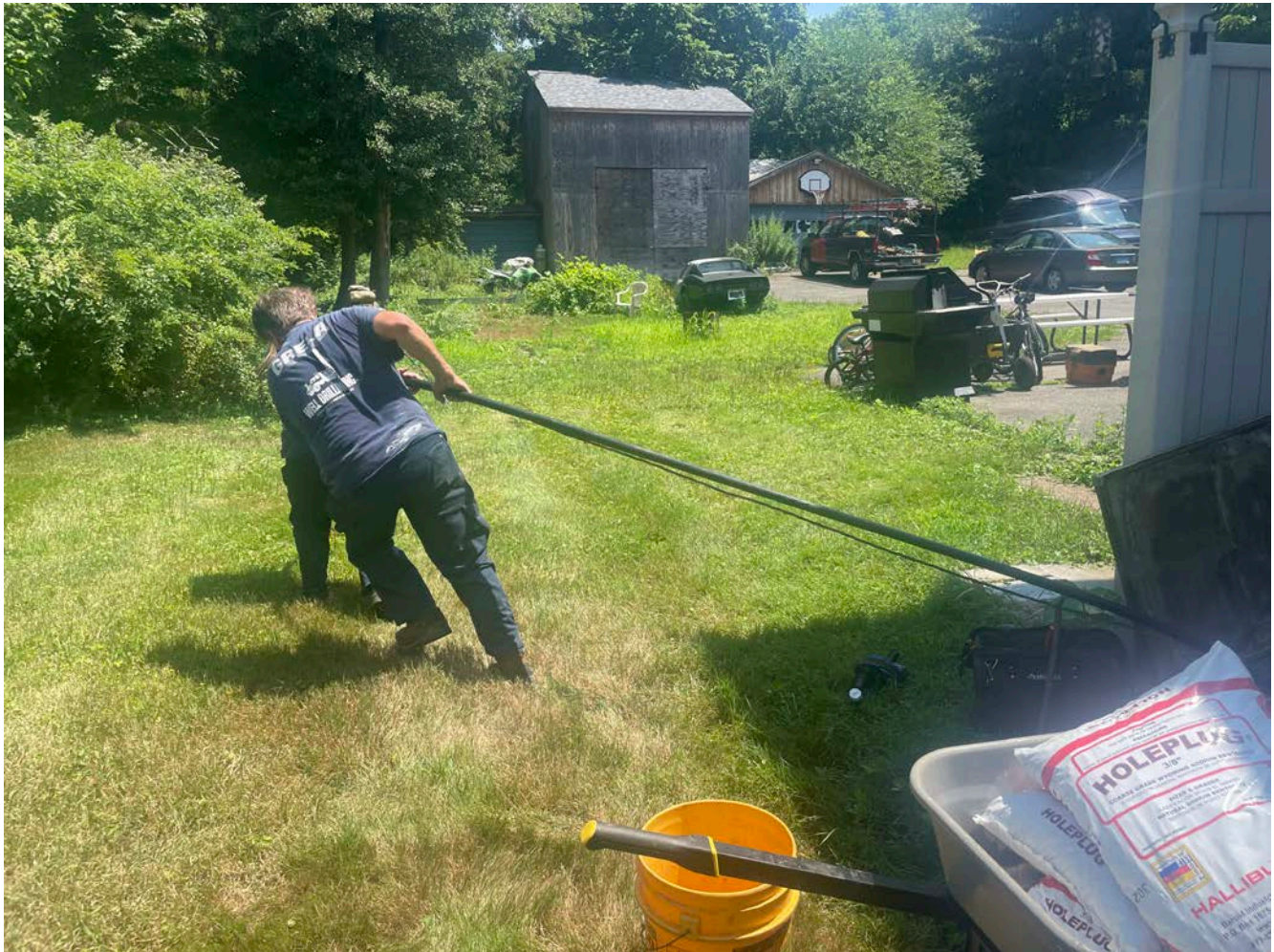
Picture 9: Grela pulling the well line and attached pump from the well located in the basement of the 173 Maple Avenue residence. View to the east.
