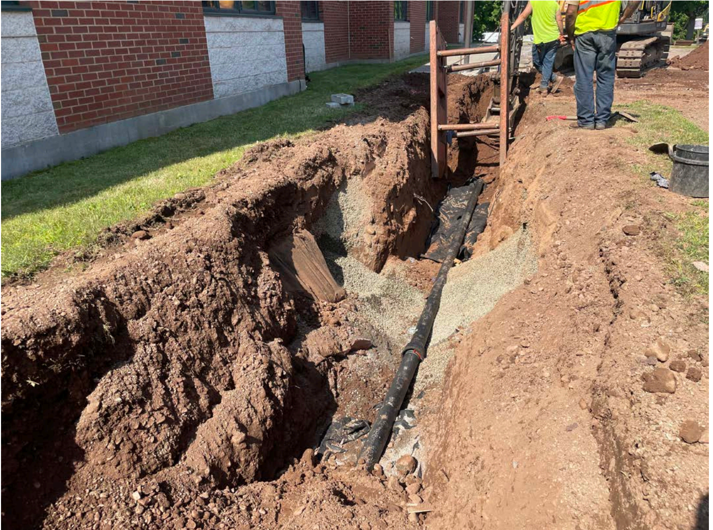
Picture 6: 4" DIP that Ludlow is in the process of installing on the north side of the high school. View to the west.
