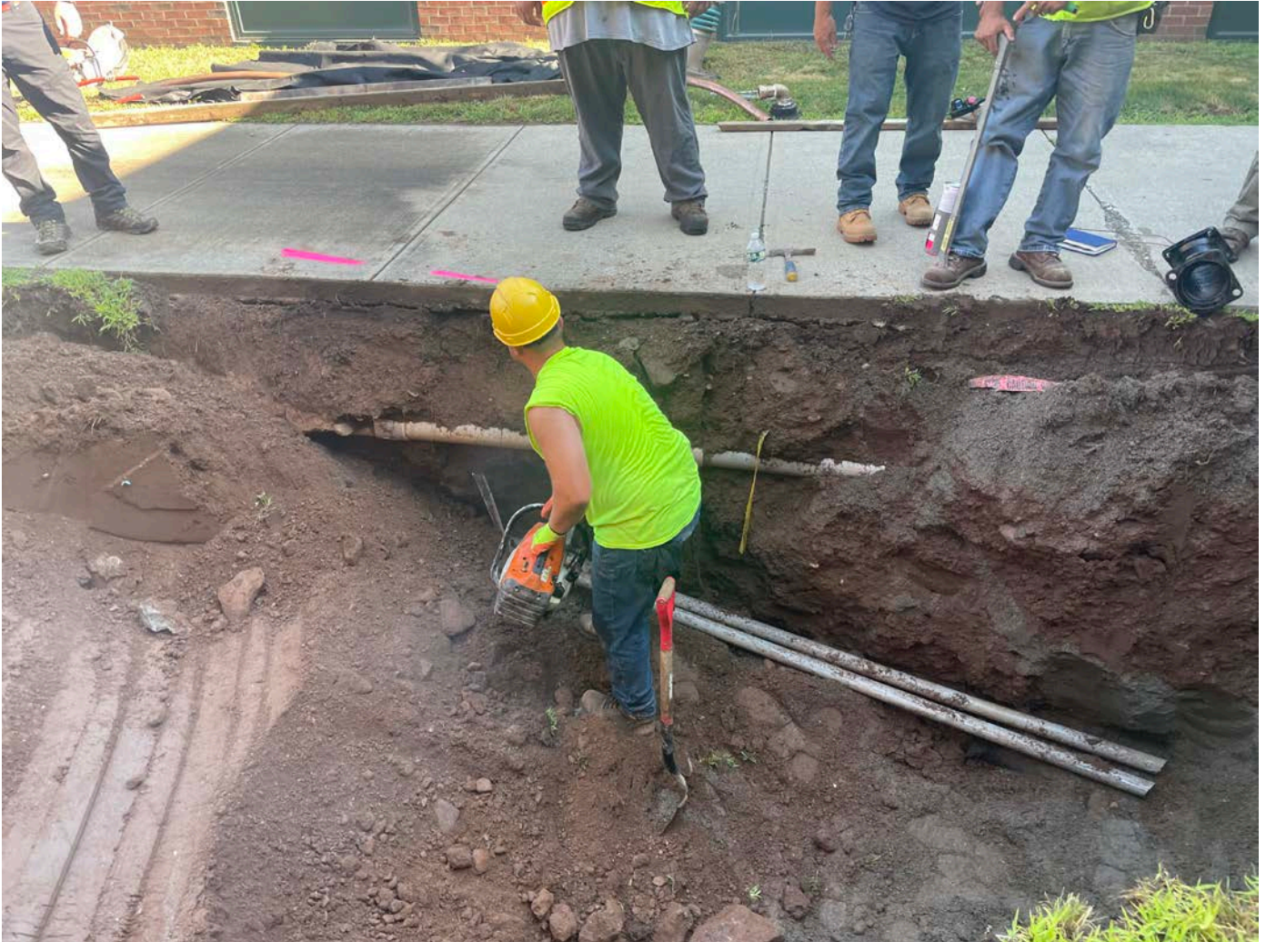
Picture 4: Ludlow using a cutoff saw to cut two sections of 2" PVC conduit at Station ~554+30. The PVC was already severed (right side of the photograph) when it was daylighted by Ludlow. View to the north.
