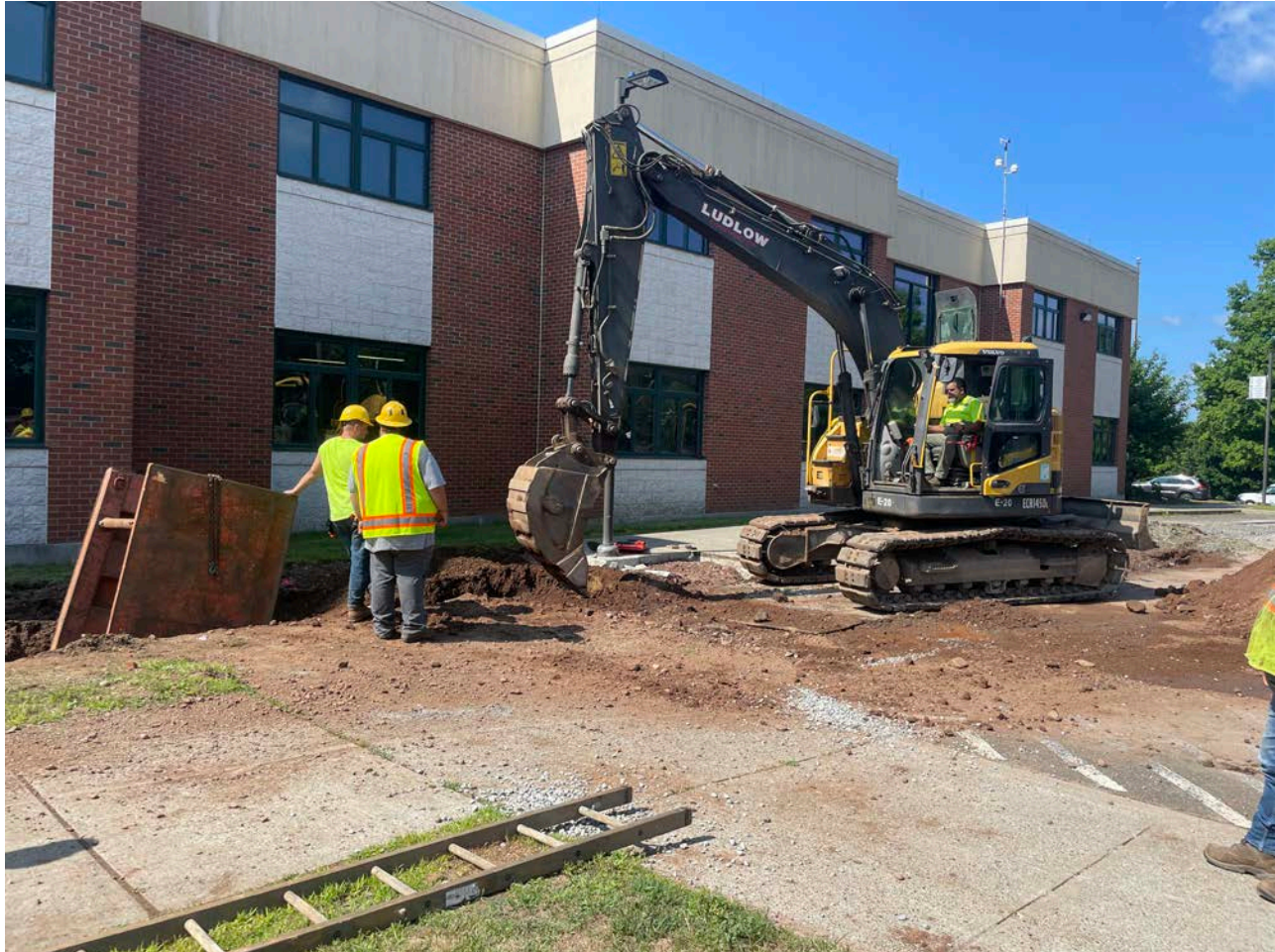
Picture 5: Ludlow excavating on the north side of the high school as they continue to install 4" DIP water line. View to the southwest.
