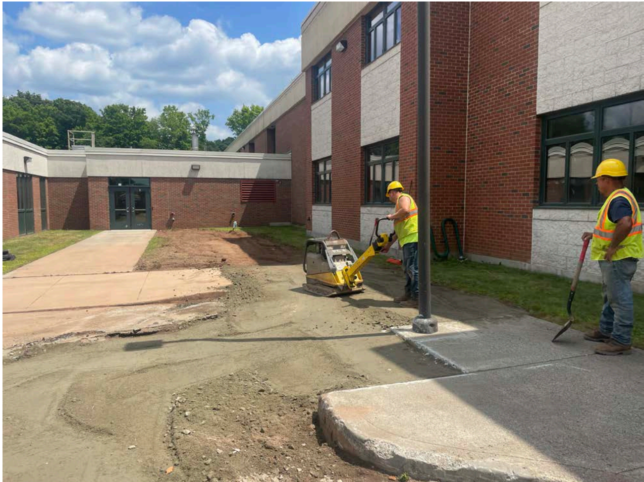
Picture 9: Ludlow using a plate compactor on backfill they placed when backfilling the trench they excavated on the north side of the high school when installing 4" DIP water line. View to the east.
