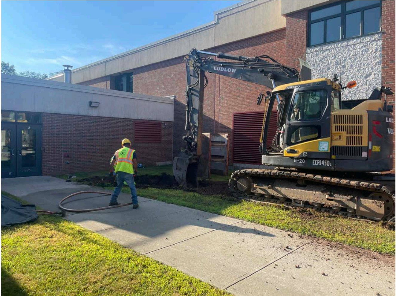
Picture 2: Ludlow excavating at Station ~554+30 as they continue to install 4" DIP on the north side of the Coginchaug Regional High School. View to the southeast.
