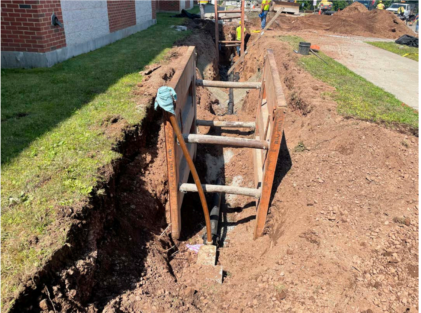
Picture 7: 2" copper blow-off line that Ludlow installed on the east end of the 4" DIP they installed in order to pressure test the line before they connect it to the high school. View to the west.
