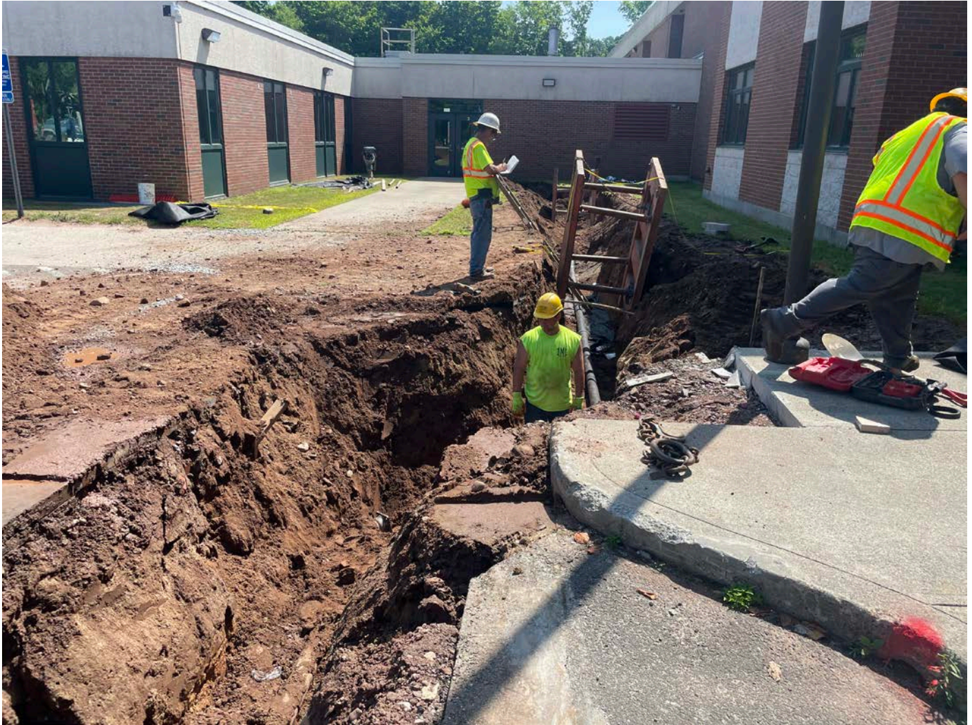
Picture 8: View of Ludlow installing 4" DIP on the north side of the high school. View to the east.
