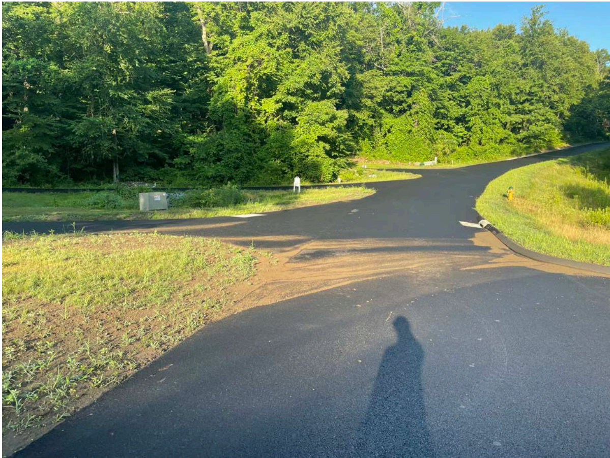
Picture 1: Shared Access Driveway in Middletown showing minor erosion after heavy rains yesterday. ~Station 14+25, view to the west.
