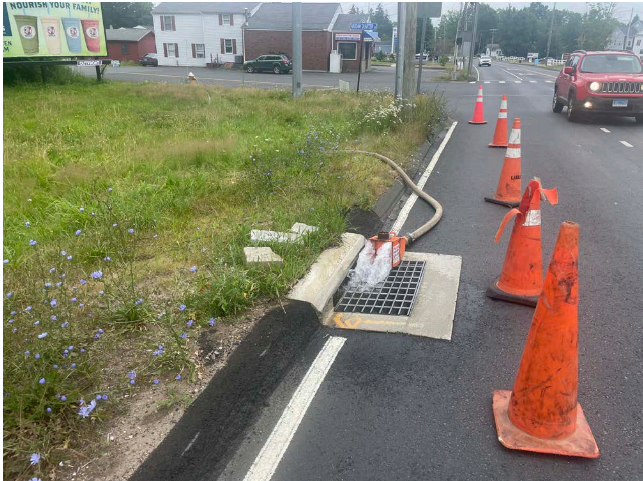
Picture 3: Ludlow discharging water into a catch basin located on the east side of Main Street that they are flushing from a hydrant located on Haddam Quarter Road. View to the south.
