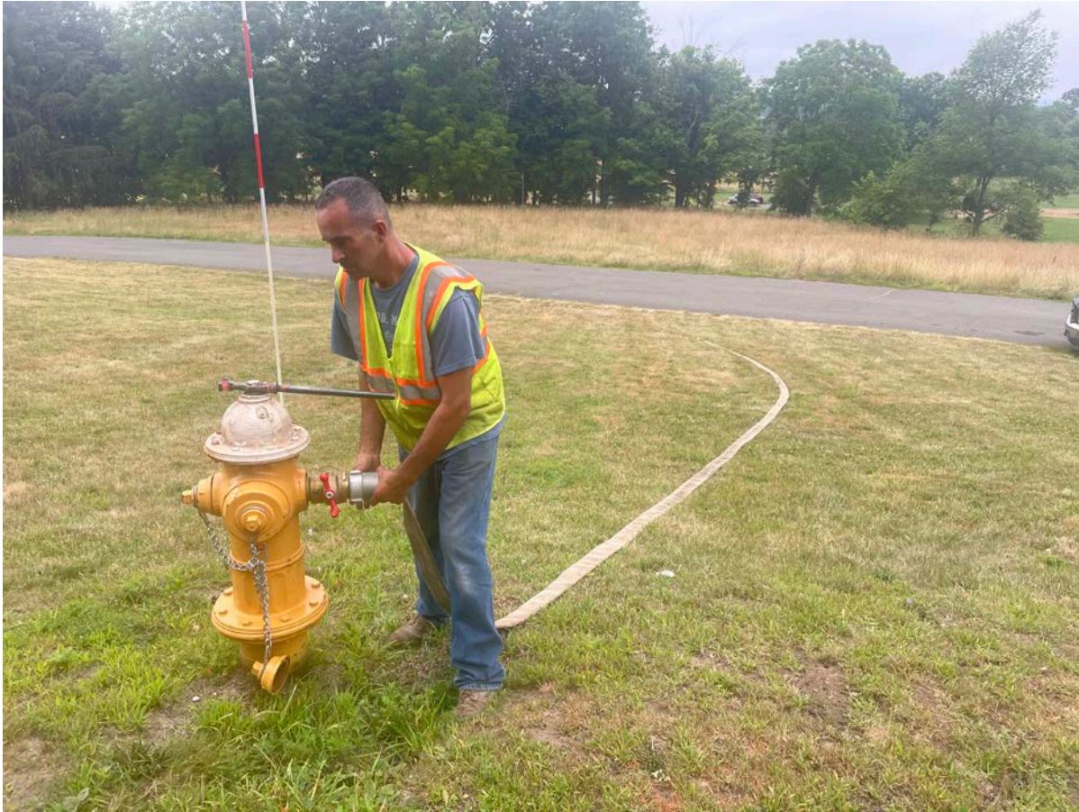
Picture 1: Ludlow setting up on a hydrant located at ~Station 900+00 to flush the water line on Maple Avenue. View to the west.
