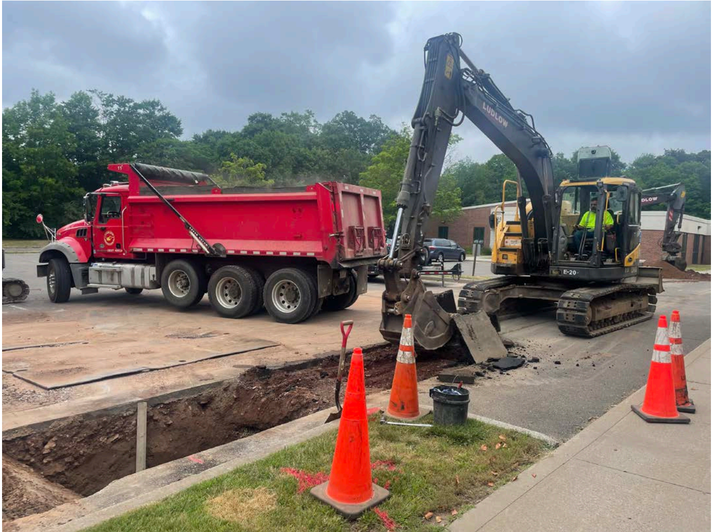
Picture 6: Ludlow removing pavement from the footprint of the trench they are excavating at Station 529+64 in the parking lot located on the north side of the CRHS for the installation of a 4" DIP water line. View to the northeast.
