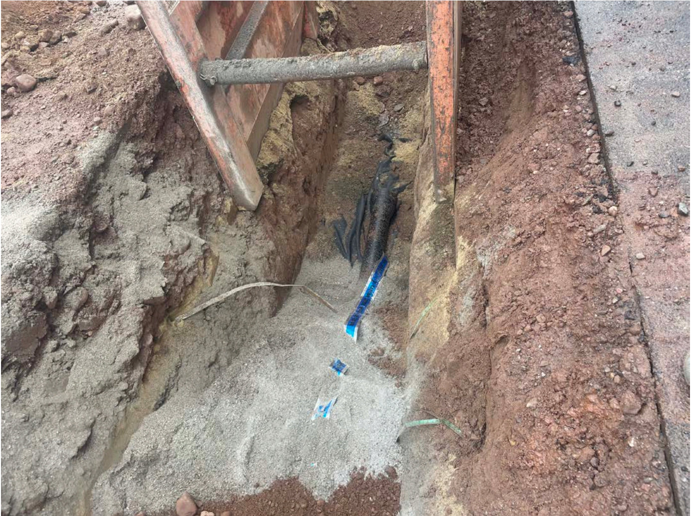
Picture 10: Sand and caution tape that Ludlow placed over 4" DIP that they installed on the north side of the CRHS at Station 529+64. View to the east.
