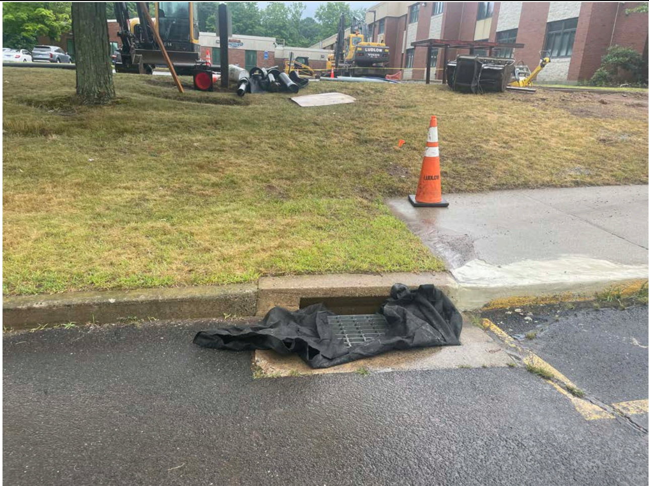
Picture 11: One of the catch basins located near the work zone next to the Coginchaug Regional High School that Ludlow lined with filter fabric to keep solids from entering the catch basin. View to the southwest.
