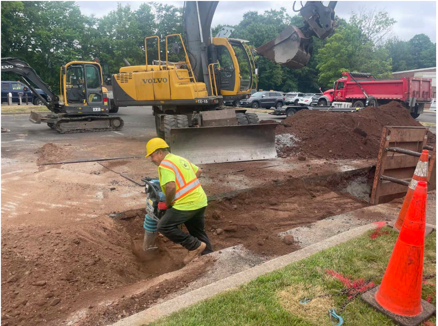
Picture 8: Ludlow using a jumping jack to compact the backfill they have placed over a section of 4" DIP they just installed at Station 529+64. View to the northeast.
