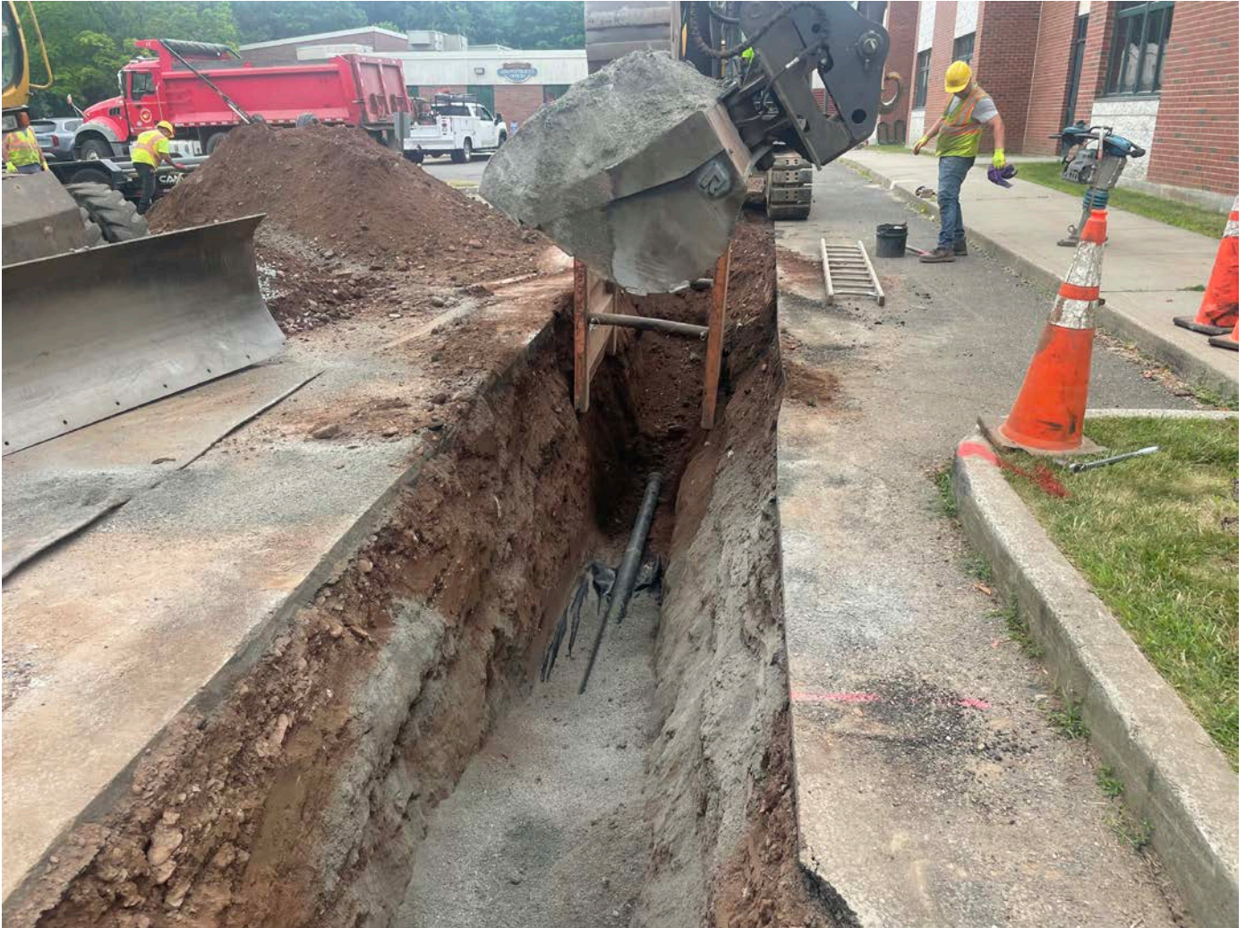
Picture 7: Ludlow about to place sand over a section of 4" DIP in the trench they excavated across the parking lot located on the north side of the Coginchaug Regional High School. View to the east.
