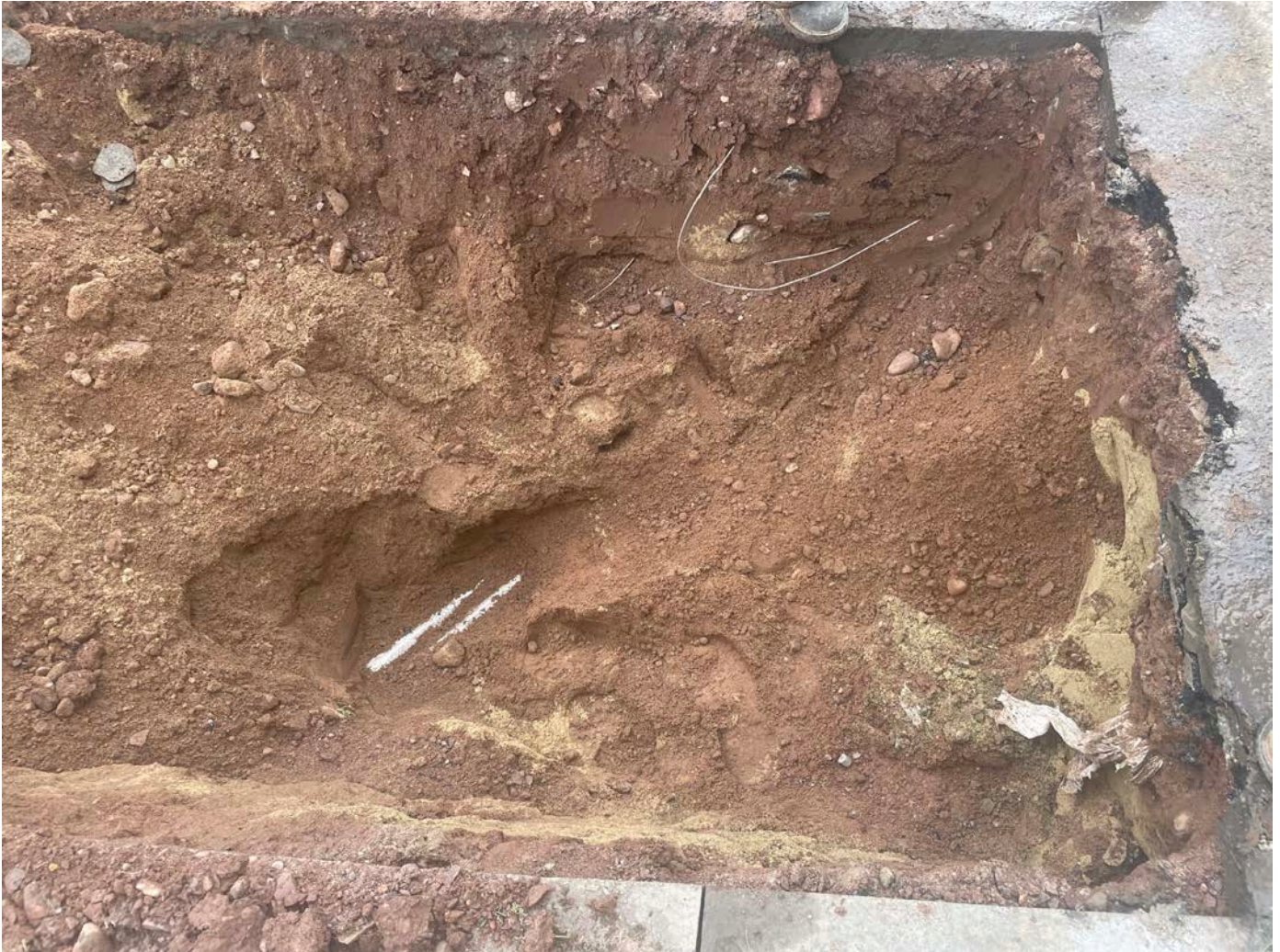
Picture 4: PVC conduits that Ludlow daylighted on the north side of the Coginchaug Regional High School while installing 4" at Station 529+64. The severed wire at the top right of the photo is believed to be an inactive line.
