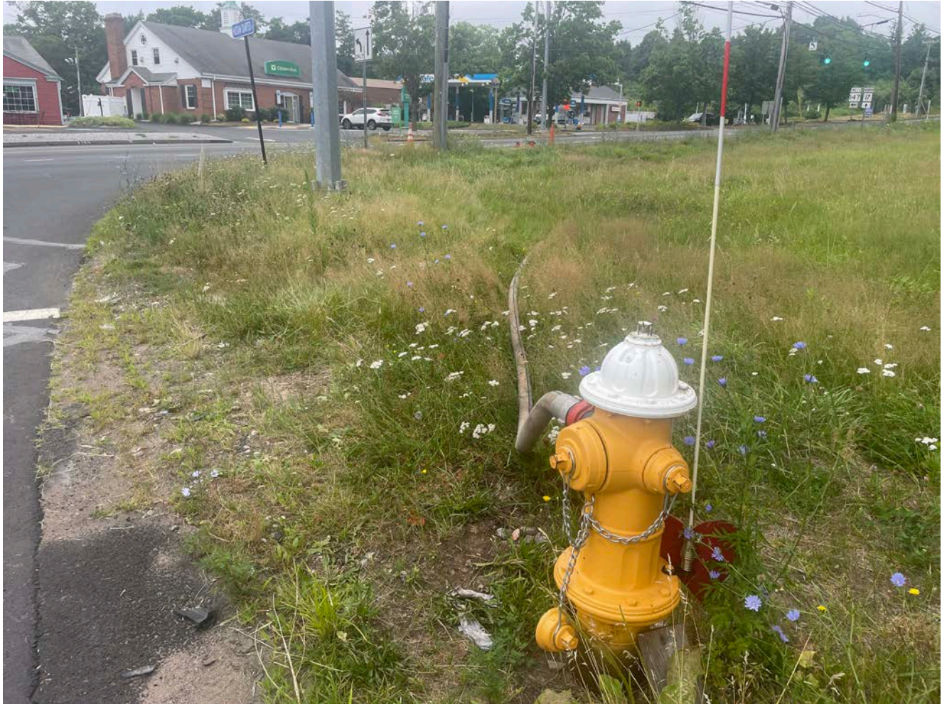
Picture 2: Ludlow set up on a hydrant located on Haddam Quarter Road next to where it intersects with Main Street to flush the water line on Main Street. View to the northwest.
