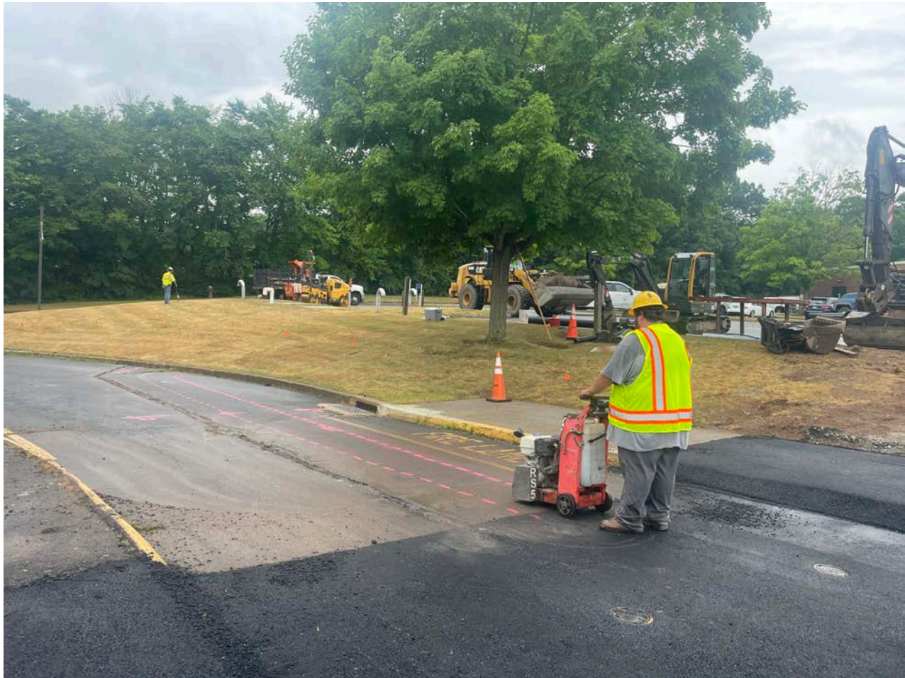
Picture 9: Ludlow saw-cutting on the northbound lane of the access road located on the west side of the CRHS as they prepare to install 8" DIP that will connect to the vault located further north. View to the north.
