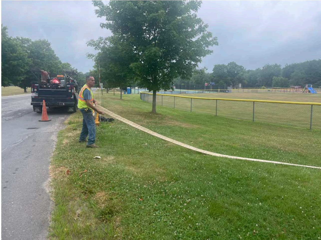
Picture 5: Ludlow setting up on a hydrant located at ~Station 525+00 to flush the water line on Pickett Lane, Durham. View to the west.
