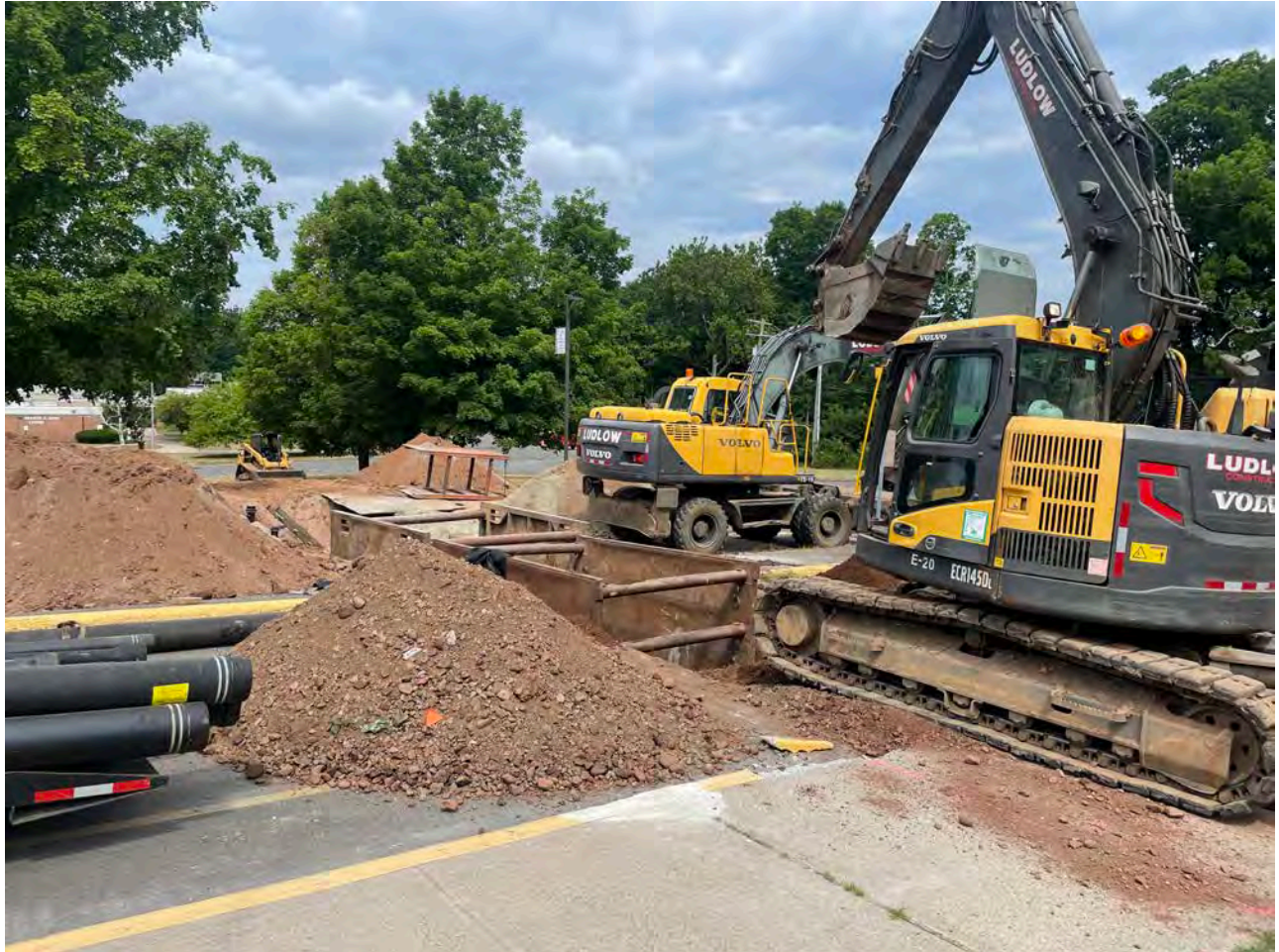
Picture 5: Ludlow excavating across the northbound lane of the access road located on the west side of the CRHS as they continue to install 4" and 8" DIP. View to the northwest.
