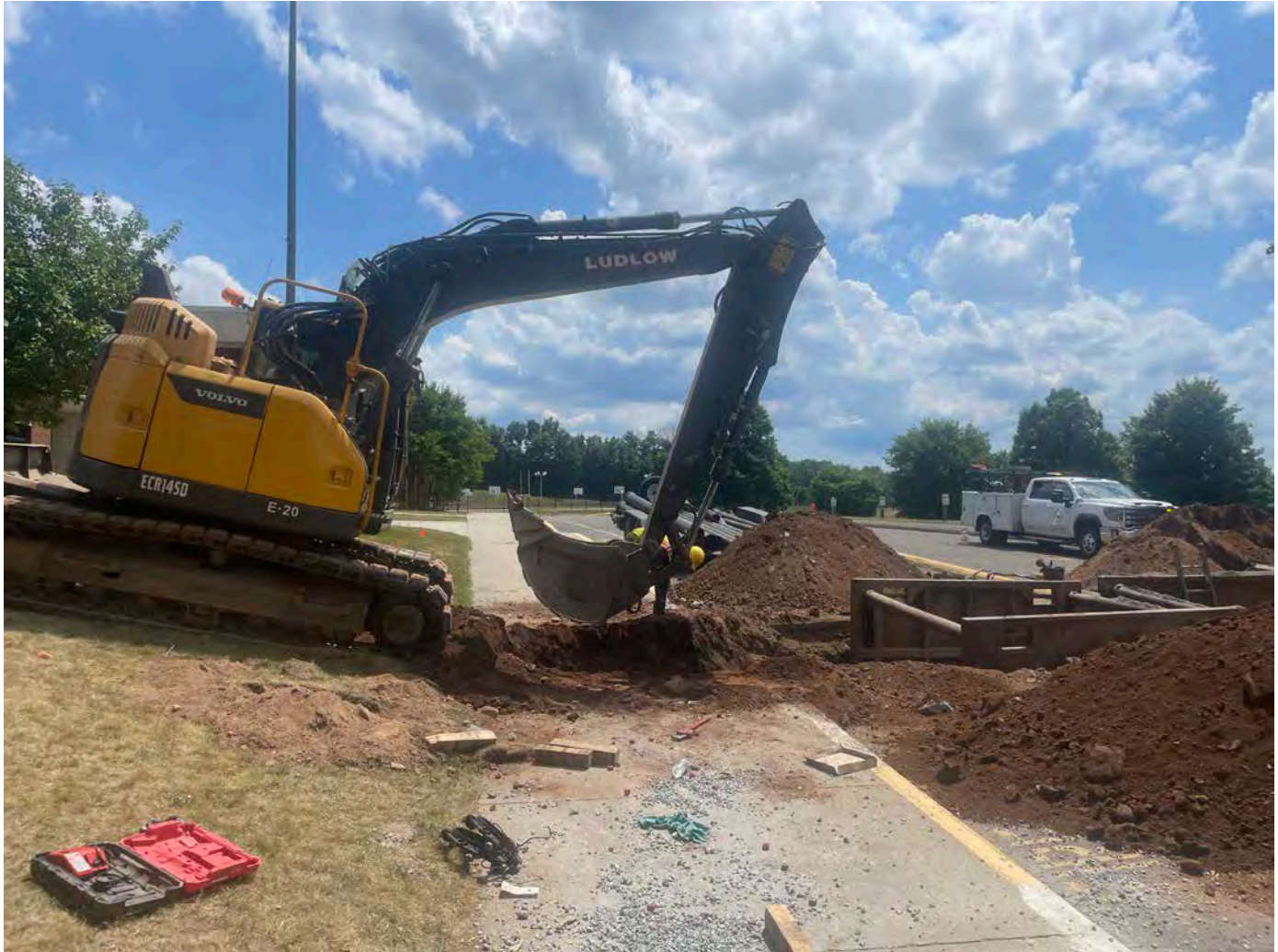
Picture 7: Ludlow excavating a trench across the sidewalk located on the west side of the CRHS as they continue to install 4" and 8" DIP. View to the south.
