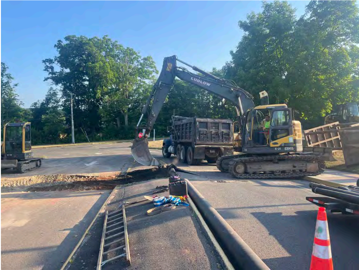
Picture 1: Ludlow removing asphalt from the median strip located on the west side of the CRHS as they continue to install 4" and 8" DIP. View to the north.
