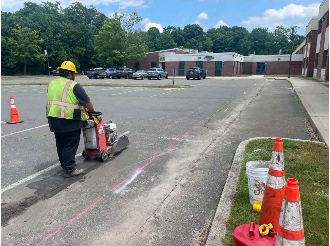
Picture 6: Ludlow saw-cutting the footprint of a trench on the pavement of the parking lot located on the north side of the CRHS. View to the east.
