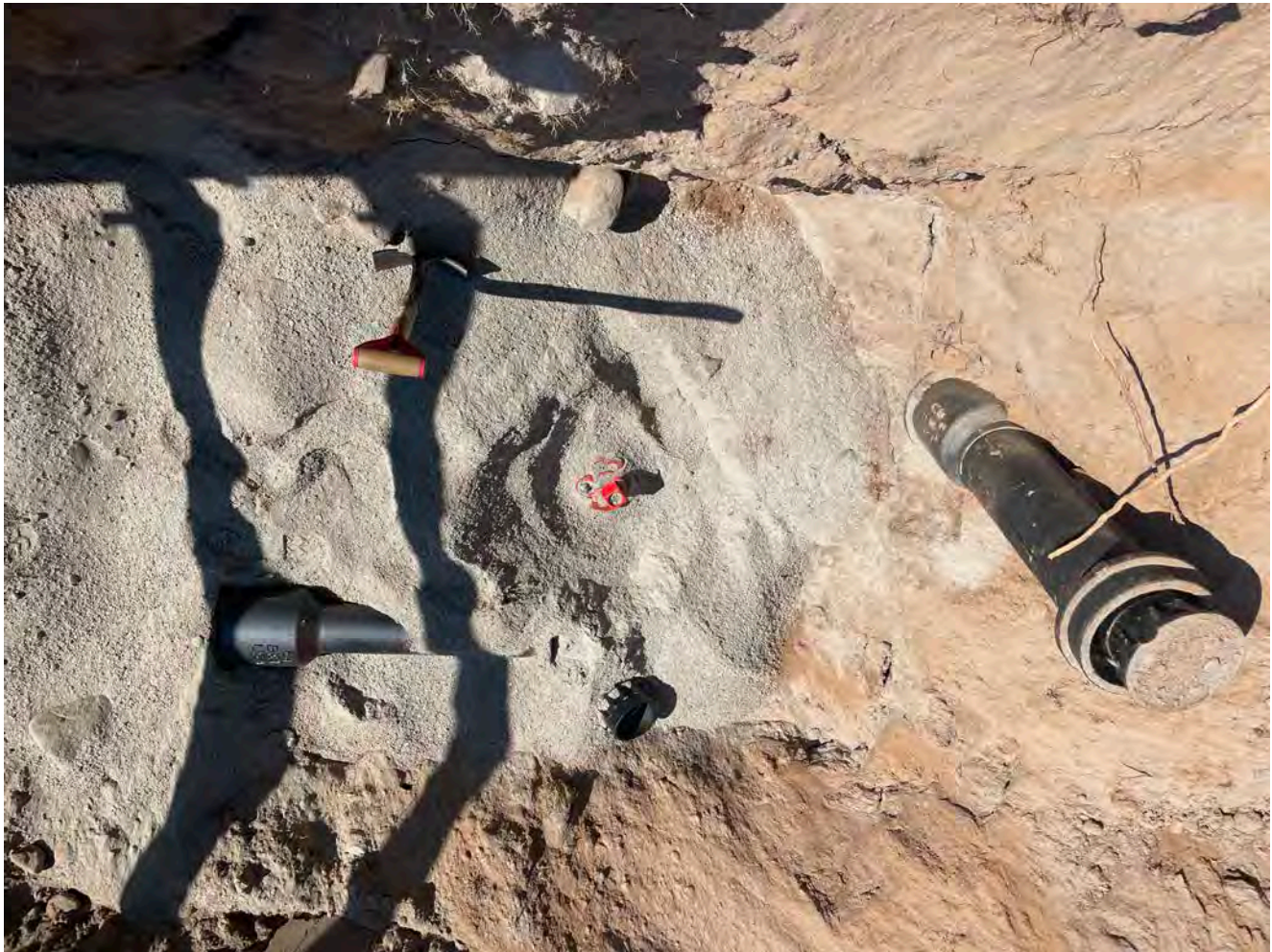
Picture 2: 8" Gate valve that Ludlow installed at Station 551+78 (the red top of the valve is visible in the center of the photograph).
