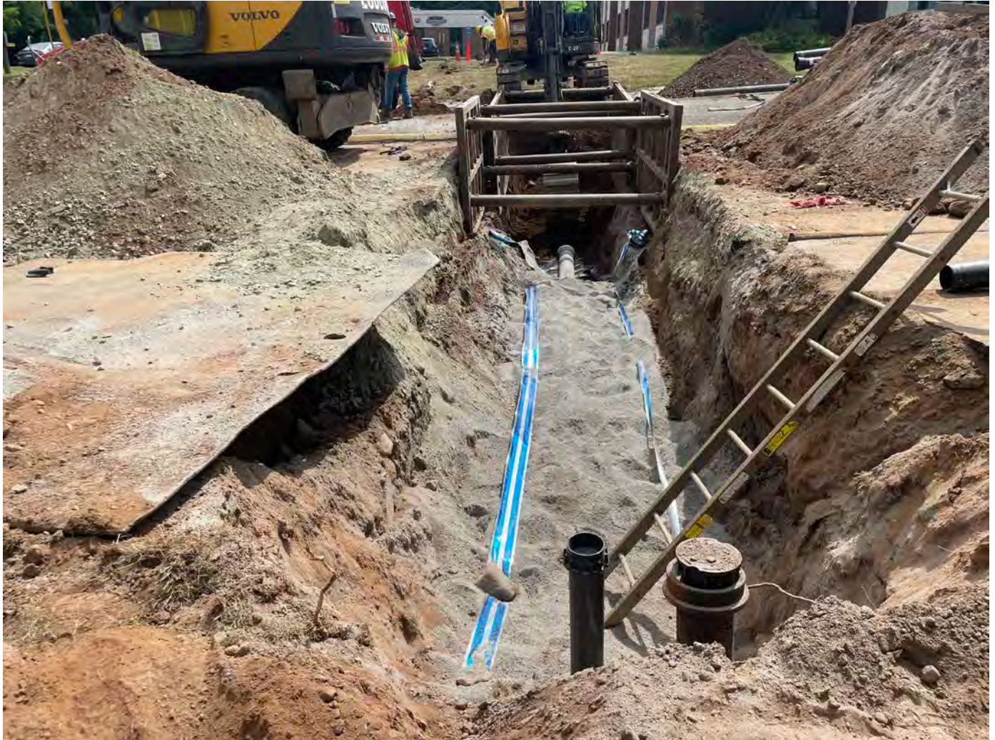
Picture 4: Sand and caution tape that Ludlow placed over 4" and 8" DIP that they installed at Stations 529+64 and 529+56, respectively. View to the east.
