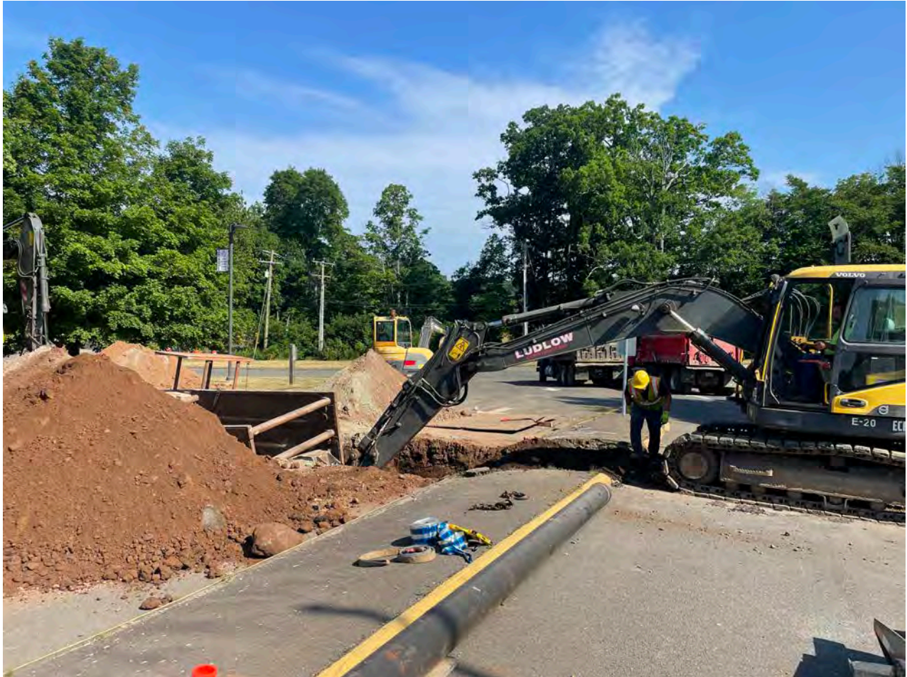
Picture 3: Ludlow excavating a trench across the southbound lane of the access road located on the west side of the CRHS as they continue to install 4" and 8" DIP. View to the north.
