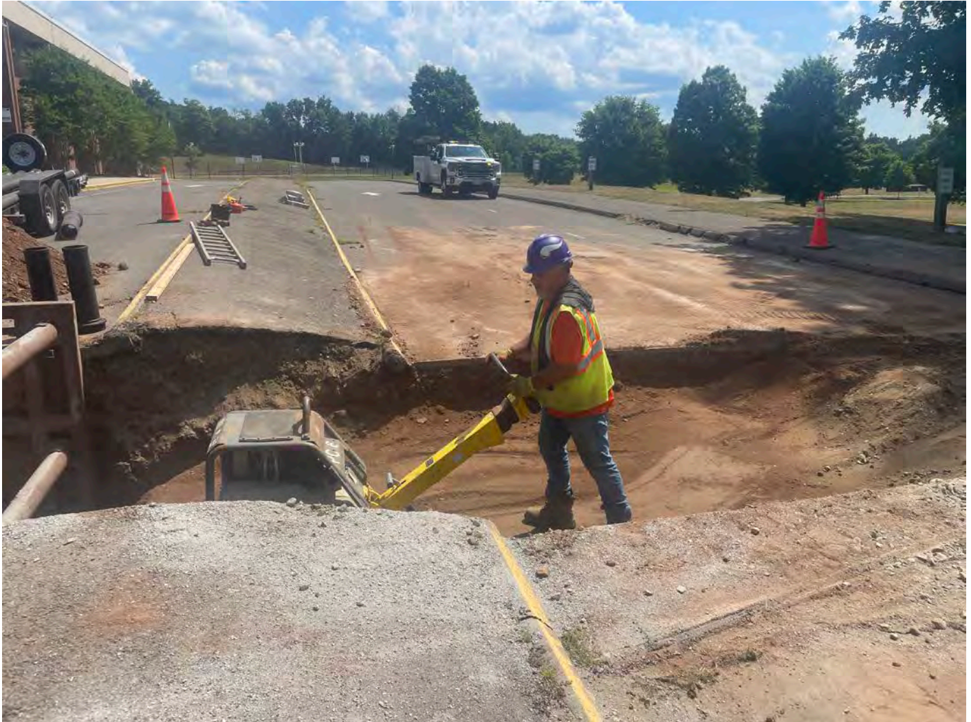
Picture 8: Ludlow using a plate compactor on the backfill they have placed over the 4" and 8" DIP they installed today at Stations 529+56 and 529+64. View to the south.
