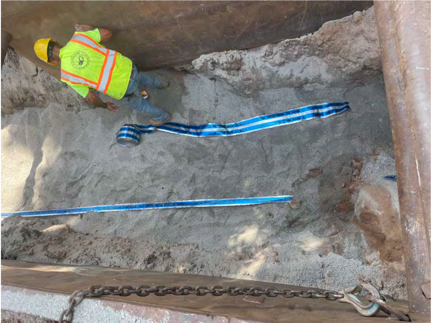
Picture 9: Caution tape that Ludlow is placing over the sand they put over the 4" and 8" DIP located at Stations 529+56 and 529+64. View to the south.
