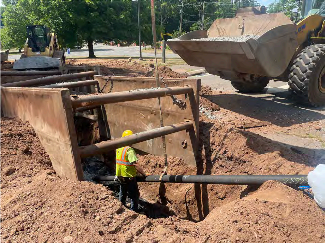
Picture 10: Ludlow in the process of installing a 20' section of 4" DIP at Station 529+64. View to the northwest.
