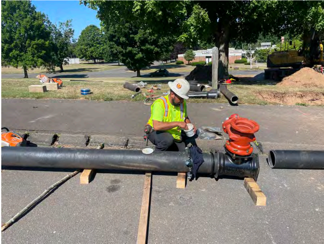
Picture 3: Ludlow working on attaching a section of 8" DIP to an 8"x8"x6" TEE (to which a 6" gate valve has already been attached). View to the west.
