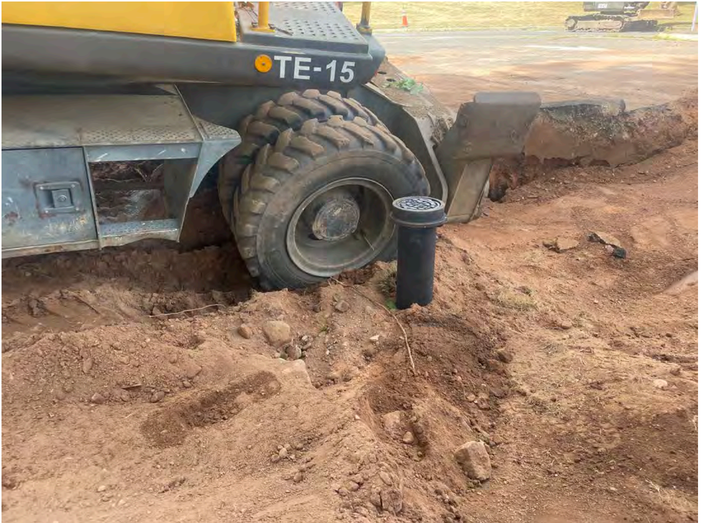
Picture 11: Road box that was placed over the valve stem of the 6" gate valve that Ludlow installed at Station 551+73.
