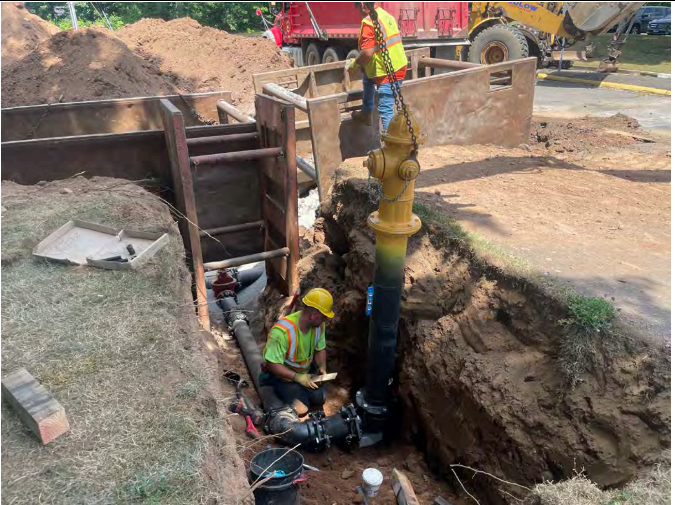
Picture 7: Hydrant that Ludlow just installed Station 551+94. View to the northeast.
