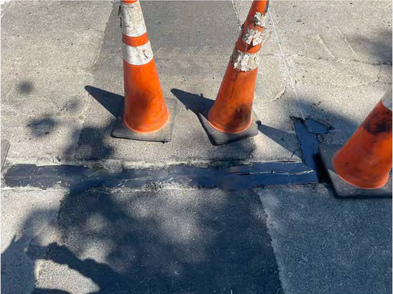
Picture 2: Break in a traffic loop at the intersection of Pickett Lane and Main Street that Ludlow's contractor KTM Electrical Contractors repaired and covered with black sealant.
