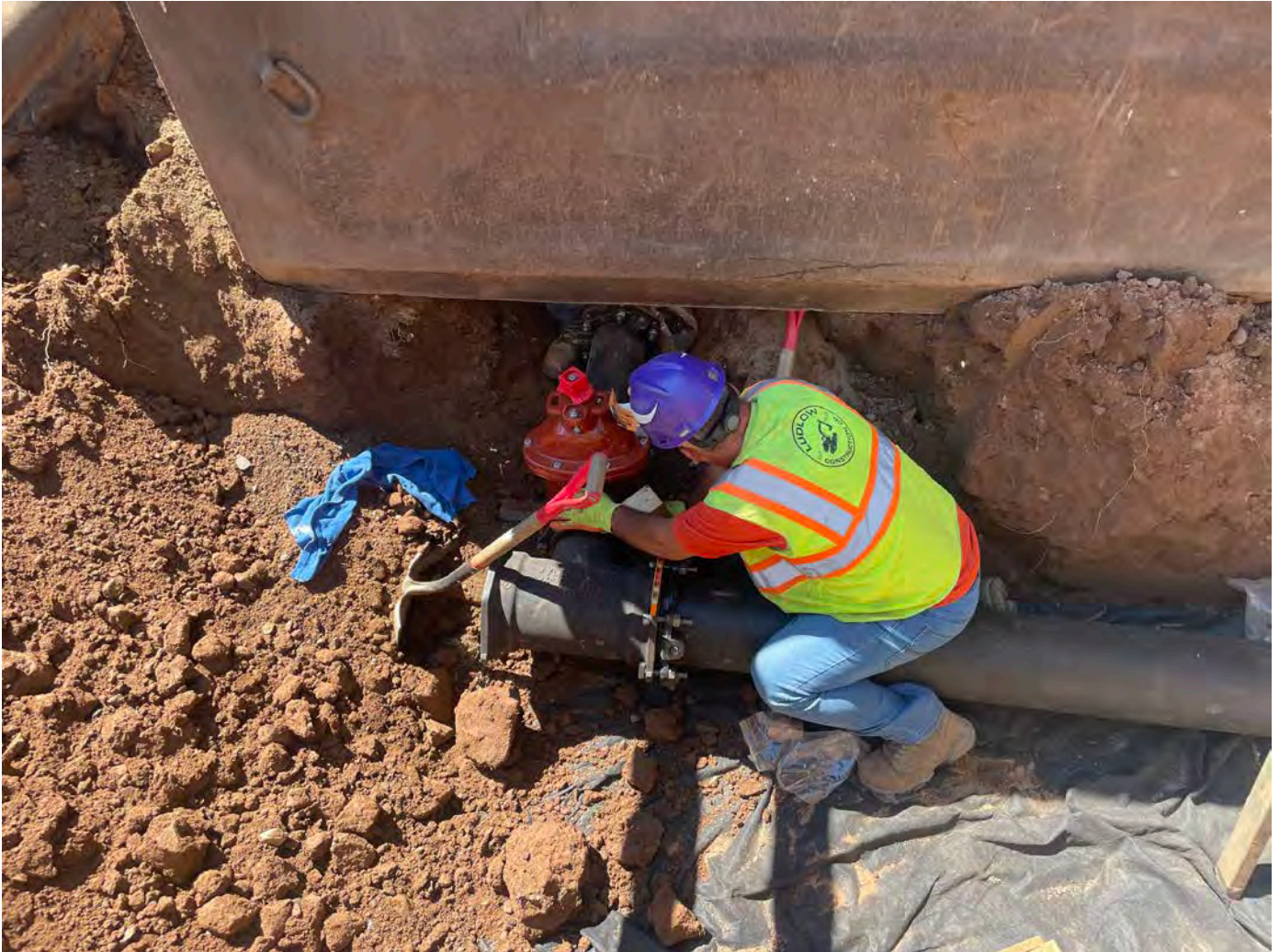
Picture 4: Ludlow installing a 6" gate valve at Station 551+73. View to the south.
