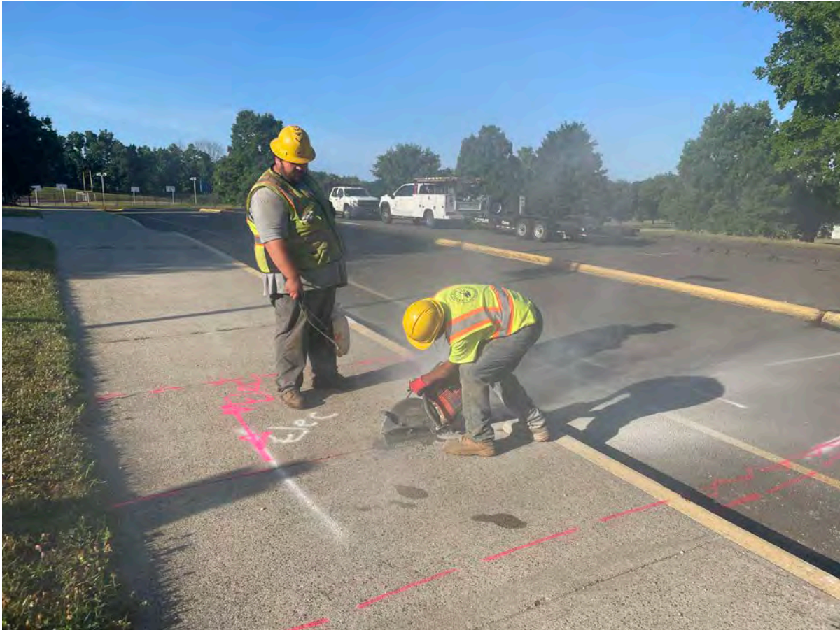
Picture 1: Ludlow saw cutting a sidewalk at the Coginchaug Regional High School at Station 529+64 as they continue to install 4" and 8" DIP. View to the southwest.
