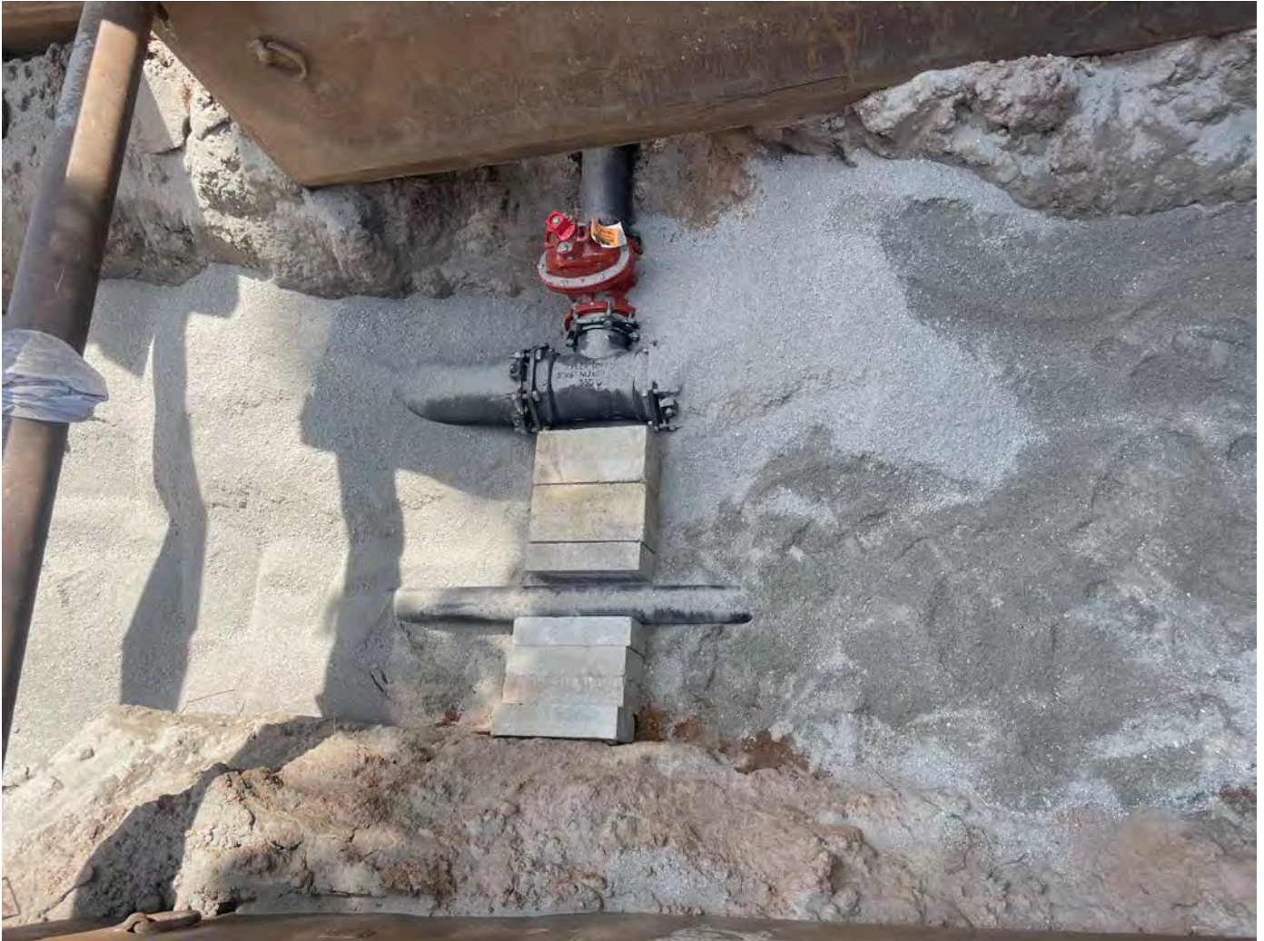
Picture 8: Thrust blocks that Ludlow installed on the north side of the 8"x8"x6" DIP TEE at ~Station 551+73. View to the southeast.
