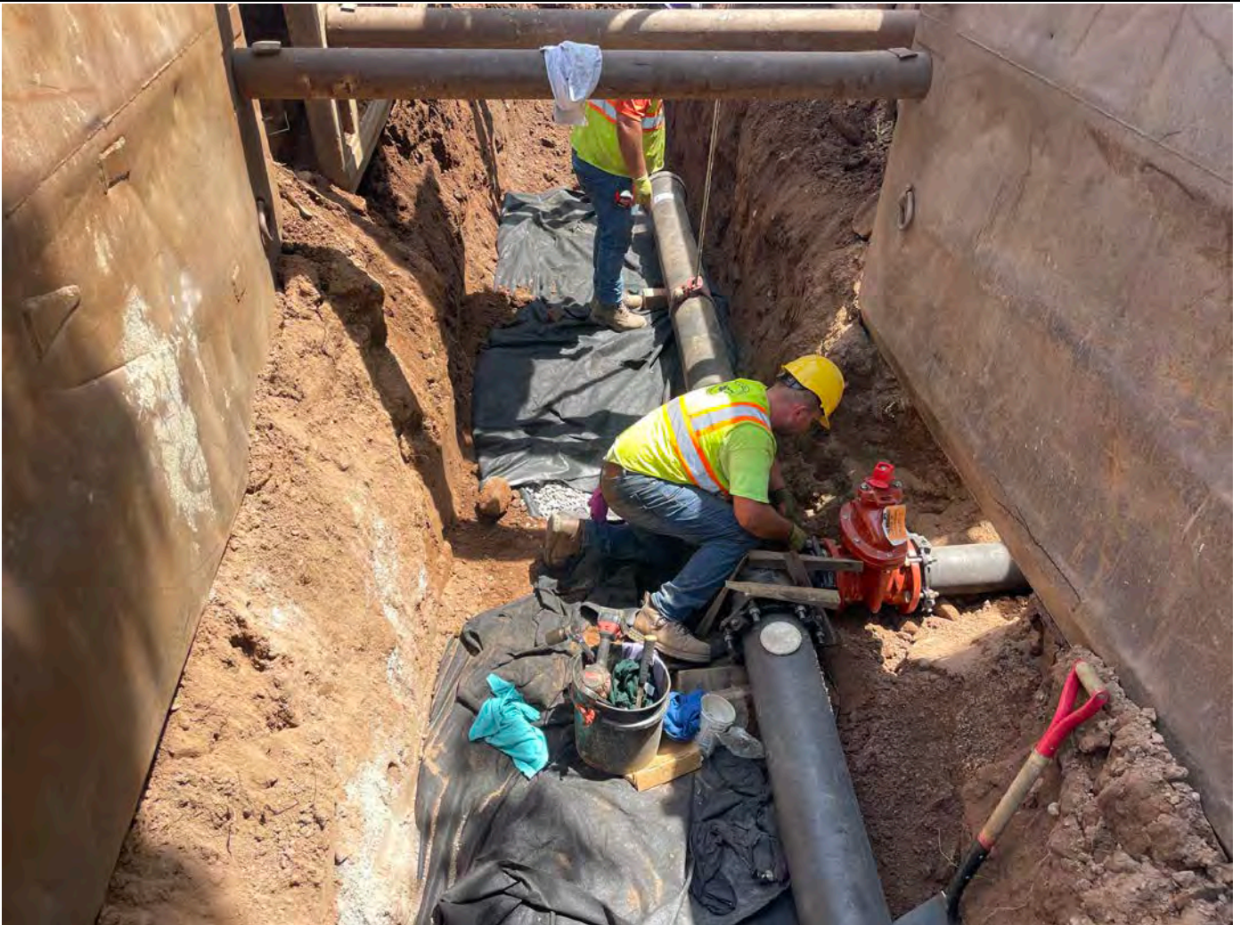
Picture 6: Ludlow connecting a section of 8" DIP to the east side of an 8"x8"x6" DIP TEE at ~Station 551+73.
