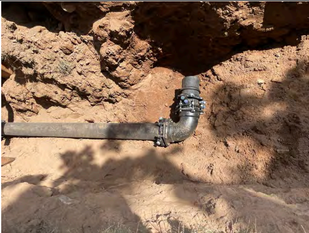
Picture 5: 6" DIP that Ludlow is installing for the placement of a hydrant at Station 551+94. View to the east.
