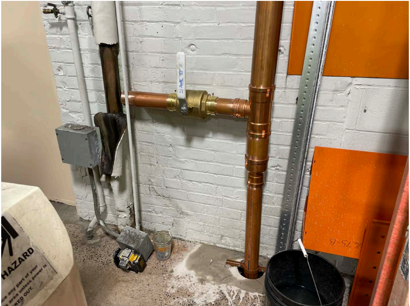
Picture 7: 4" copper pipe that West State Mechanical installed on the north side of the Durham Manufacturing facility.
