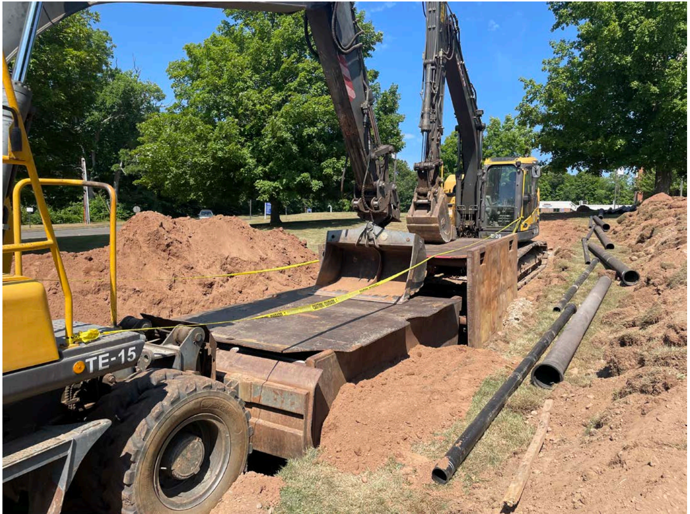
Picture 9: The excavation that Ludlow made at Station 529+64 at the end of the day after they secured the work zone with their equipment and steel plate on top of the trench boxes. View to the northeast.
