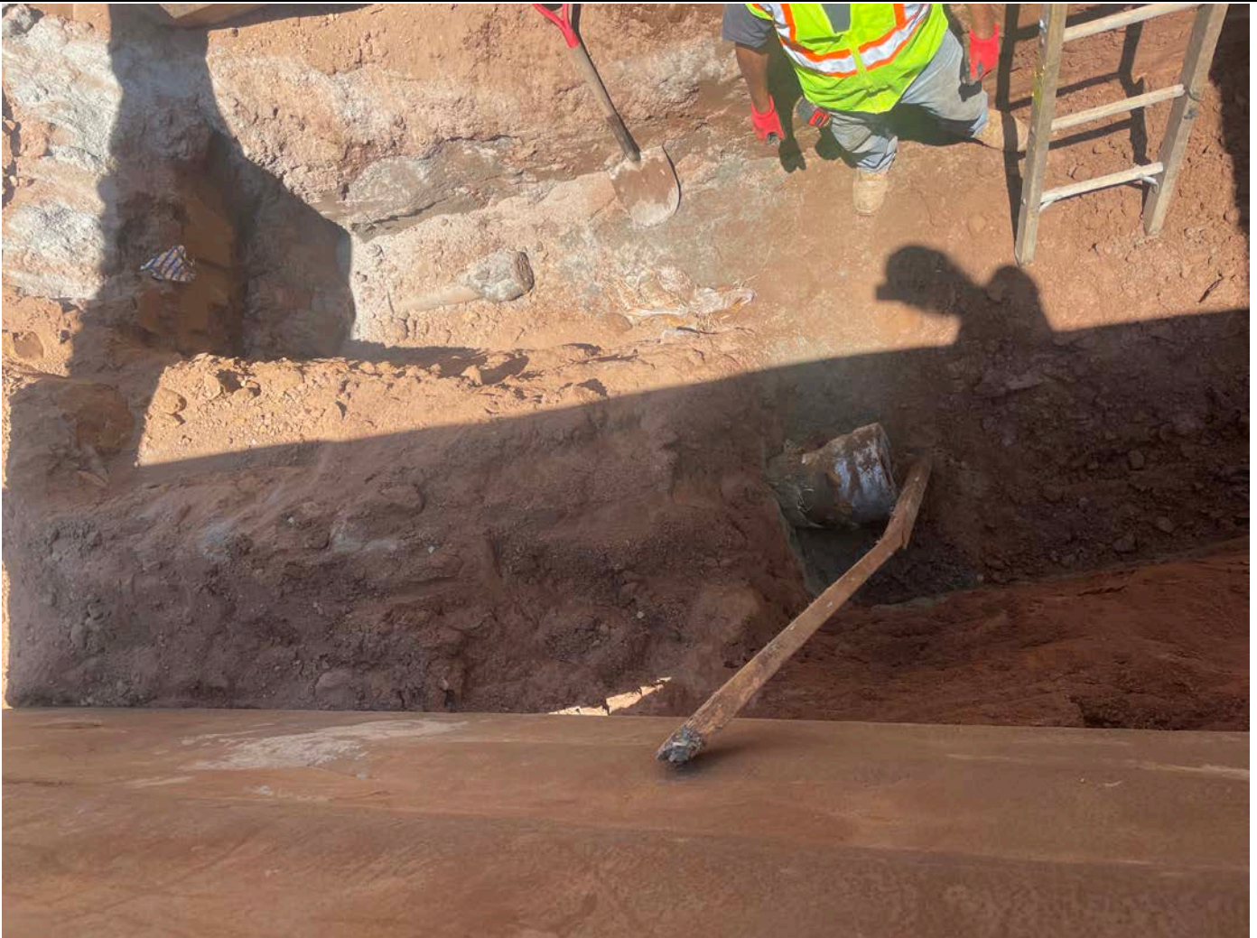
Picture 5: The east ends of 4" and 8" DIP that Ludlow previously installed at Station 529+64 on Pickett Lane. View to the north.
