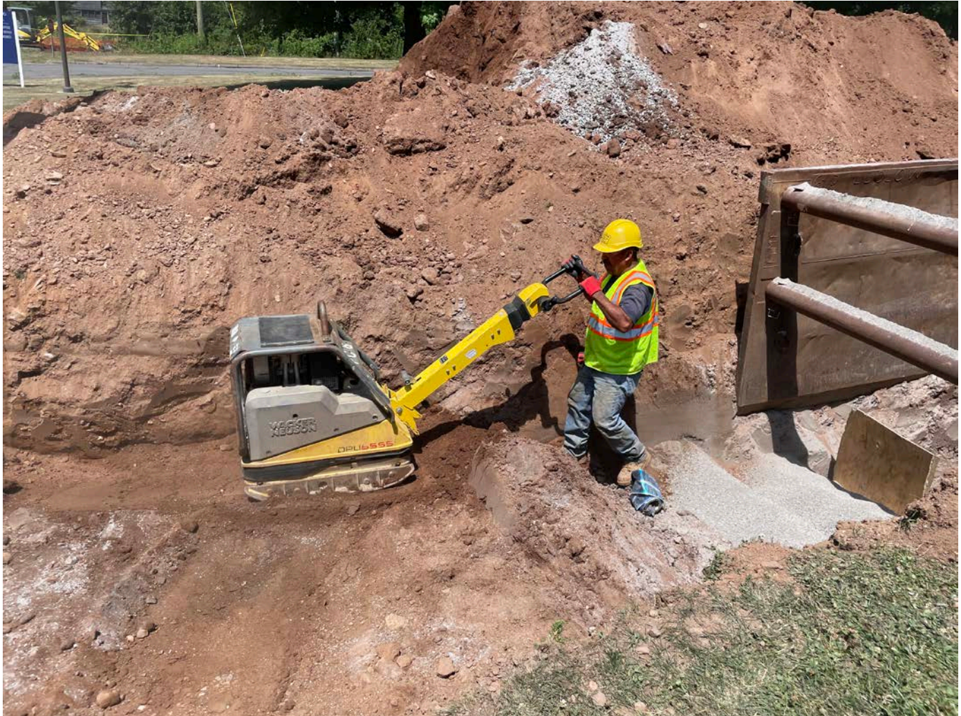
Picture 8: Ludlow using a plate compactor on backfill they placed over 4" and 8" DIP they installed at Station 529+64. View to the north.
