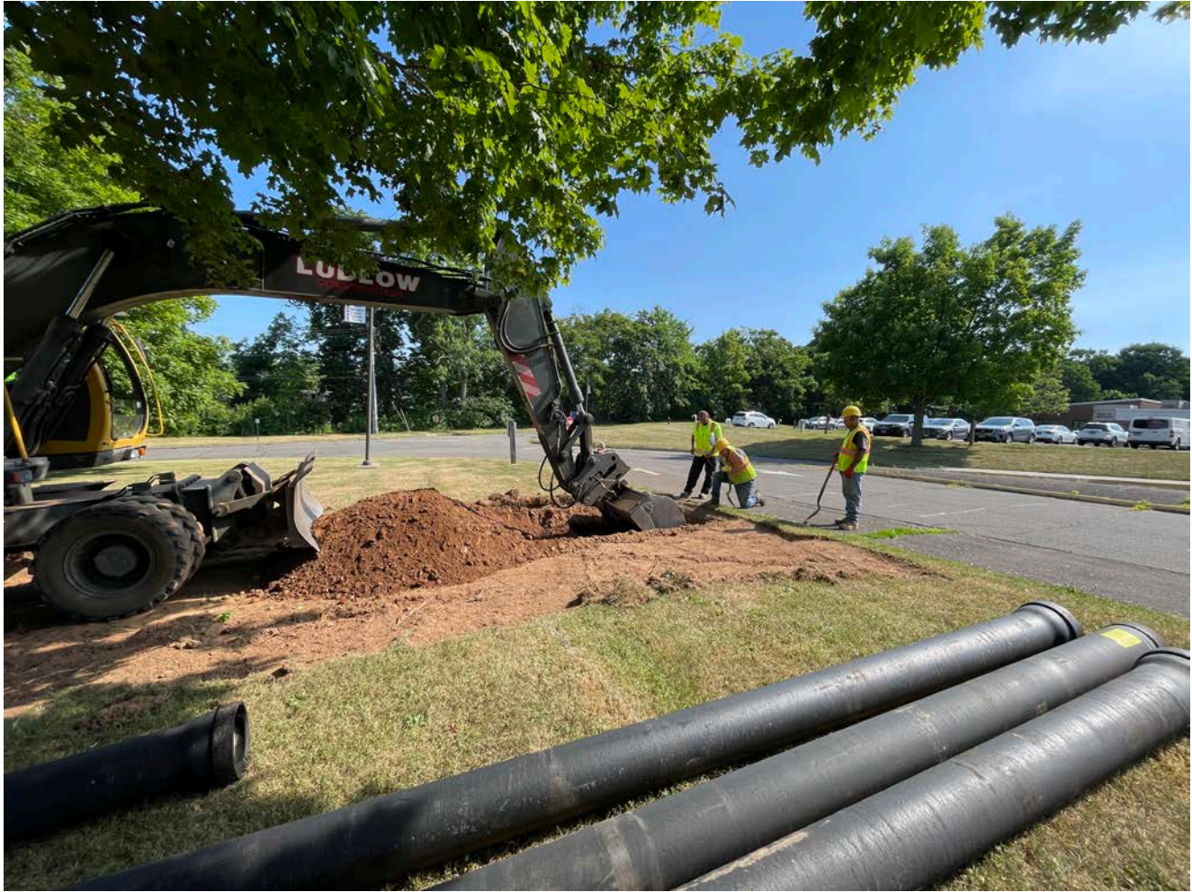
Picture 2: Ludlow excavating a test pit at Station 529+64 to locate subsurface utilities prior to the installation of 4" and 8" DIP. View to the northeast.
