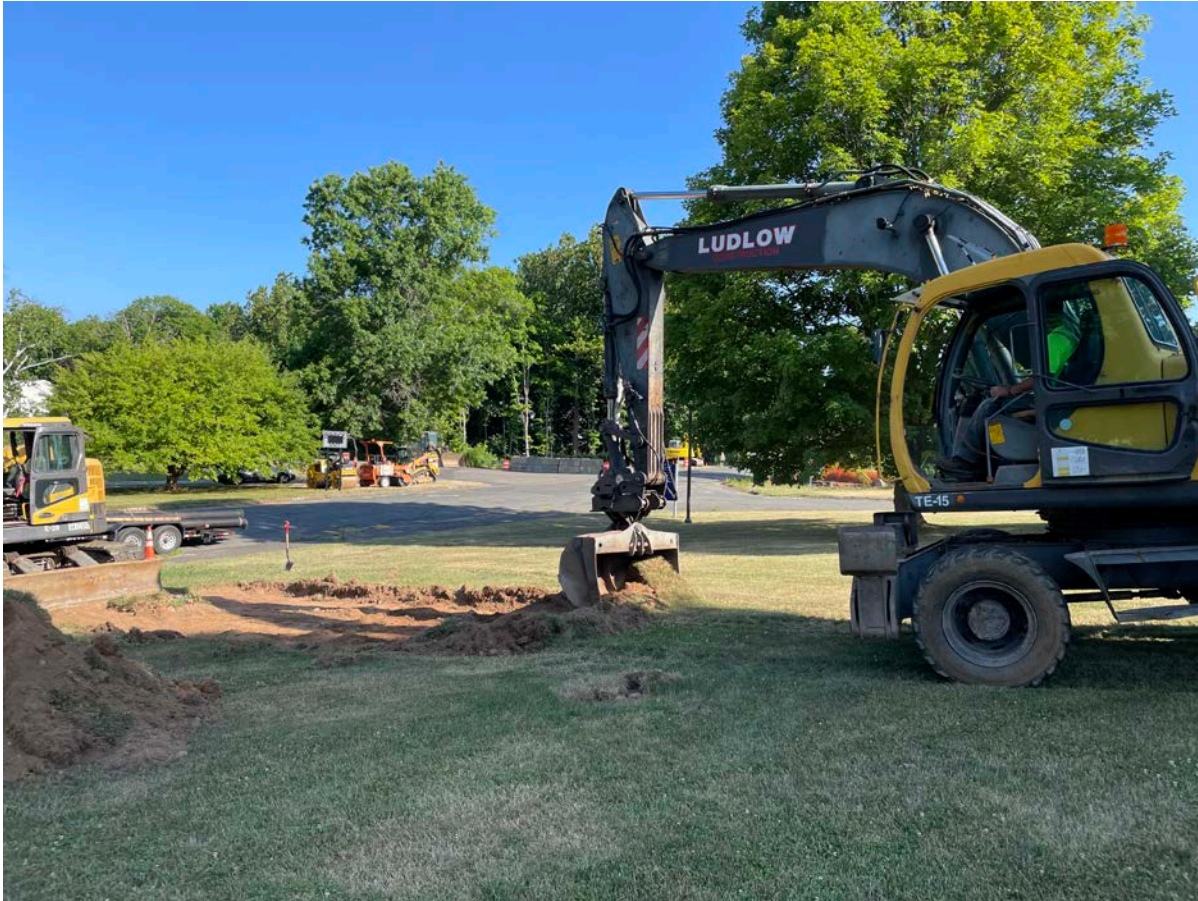
Picture 1: Ludlow stripping turf from the footprint of where they plan to install 4" and 8" DIP at Station 529+64 on Pickett Lane, Durham. View to the north.
