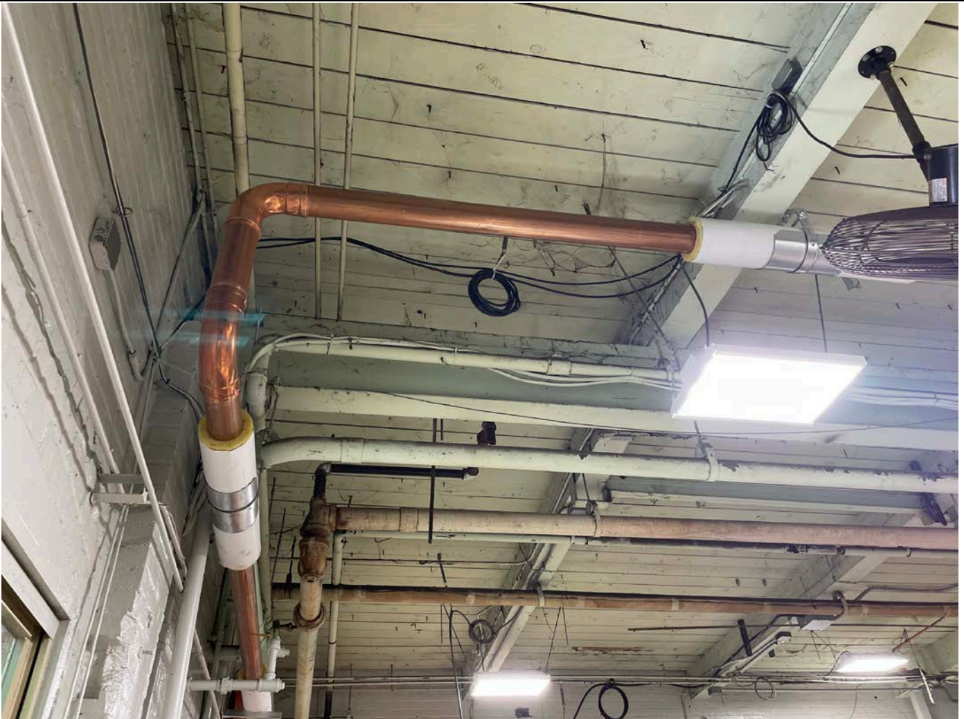
Picture 6: 4" copper pipe that West State Mechanical installed on the ceiling of the Durham Manufacturing facility.
