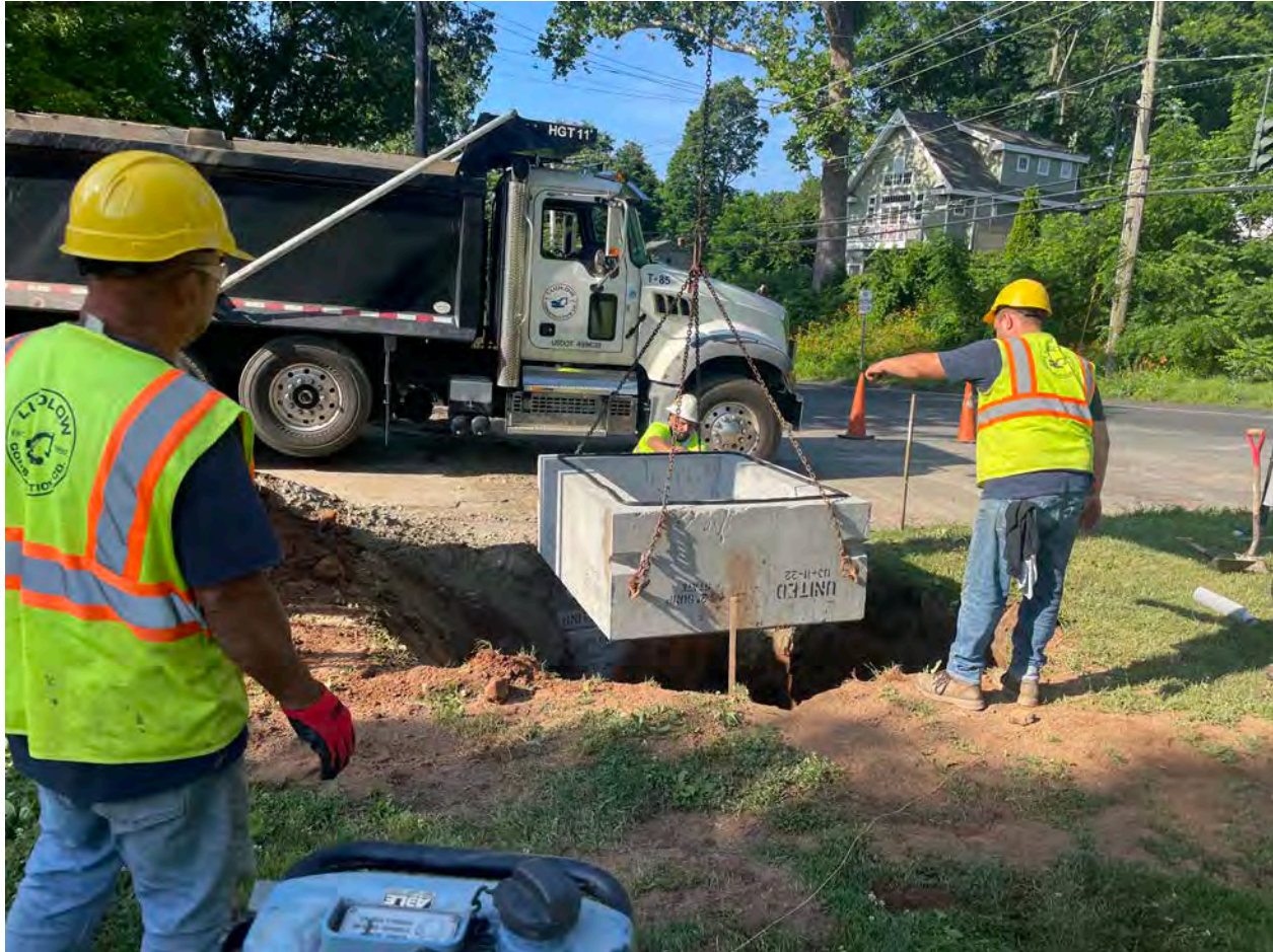
Picture 3: Ludlow placing a section of the second catch basin they are installing at Station 500+50; immediately north of the catch basin they installed on Pickett Lane on June 30, 2022. View to the southwest.
