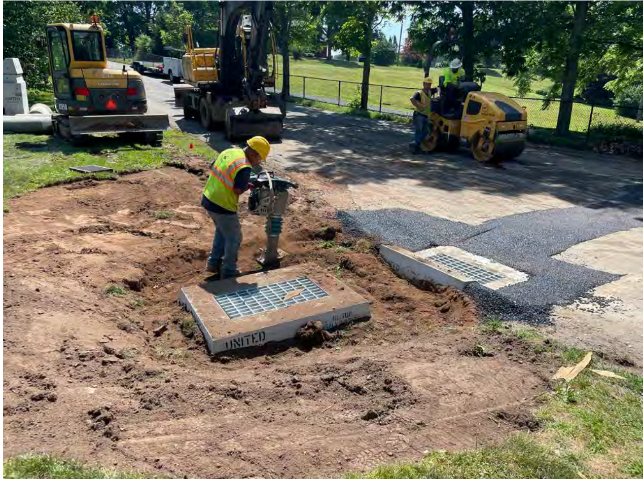
Picture 8: Ludlow compacting backfill around the catch basin they installed today at Station 500+50 to the north of Pickett Lane. View to the southeast.
