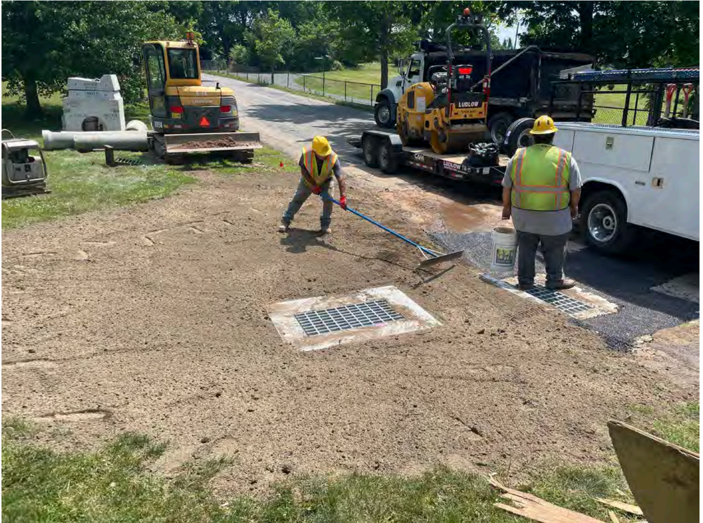
Picture 10: Ludlow raking out loam and grass seed that was spread around the catch basin they just installed at Station 500+50 north of Pickett Lane. View to the southeast.
