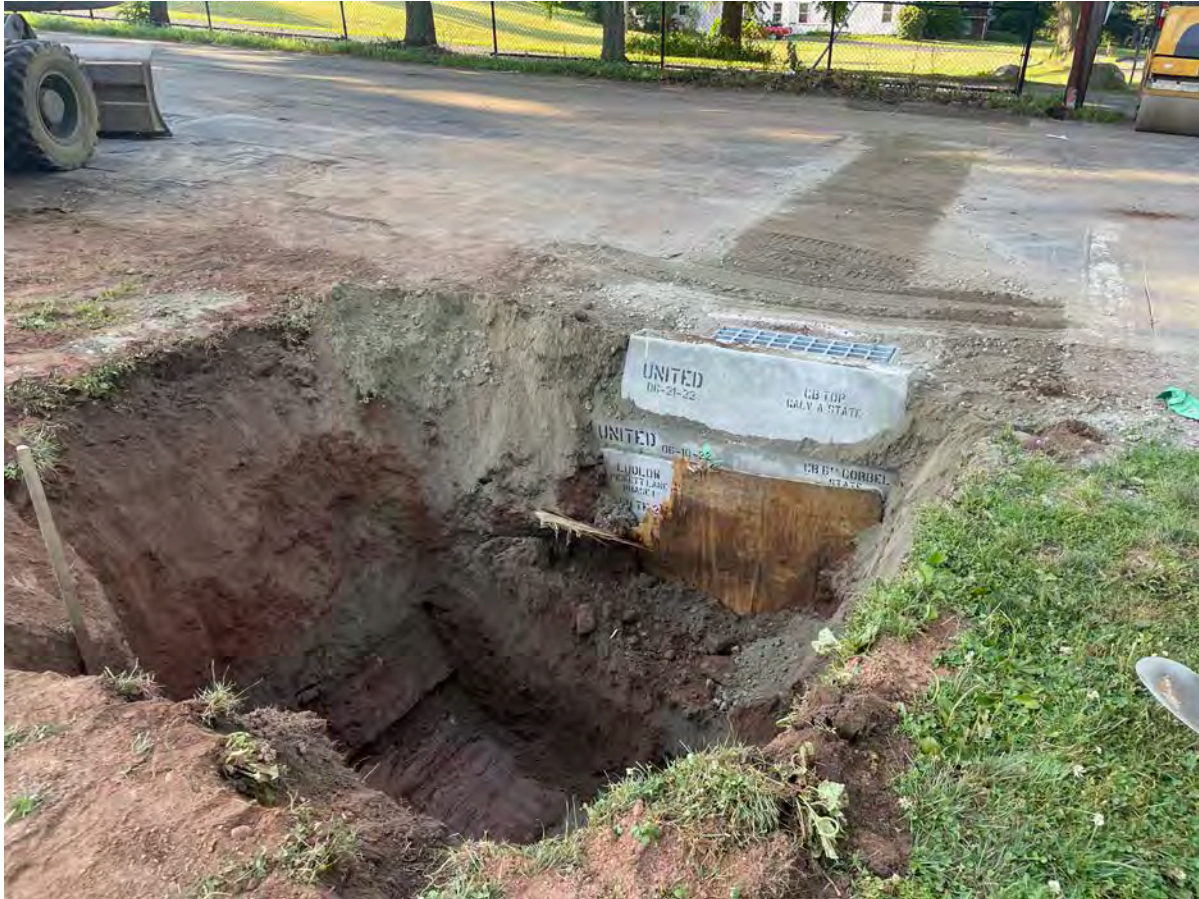
Picture 1: Excavation that Ludlow made on the north side of the catch basin they installed on June 30, 2022 at Station 500+50 on the north side of Pickett Lane, Durham. Ludlow will be installing a second catch basin in the excavation. View to the south.
