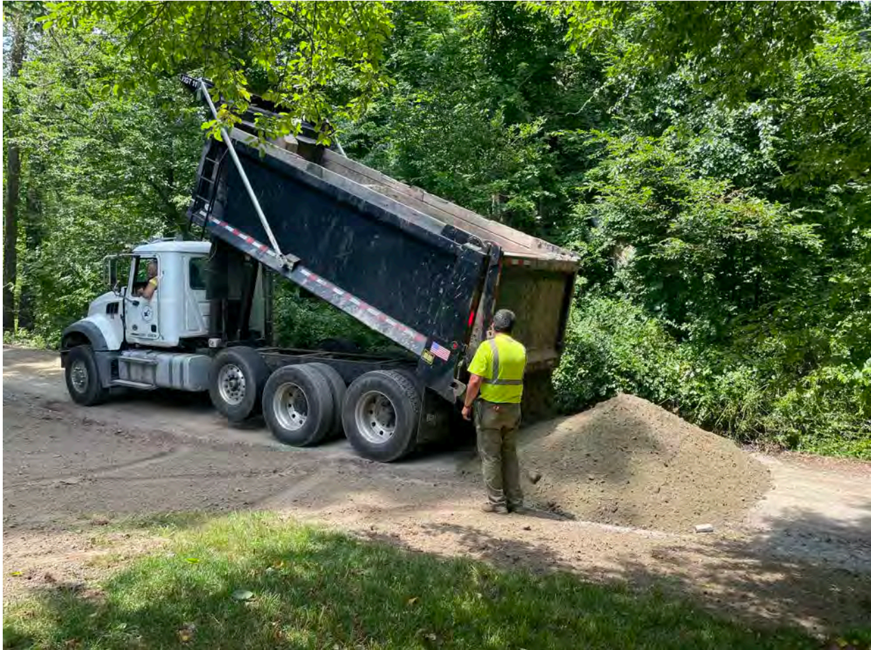
Picture 11: Ludlow placing gravel on the driveway of the 114 Maiden Lane as they work to finish restoration efforts after the installation of a 2" copper water service line. View to the west.
