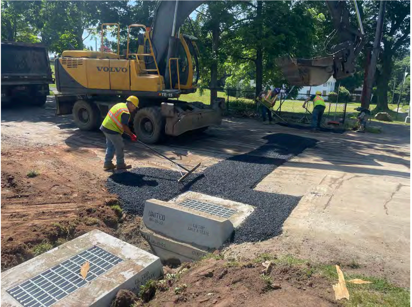
Picture 7: Ludlow raking out freshly-placed asphalt on Pickett Lane at Station 500+50, where they replaced a section of 12" RCP and installed a catch basin on the north side of the road. View to the south.
