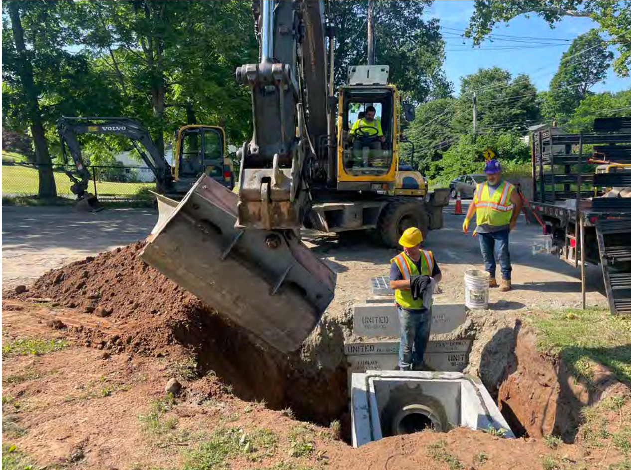
Picture 6: Ludlow placing fill on the east side of the catch basin they are installing at Station 500+50. View to the south.
