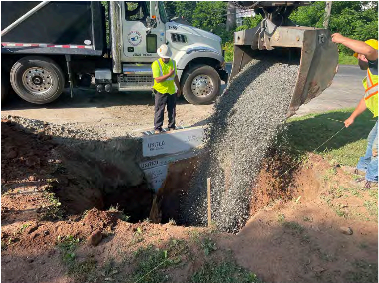
Picture 2: Ludlow placing ¾" stone into the bottom of the excavation that Ludlow made on the north side of the catch basin they installed on June 30, 2022 at Station 500+50 as they prepare to install a second catch basin. View to the southwest.
