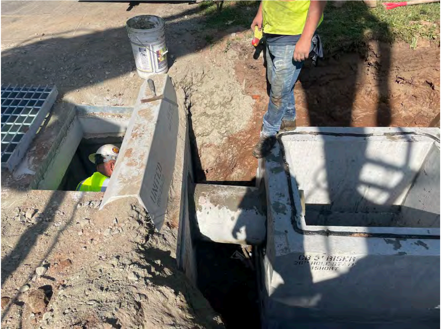
Picture 5: Ludlow placing mortar around a section of 15" RCP that connects the catch basin that Ludlow installed at Station 500+50 to the catch basin they installed today on July 1, 2022. View to the west.
