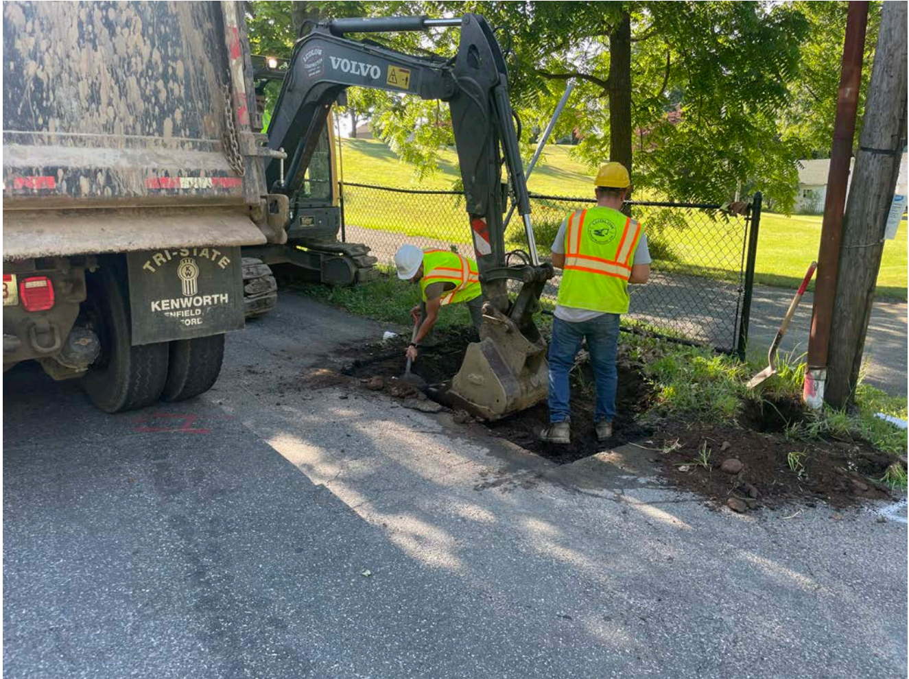
Picture 2: Ludlow excavating at Station 500+50 on the south side of Pickett Lane, Durham, to locate subsurface utilities. View to the southeast.
