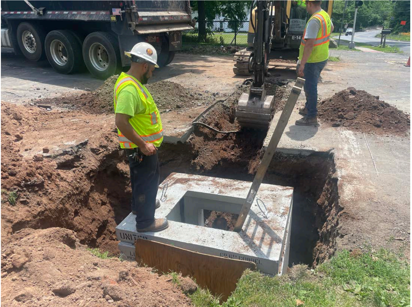
Picture 7: Ludlow excavating across the westbound lane of Pickett Lane as they work to replace a section of 12" RCP that will connect to the south side of the catch basin the just installed. View to the south.
