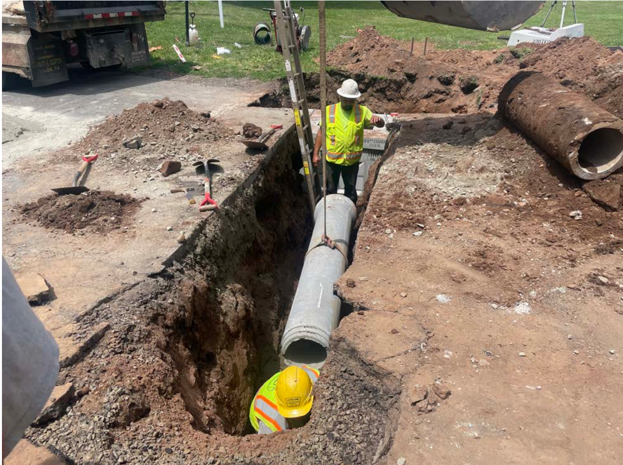
Picture 8: Ludlow installing a section of 12" RCP that will connect to the south side of the catch basin the just installed. View to the north.
