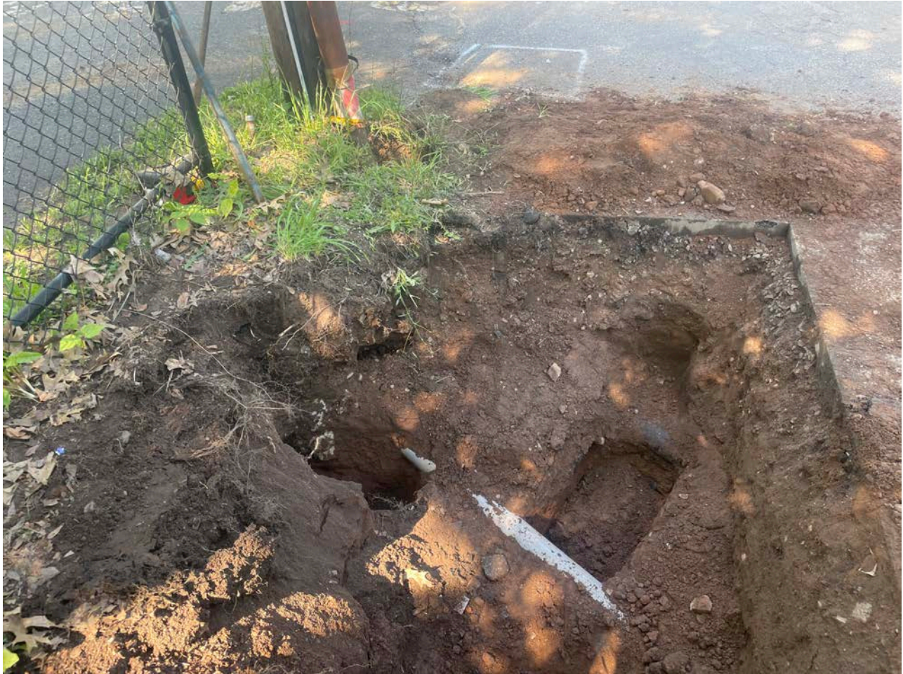
Picture 4: Subsurface utilities that Ludlow daylighted on the south side of Picket Lane at Station 500+50. View to the southwest.
