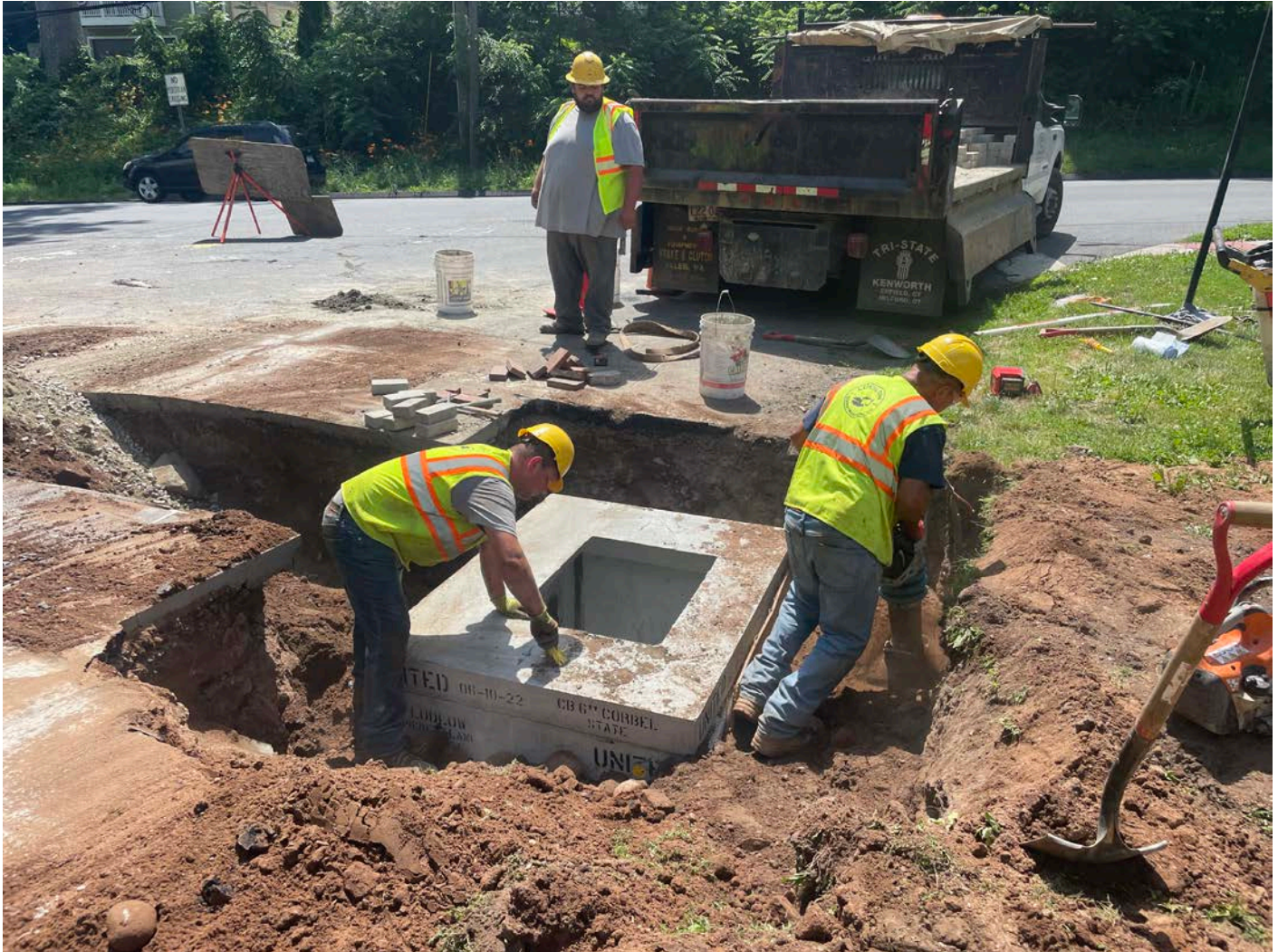
Picture 9: Ludlow compacting fill around sections of a catch basin they are installing on the north side of Pickett Lane at Station 500+50. View to the southeast.
