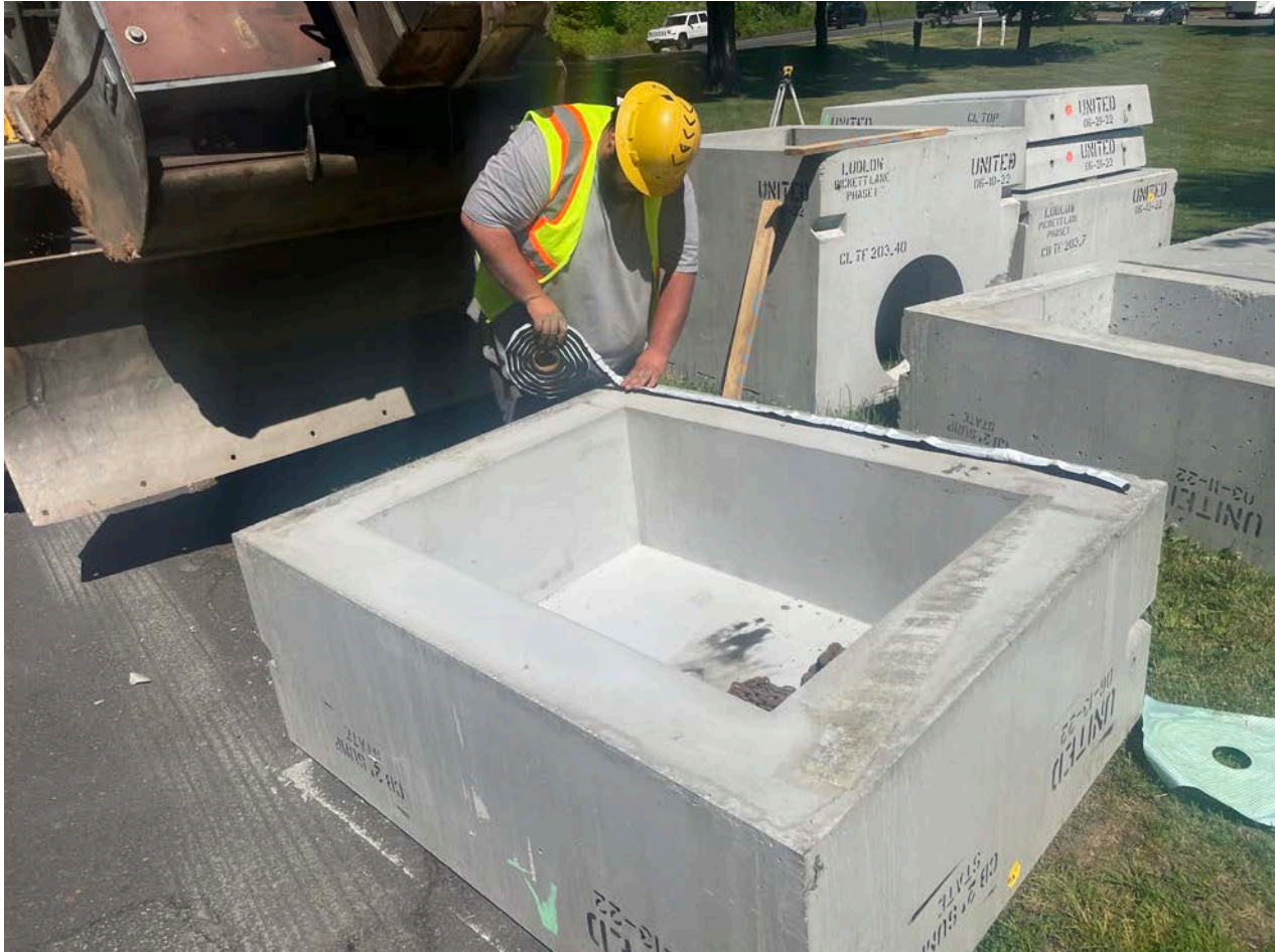
Picture 6: Ludlow placing ConSeal tape to a section of the catch basin they are about to install at Station 500+50 on the north side of Pickett Lane.
