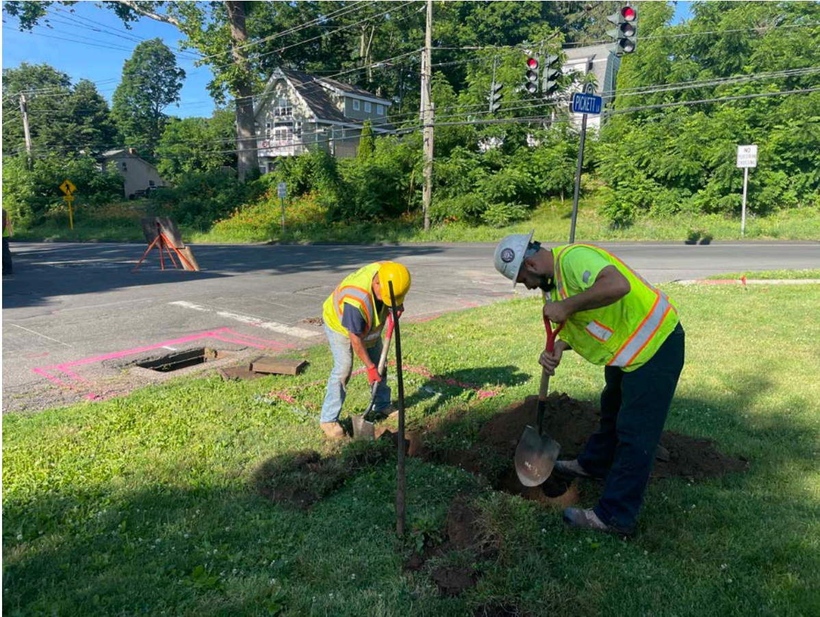
Picture 1: Ludlow hand excavating at Station 500+50 on the north side of Pickett Lane, Durham, to located subsurface utilities before installing a new catch basin. View to the southwest.
