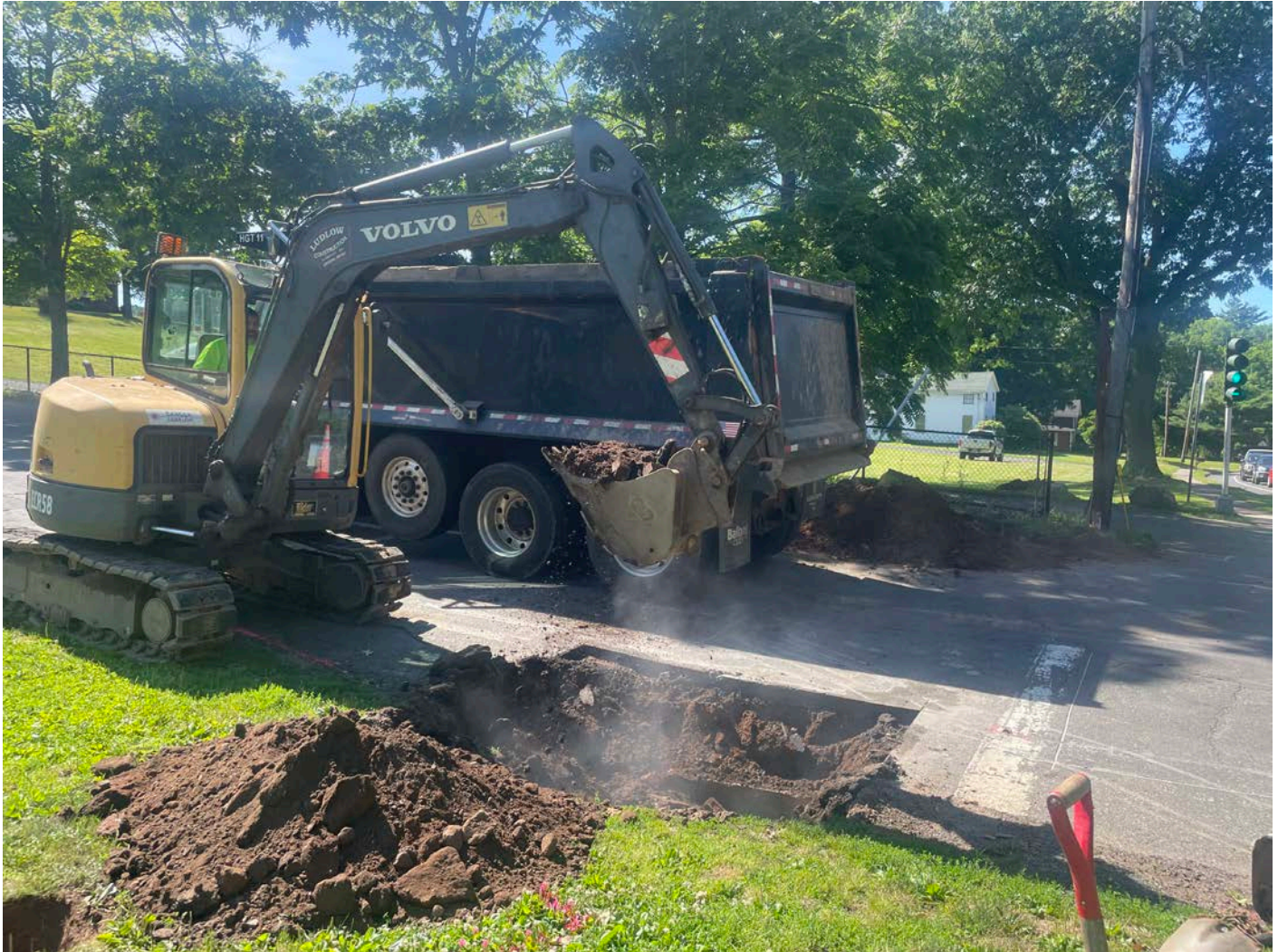
Picture 5: Ludlow excavating on the north side of Picket Lane at Station 500+50 after removing the existing catch basin. View to the south.
