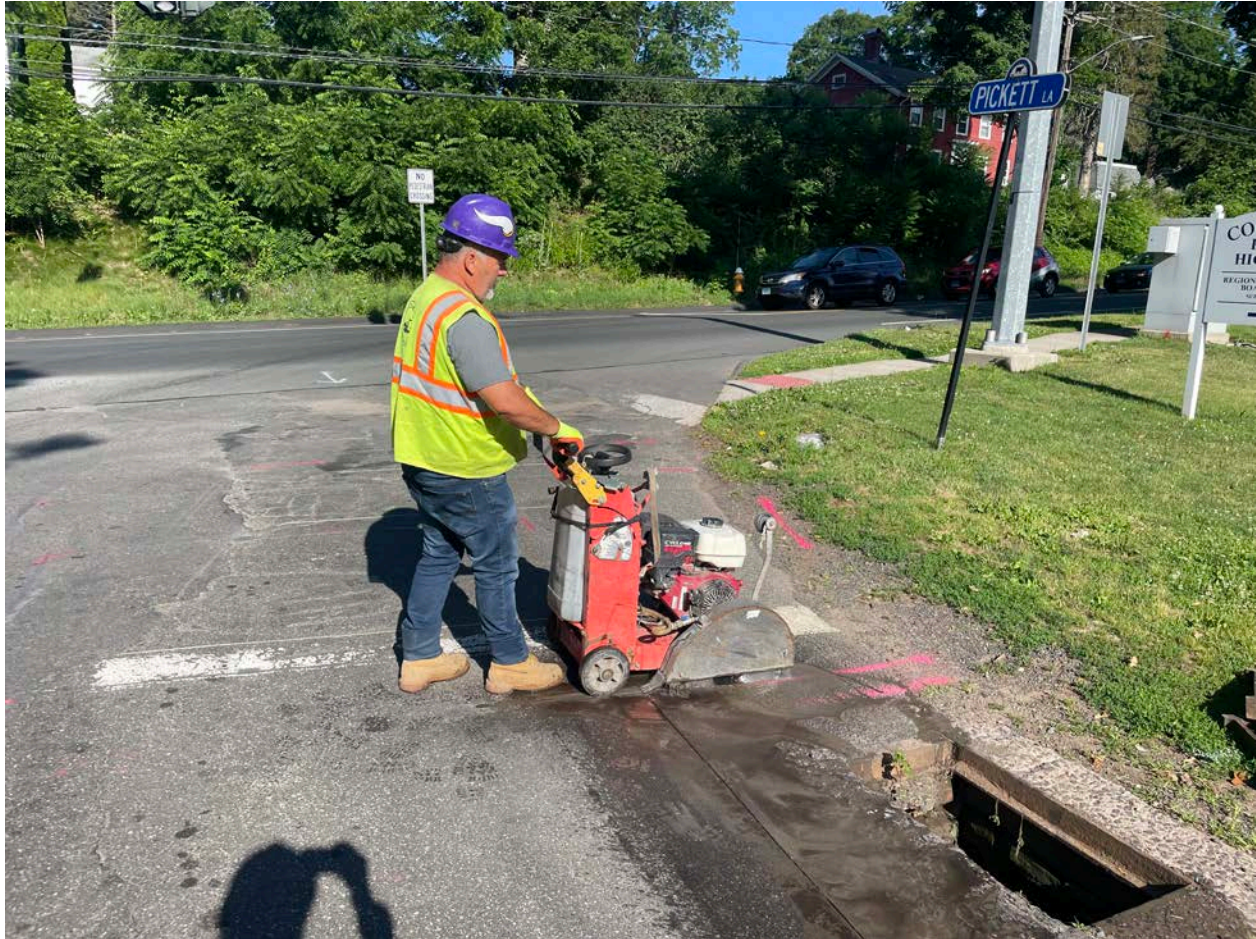
Picture 3: Ludlow saw-cutting around a catch basin that they are replacing today on Pickett Lane, Durham. View to the west.
