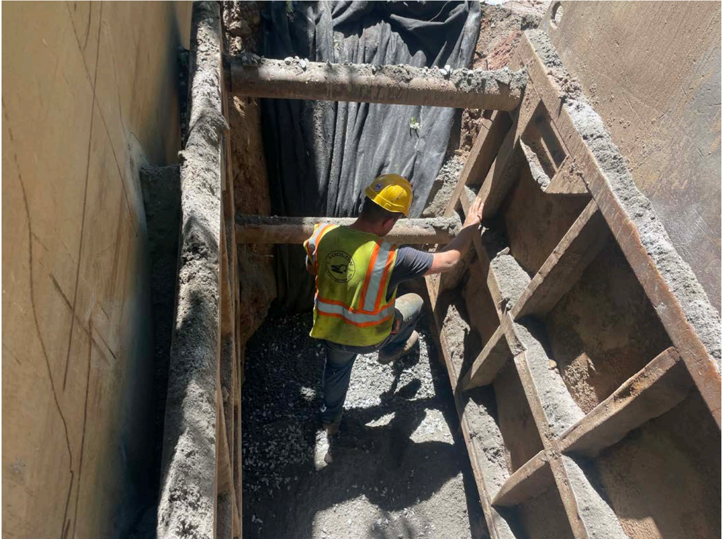
Picture 7: Ludlow placing ¾" gravel on the north side of the Ball Brook culvert located on the 114 Maiden Lane driveway after backfilling over the 2" copper water service line they just finished installing. View to the south.
