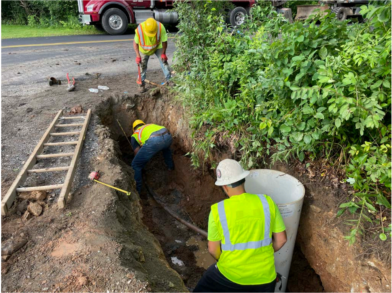
Picture 2: Ludlow installing 2" copper water service line on the west side of the 114 Maiden Lane, Durham, driveway. Note the meter vault located in the foreground on the right that Ludlow is in the process of installing. View to the southwest.
