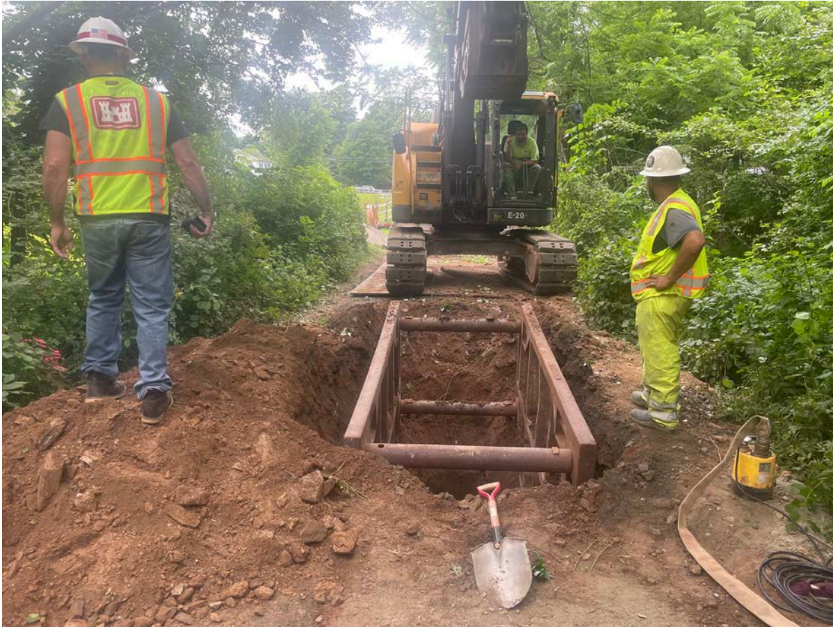
Picture 1: Trench box that Ludlow has just placed into an excavation they made on the north side of the Ball Brook Culvert located on the 114 Maiden Lane, Durham, driveway as they continue to install a 2" copper water service line. View to the south.
