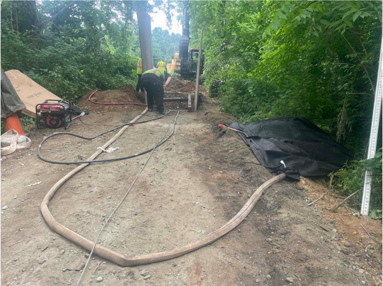
Picture 2: Ludlow pumping water from the excavation they made on the north side of the 114 Maiden Lane, Durham, driveway as they work to install a 2" copper water service line. The water is being pumped to the west side of the road through a filter bag. View to the south.
