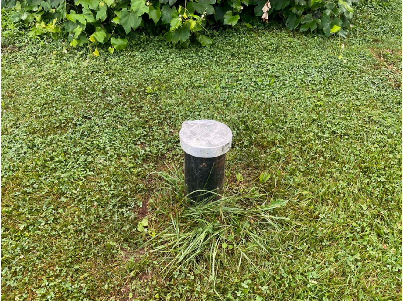
Picture 5: Lockable cap that Grela placed on top of a new section of steel riser that they welded onto the well located on the south side of the 110 Maple Avenue, Durham, property. View to the north.
