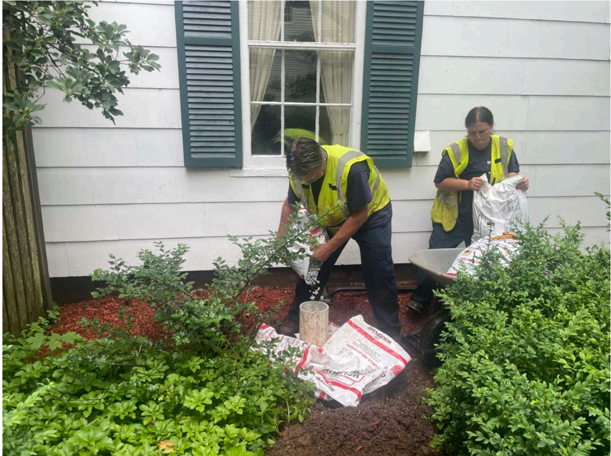
Picture 3: Grela placing bentonite chips into the well located on the south side of the 252 Main Street, Durham, residence as part of well decommissioning activities. View to the north.
