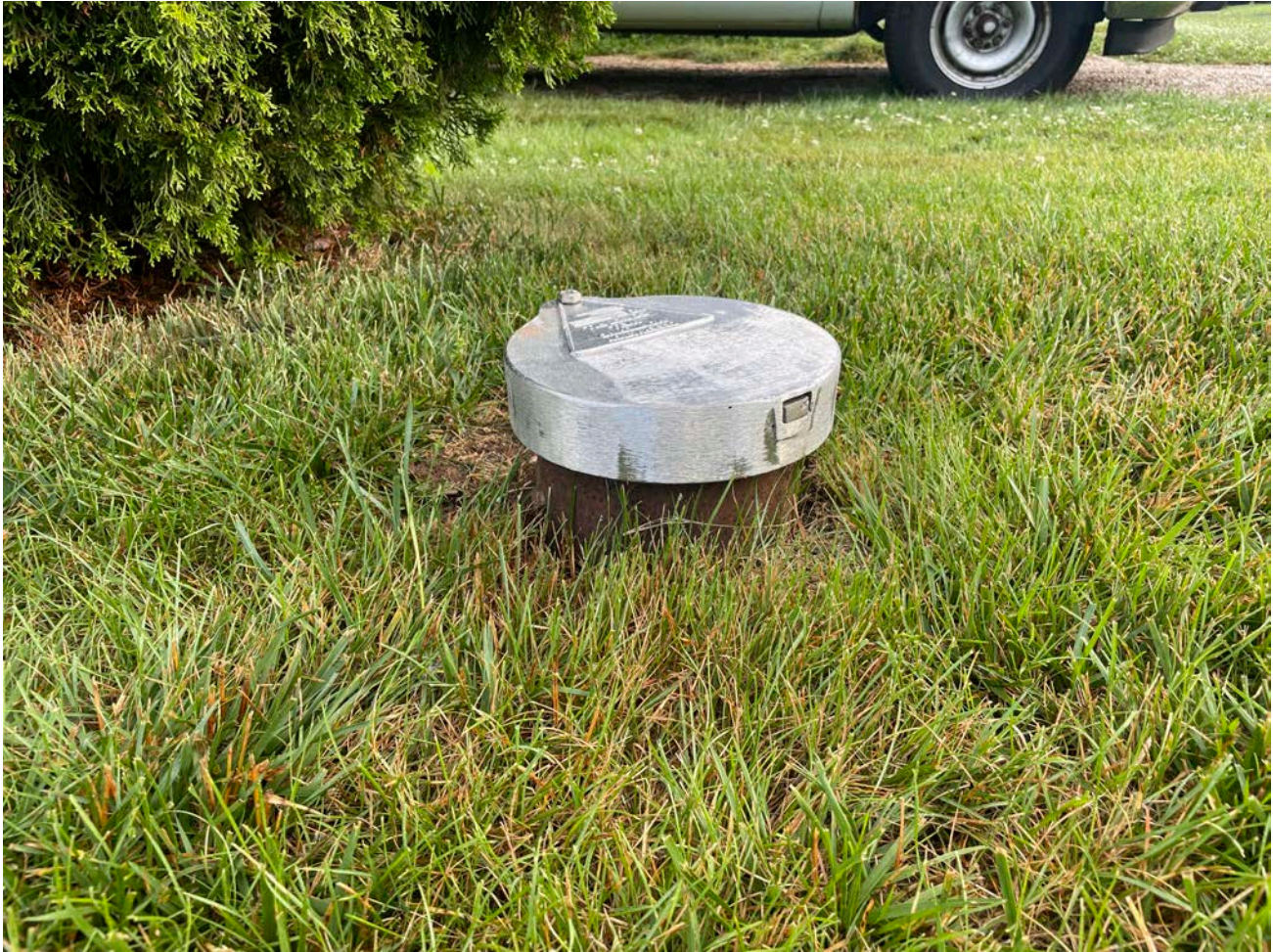
Picture 4: Lockable cap that Grela placed on top of the casing of the well located on the north side of the 166 Maple Avenue, Durham, property. View to the northwest.
