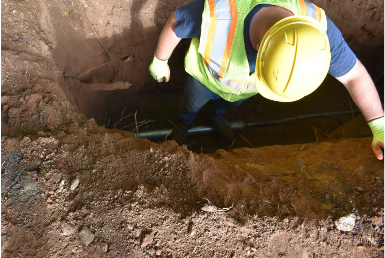
Photo 2: Ludlow operator guiding “Mole” drilling tool at south end of north trench at 114 Maiden Lane.
