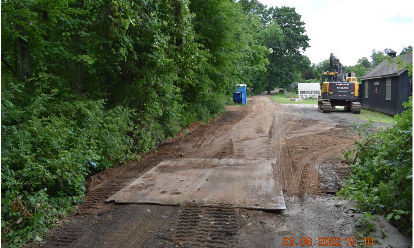
Photo 6: Pipe trench at 114 Maiden Lane at the end of the workday. Steel plate covers small length of open trench. View to the north.
