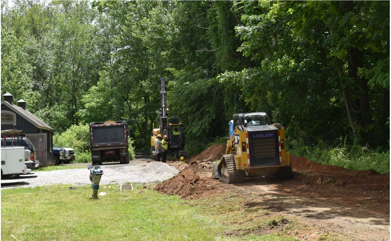
Photo 5: Ludlow extending pipe trench near “Farm Market” building at 114 Maiden Lane. View to the southwest.
