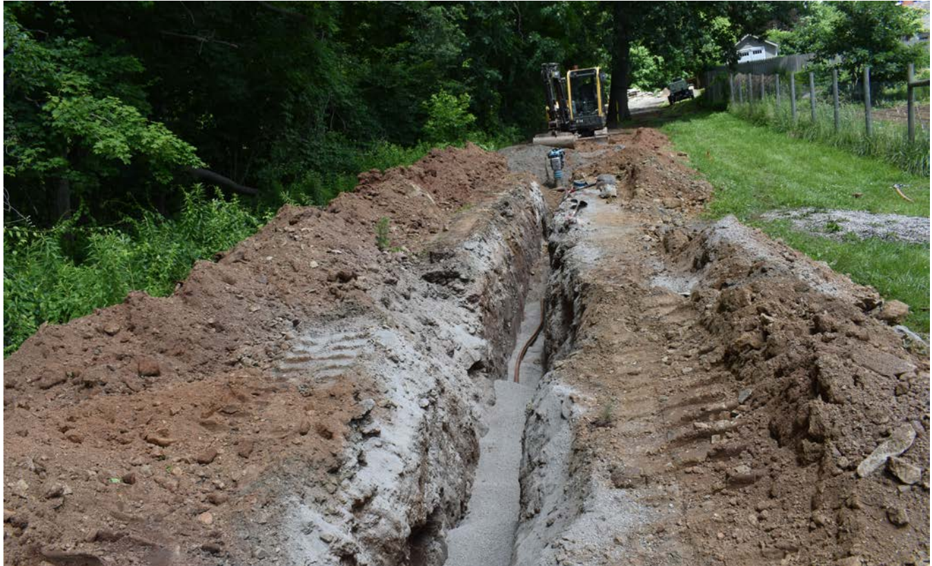
Photo 3: Water pipe laid in trench. Ludlow has added sand bedding at 114 Maiden Lane. View to the north.
