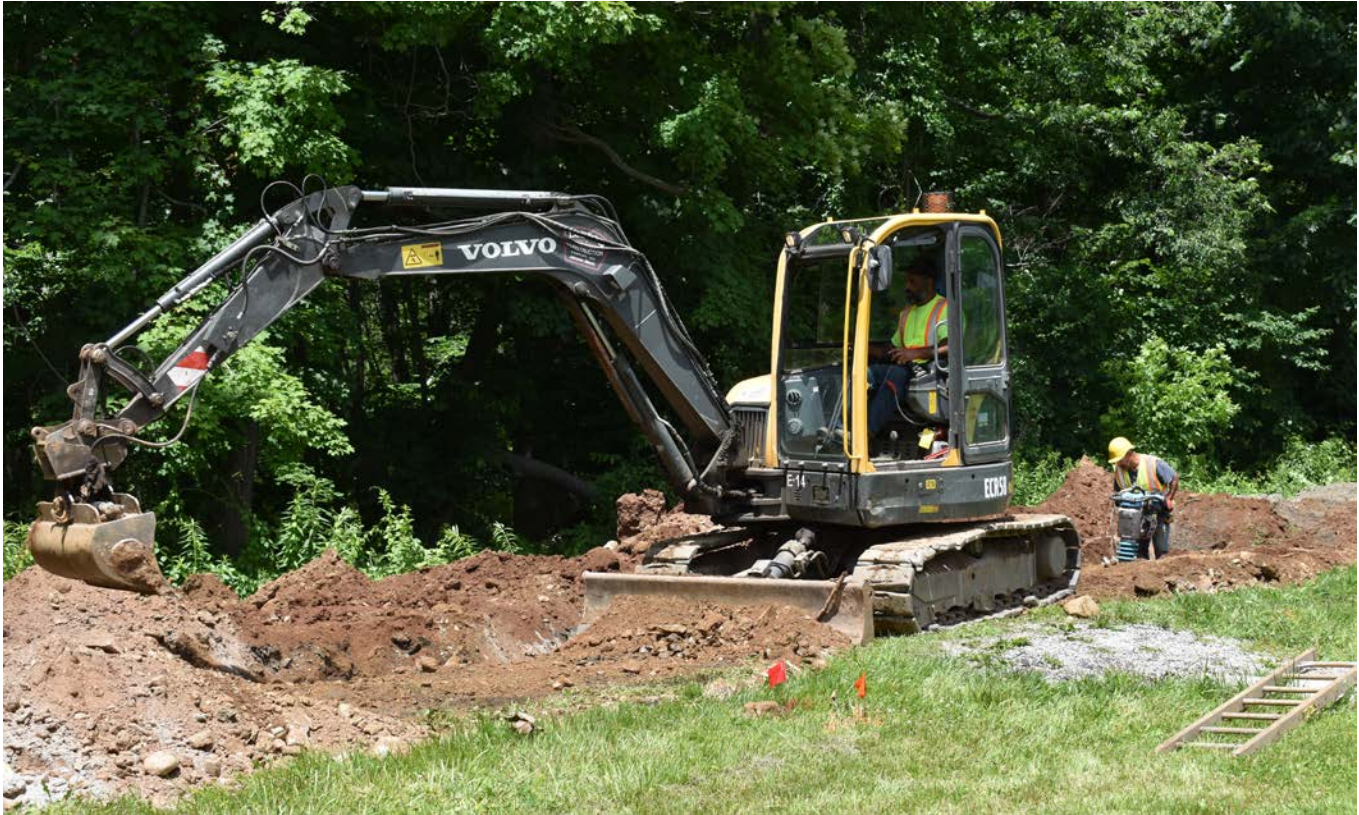
Photo 4: Ludlow operators backfilling and compacting pipe trench at 114 Maiden Lane. View to the northwest.
