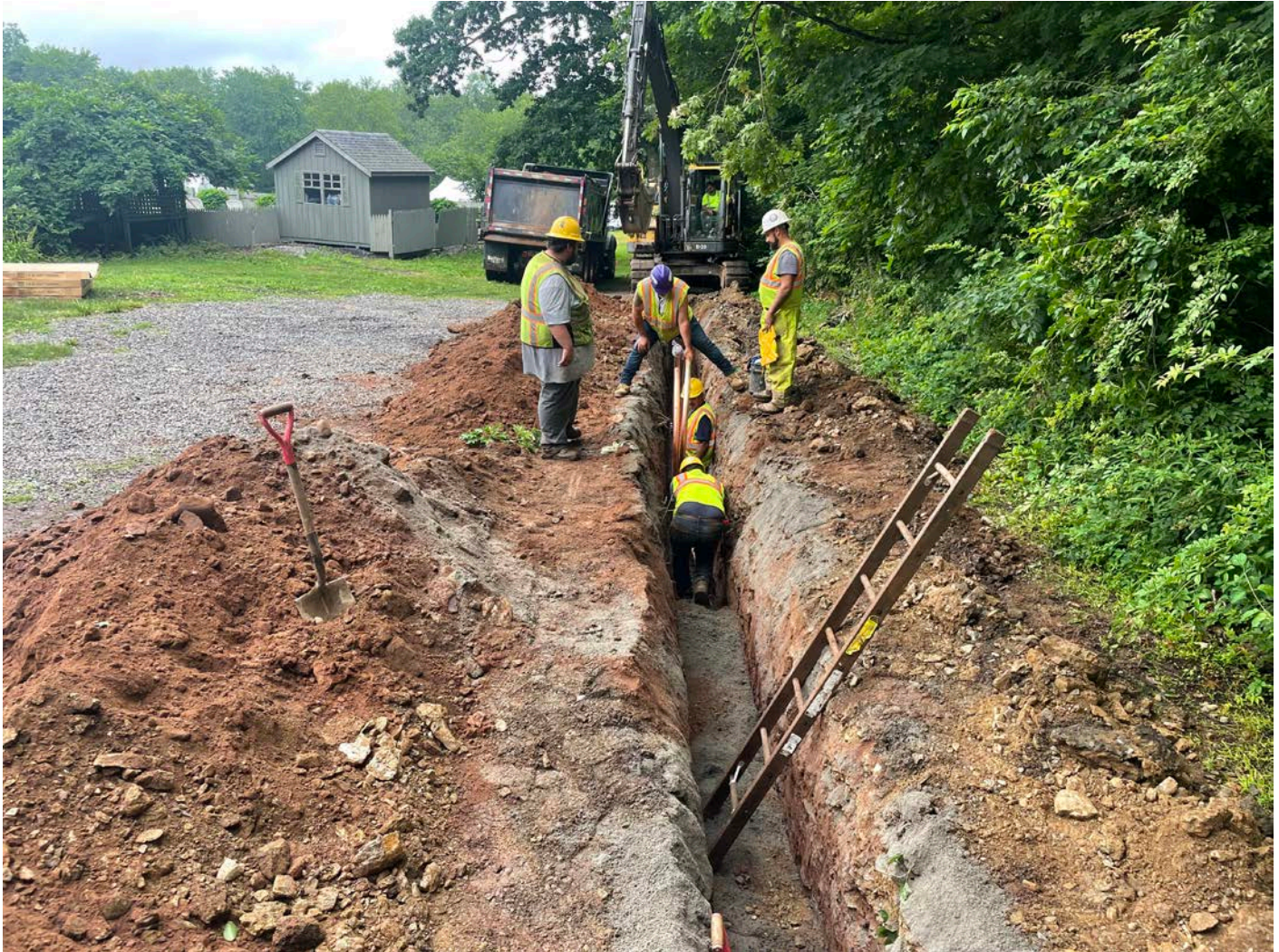
Picture 9: Ludlow installing a 2" copper water service line in the trench they excavated down the driveway of the 114 Maiden Lane, Durham, property. View to the south.
