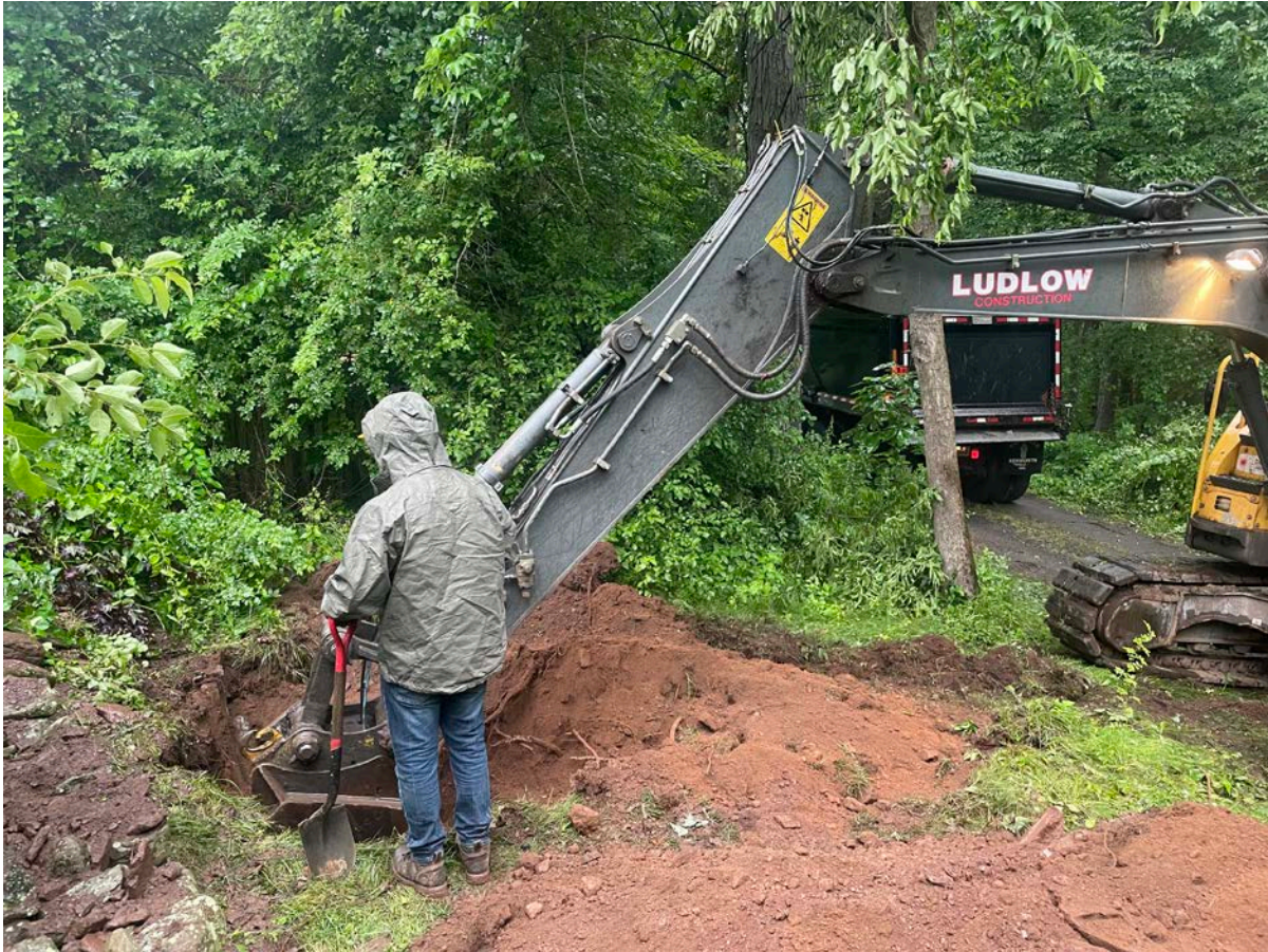
Picture 1: Ludlow excavating on the west side of a stone wall located next to the northwest corner of the 114 Maiden Lane, Durham, residence as they work to install a 2" copper water service line. View to the south.
