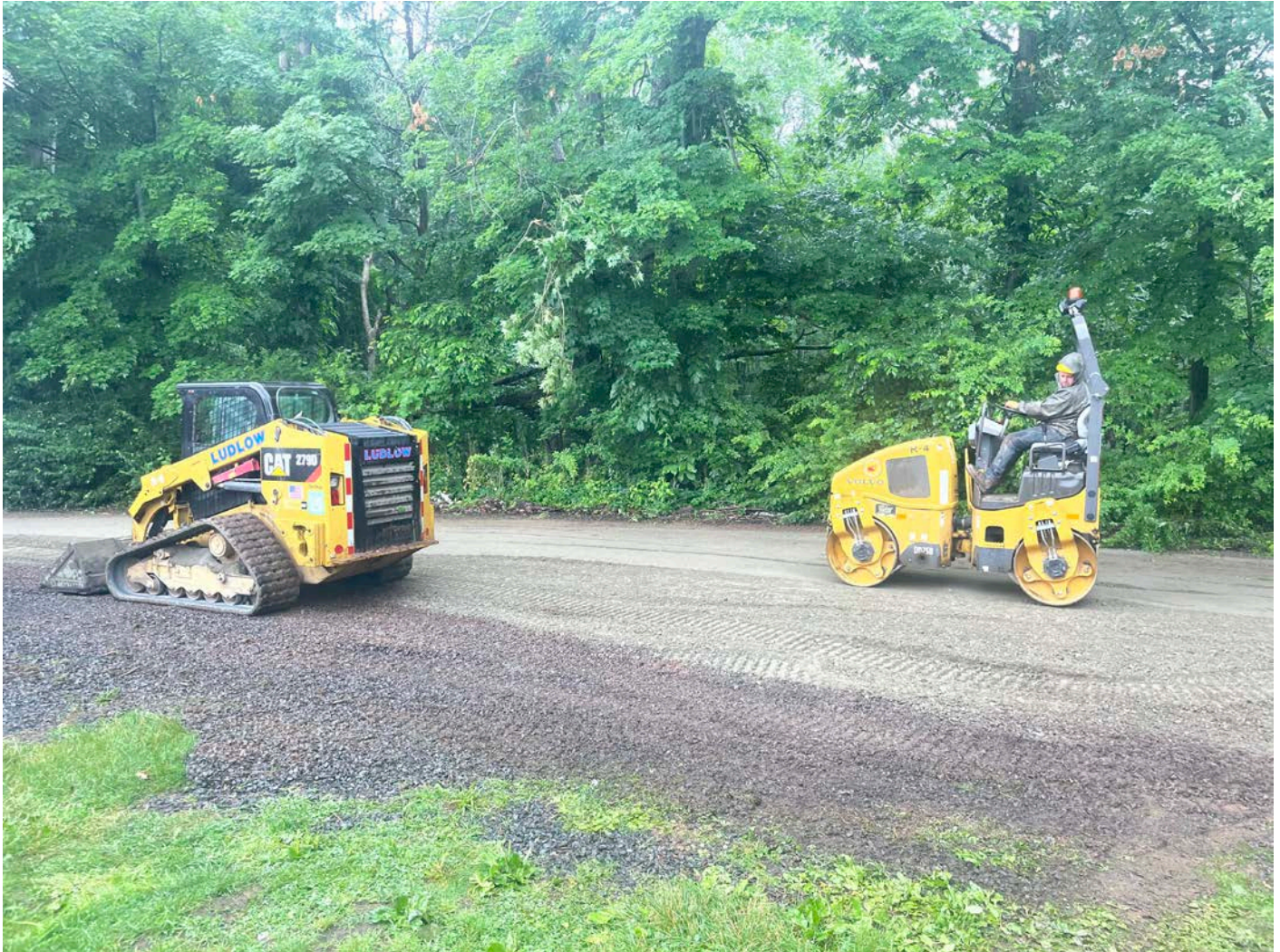
Picture 11: Ludlow grading and compacting the material that was backfilled over the 2" copper water service line they installed at the 114 Maiden Lane, Durham, property. View to the west.
