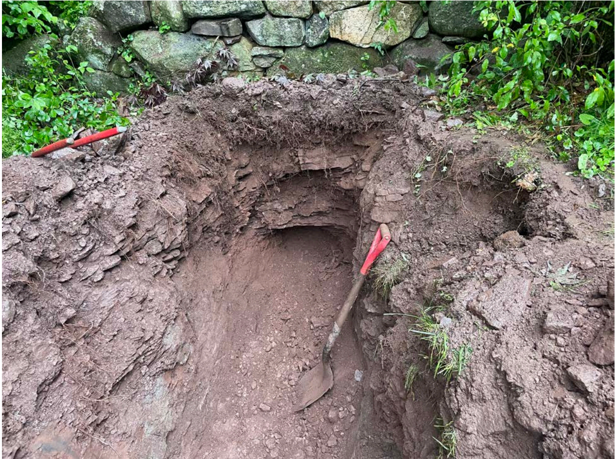
Picture 3: Ludlow having excavated on both sides of the stone wall located next to the northwest corner of the 114 Maiden Lane, Durham, residence where they will use a pneumatic mole to punch a hole beneath the wall to install a 2" copper water service line. View to the west.
