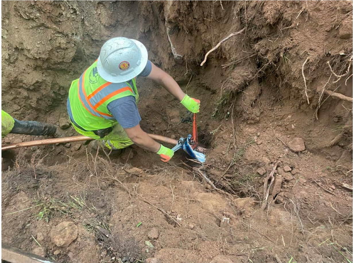
Picture 7: Ludlow preparing to use a brass union to connect two sections of 2" copper water service line at the 114 Maiden Lane, Durham, property.
