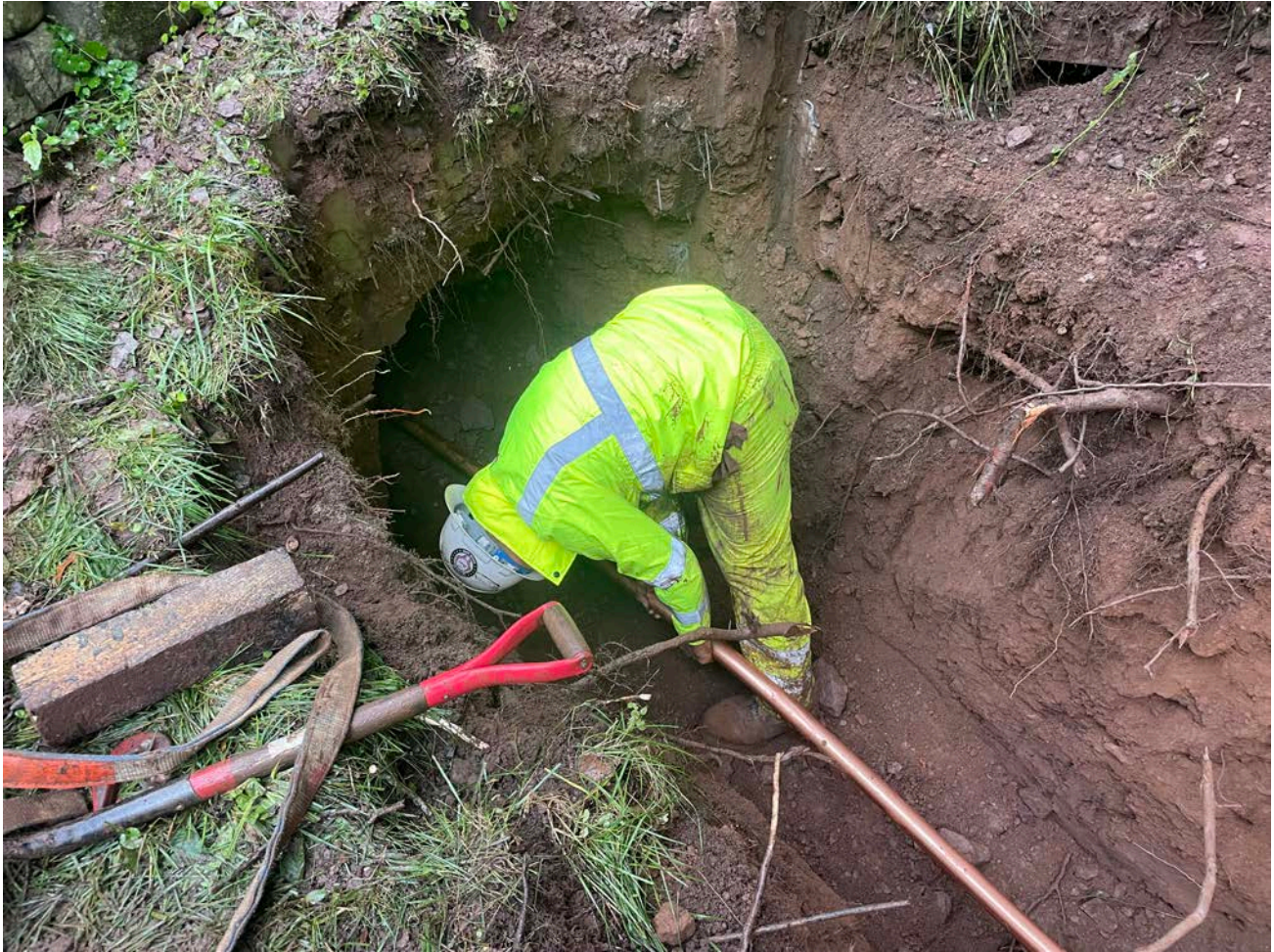
Picture 4: Ludlow running a 2" copper water service line beneath the stone wall located next to the northwest corner of the 114 Maiden Lane, Durham, residence. View to the southeast.
