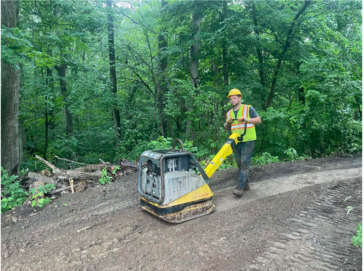
Picture 10: Ludlow compacting the material that was backfilled over the 2" copper water service line they installed at the 114 Maiden Lane, Durham, property. View to the northwest.
