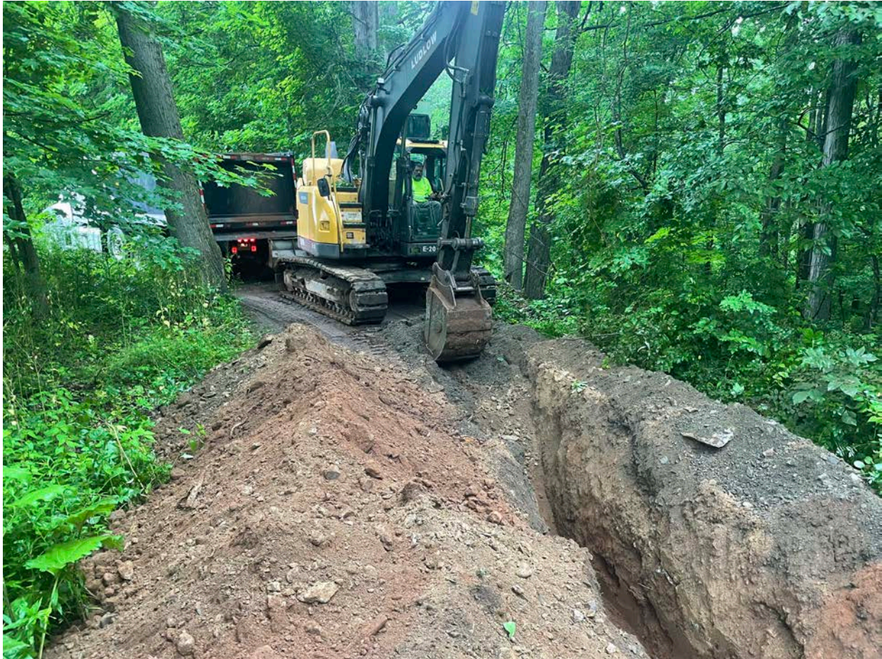
Picture 8: Ludlow excavating down the driveway of the 114 Maiden Lane, Durham, property as they install a 2" copper water service line. View to the southwest.
