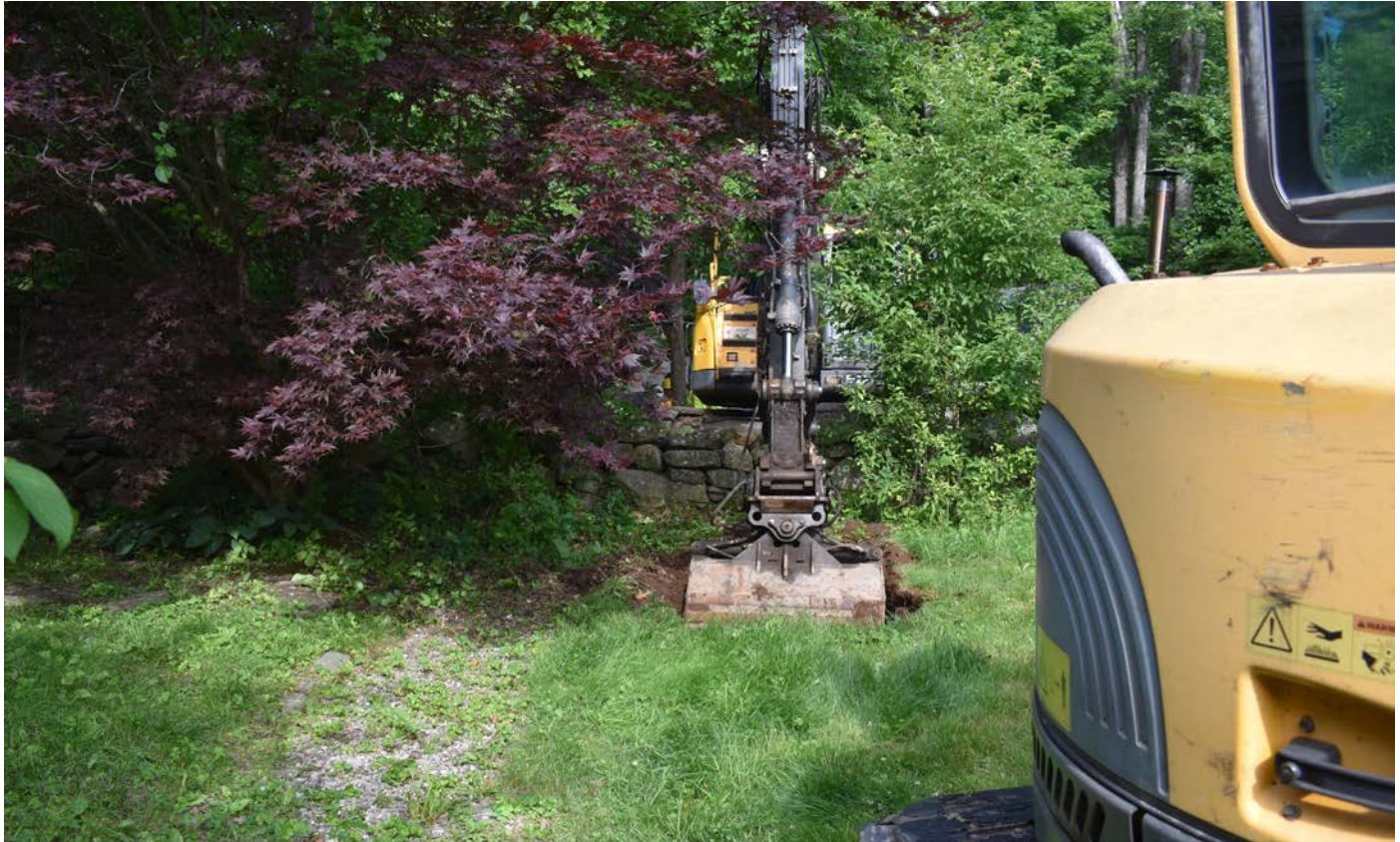
Photo 1: Ludlow crew starting to excavate trench for new pipe on west side of house at 114 Maiden Lane. View to the west.
