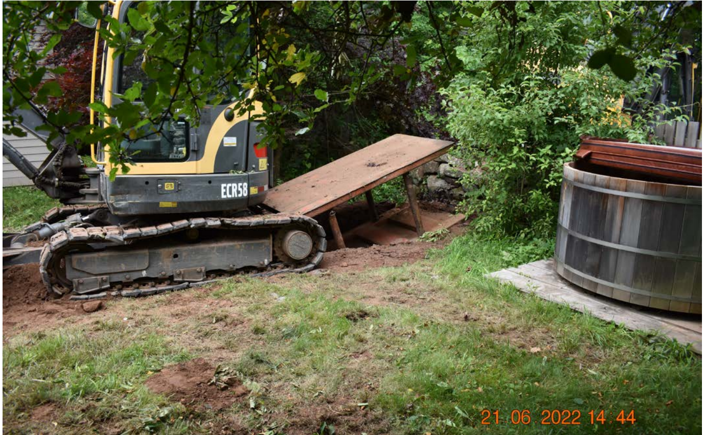
Photo 9: Western end of pipe trench at 114 Maiden Lane. Small excavator and small trench box used to provide barriers for approx. 8-foot length of open trench; remainder of trench has been backfilled. View to the south.
