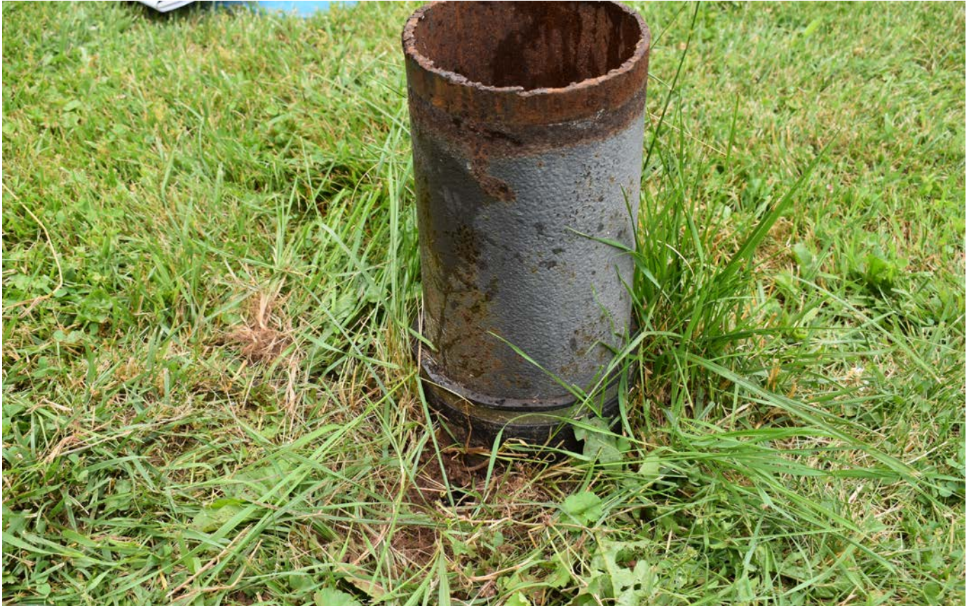
Photo 5: Well casing for former drinking water well at 110 Maple Avenue. The top edge of the rubber coupler can be seen just above the surrounding grass. View to the southeast.
