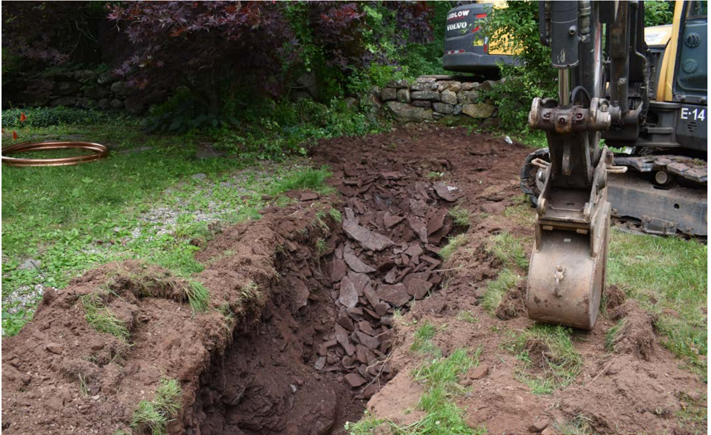
Photo 4: West end of pipe trench at 114 Maiden Lane, showing presence of dense rocky material. Stone wall seen beyond trench. View to the west.
