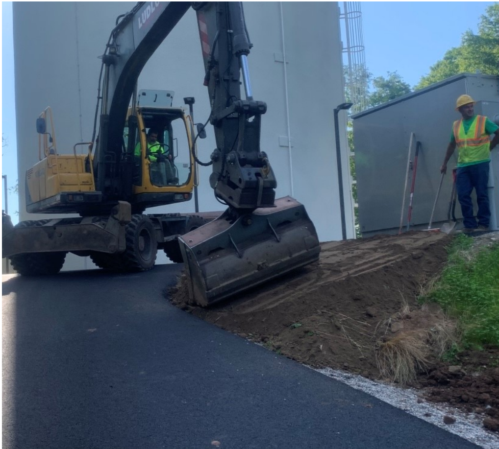
Picture 1: Ludlow at the end of the Shared Access Driveway (Water Tank) is placing topsoil around newly placed asphalt using Ludlow personnel, and an excavator.
