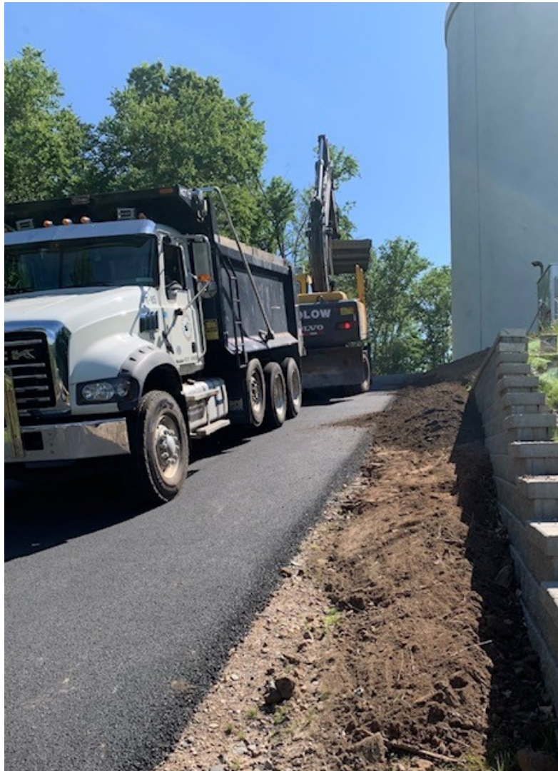
Picture 4: Ludlow at the Shared Access Driveway (Water Tank) is continuing the placement of topsoil around the newly paved asphalt.
