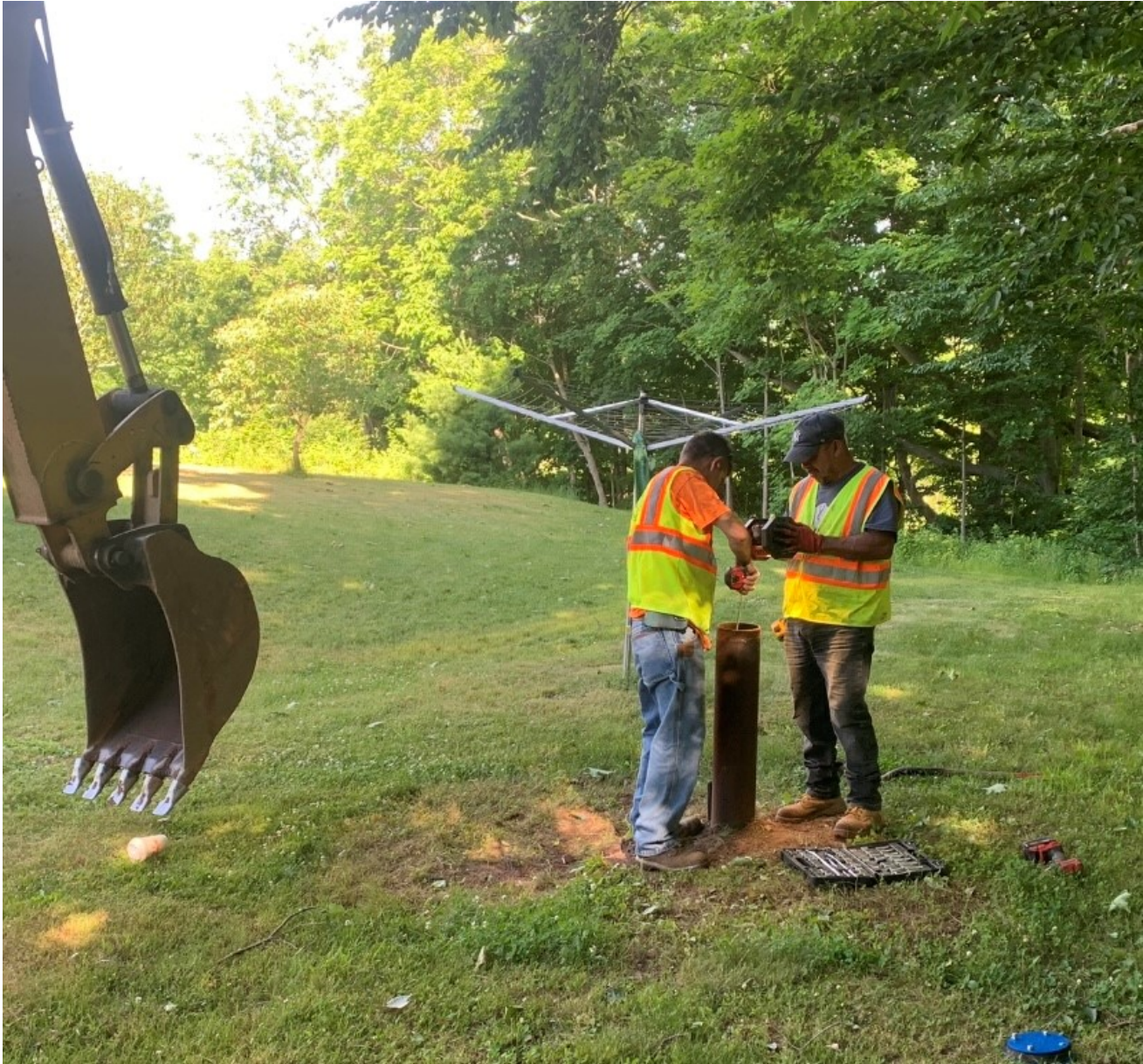
Picture 2: Ludlow at 10 Johns way is measuring the depth to the pitless adapter, the measurement came out to be 4 feet.
