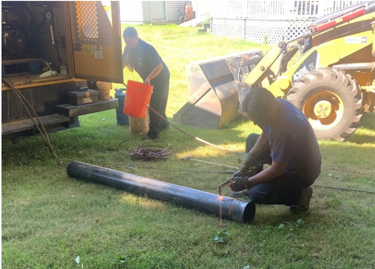
Picture 5: Grela Well Drilling at 10 Johns Way cutting the new well casing to the appropriate length.
