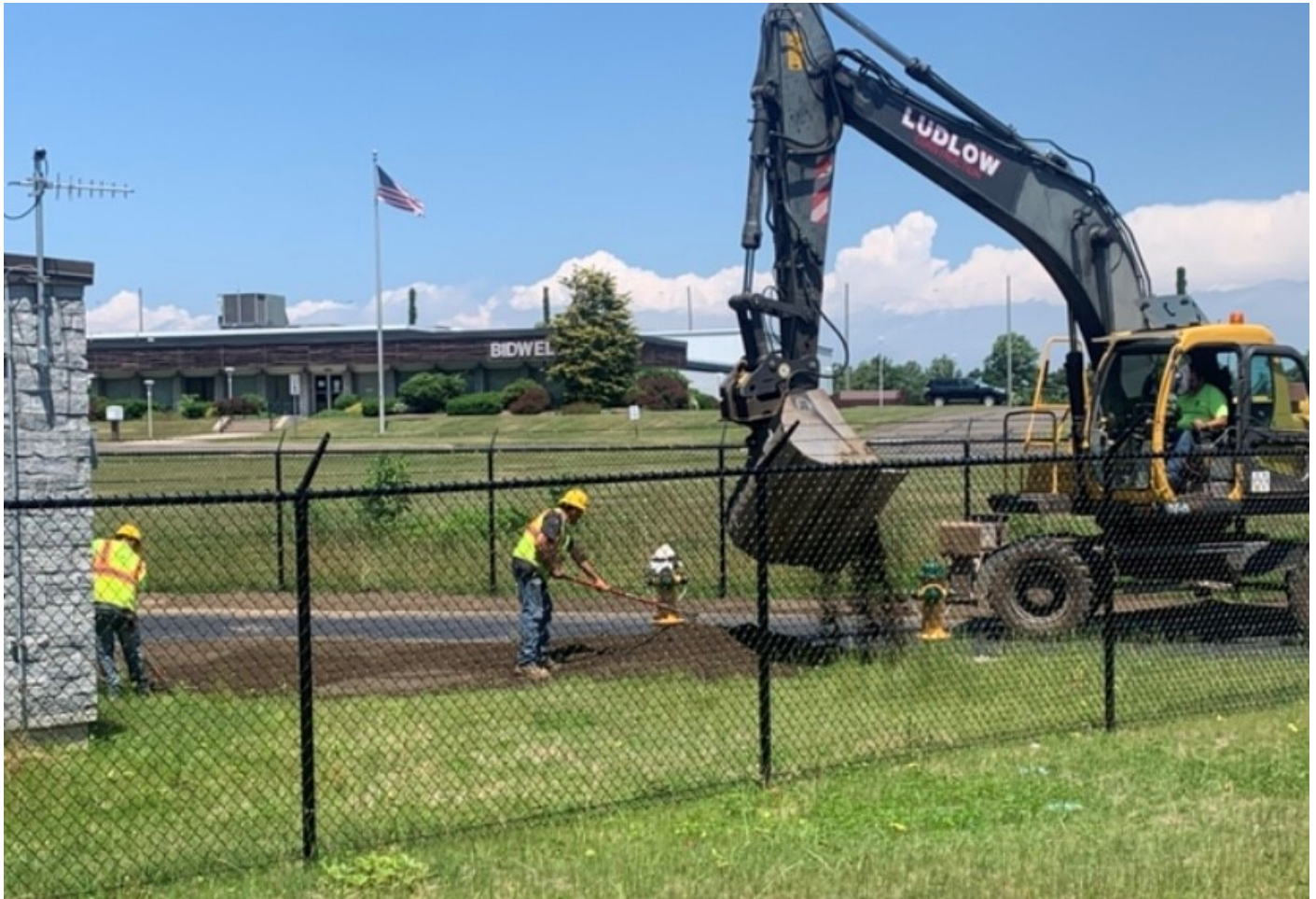
Picture 3: Ludlow at the Talcott Ridge Booster Station placing topsoil with an excavator, and having Ludlow personnel to adjust the topsoil placement using rakes.
