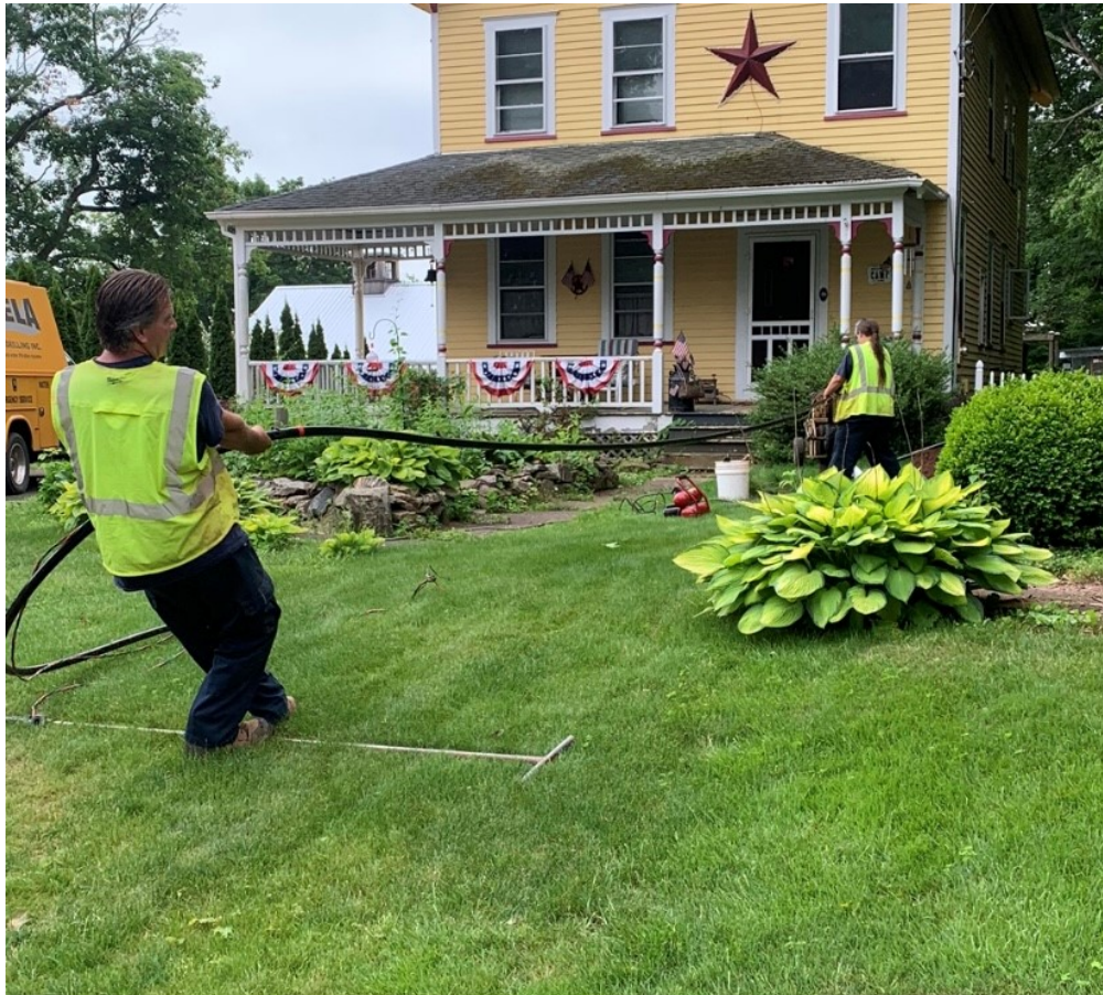
Picture 1: Grela is in the process of pulling out the well piping and pump at 29 Maiden Lane.
