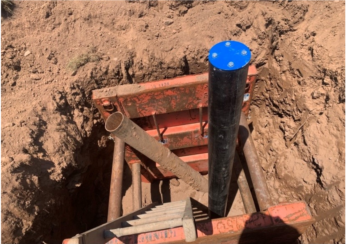
Picture 6: Grela at Mill Pond Road removing a section of the old well casing, and replacing it with a new one but retaining the same well cap.
