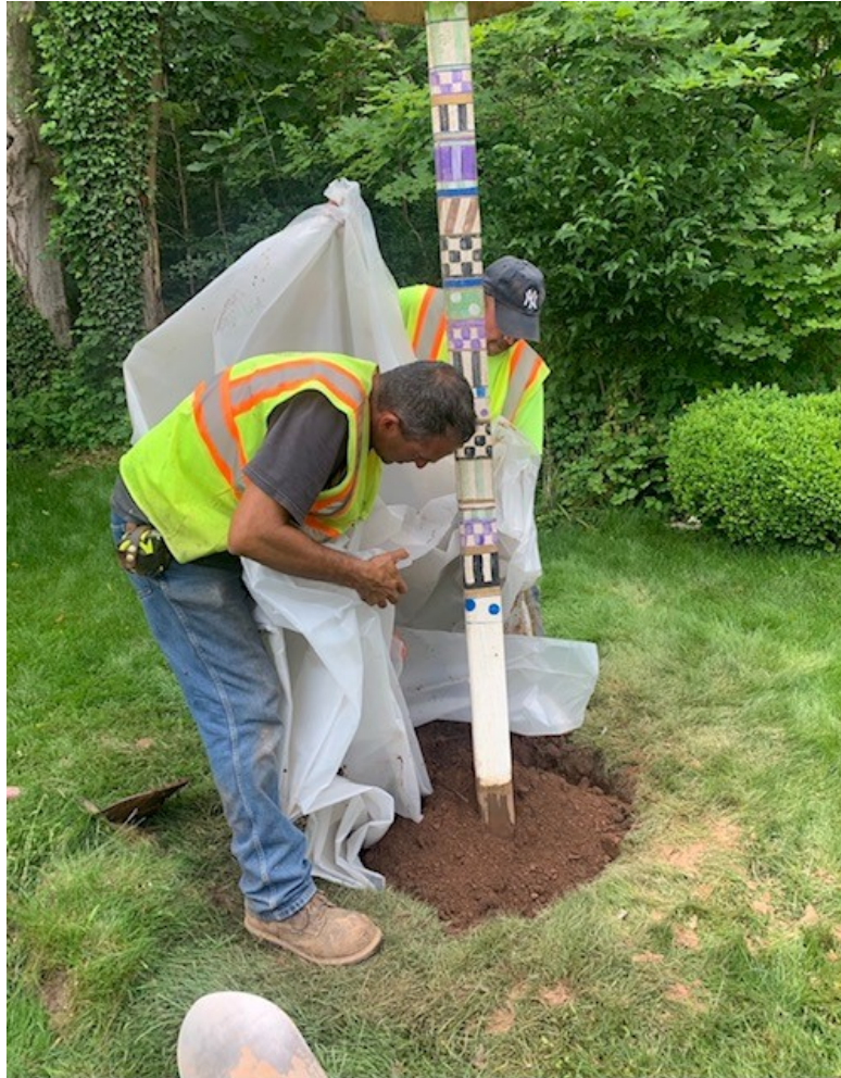
Picture 7: Ludlow at 29 Maiden Lane Backfilling the excavated area, and in the process of fully restoring the area to its previous state.
