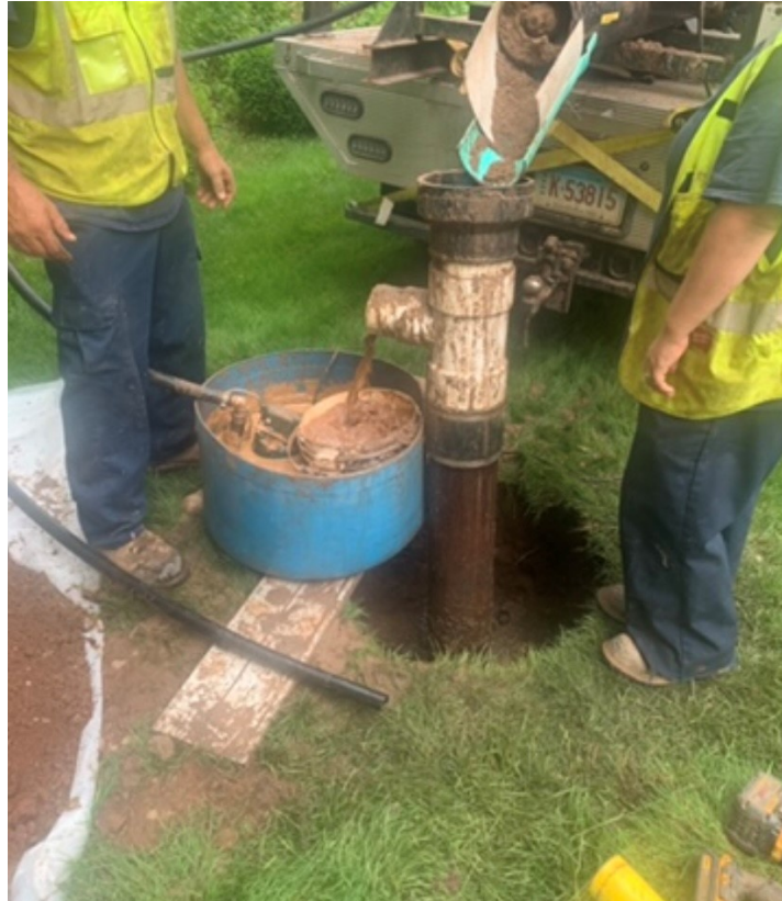
Picture 2: Grela at 29 Maiden Lane filling the well with sand, and then bentonite clay to fully decommission the well.
