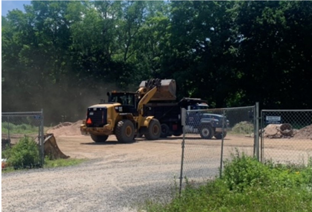
Picture 5: Ludlow loading topsoil onto a loading truck to transported to the Talcott Ridge Booster Station.
