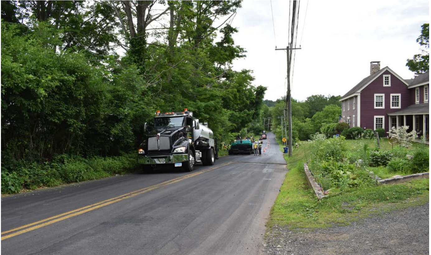
Photo 1: Paving crew adjacent to 35 Maiden Lane. View to the east.
