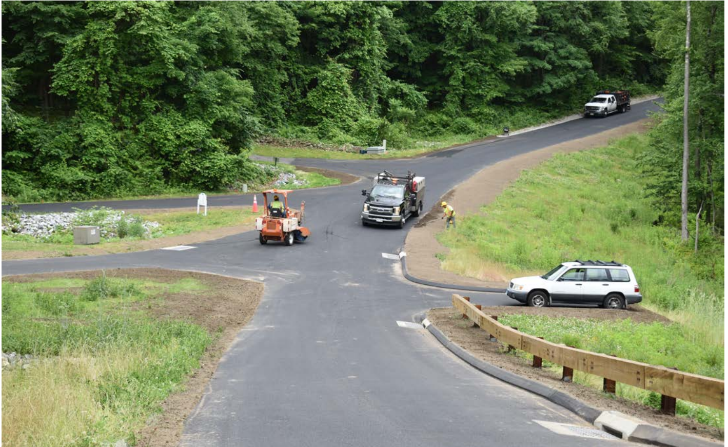
Photo 6: Ludlow crew continuing with loam and seed on Shared Access Driveway. View to the west.
