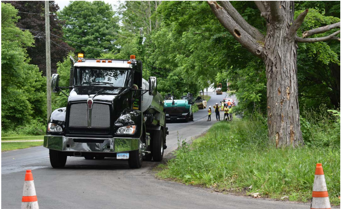
Photo 7: Paving crew on Talcott Lane. View to the east.
