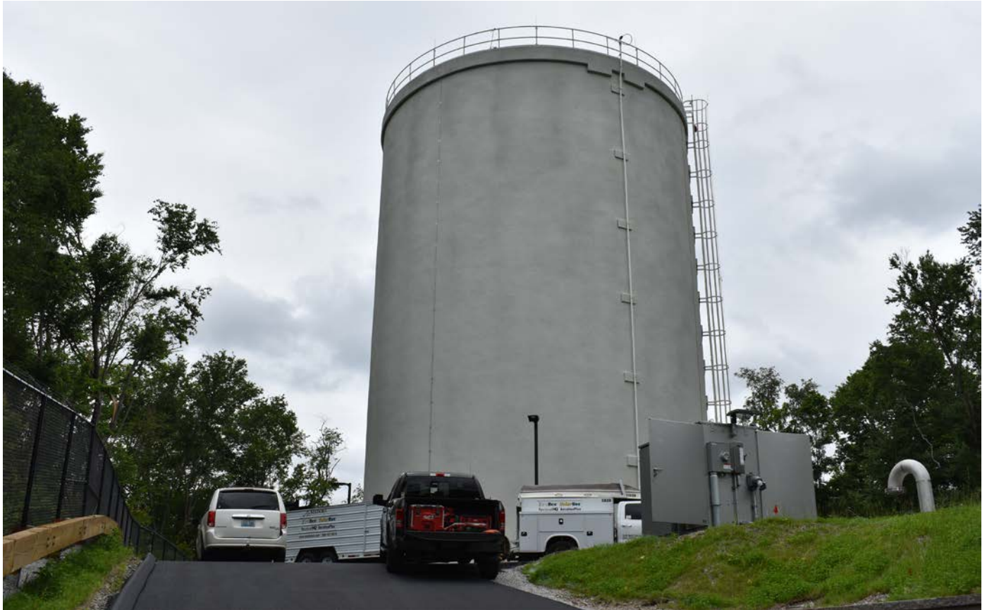
Photo 5: Tank area after completion of lifting work. View to the east.
