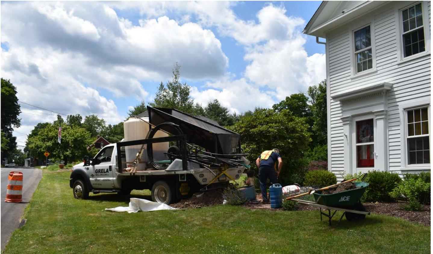
Photo 1: Grela Well Drilling filling well casing at 24 Maiden Lane with sand. View to the northwest.
