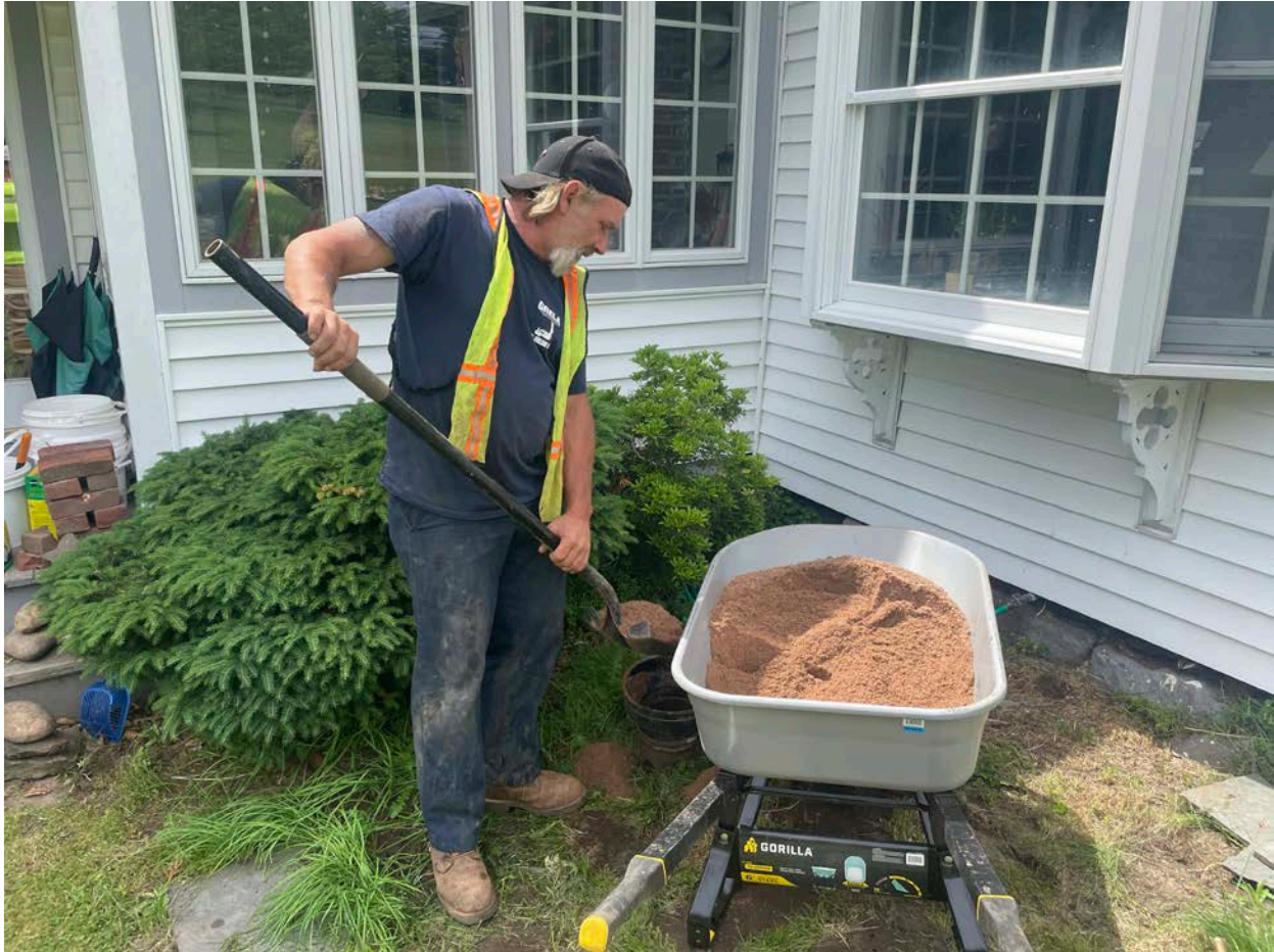
Picture 8: Grela placing sand into the well located on the east side of the 146 Maple Avenue, Durham, residence as part of well decommissioning activities. View to the northwest.
