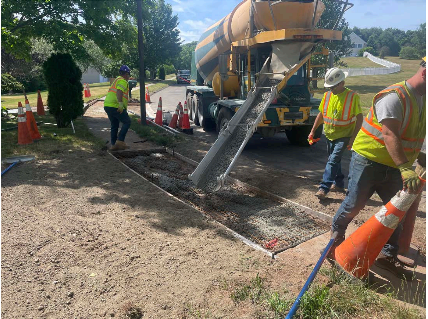
Picture 9: Ludlow placing concrete to repair the sidewalk located at Station 40+41, which was disturbed when Ludlow connected the 12" DIP water line running up from Round Hill Road to the 16" waterline located on Talcott Ridge Drive. View to the southwest.
