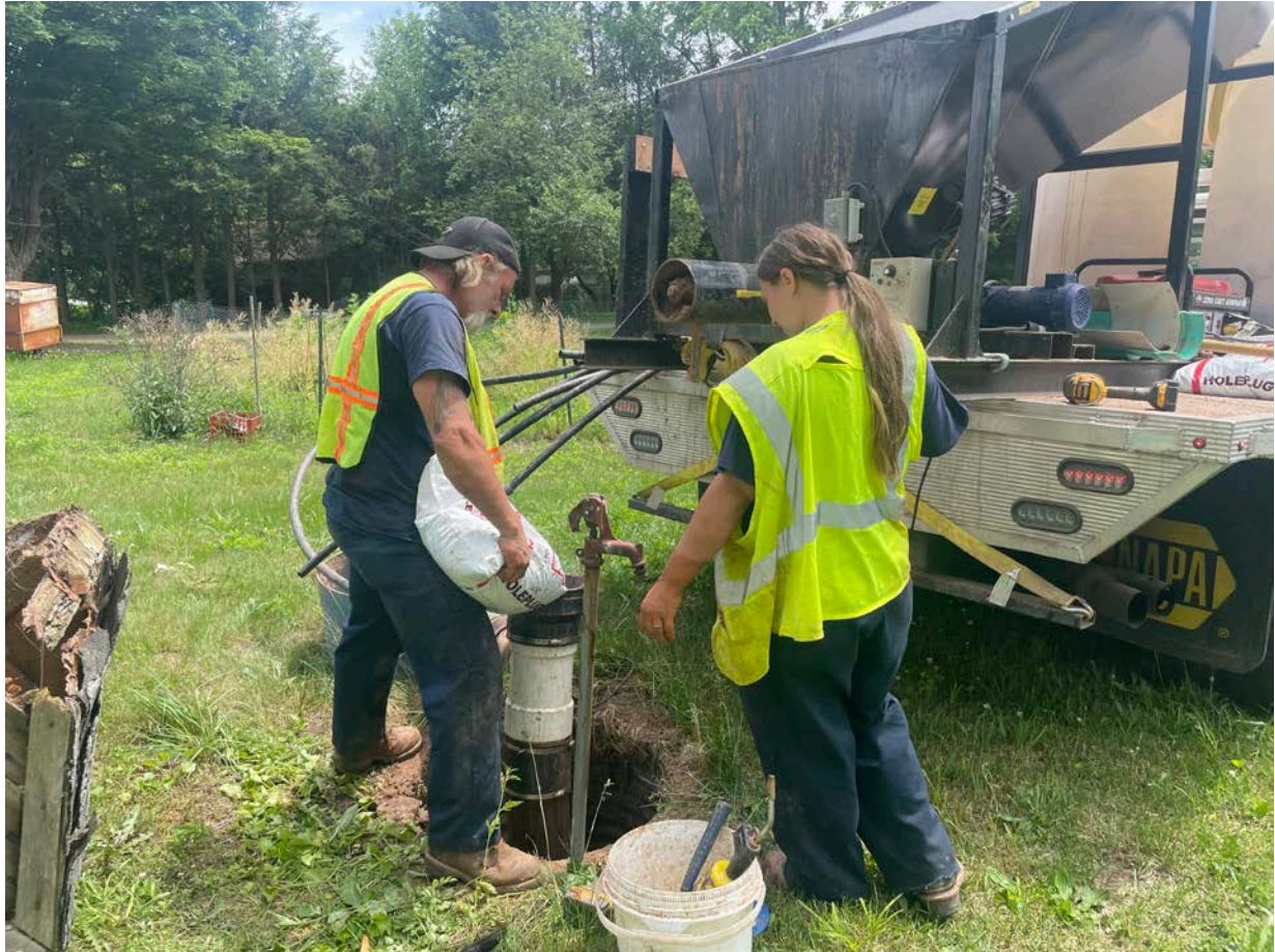
Picture 7: Grela placing bentonite chips over the sand that was placed into the well located on the west side of the 230 Maple Avenue, Durham, property as part of well decommissioning activities. View to the west.
