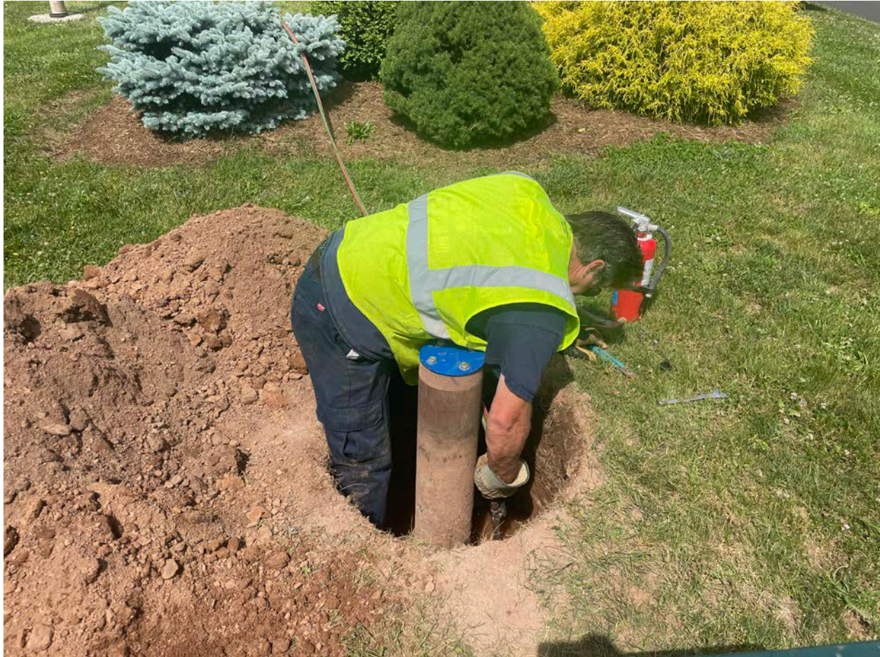
Picture 3: Grela cutting the 6" steel well casing of the easternmost well located on the 38 Town House Road property in Durham as part of well decommissioning activities. View to the west.
