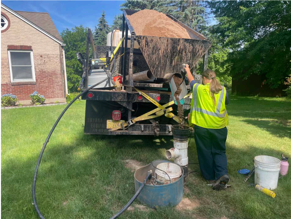
Picture 1: Grela placing sand into the well located on the east side of the 188 Maple Avenue, Durham, residence as part of well decommissioning activities. View to the west.
