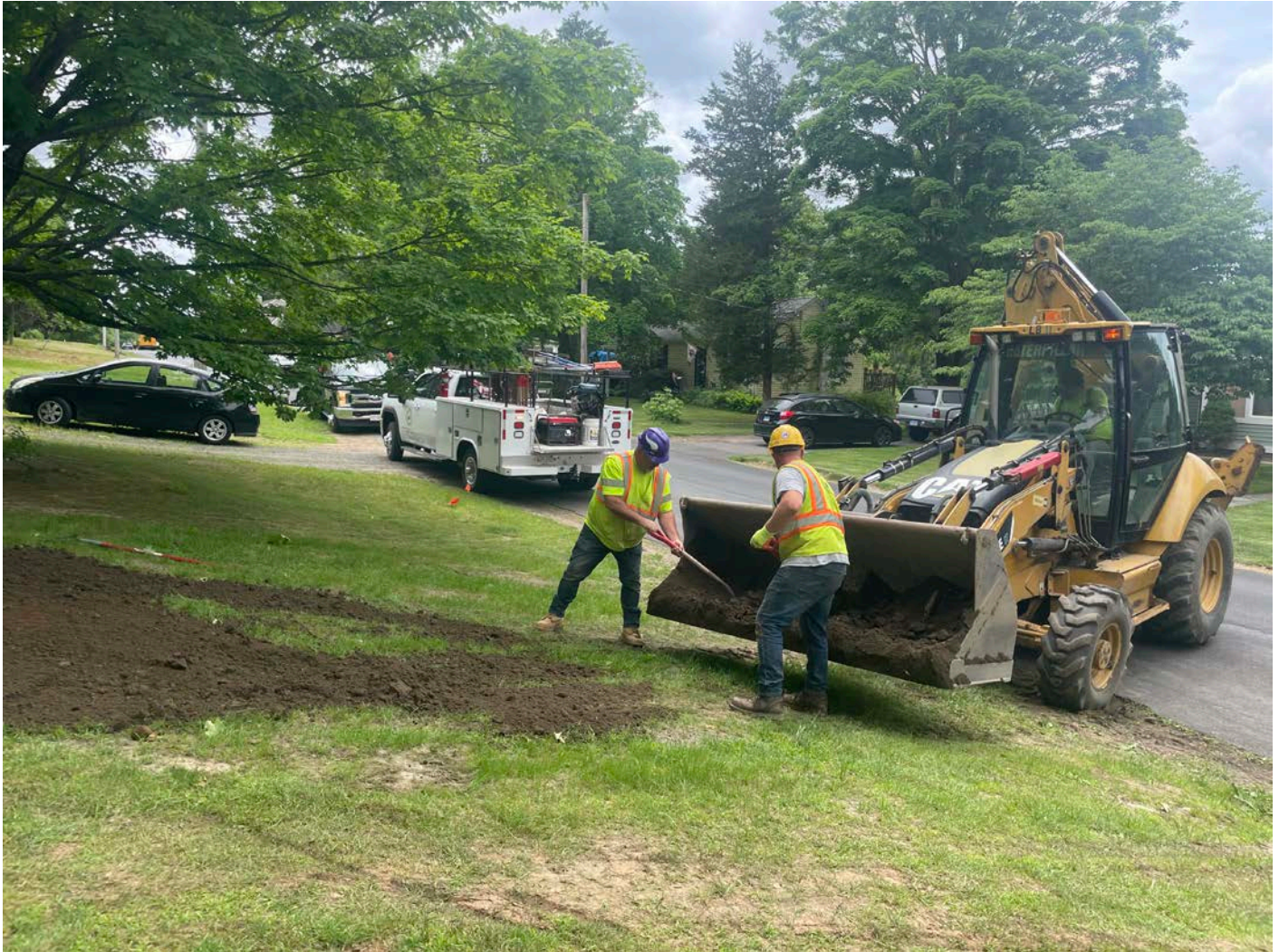
Picture 14: Ludlow placing loam on the 187 Maple Avenue property after they backfilled the hole left after Grela decommissioned the property's well. View to the southwest.
