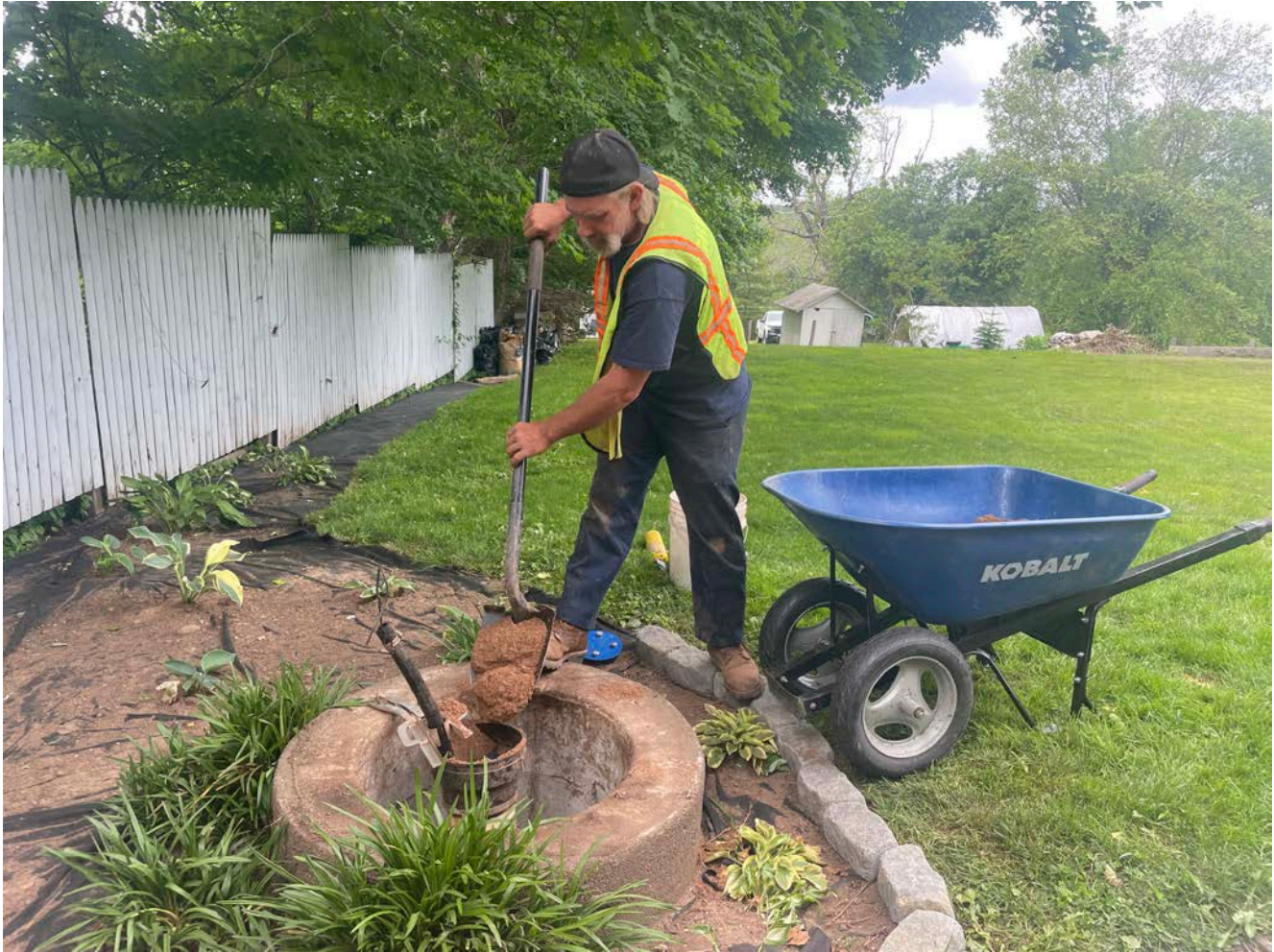
Picture 5: Grela placing sand into the well located on the west side of the 158 Maple Avenue, Durham, residence as part of well decommissioning activities. View to the west.
