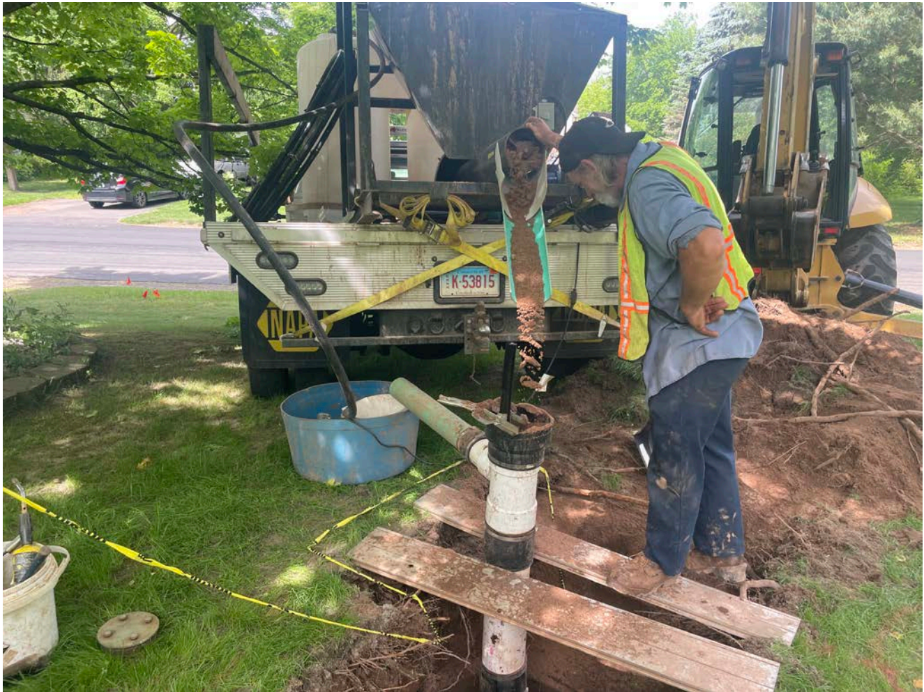
Picture 2: Grela placing sand into the well located on the west side of the 187 Maple Avenue, Durham, residence as part of well decommissioning activities. View to the west.
