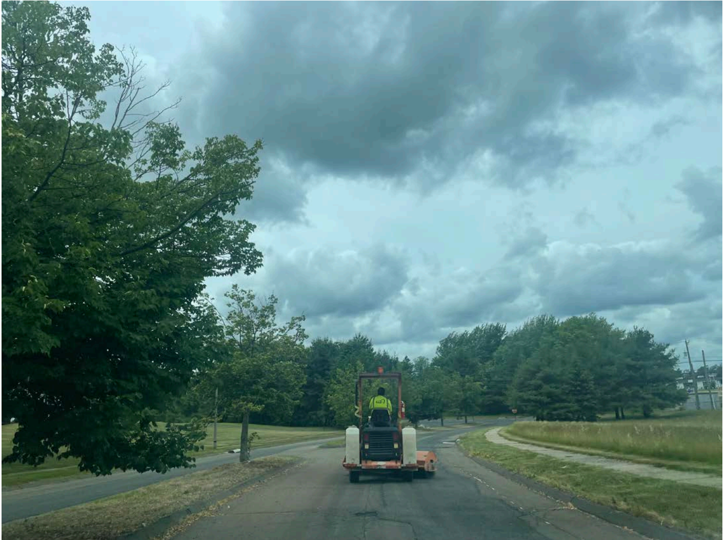
Picture 13: Ludlow cleaning the westbound lane of Talcott Ridge Drive with a Broce Broom. View to the west.
