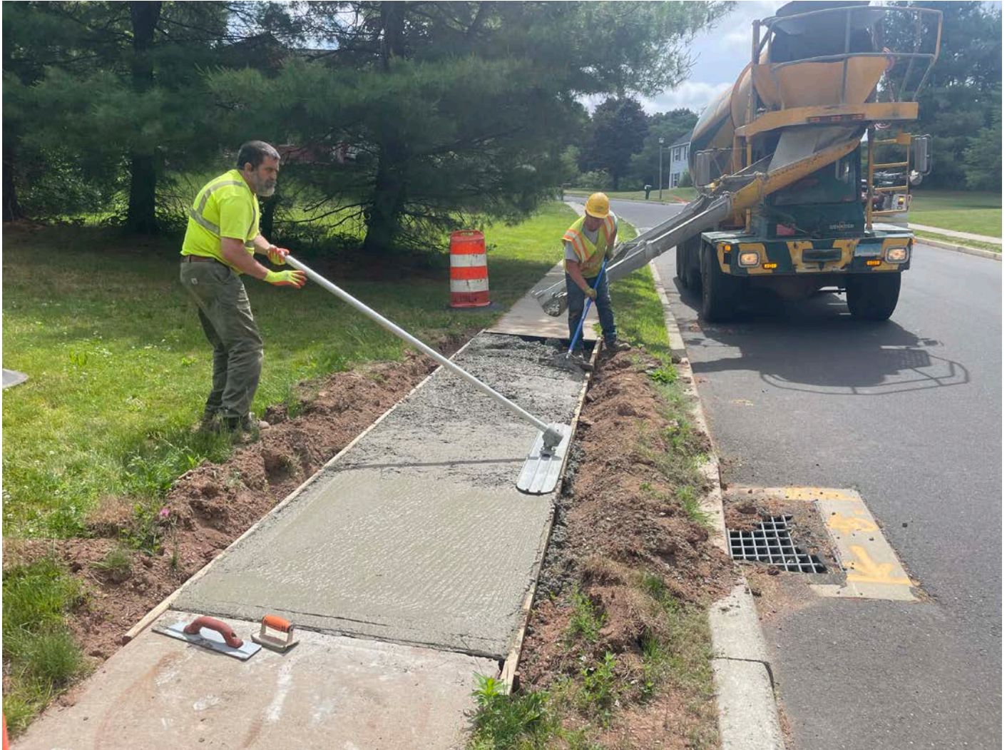
Picture 12: Ludlow using a bull float to level the concrete they are placing on the north side of Acorn Drive in Middletown as they repair a sidewalk they previously damaged while working on the construction of the Water Meter Building. View to the east.
