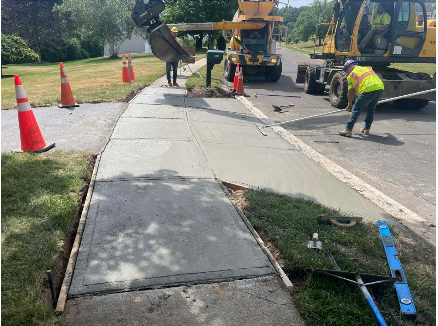
Picture 11: Ludlow using a float to smooth the surface of the concrete they just placed on the footprint of the driveway apron for the 124 Talcott Ridge Drive property. View to the south.
