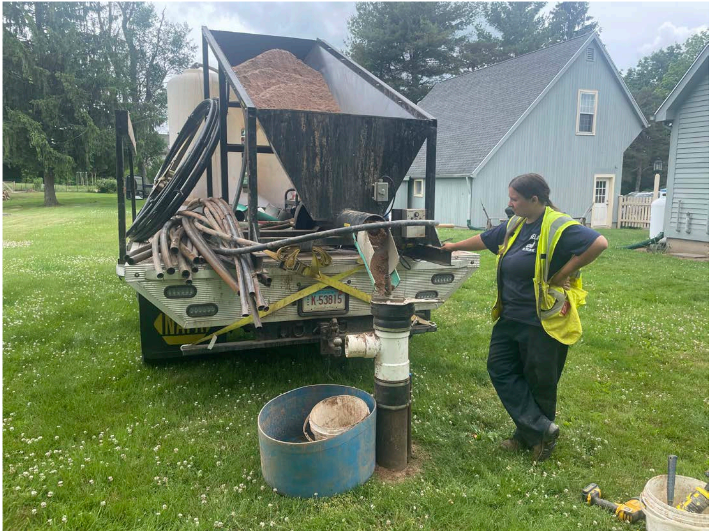
Picture 6: Grela placing sand into the well located on the east side of the 109 Maple Avenue, Durham, residence as part of well decommissioning activities. View to the south.
