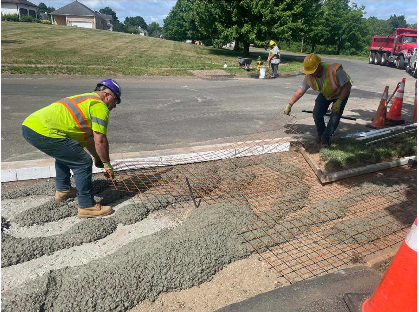
Picture 10: Ludlow placing 4" steel mesh on the footprint of the driveway apron for the 124 Talcott Ridge Drive property as concrete is being poured. View to the west.
