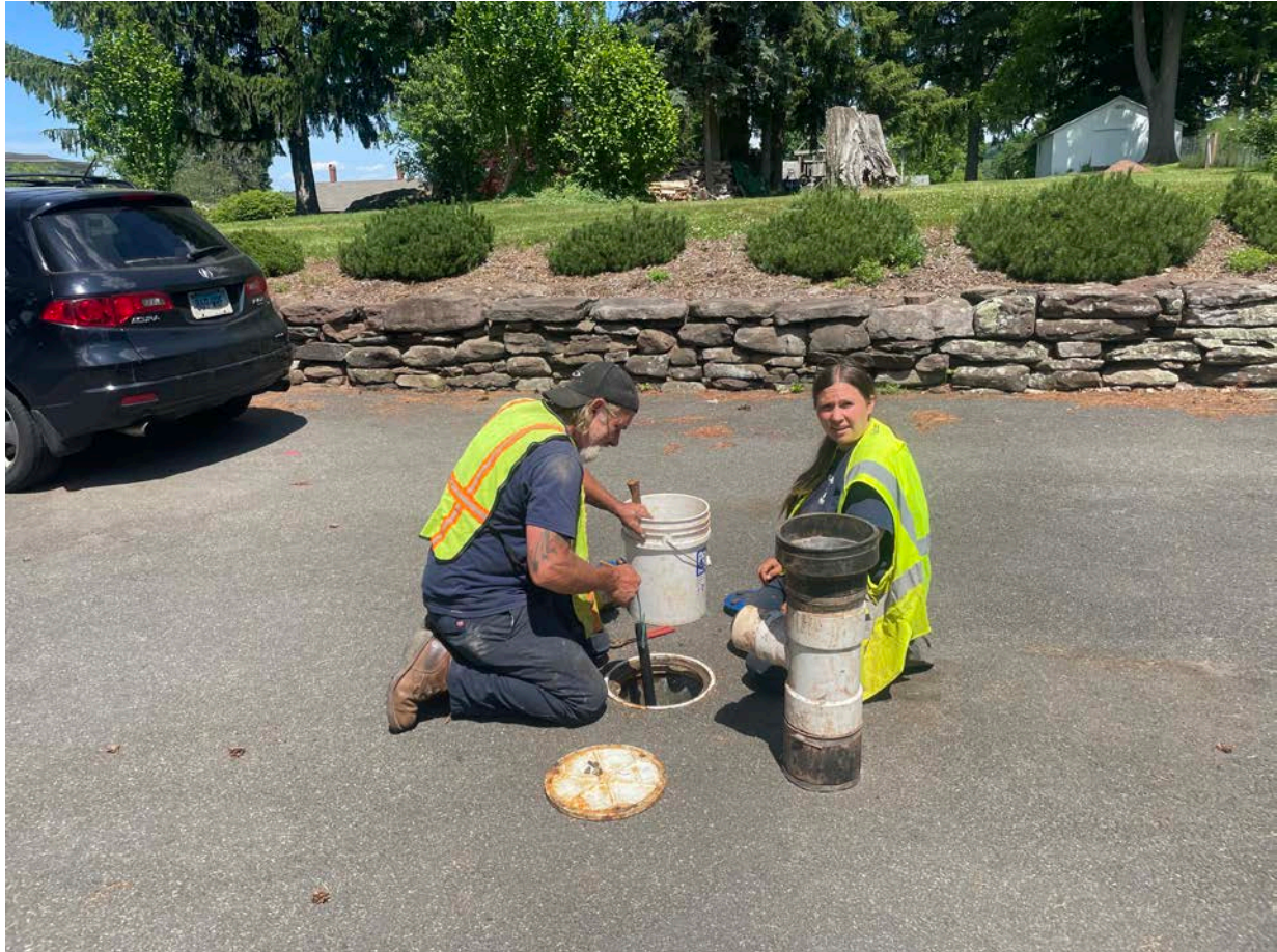
Picture 9: Grela preparing to sand into the well located to the northeast of the 95R Maple Avenue, Durham, residence as part of well decommissioning activities. View to the southeast.
