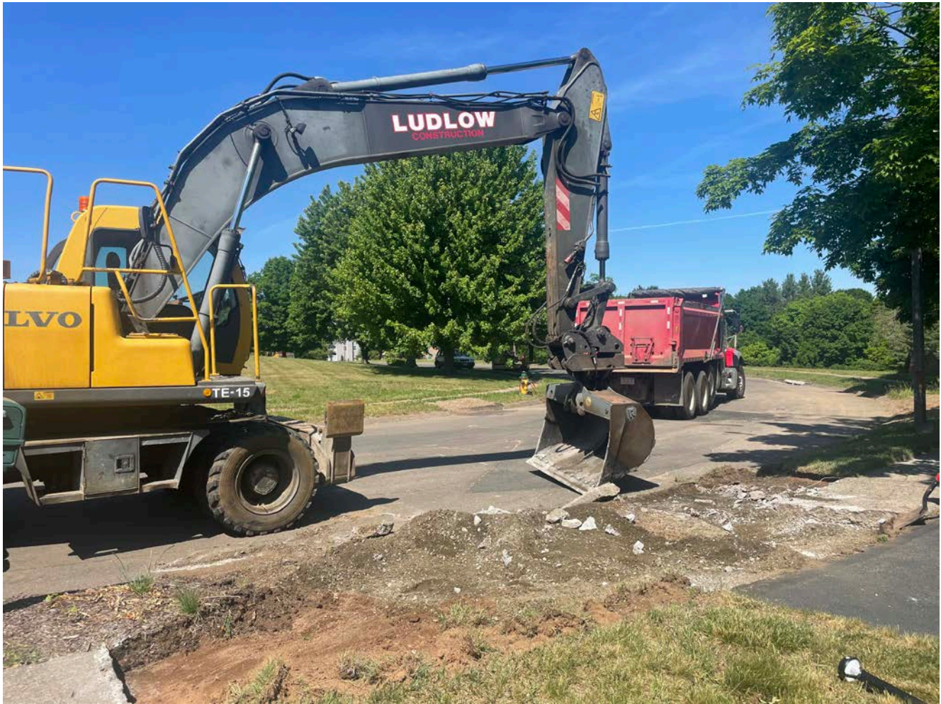
Picture 5: Ludlow using an excavator to remove concrete from the driveway apron of the 124 Talcott Ridge Drive property. View to the northwest.
