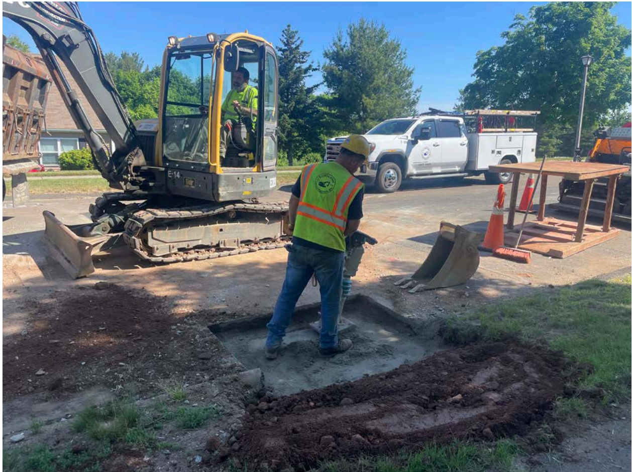
Picture 3: Ludlow compacting fill after realigning the road box located at Station ~44+12 on Talcott Ridge Drive. View to the north.
