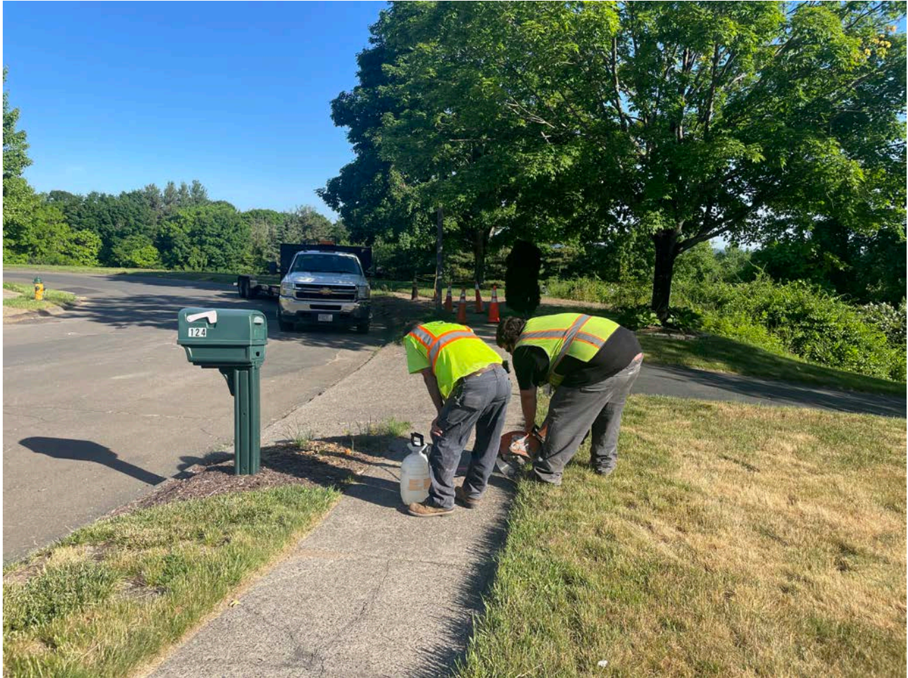
Picture 2: Ludlow saw cutting the concrete apron of the 124 Talcott Ridge Driveway in Middletown. View to the northwest.
