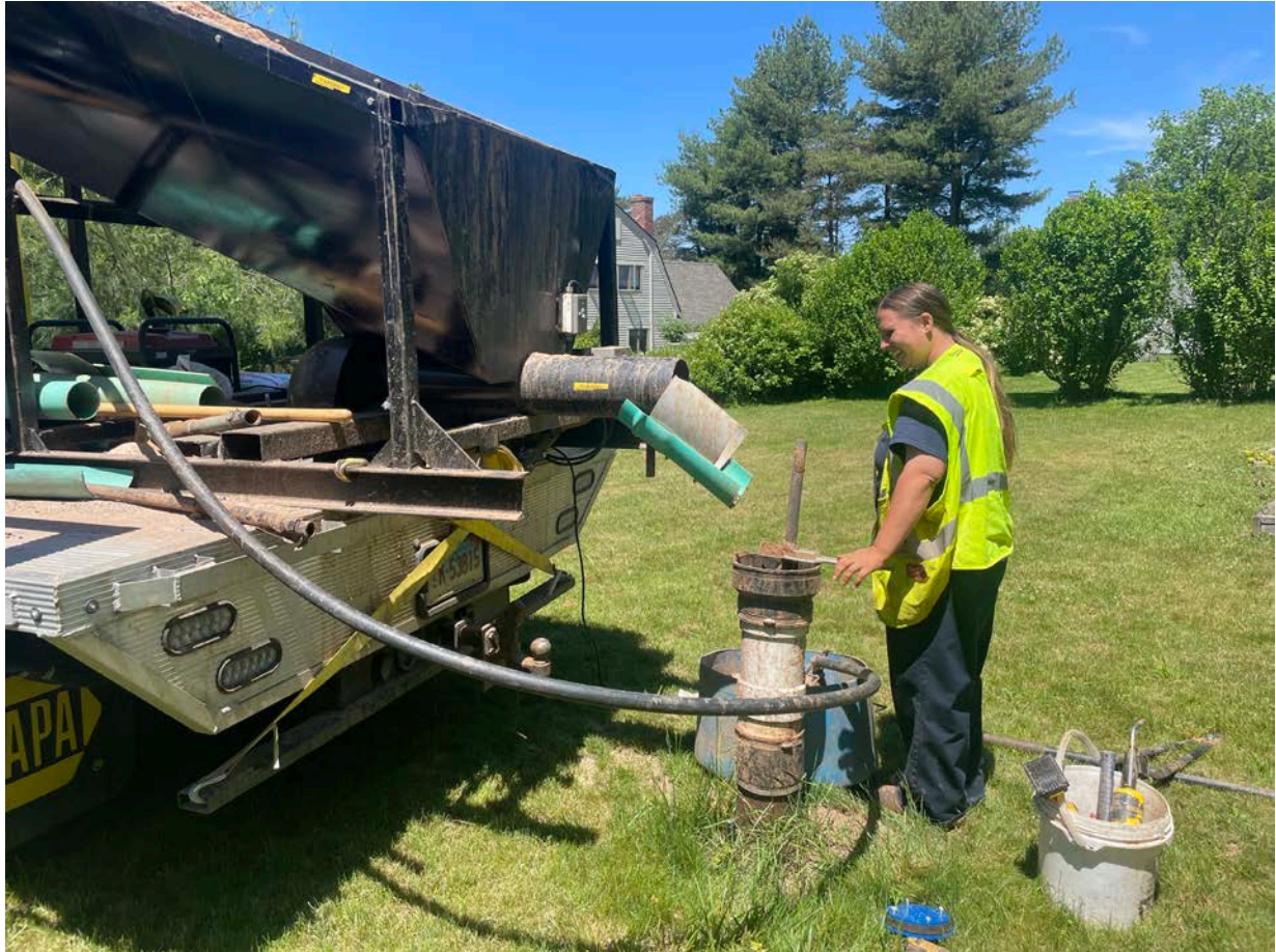
Picture 7: Grela placing sand into the well located on the northeast side of the 95R Maple Avenue, Durham, property as part of well decommissioning activities. View to the northeast.
