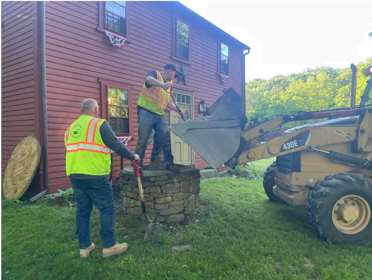
Picture 1: Ludlow filling the remaining void within the well tile at the 153 Main Street, Durham, property with - 3" gravel. View to the southeast.
