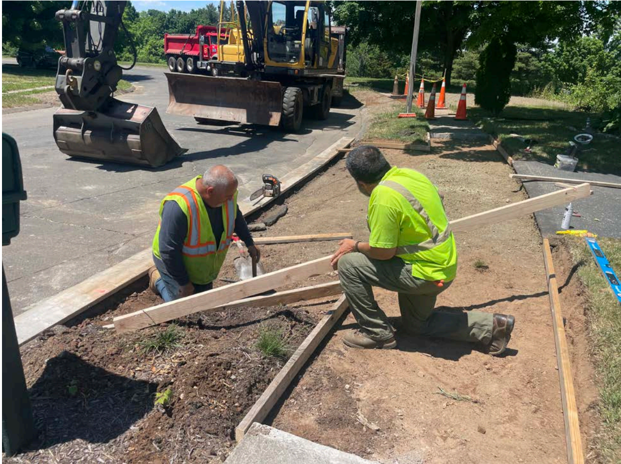
Picture 8: Ludlow constructing a concrete form on the footprint of the apron of the driveway for the 124 Talcott Ridge Drive property. View to the northwest.
