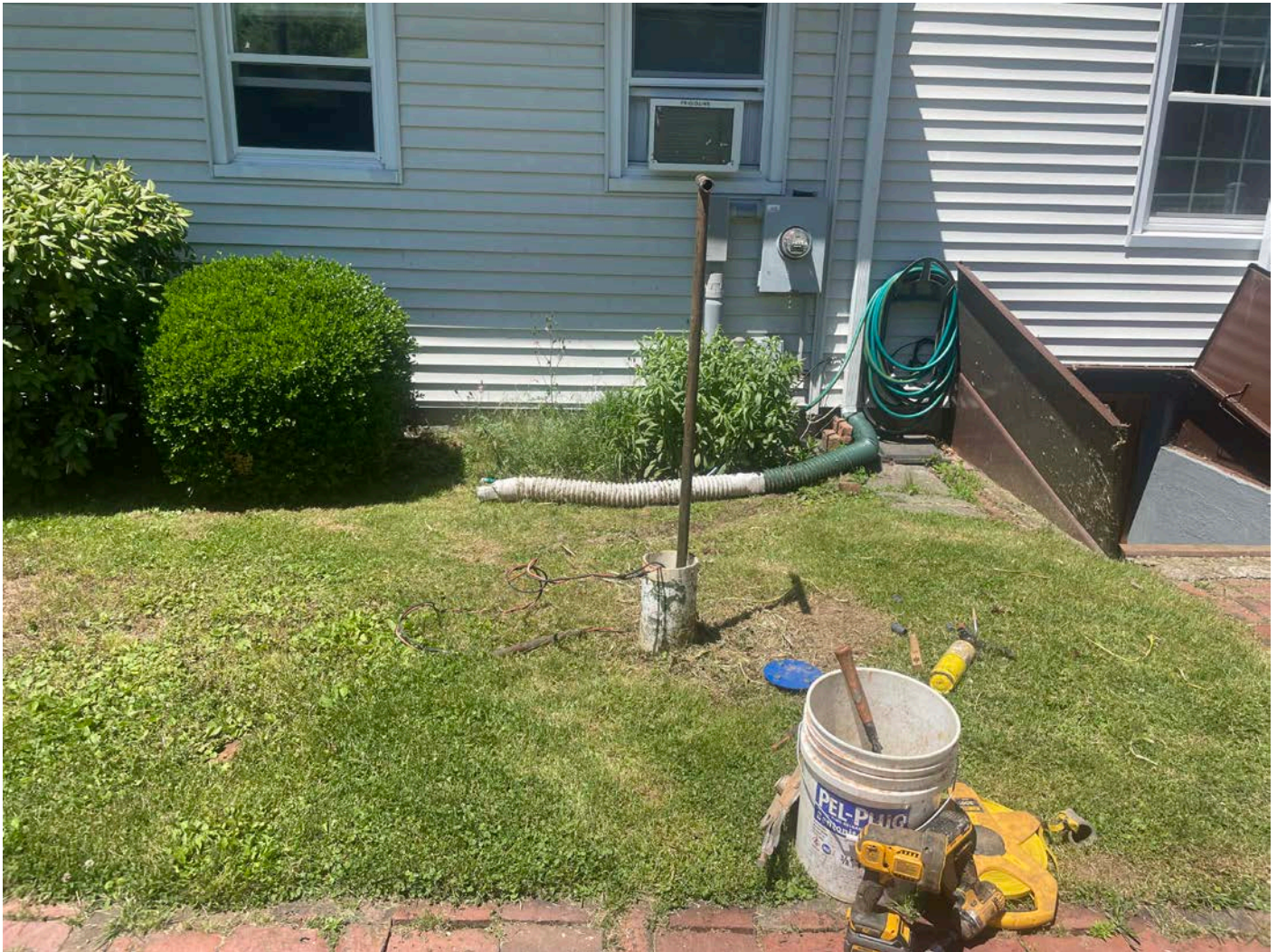
Picture 6: The well located on the east side of the 41 Maple Avenue, Durham, residence where Grela is preparing to pull the pump from the well and then fill it with sand and bentonite as part of well decommissioning activities. View to the west.
