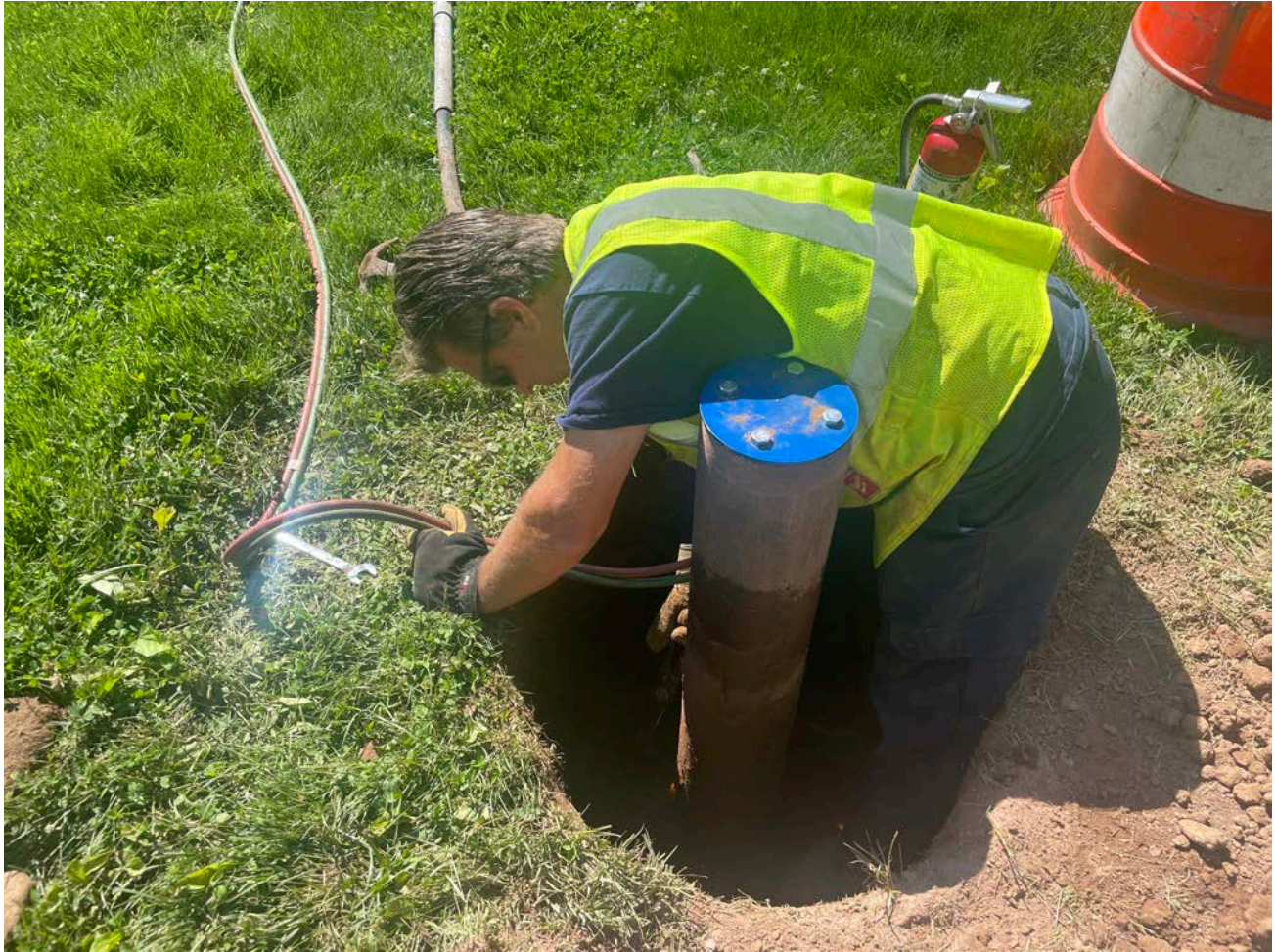
Picture 4: Grela cutting the 6” steel well casing located on the northeast corner of the 172 Maple Avenue, Durham, property as part of well decommissioning activities. View to the southeast.
