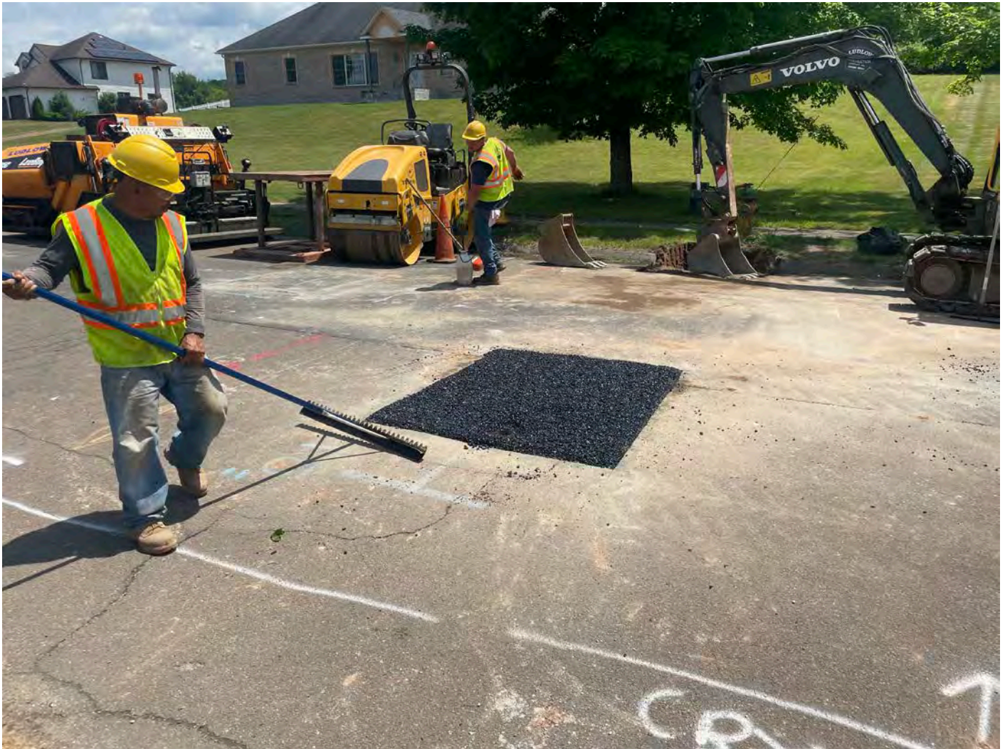
Picture 13: Ludlow placing asphalt over the backfilled excavation they made in order to realign the roadbox located at Station 44+64 on Talcott Ridge Drive.
