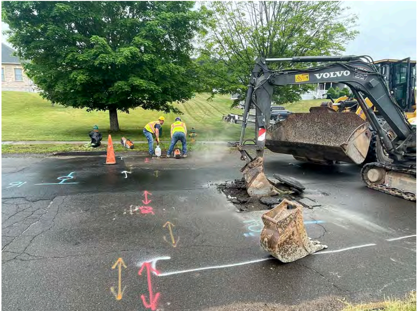
Picture 6: Ludlow excavating to realign a road box on the north side of Talcott Ridge Drive at Station 44+53. View to the south.
