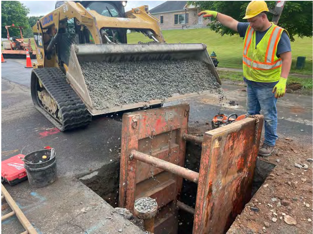
Picture 7: Ludlow placing fill around the road box located on Talcott Ridge Drive at Station 44+64 after they realigned the roadbox. View to the southeast.
