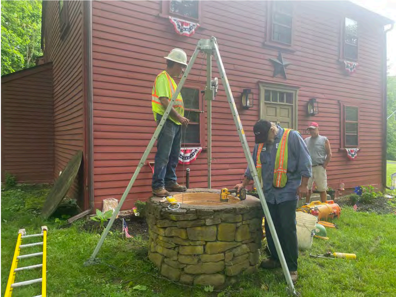
Picture 4: Ludlow and Grela personnel work on confined space standby as another Grela technician works inside of the well tile located on the west side of the 153 Main Street, Durham, residence. View to the southeast.
