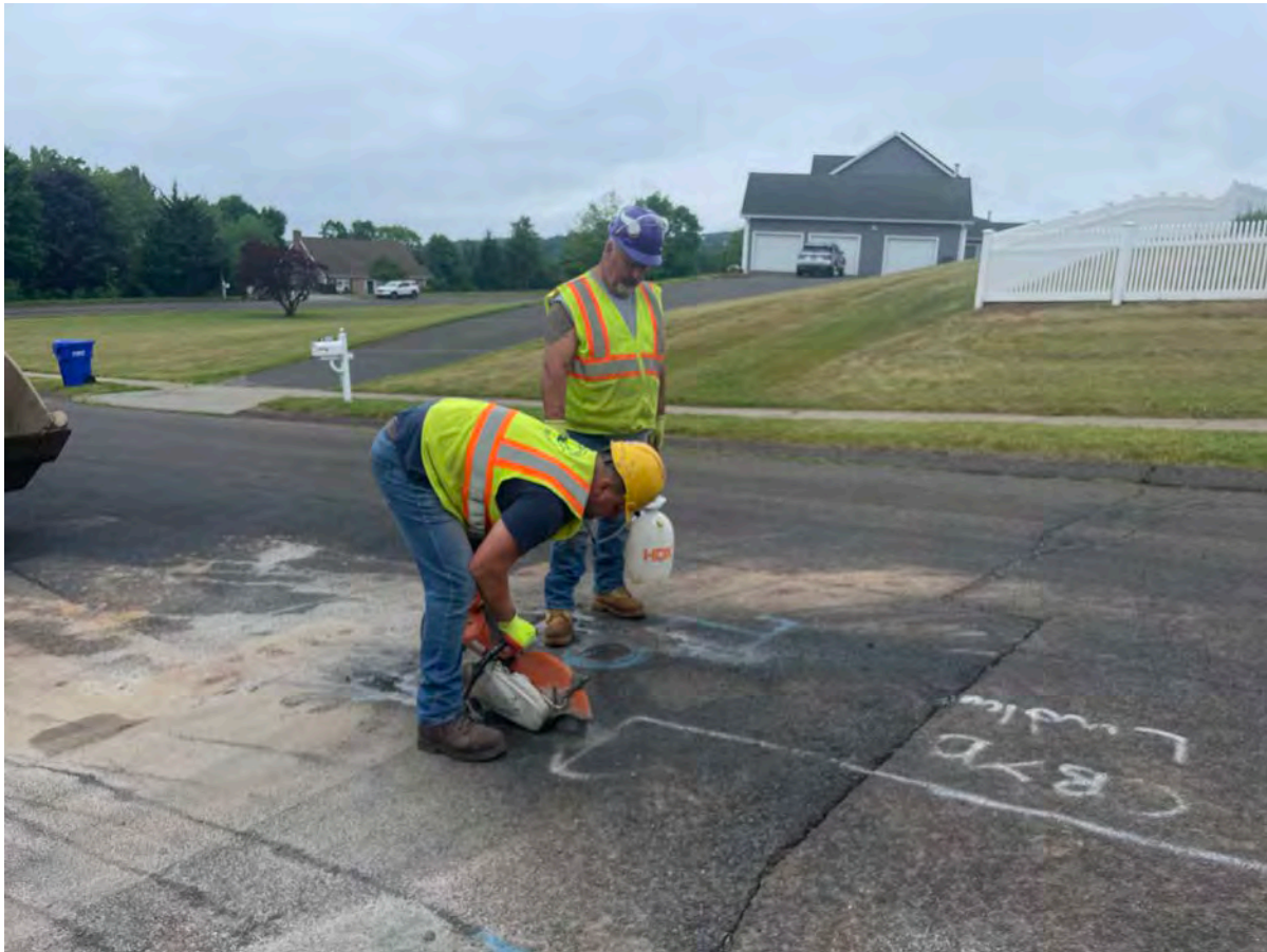
Picture 1: Ludlow saw-cutting around the roadbox located on Watch Hill Drive near Station 607+12 as they prepare to realign it. View to the northeast.
