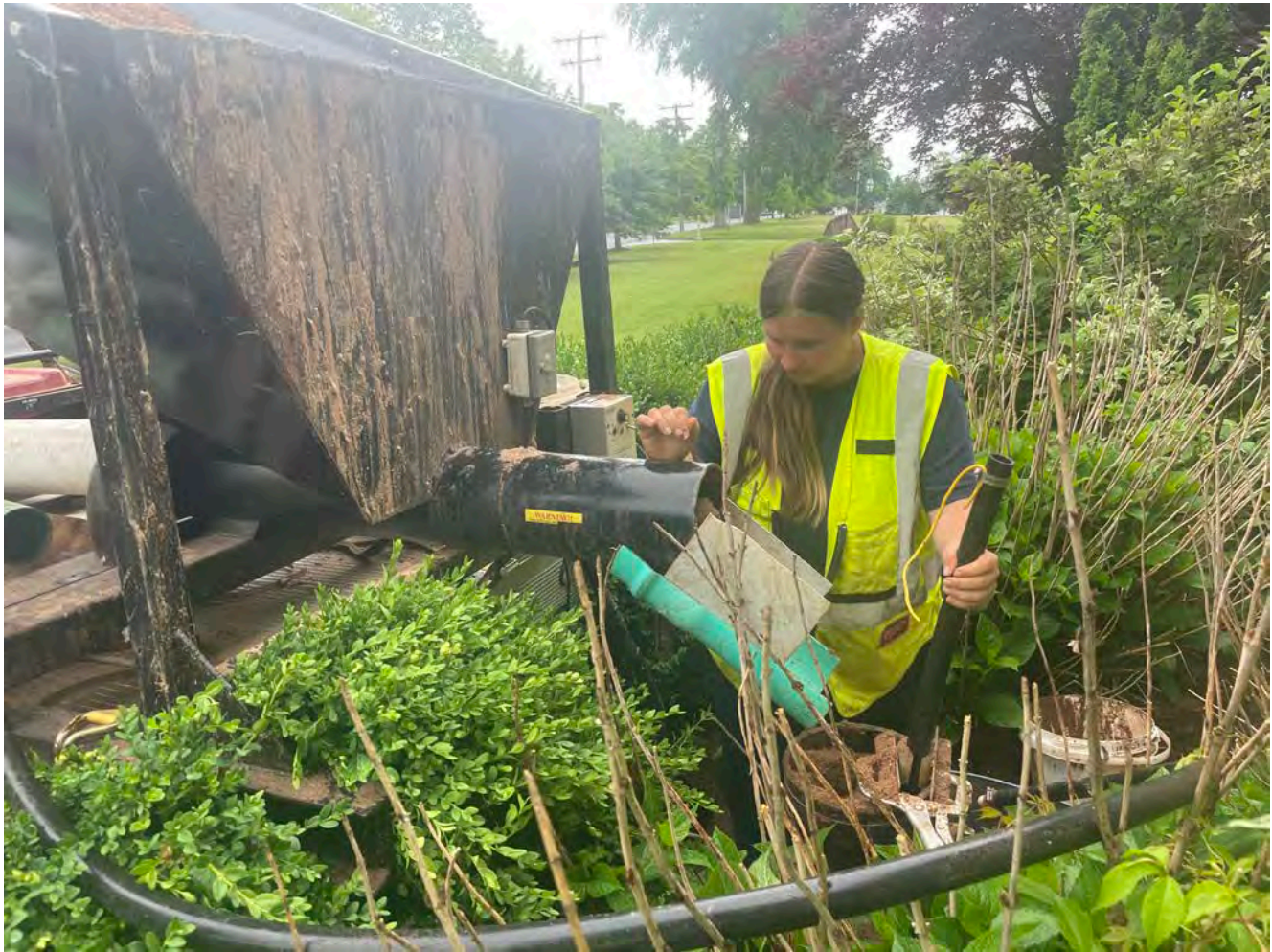
Picture 5: Grela placing sand into the well located on the east side of the 7 Maple Avenue, Durham, property as part of well decommissioning activities. View to the south.
