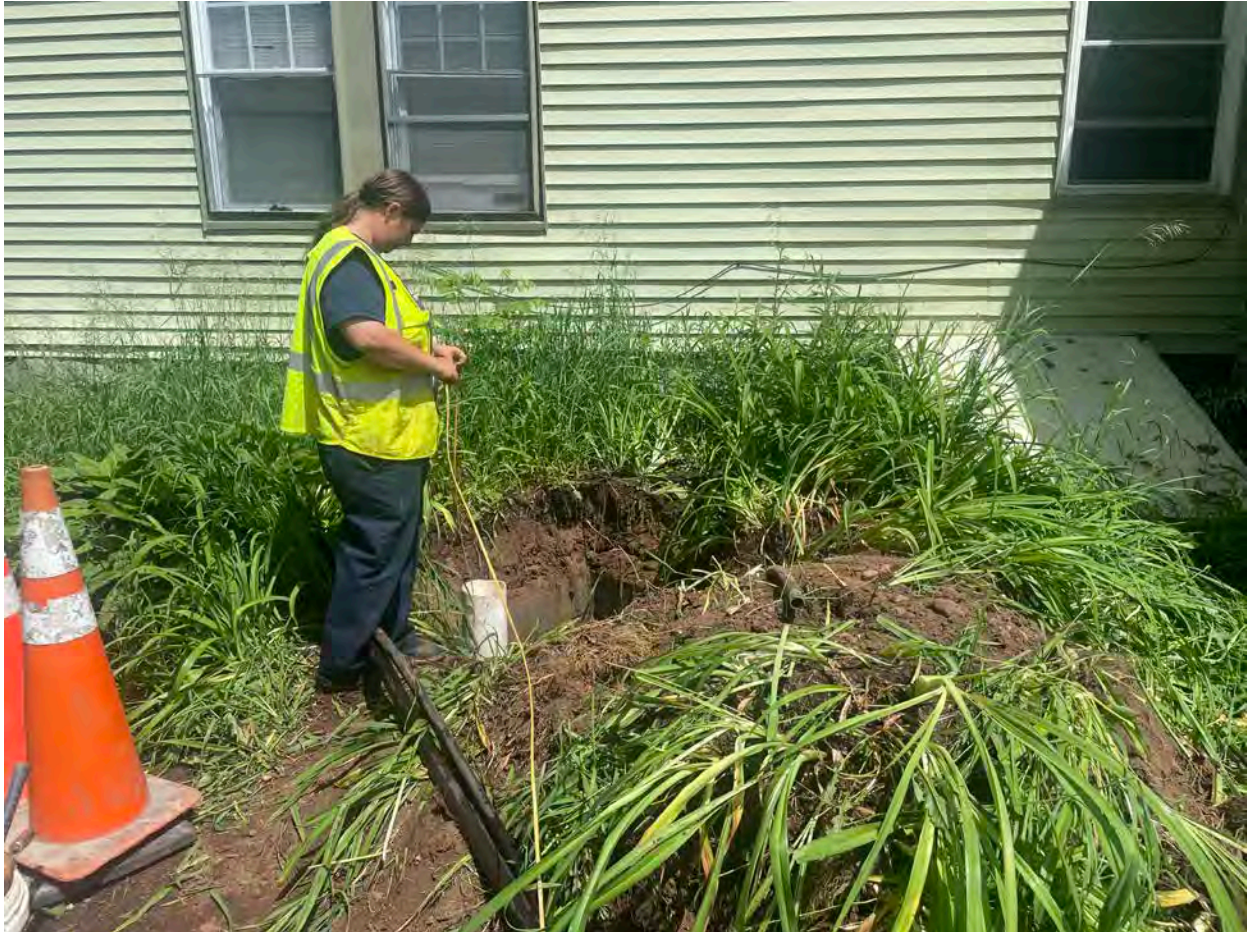
Picture 8: Ludlow collecting well depth data from the (second) well located on the south side of the 176 Main Street residence that they decommissioned. View to the north.
