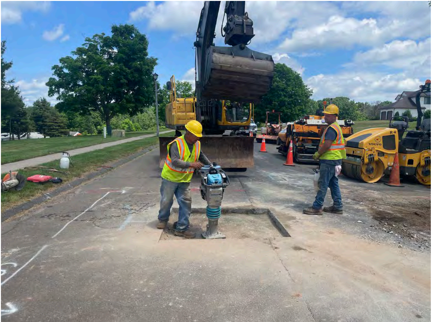
Picture 12: Ludlow compacting backfill at the excavation they made while realigning the roadbox located at Station 44+64 on Talcott Ridge Drive. View to the east.
