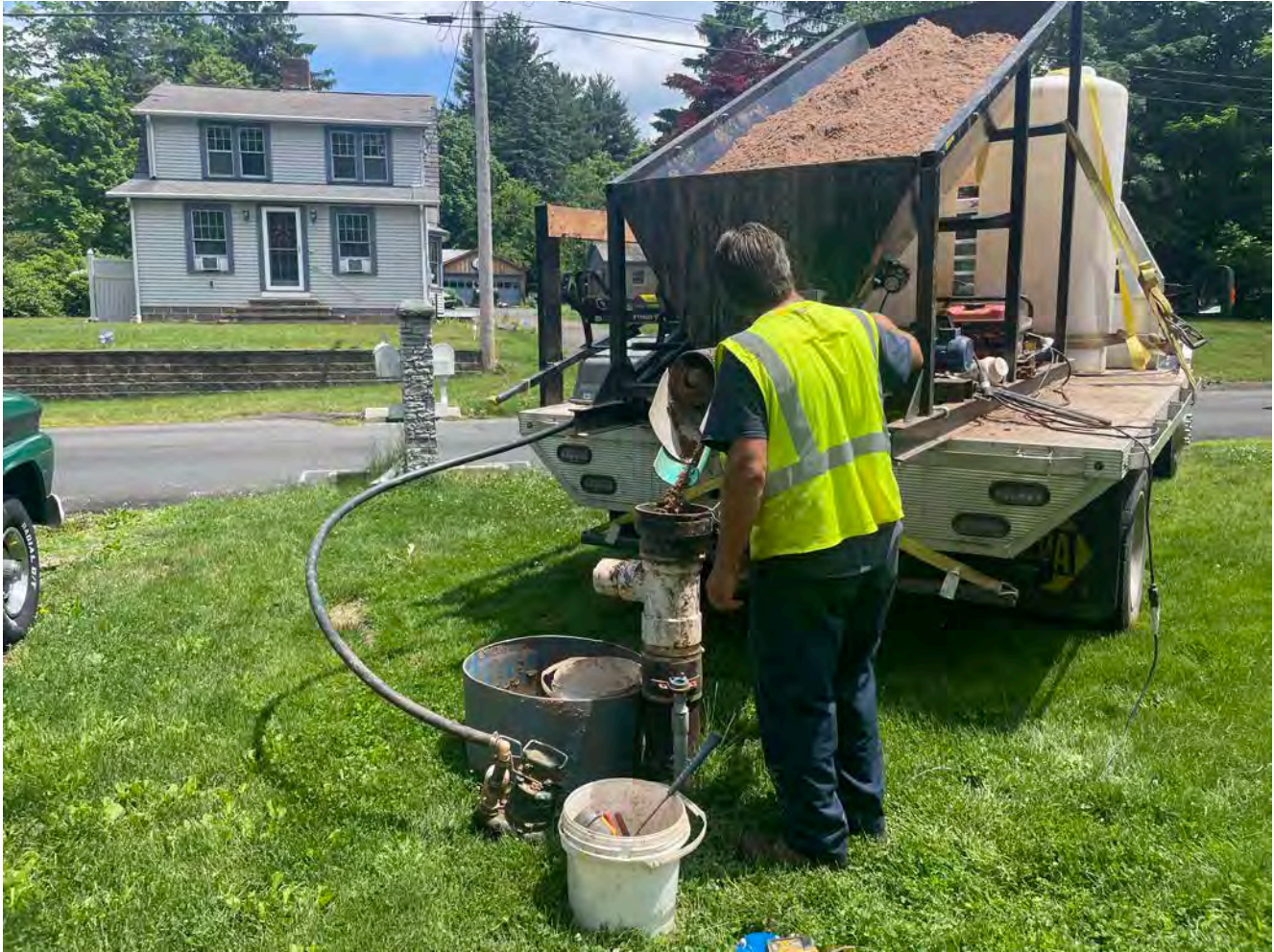
Picture 11: Grela placing sand into the well located on the east side of the 172 Maple Avenue, Durham, property as part of well decommissioning activities. View to the east.
