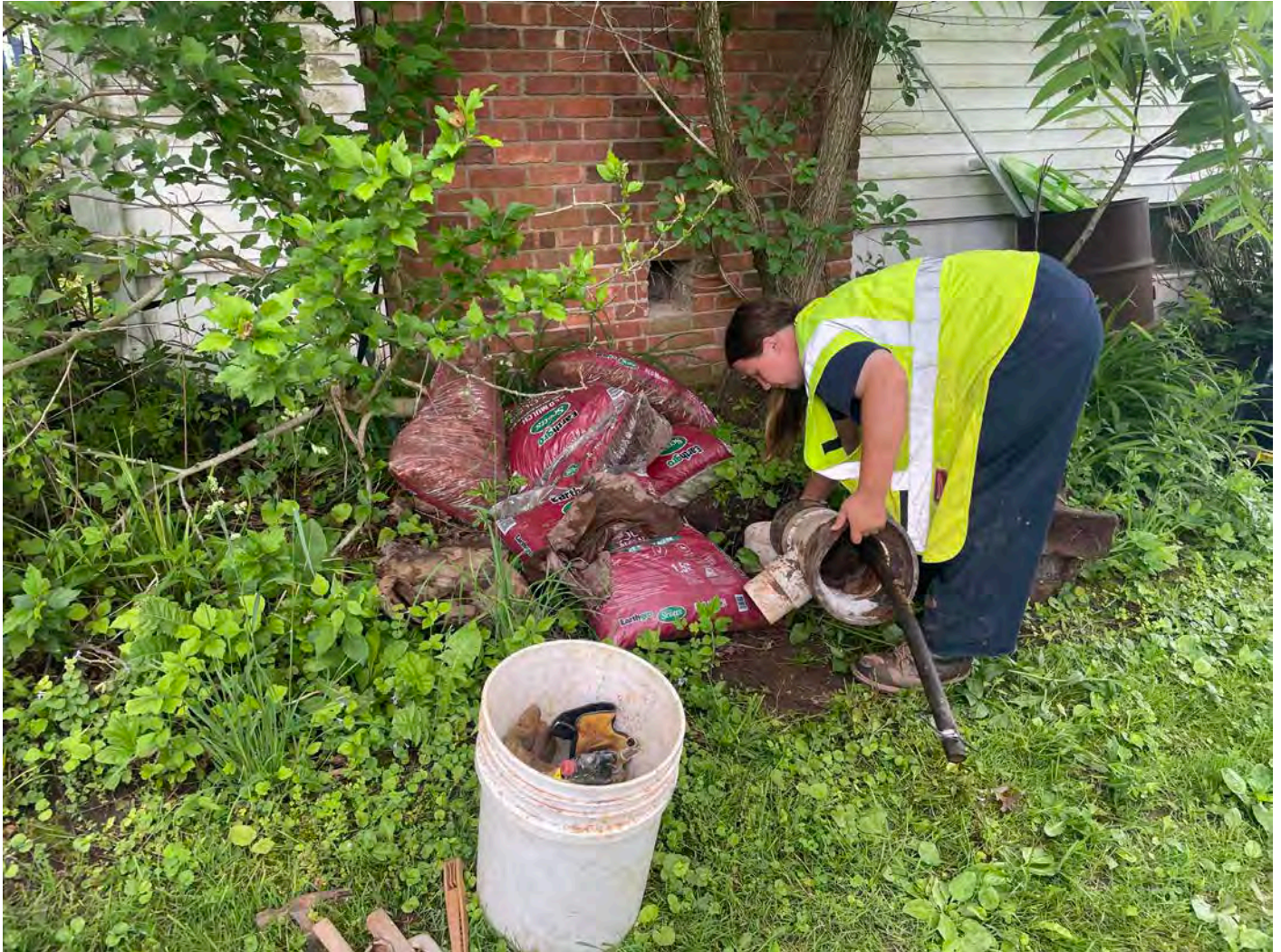
Picture 14: Grela preparing to decommission the well located on the north side of the 162 Maple Avenue, Durham, residence. View to the south.
