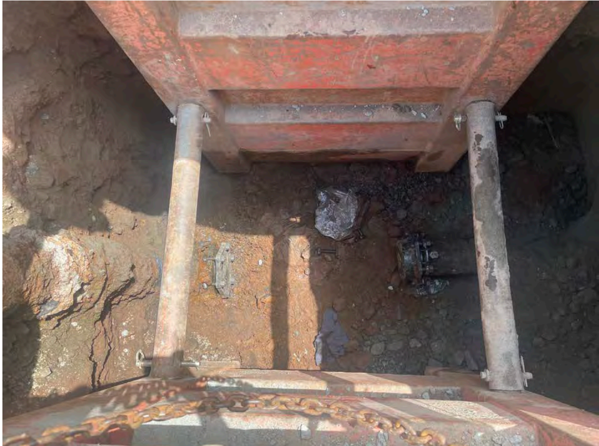
Picture 9: 6" DIP located at Station 44+64 where Ludlow cut the pipe and placed a DIP plug on the cut end of the pipe.
