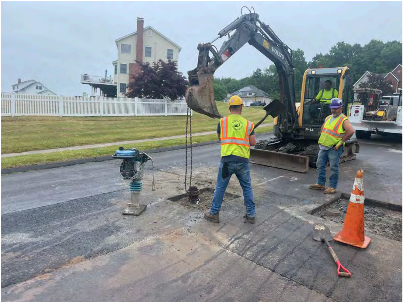
Picture 2: Ludlow in the process of realigning the roadbox located on Watch Hill Drive at Station 607+12. View to the southeast.
