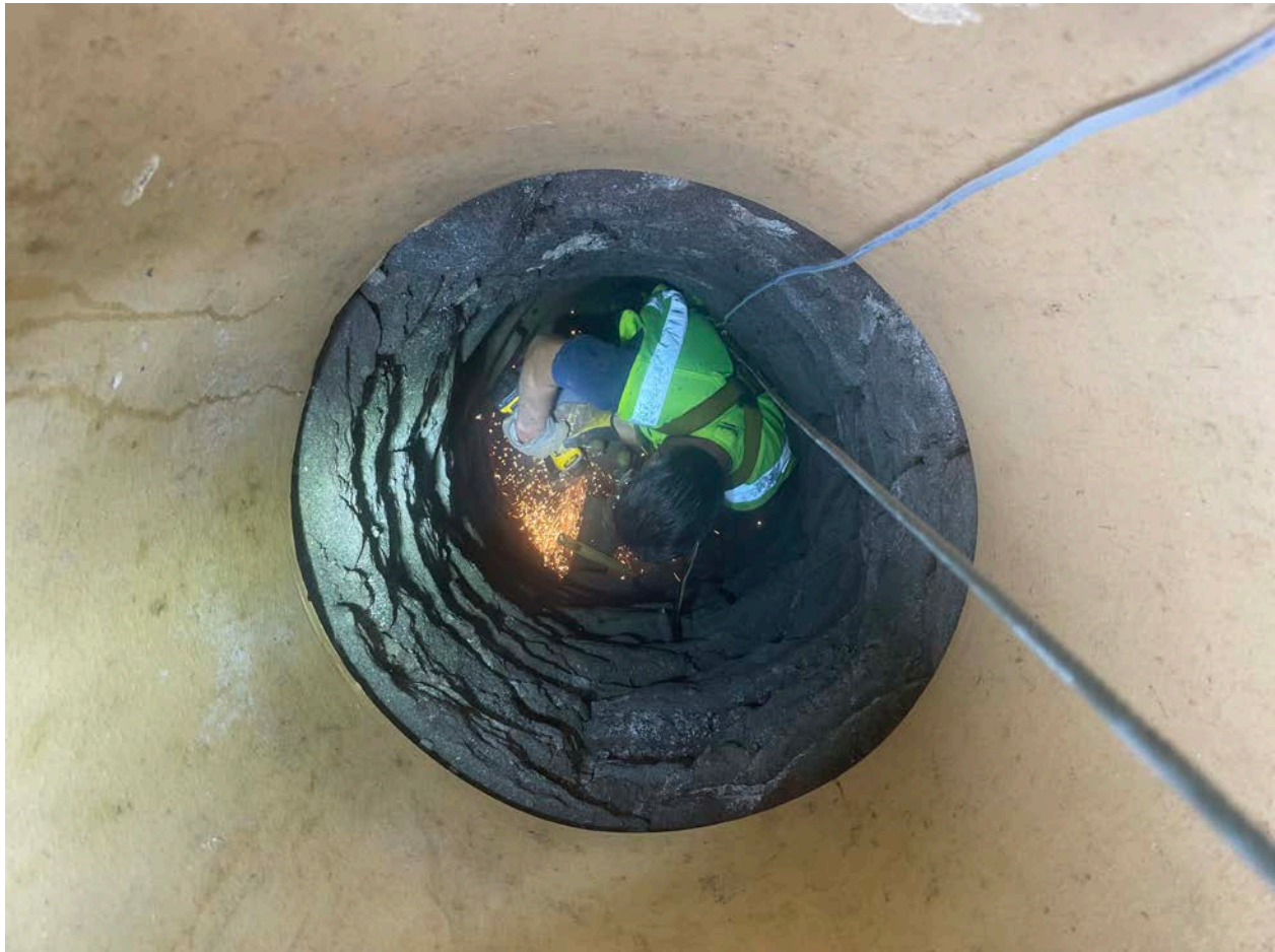
Picture 3: Grela cutting the well head off of the well casing inside of the well tile on the west side of the 153 Main Street, Durham, property as part of well decommissioning activities.
