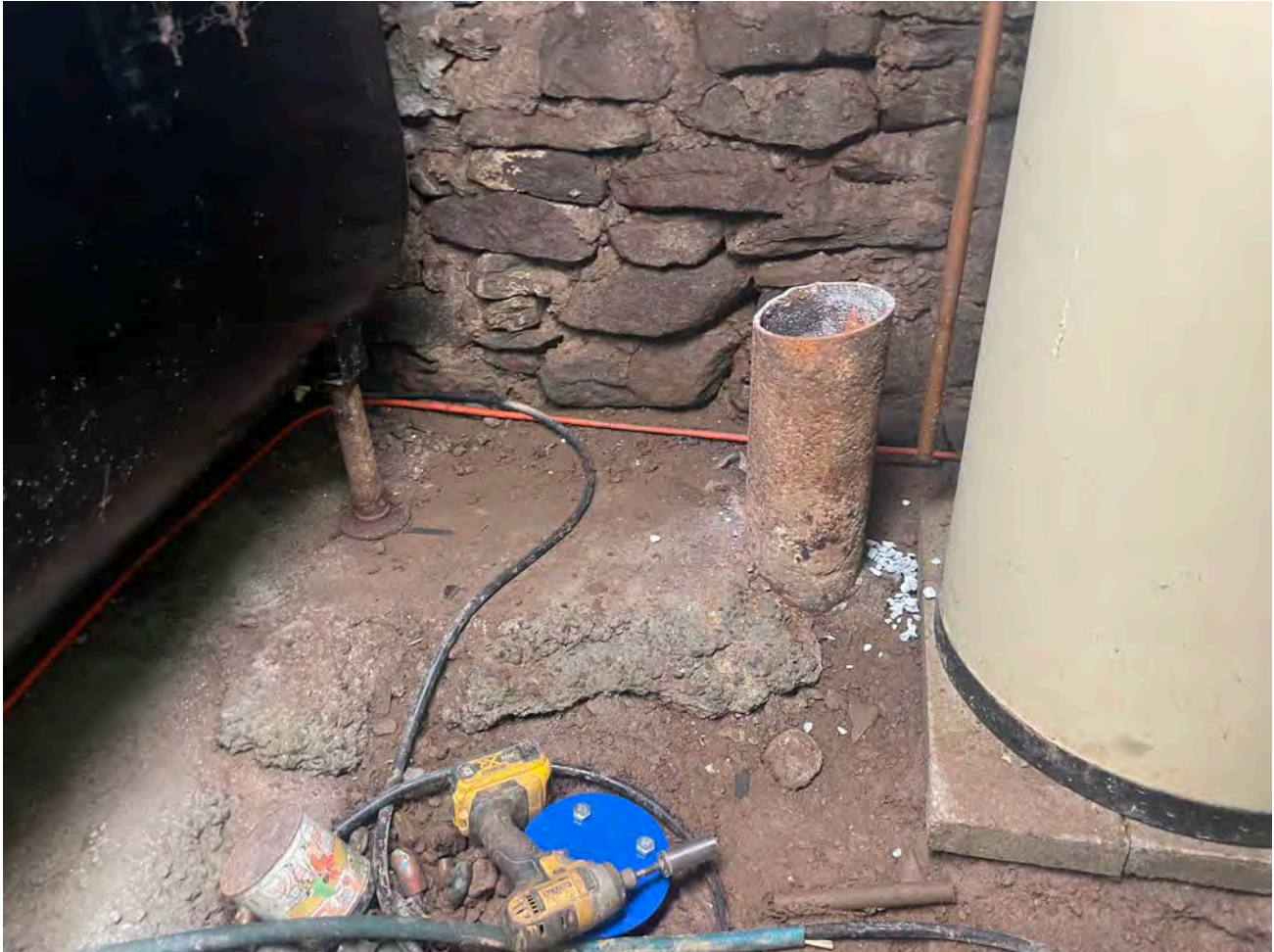
Picture 10: The well located on the north side of the 176 Maple Avenue, Durham, residence where Grela has decommissioned the well by filling it with sand and bentonite chips. View to the north.
