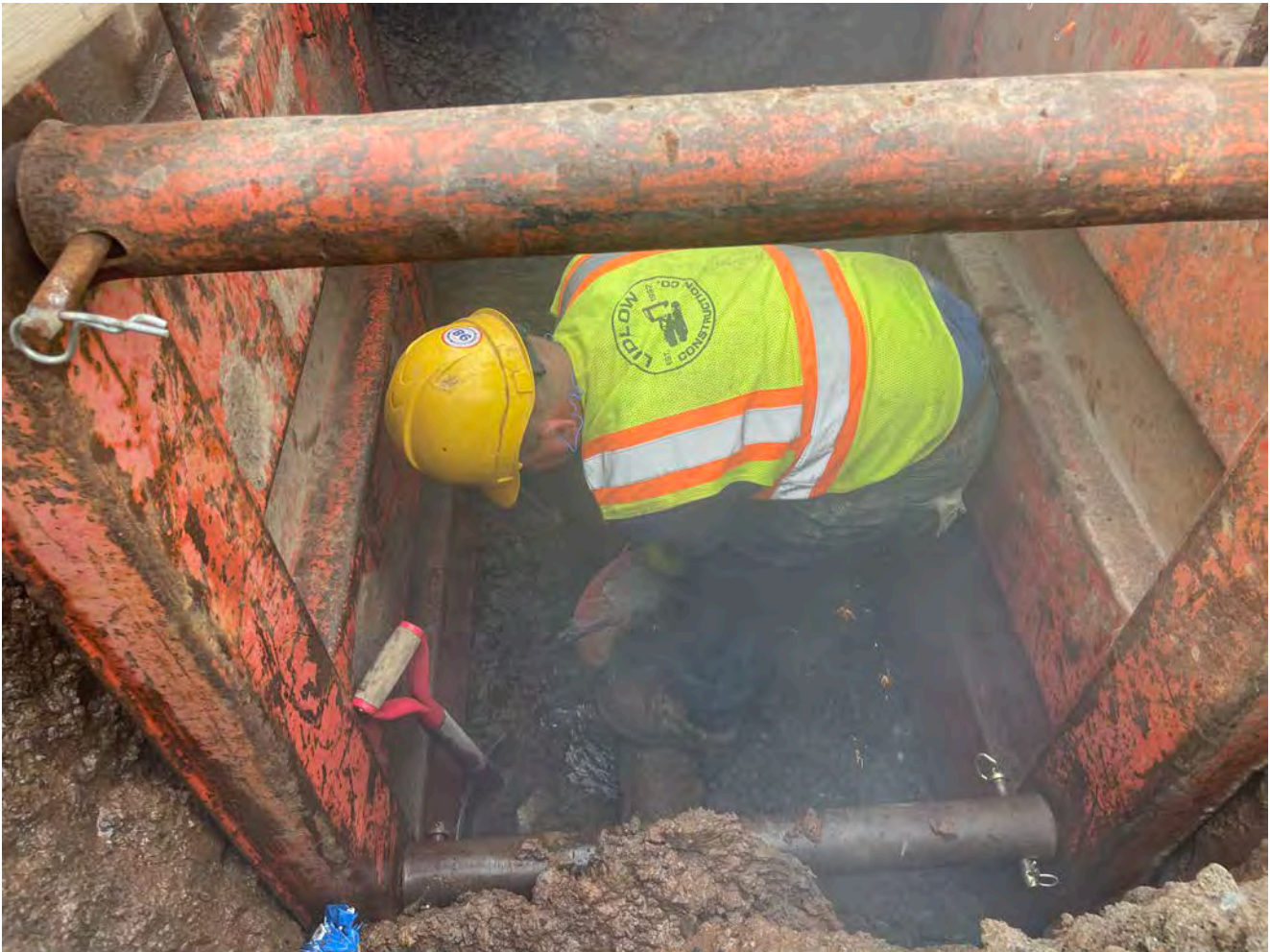
Picture 2: Ludlow using a cutoff saw to remove the 6” DIP water line that fed the hydrant they are removing at Station 604+31 on the south of Watch Hill Drive.
