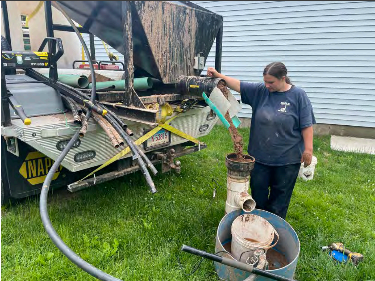
Picture 10: Grela placing sand into the well located on the south side of the 212R Maple Avenue property as part of well decommissioning activities. View to the southeast.
