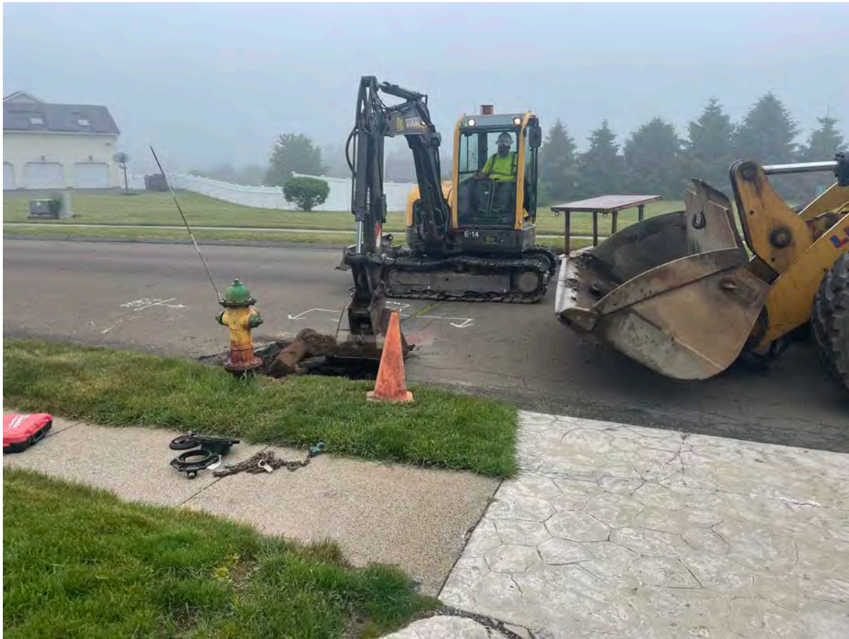
Picture 1: Ludlow excavating to remove the old hydrant located on the south of Watch Hill Drive at Station 604+31. View to the north.
