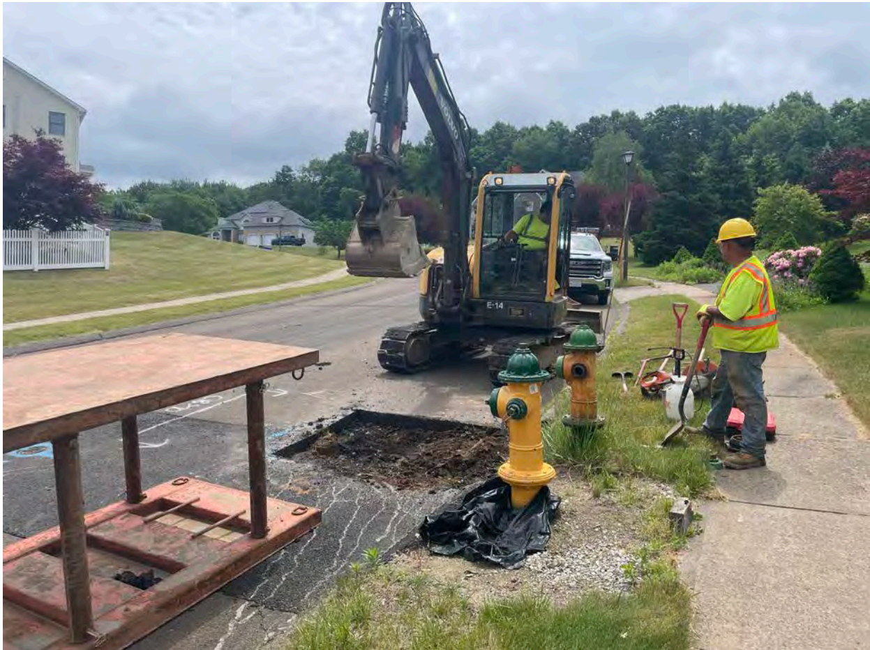
Picture 8: Ludlow excavating to remove an old hydrant at Station 607+12 on Watch Hill Drive in Middletown. View to the south.
