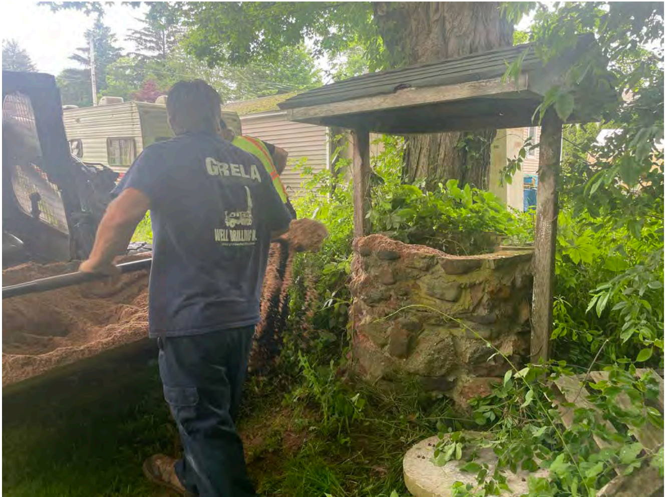
Picture 5: Grela placing sand into the dug well located on the south side of the 176 Maple Avenue property as part of well decommissioning activities. View to the southeast.
