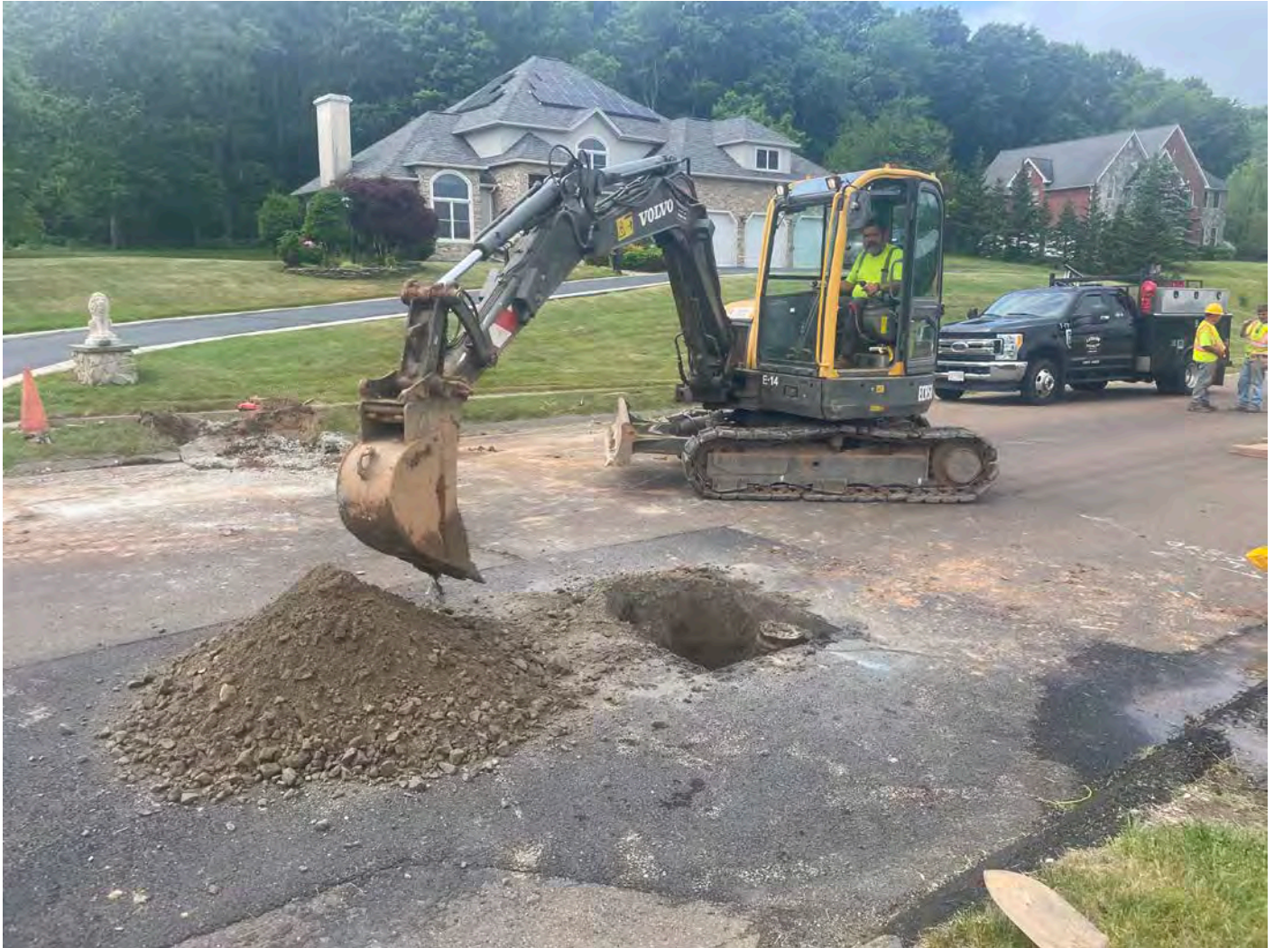
Picture 6: Ludlow excavating to realign a road box on the north side of Watch Hill Drive at Station 604+31. View to the southwest.
