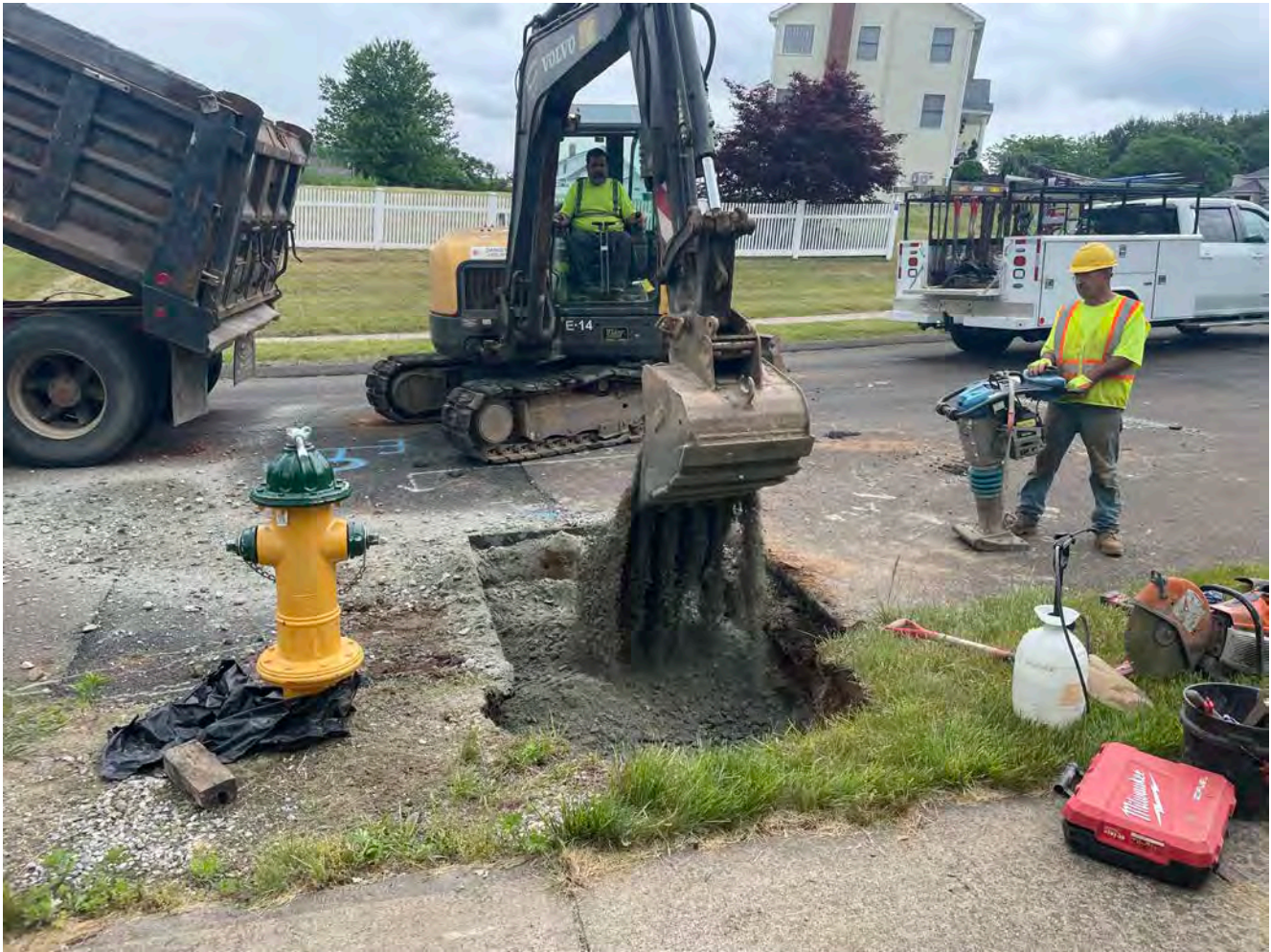
Picture 11: Ludlow backfilling the excavation they made during the removal of a hydrant Station 607+12 on Watch Hill Drive. View to the southeast.
