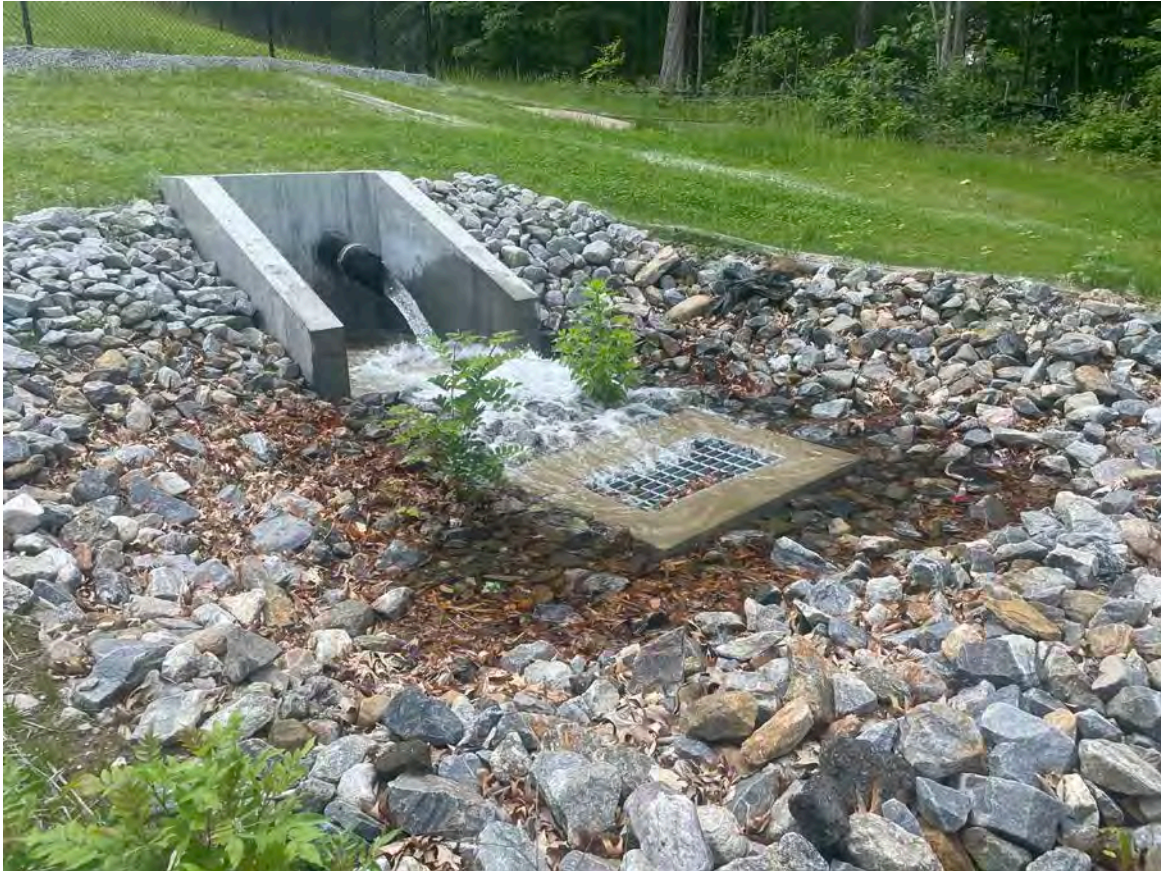
Picture 7: Water exiting the headwall located at Station 11+72 as Ludlow drains the water tank located east of the Shared Access Driveway in Middletown. View to the southeast.
