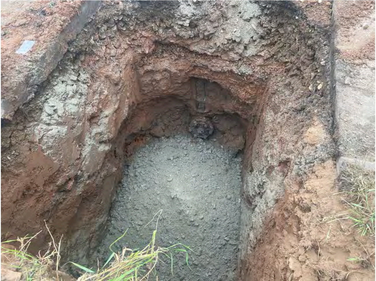
Picture 4: DIP plug that Ludlow placed on the gate valve located at Station 604+31 on Watch Hill Drive in Middletown. View to the north.
