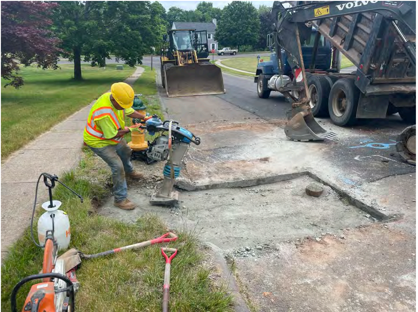
Picture 12: Ludlow backfilling the excavation they made during the removal of a hydrant Station 607+12 on Watch Hill Drive. View to the north.
