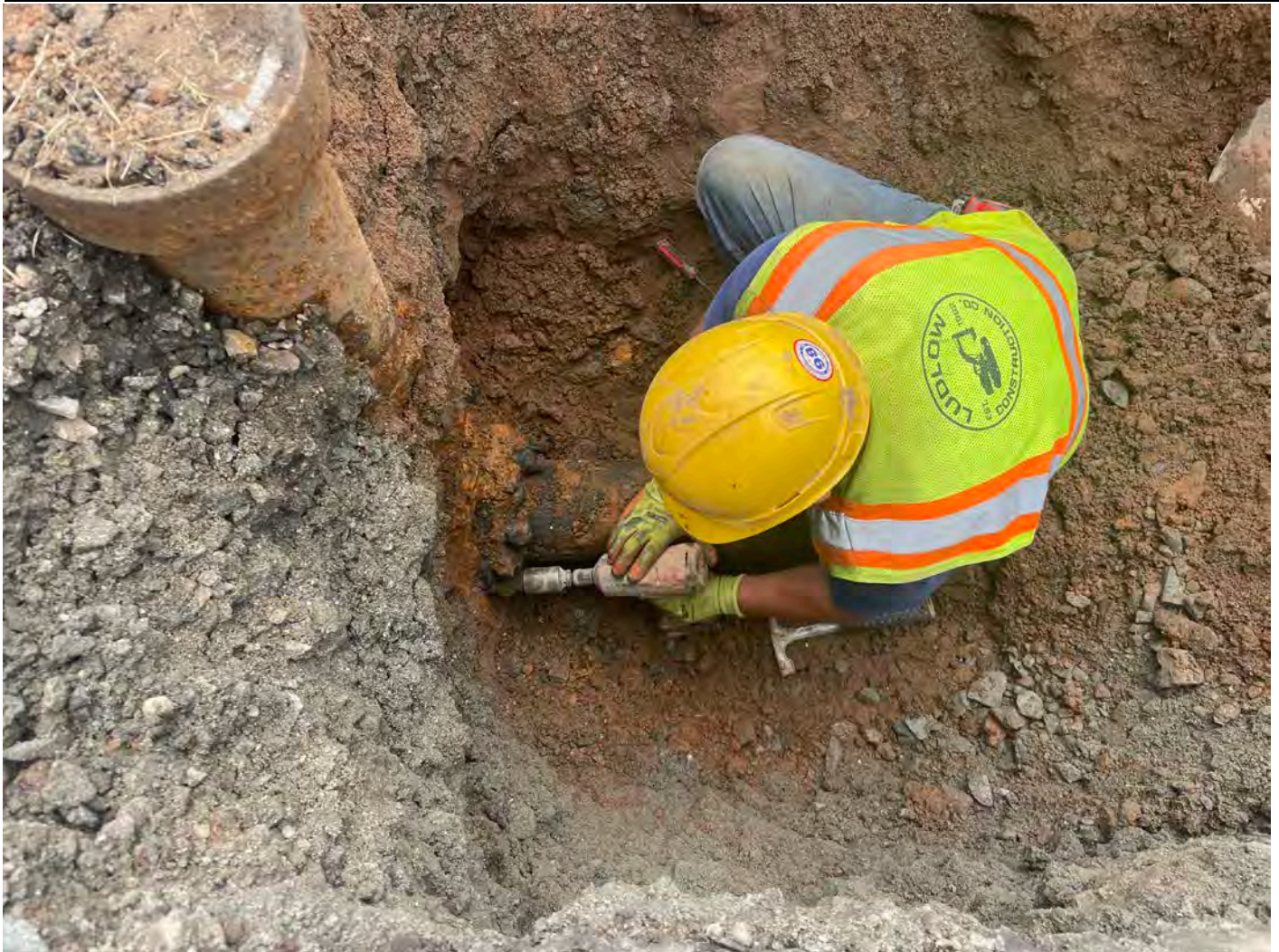
Picture 9: Ludlow unbolting a section of 6" DIP from a gate valve located at Station 607+12 as they continue to decommission the old hydrant located at the same station. View to the south.
