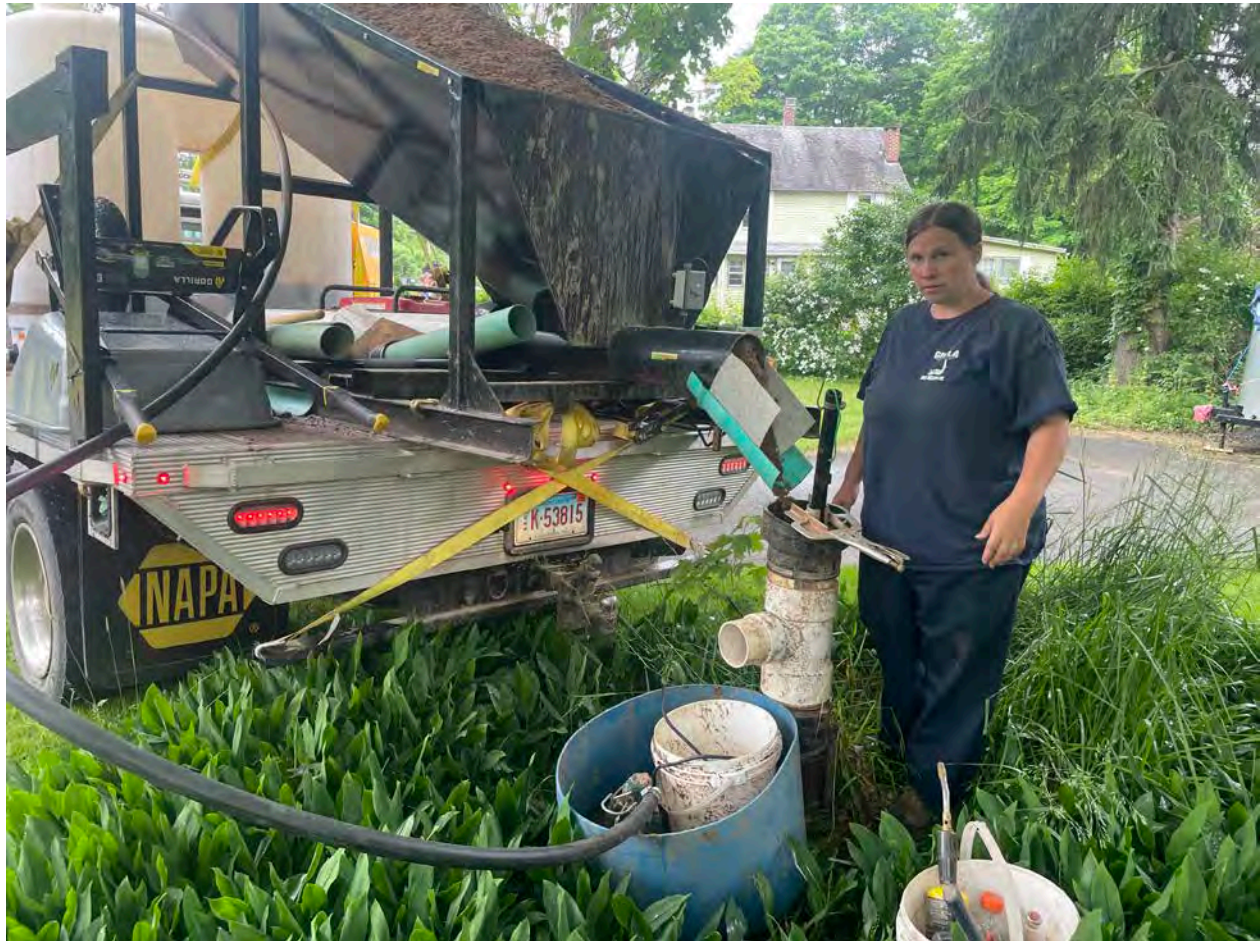
Picture 3: Grela placing sand into the well located on the east side of the 184 Maple Avenue property as part of well decommissioning activities. View to the southwest.
