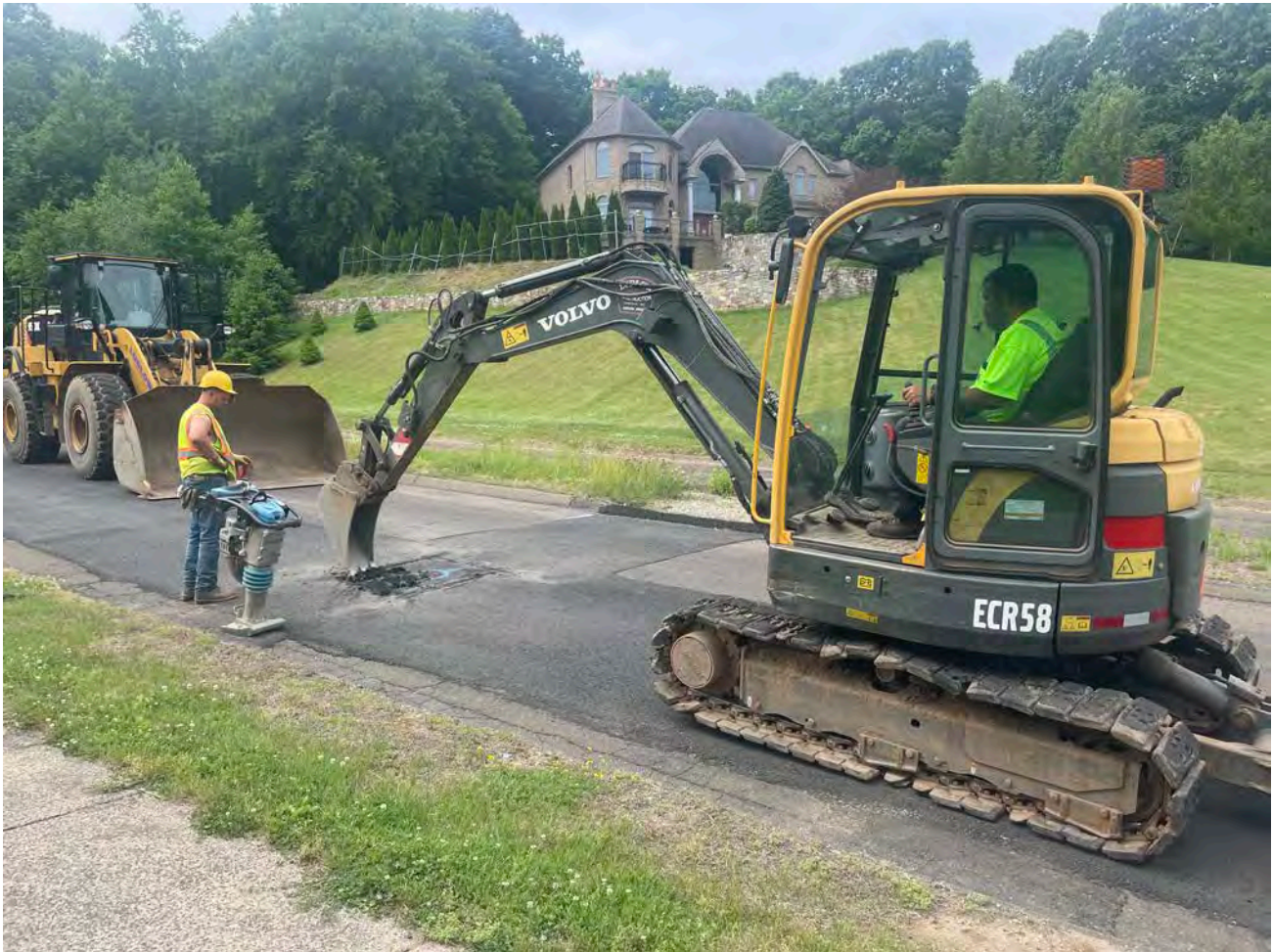
Picture 4: Ludlow excavating at Station 31+81 on Talcott Ridge Drive to realign a roadbox . View to the southeast.
