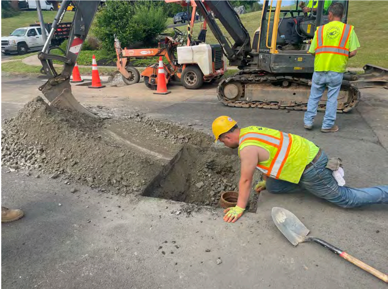
Picture 3: Ludlow working to realign a roadbox at Station 36+42 on Talcott Ridge Drive. View to the west.
