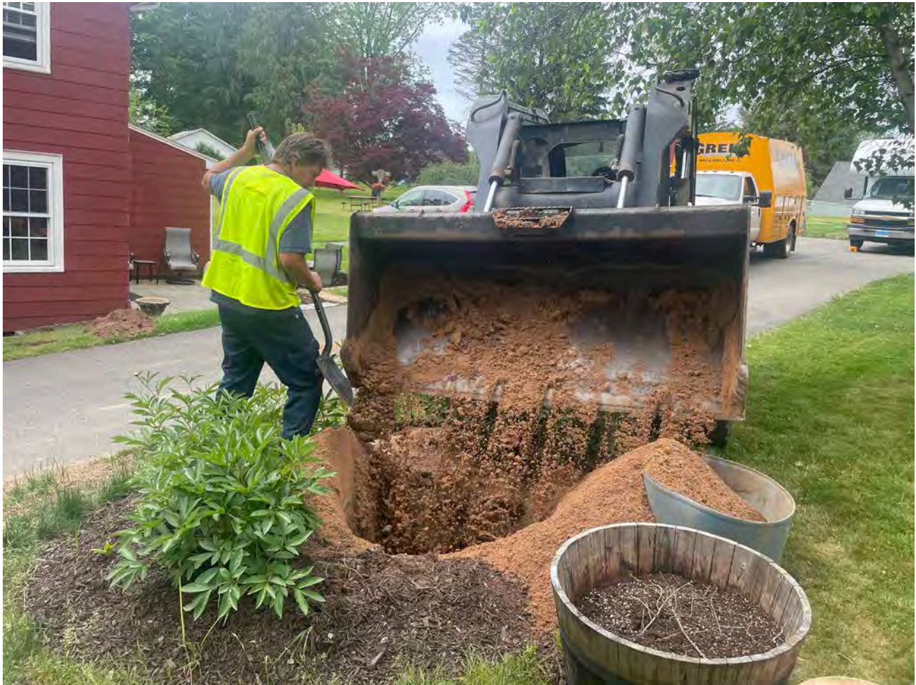
Picture 5: Grela placing sand into the well located on the property boundary of the 186 and 188 Main Street, Durham, properties as part of well decommissioning activities. View to the west.
