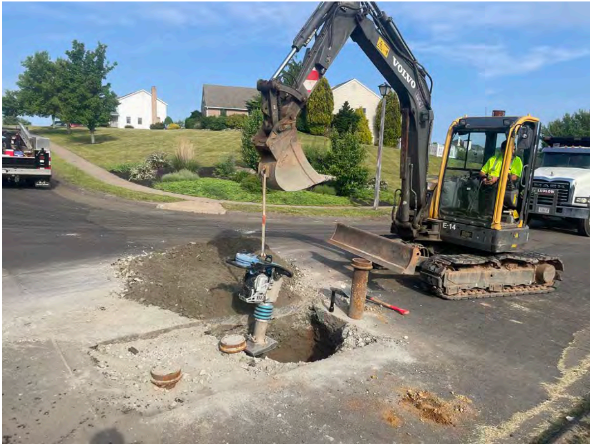
Picture 1: Ludlow working at Station 35+74 on Talcott Ridge Drive where they realigned a roadbox. View to the west.
