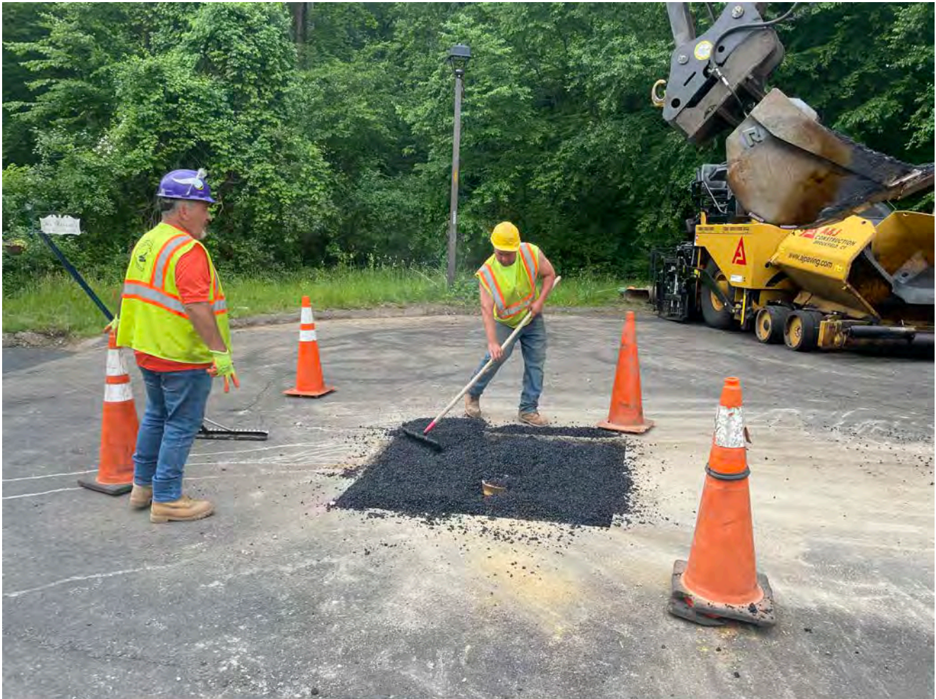
Picture 11: Ludlow placing asphalt over the backfilled excavation they made in order to realign the roadbox located at Station 23+05. View to the west.
