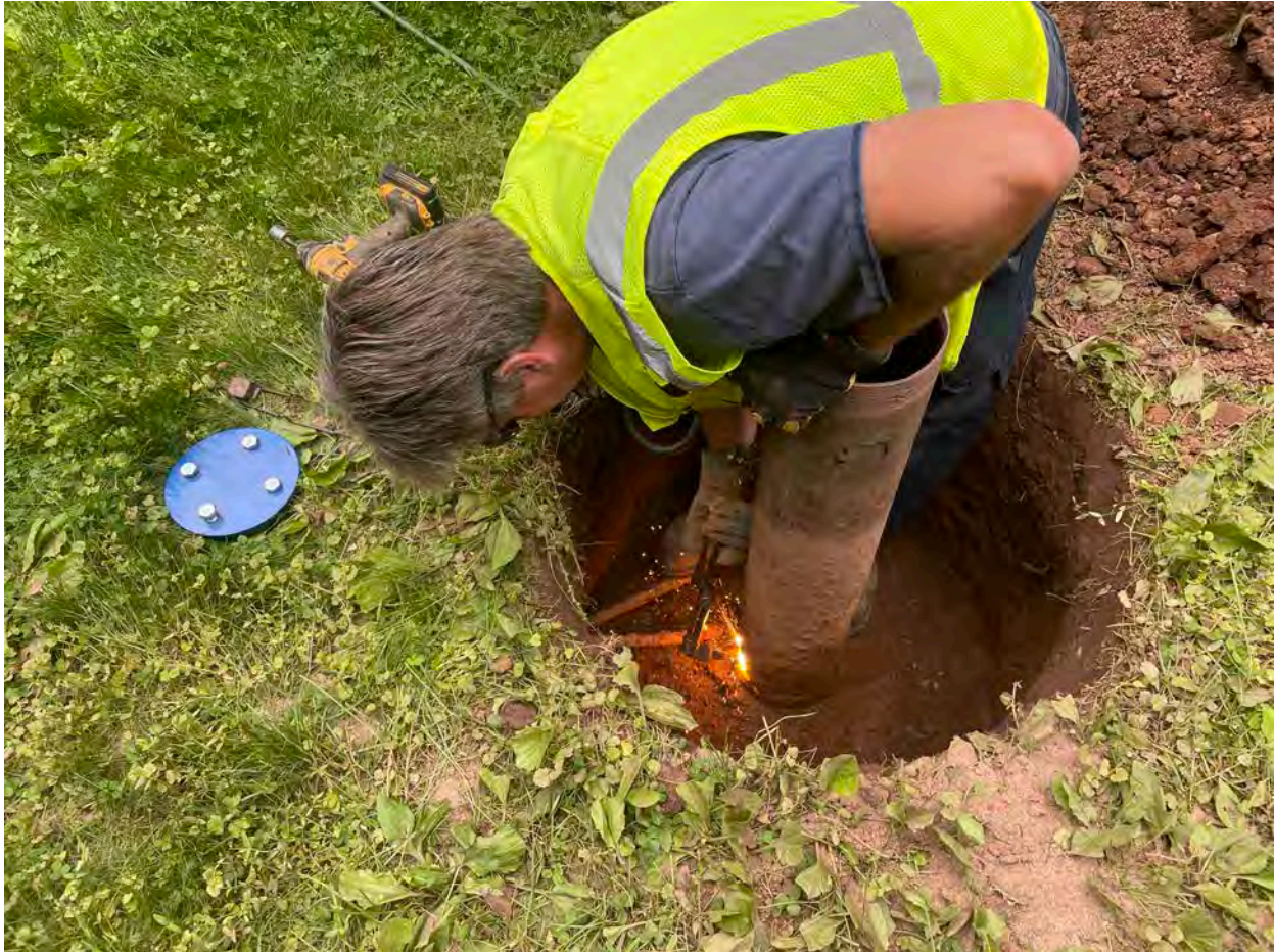
Picture 8: Grela cutting the well casing of the well located on the west side of the 120 Main Street, Durham, property as part of well decommissioning activities.
