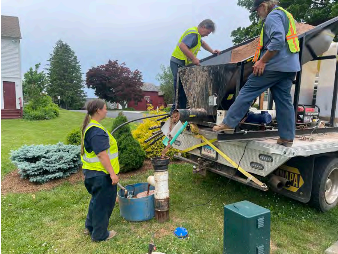
Picture 7: Grela placing sand into the eastern-most well located on the 38 Town House Road, Durham, property as part of well decommissioning activities. View to the northwest.
