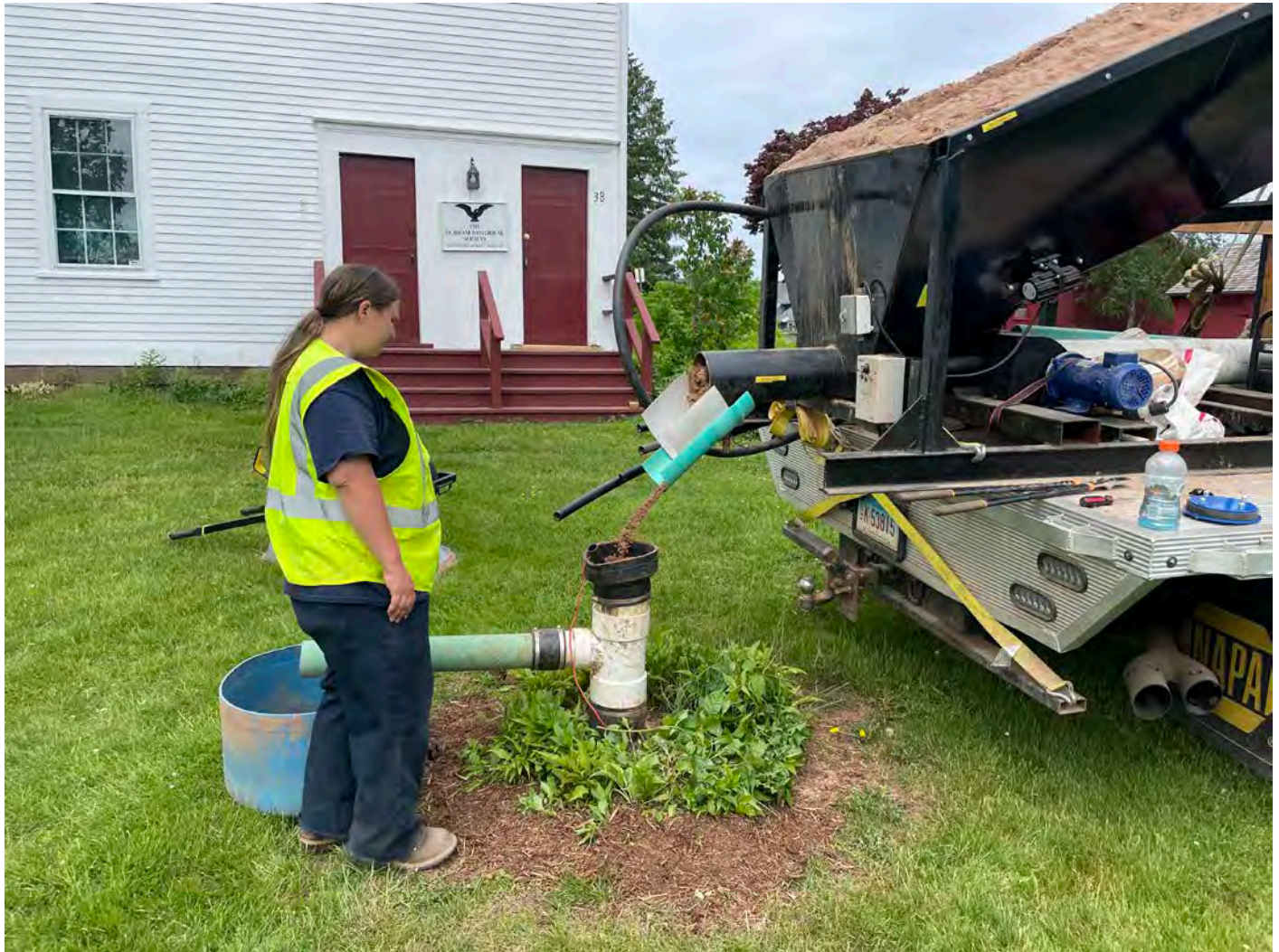
Picture 6: Grela placing sand into the western-most well located on the 38 Town House Road, Durham, property as part of well decommissioning activities. View to the west.
