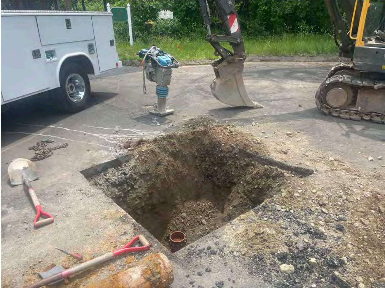
Picture 10: Roadbox located at Station 23+05 that Ludlow is in the process of realigning. View to the northwest.
