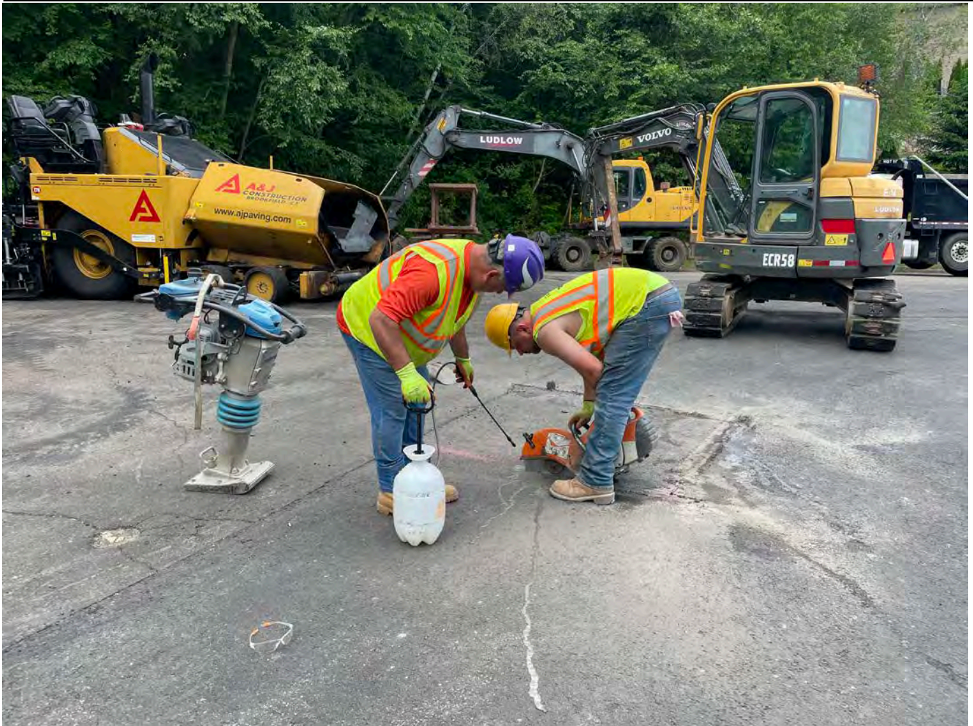
Picture 9: Ludlow saw-cutting pavement around the roadbox located at Station 23+05 that they are about to realign. View to the northwest.
