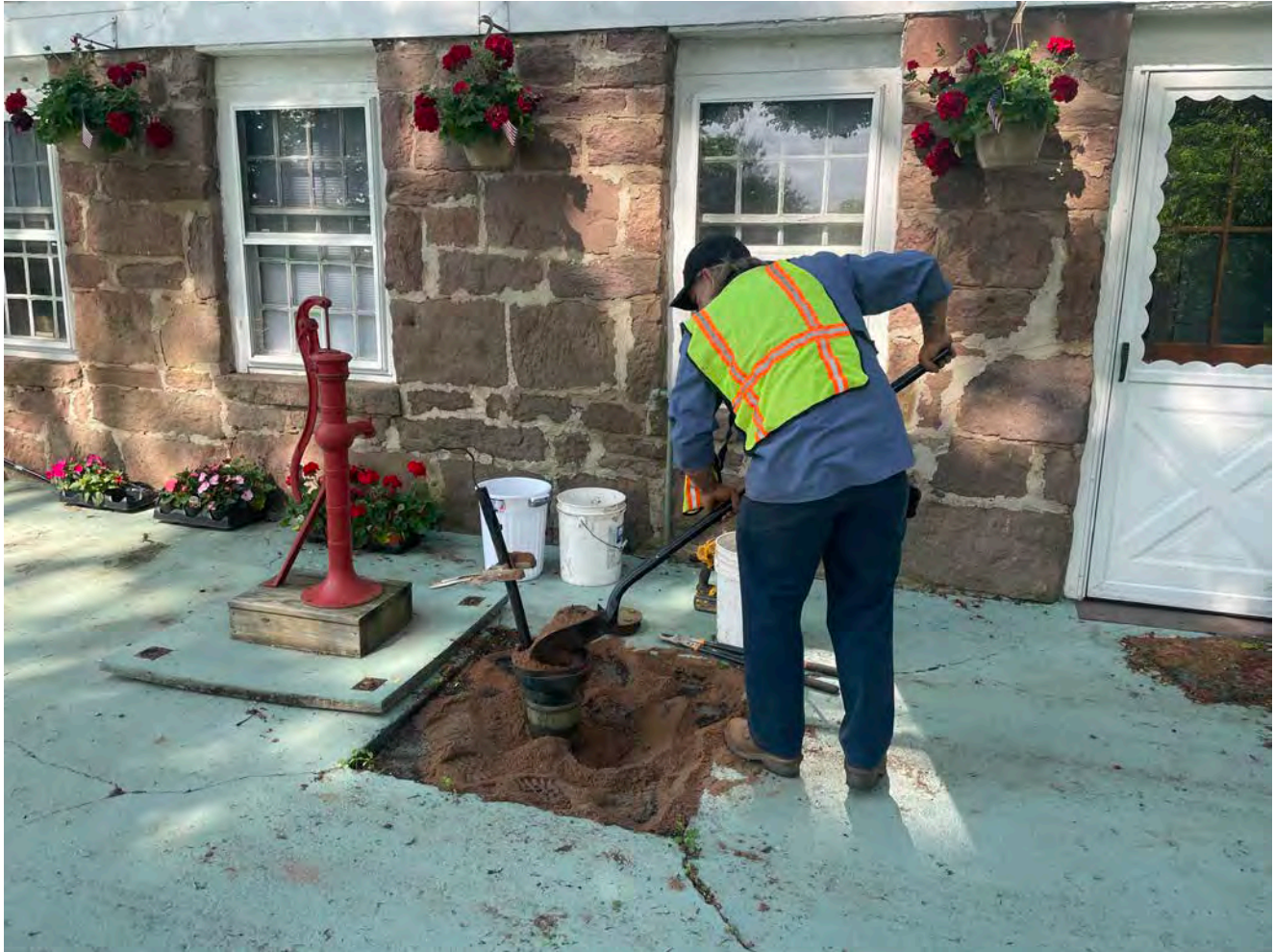
Picture 2: Grela placing sand into the well located on the east side of the 215 Main Street, Durham, residence as part of well decommissioning activities. View to the southwest.
