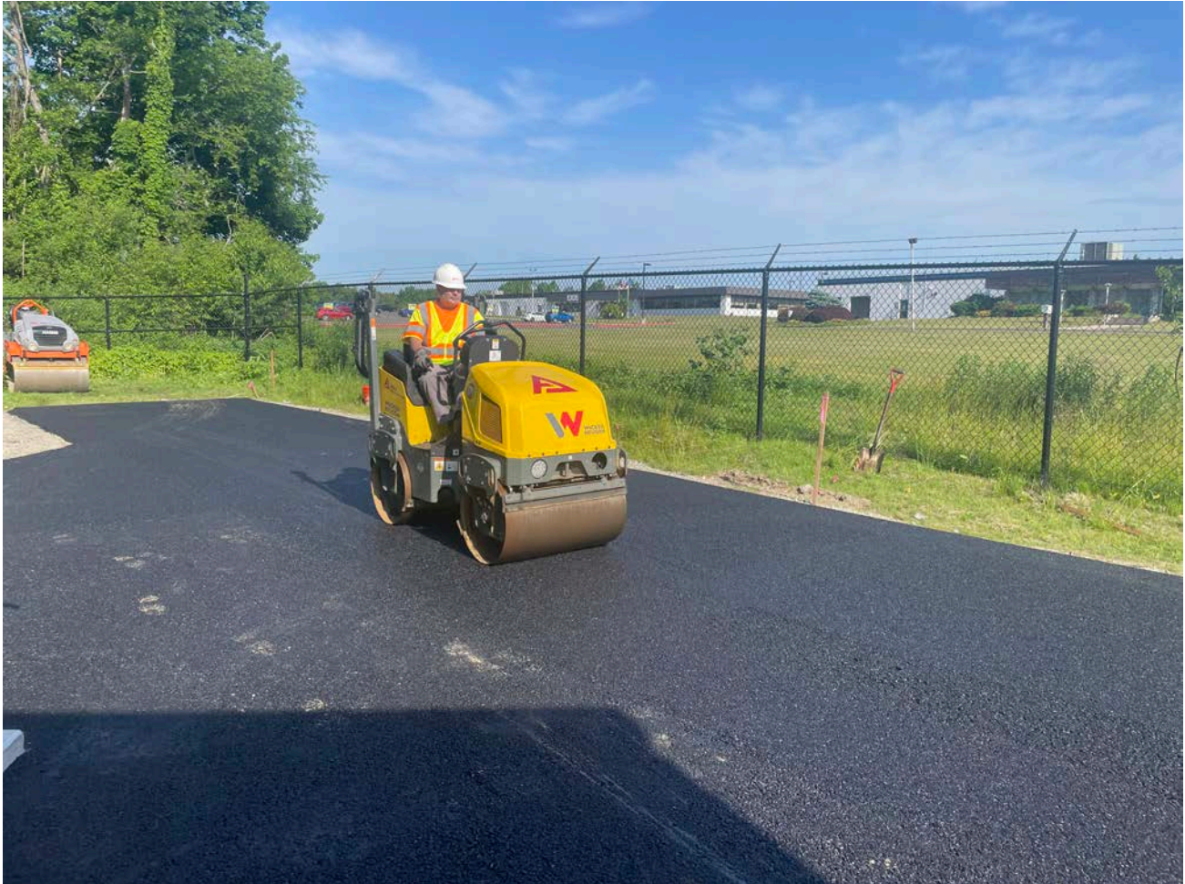
Picture 4: A&J Construction compacting the first lift of asphalt they placed at the Booster Station located on S. Main Street in Middletown. View to the west.
