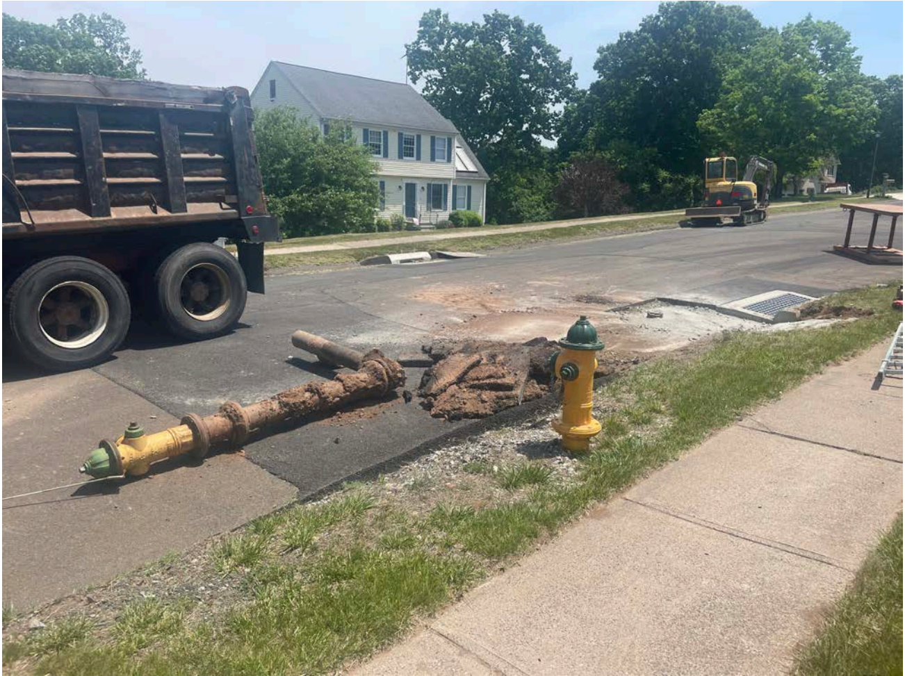
Picture 10: Station 36+28 where Ludlow removed an existing hydrant and cut and capped the 6" DIP water line that fed the hydrant. View to the east.
