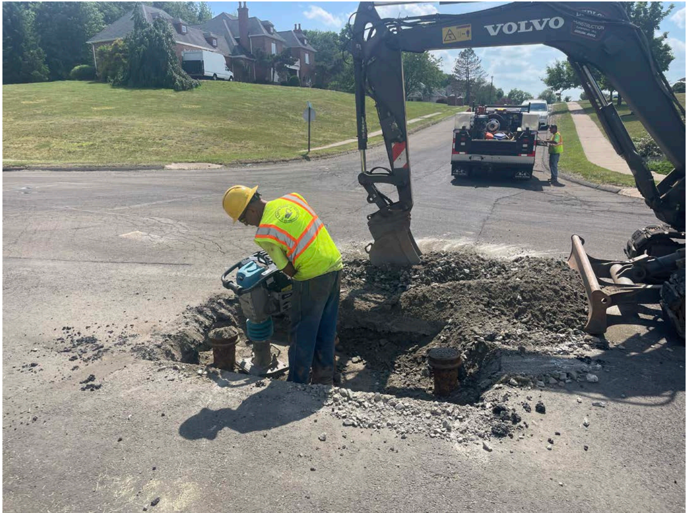
Picture 12: Ludlow backfilling around three roadboxes located at Station ~35+60 that they realigned. View to the south.
