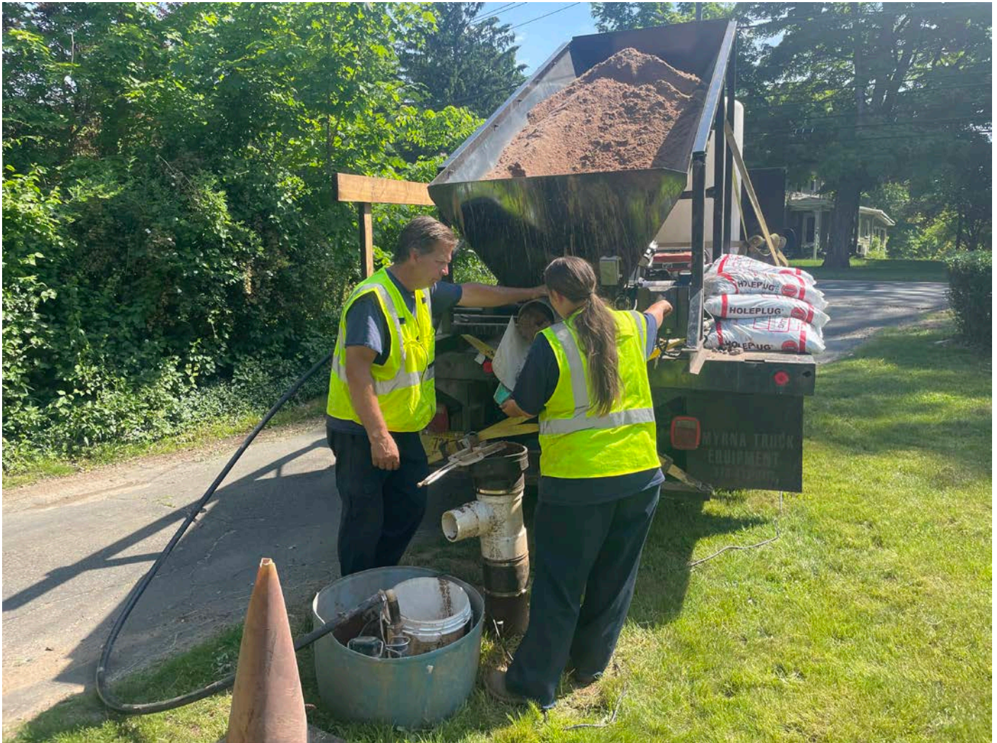
Picture 6: Grela placing sand into the well located on the east side of the 298 Main Street, Durham, residence as part of well decommissioning activities. View to the east.
