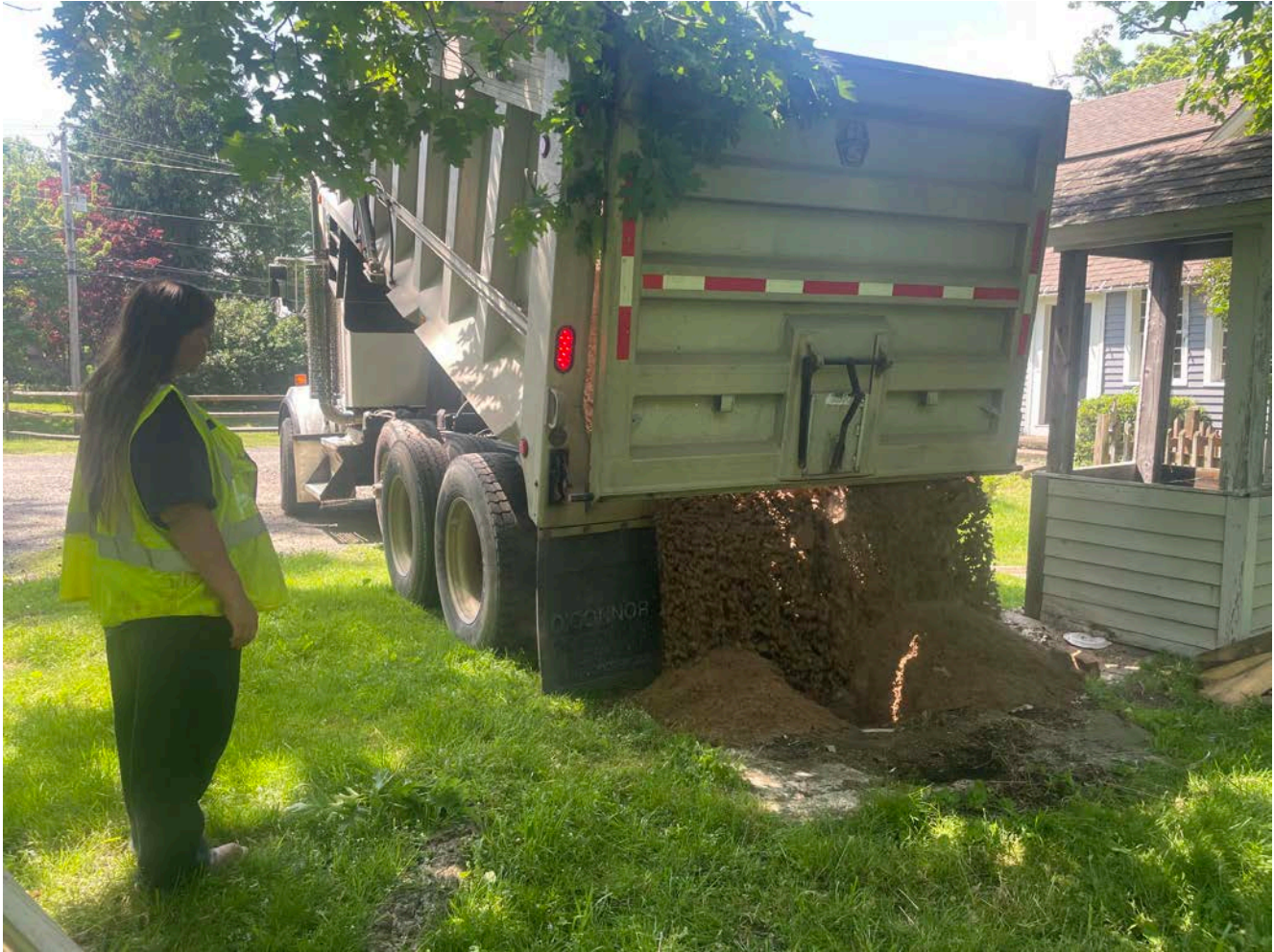
Picture 11: Grela placing sand into the dug well located on the south side of the 119 Main Street, Durham, residence as part of well decommissioning activities. View to the west.
