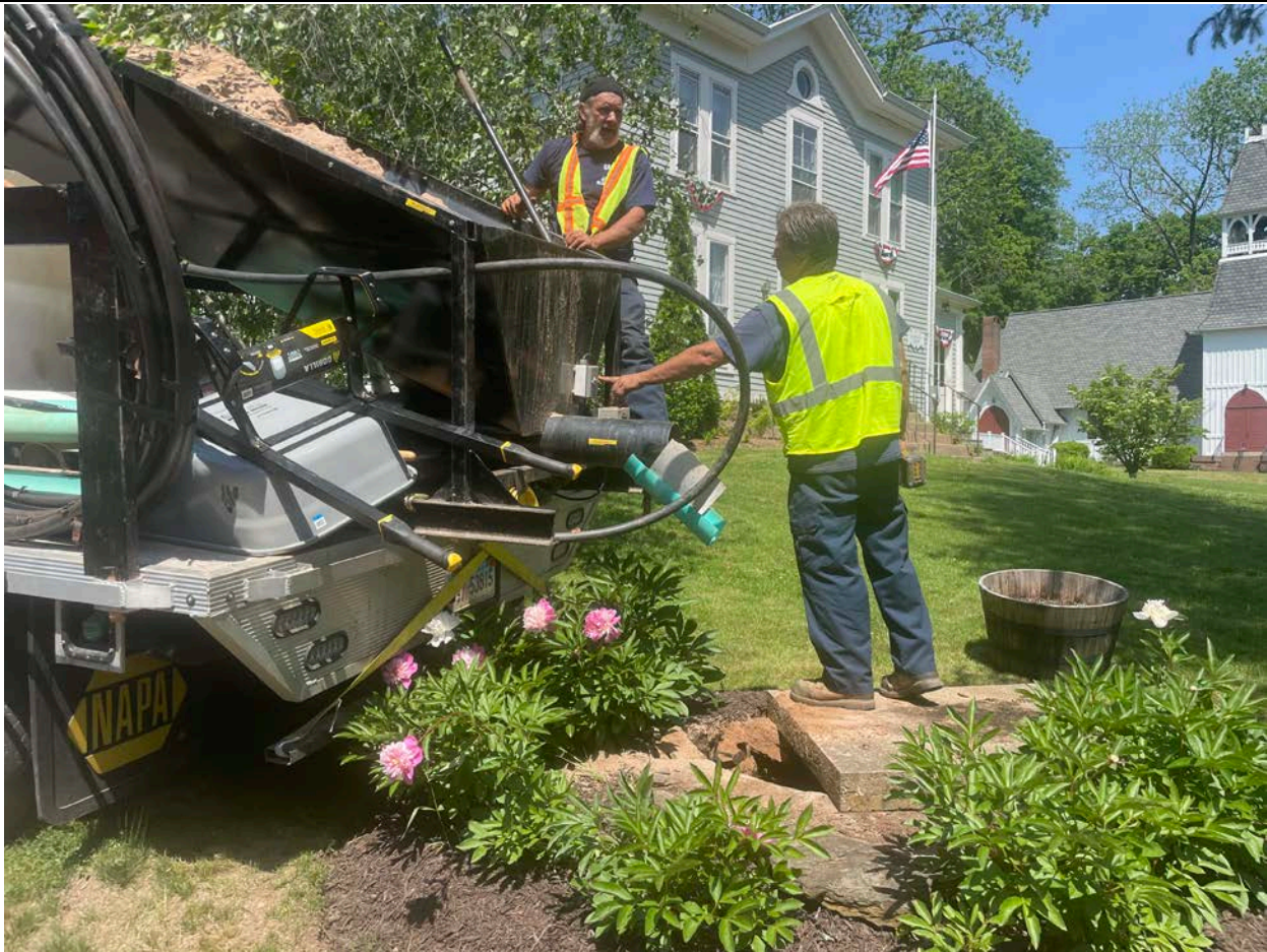
Picture 8: Grela placing sand into the dug well located on the border of the 186 and 188 Main Street, Durham, properties as part of well decommissioning activities. View to the north.
