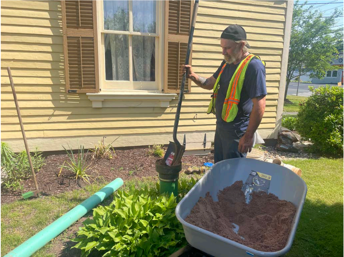
Picture 5: Grela placing sand into the well located on the south side of the 322 Main Street, Durham, residence as part of well decommissioning activities. View to the northeast.
