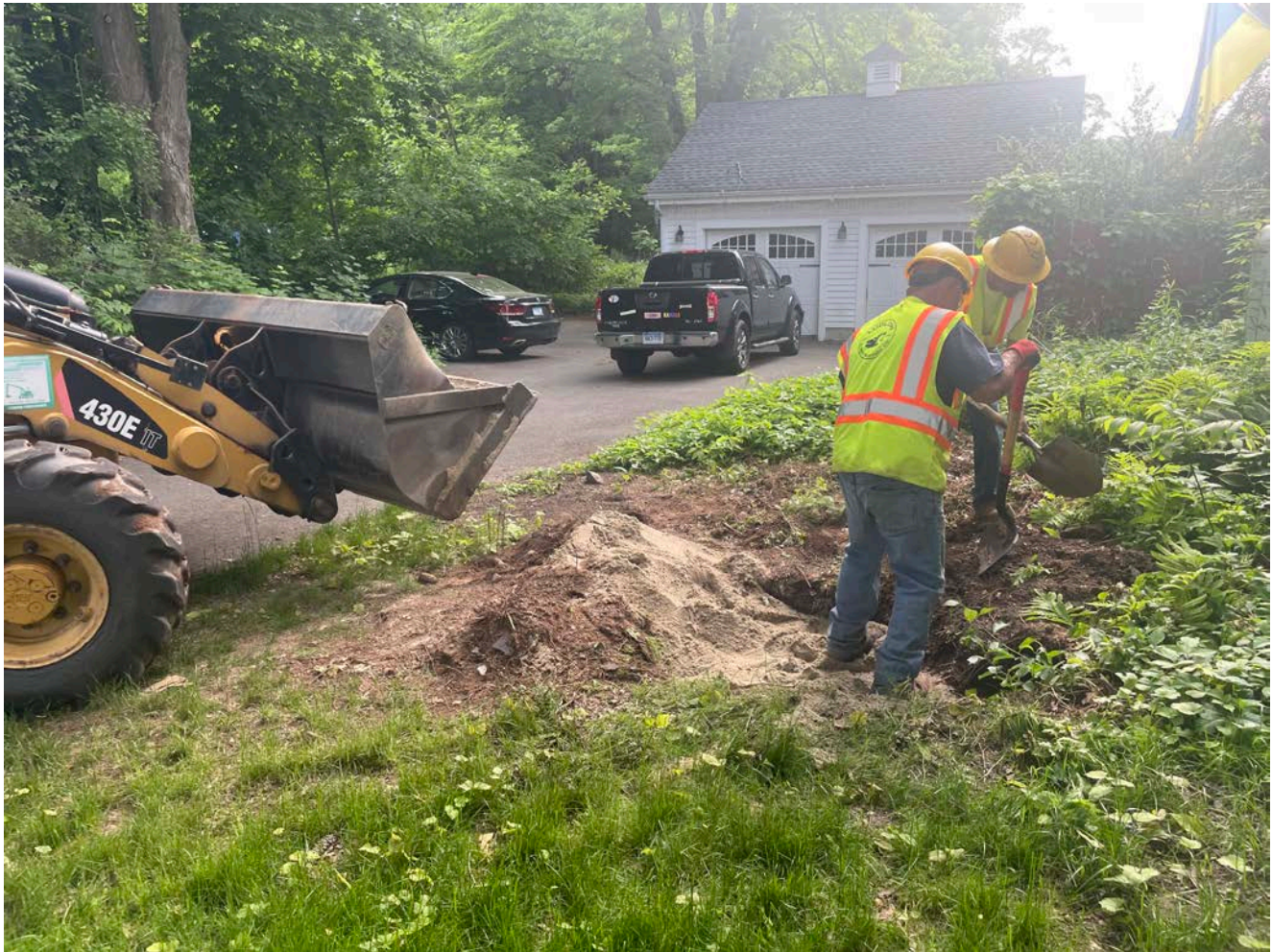
Picture 2: Ludlow backfilling over the well located on the north side of the 313 Main Street residence that was decommissioned by Grela. View to the east.
