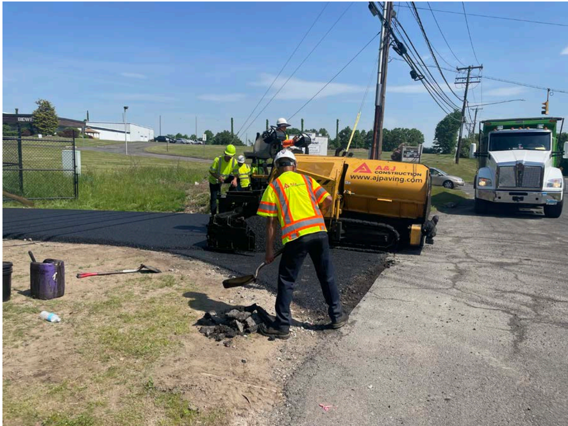
Picture 7: A&J Construction placing a second lift of asphalt on the driveway footprint of the Booster Station where it meets the west edge of S. Main Street. View to the north.
