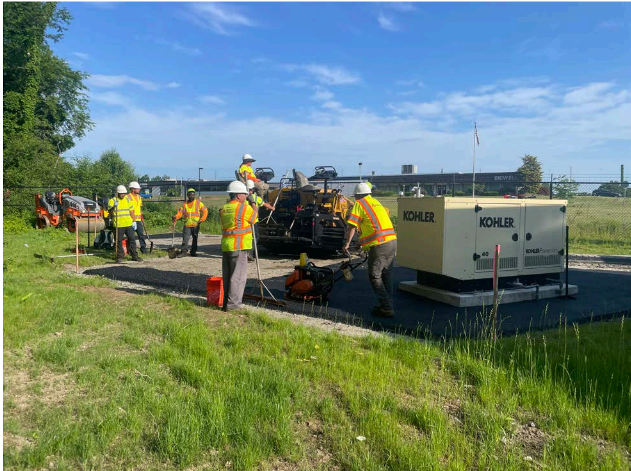
Picture 3: A&J Construction placing a first lift of asphalt around the generator located on the west side of the Booster Station. View to the northwest.
