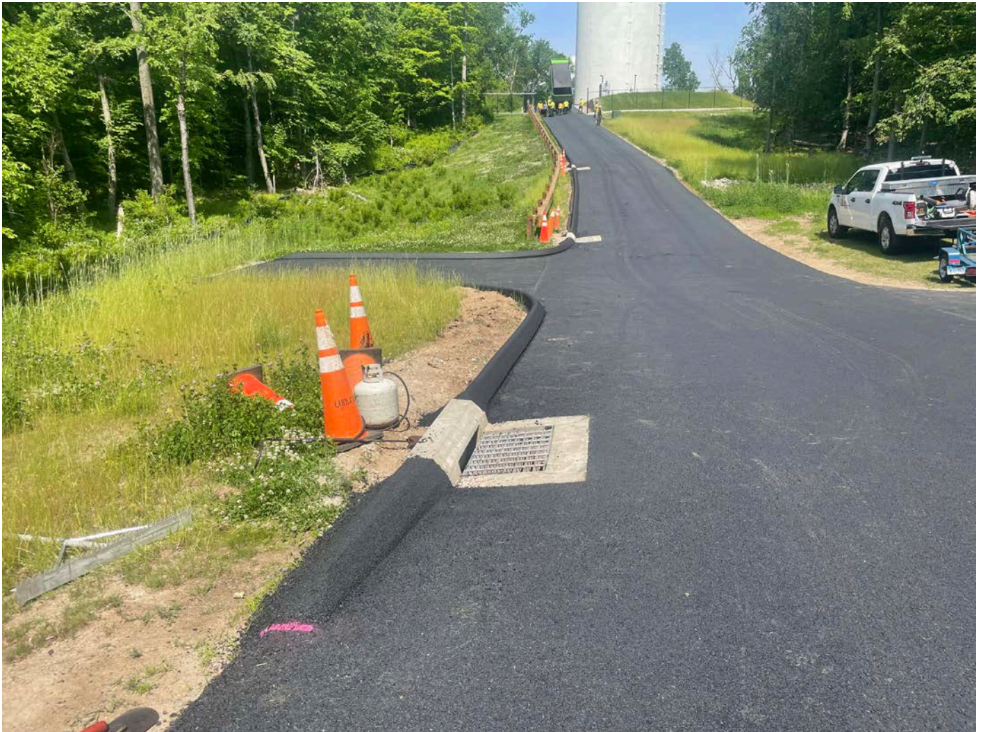
Picture 13: Asphalt curbing that A&J Construction placed on the north side of the Shared Access Driveway in Middletown. View to the east.
