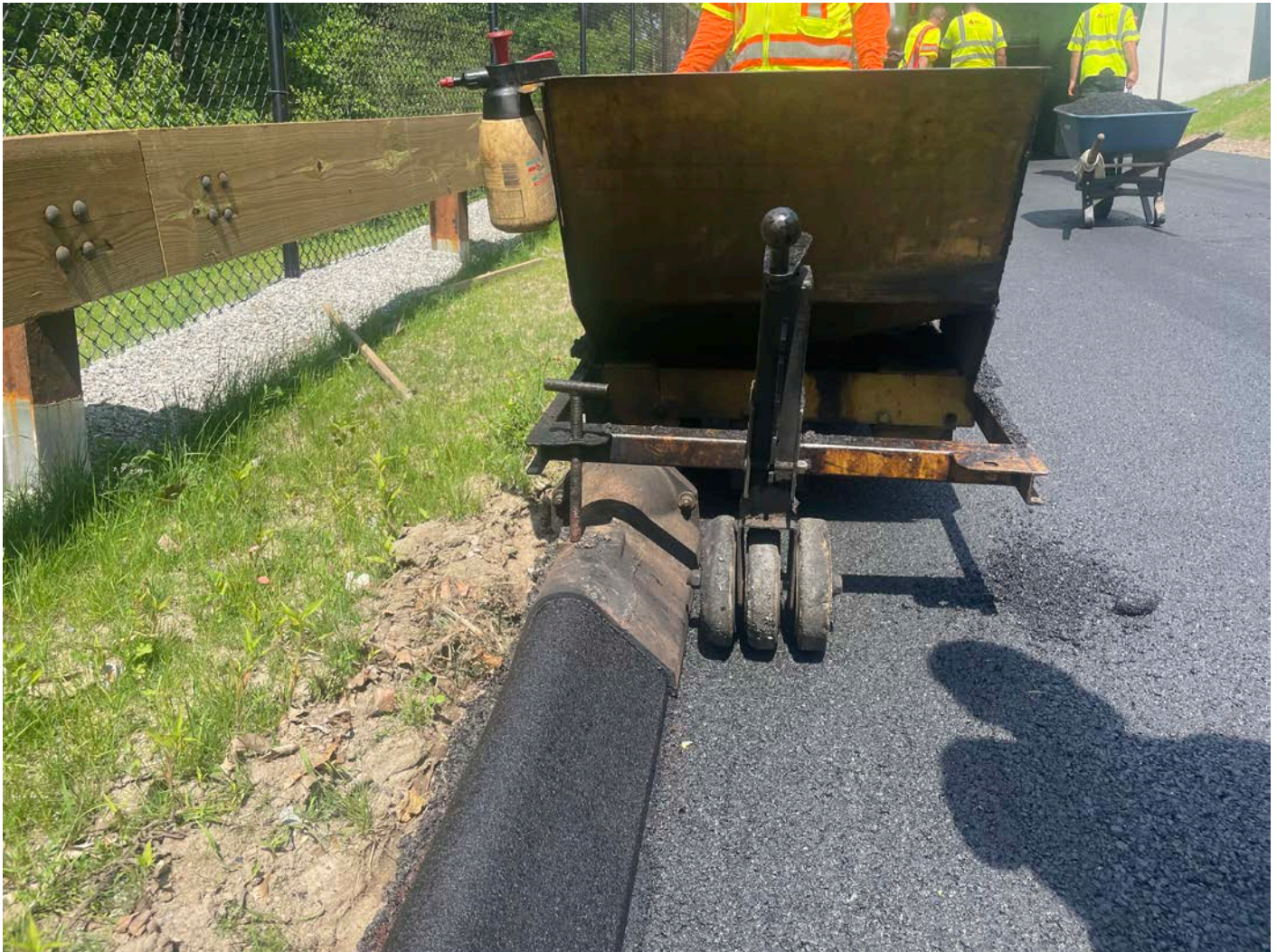
Picture 14: Asphalt curbing that A&J Construction is placing on the north side of the Shared Access Driveway in Middletown. View to the east.
