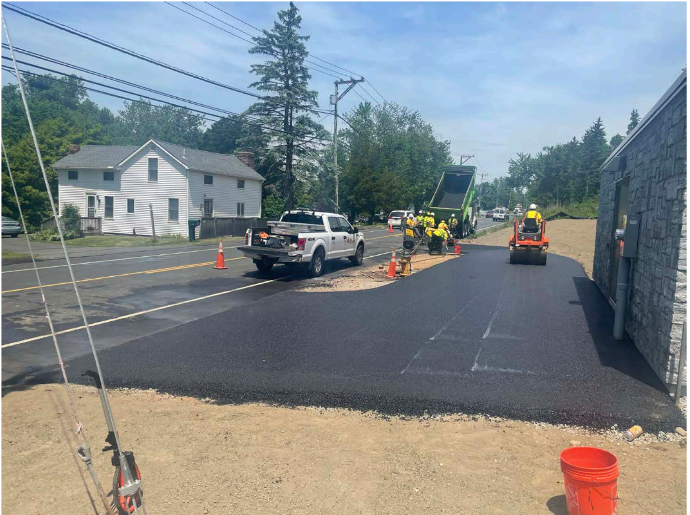
Picture 9: A&J Construction placing a second lift of asphalt on the driveway footprint of the Water Meter Building on S. Main Street, Middletown. View to the north.
