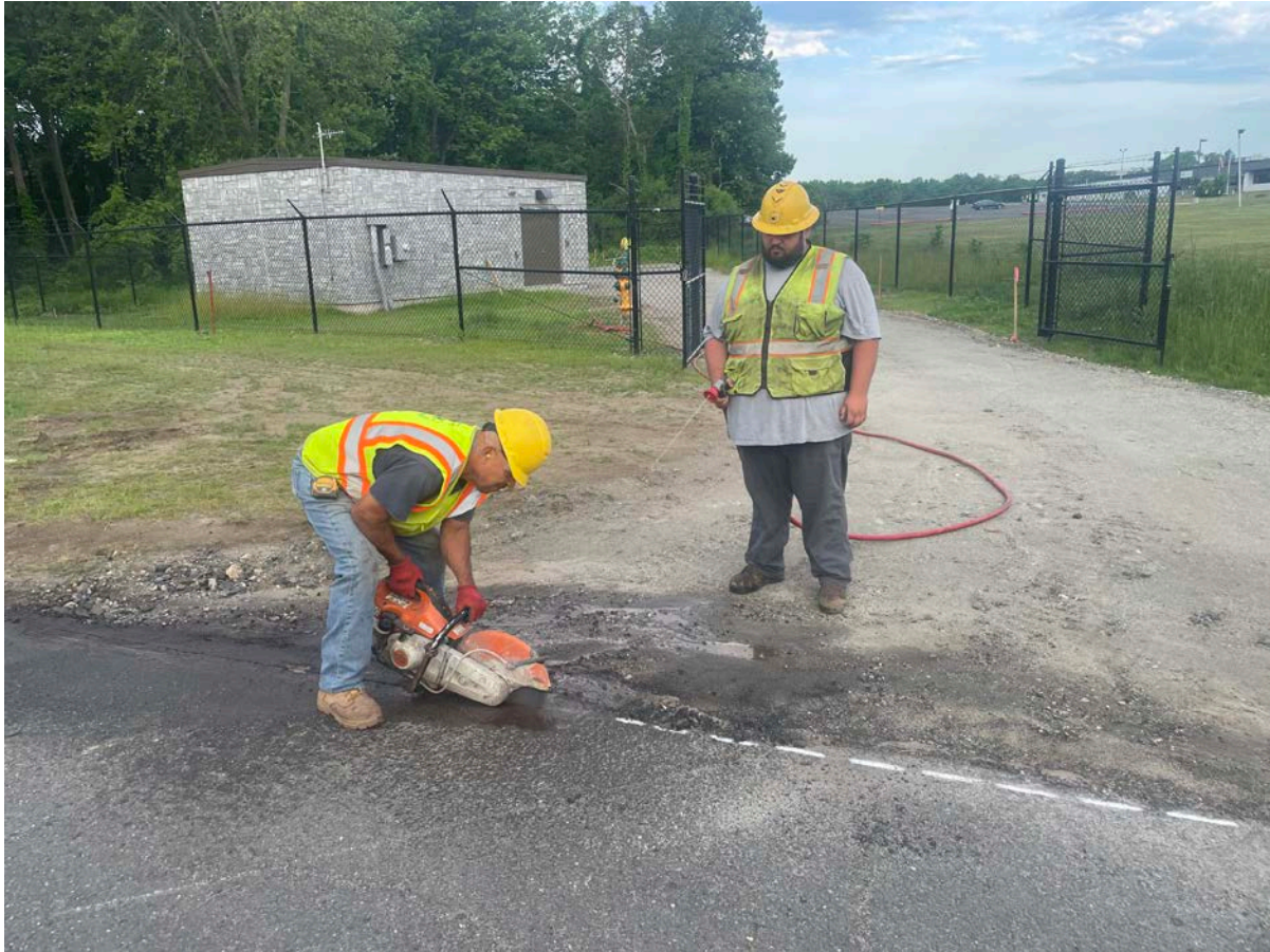
Picture 1: Ludlow saw-cutting the west side of S. Main Street. Middletown where it meets the driveway entrance to the Booster Station. View to the west.
